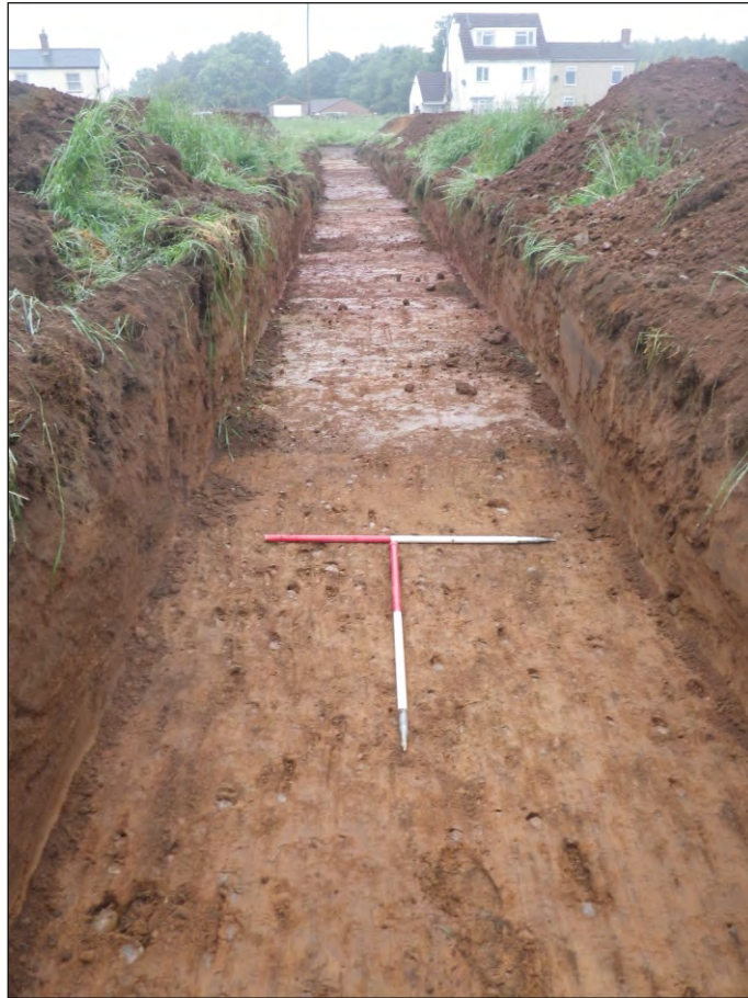
Plate 5: Trench 2 view from the south
