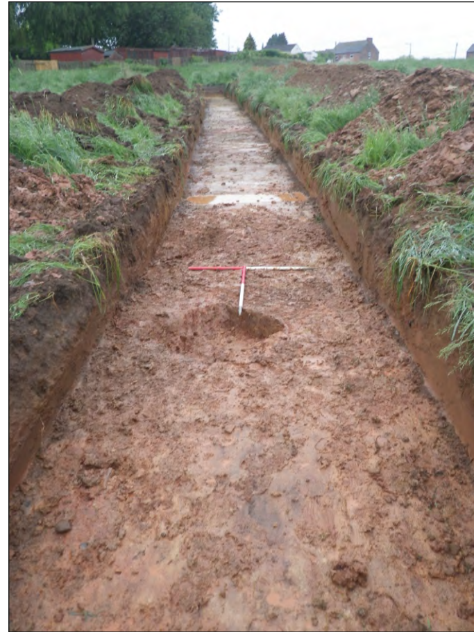
Plate 12: Trench 6 view from the south-east
