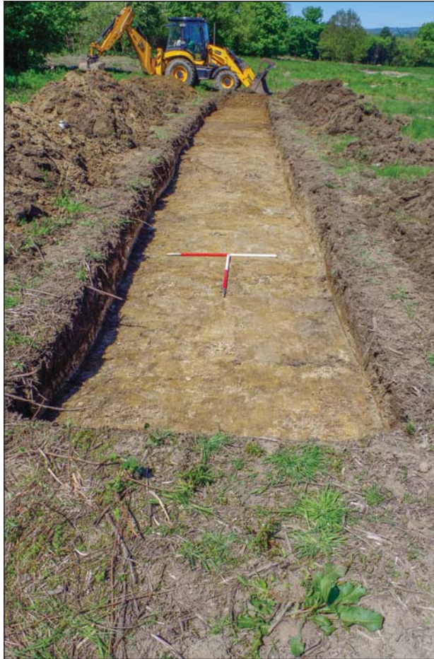
Plate 5: Trench 8, view from south-east
