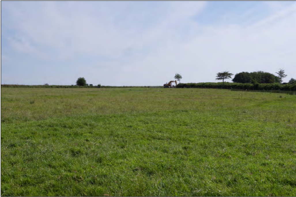
Plate 20: General view of earthworks from south, Turbine 2
