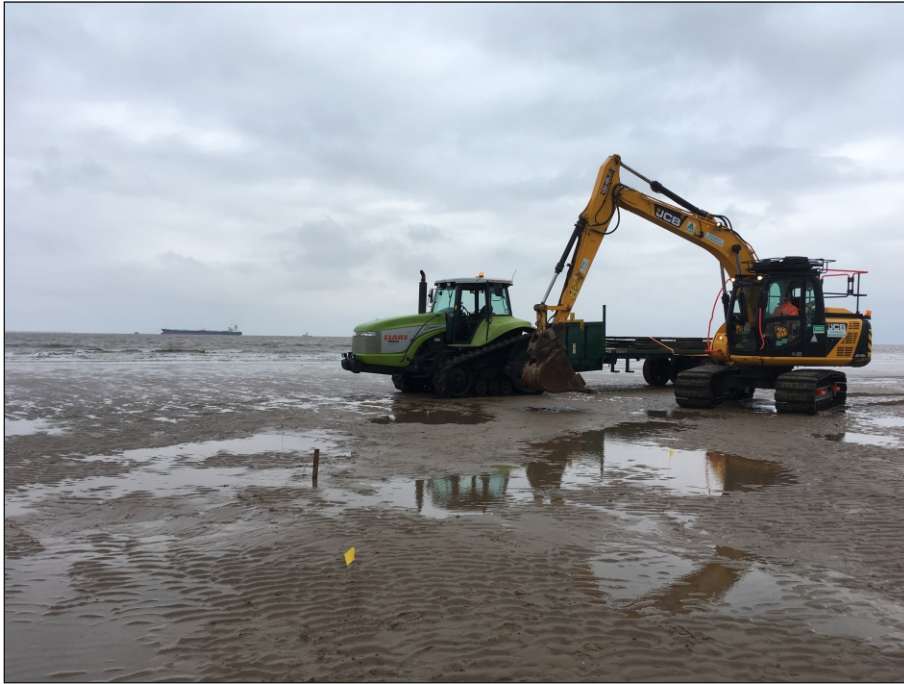
Plate 1: View of trench facing north-east
