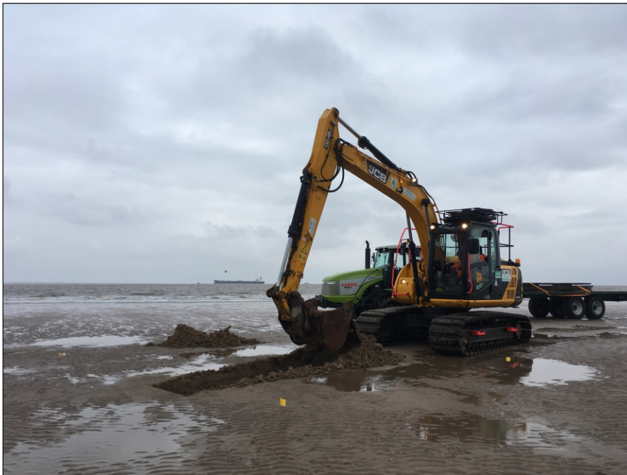
Plate 2: View of trench facing north
