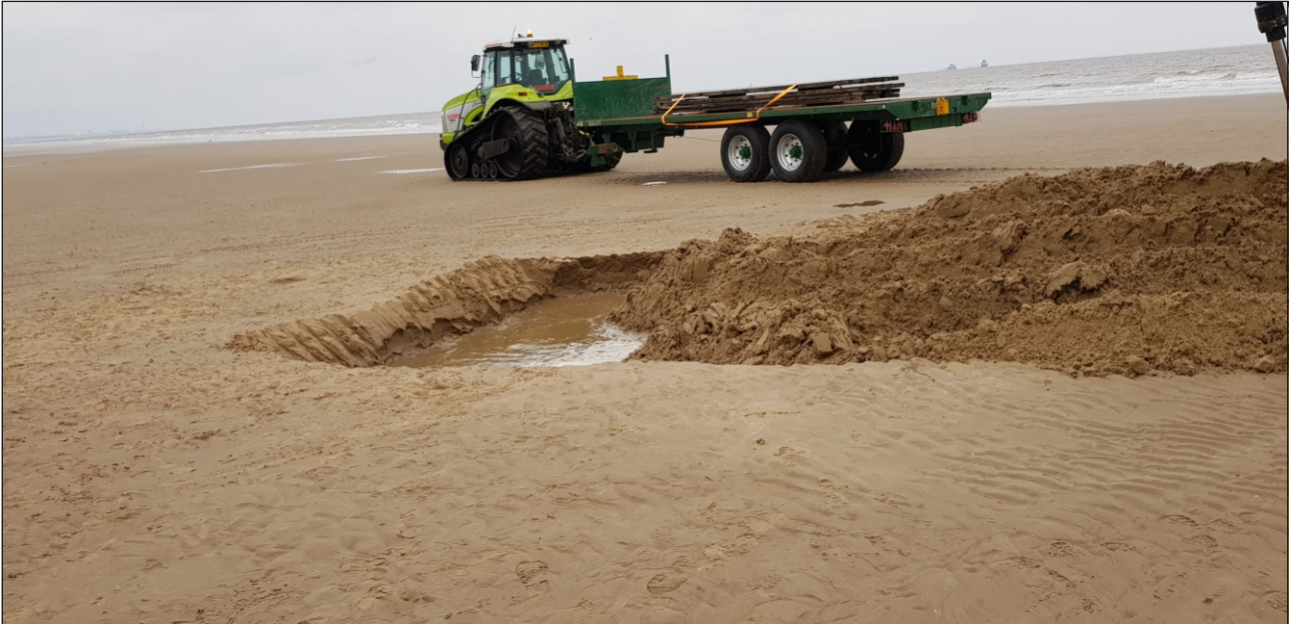
Plate 3: View of partially back filled trench facing north-west
