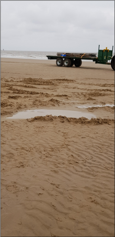
Plate 4: View of backfilled trench facing north-west
