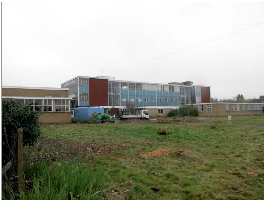
Plate 2: Hucclecote Centre viewed from the north-west
