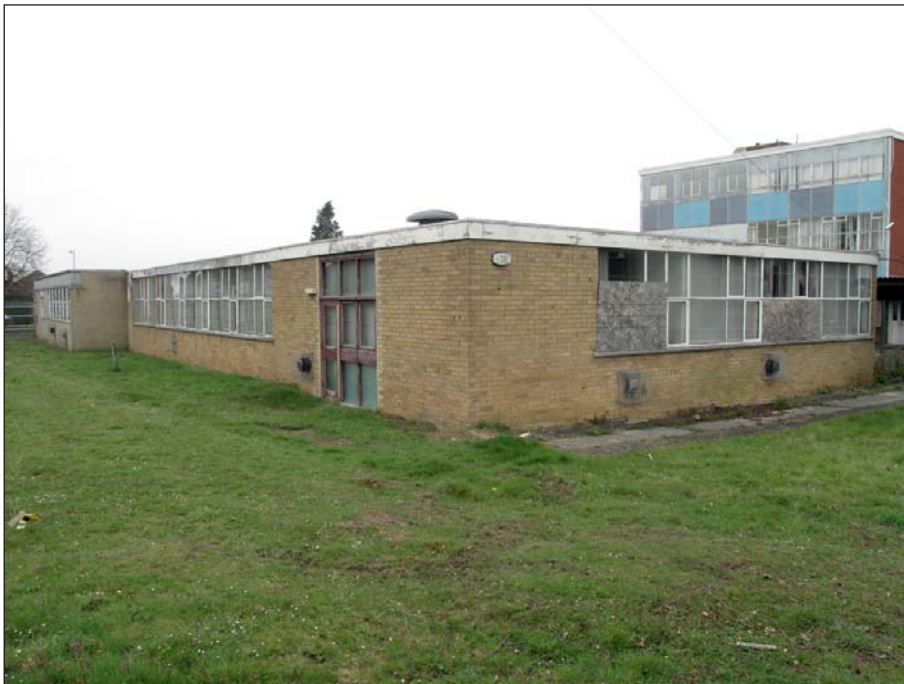
Plate 12: Large detached building to the south
