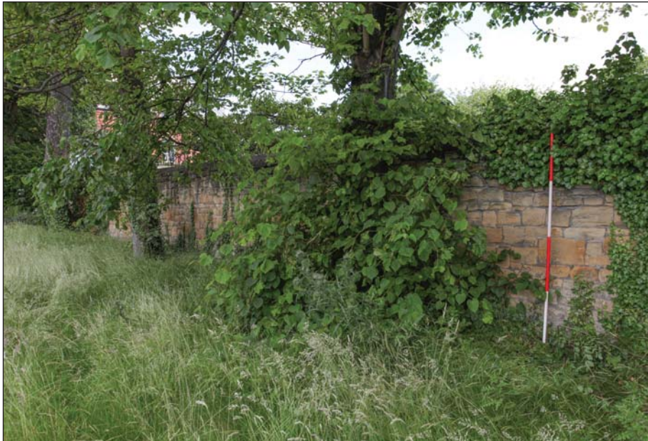
Plate 22: General view of the west face of wall, section E
