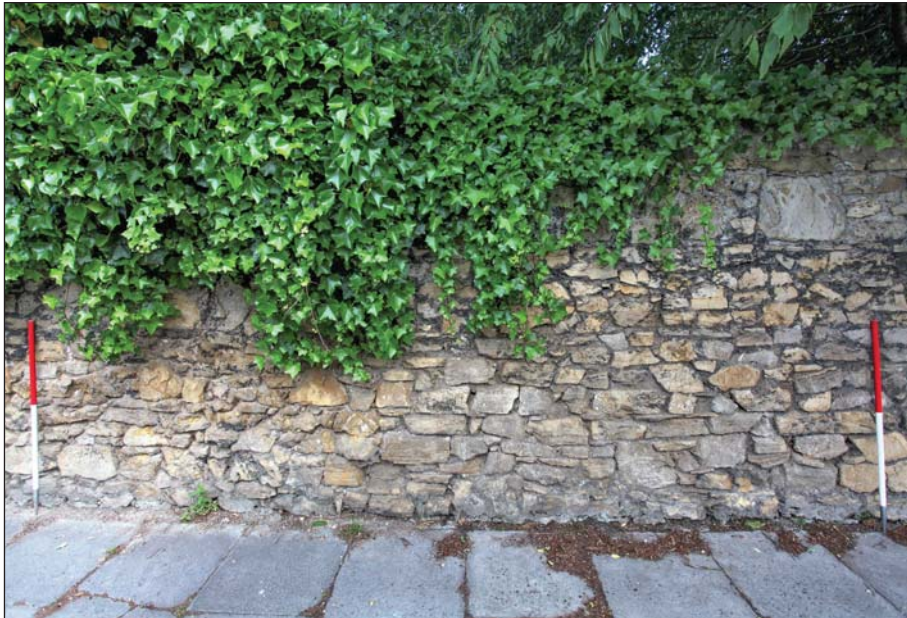
Plate 6: Detailed view of southern boundary wall, section A
