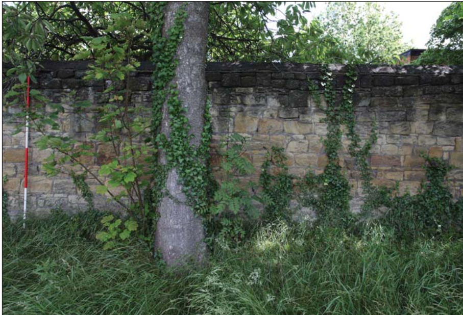
Plate 20: Detailed view of the west face of wall, section E
