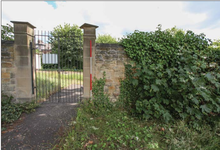
Plate 18: Gate entrance, section D
