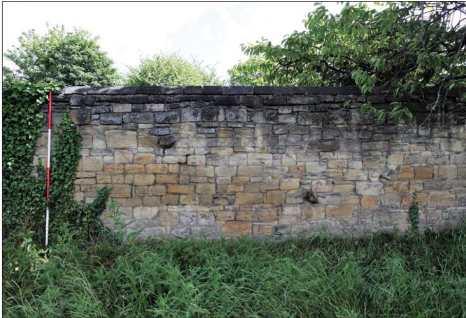
Plate 19: Detailed view of the west face of wall, section E
