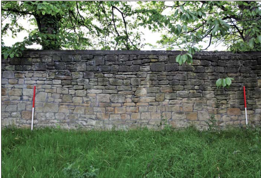
Plate 27: Detailed view of the east face of wall, section E
