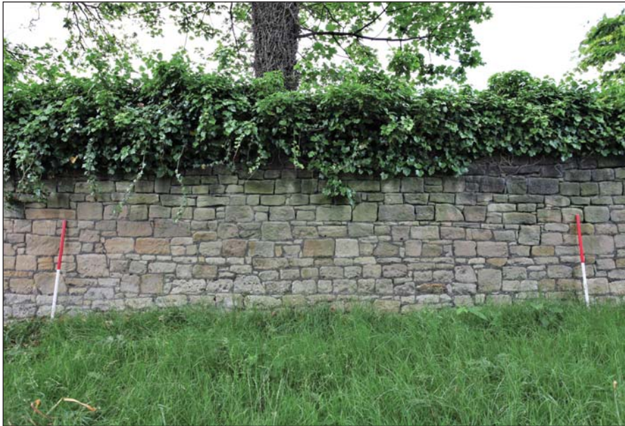
Plate 29: Detailed view of the east face of wall, section E
