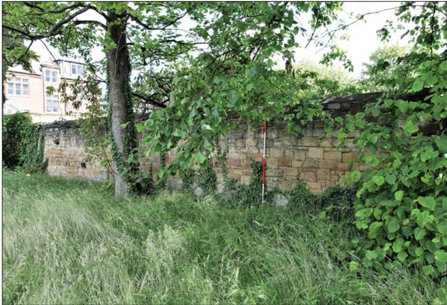
Plate 21: General view of the west face of wall, section E
