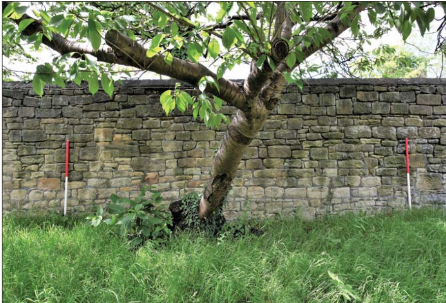
Plate 26: Detailed view of the east face of wall, section E
