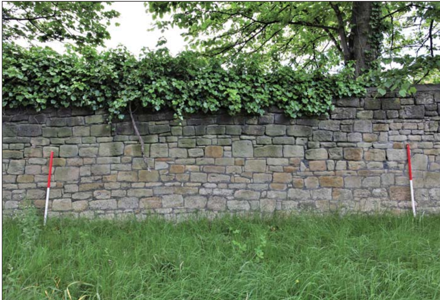
Plate 28: Detailed view of the east face of wall, section E
