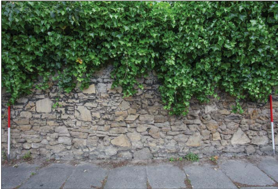
Plate 5: Detailed view of southern boundary wall, section A
