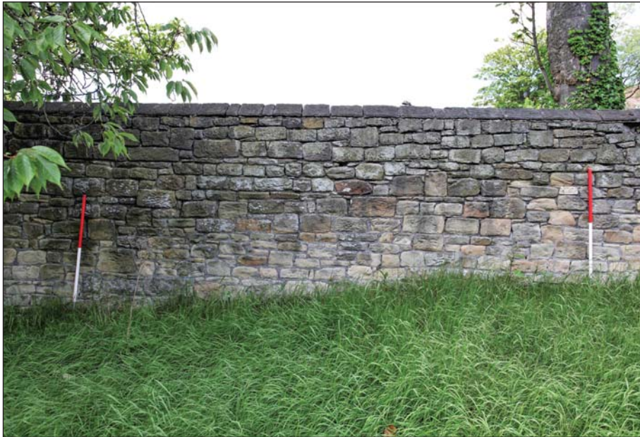
Plate 25: Detailed view of the east face of wall, section E
