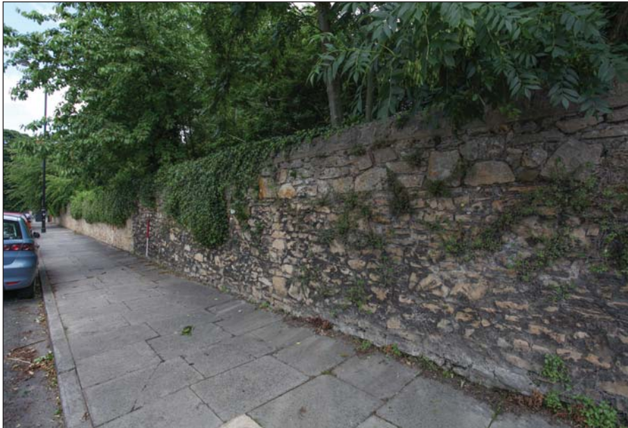
Plate 14: East end of the southern boundary wall, showing different phases
