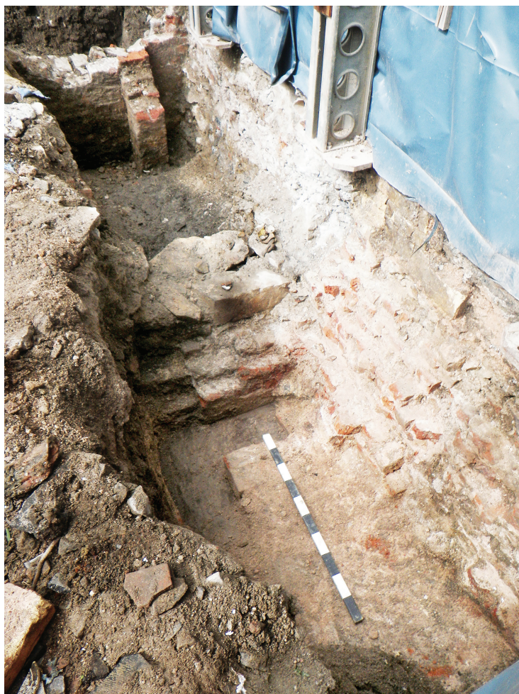
Fig. 9. Sloping stone foundation of wall 421 on the south side of 3 Green Lane, with brick walls 419 (to rear) built clear of the foundation and wall 422 (centre) bonded to it, viewed from the east (scale 1 m).
