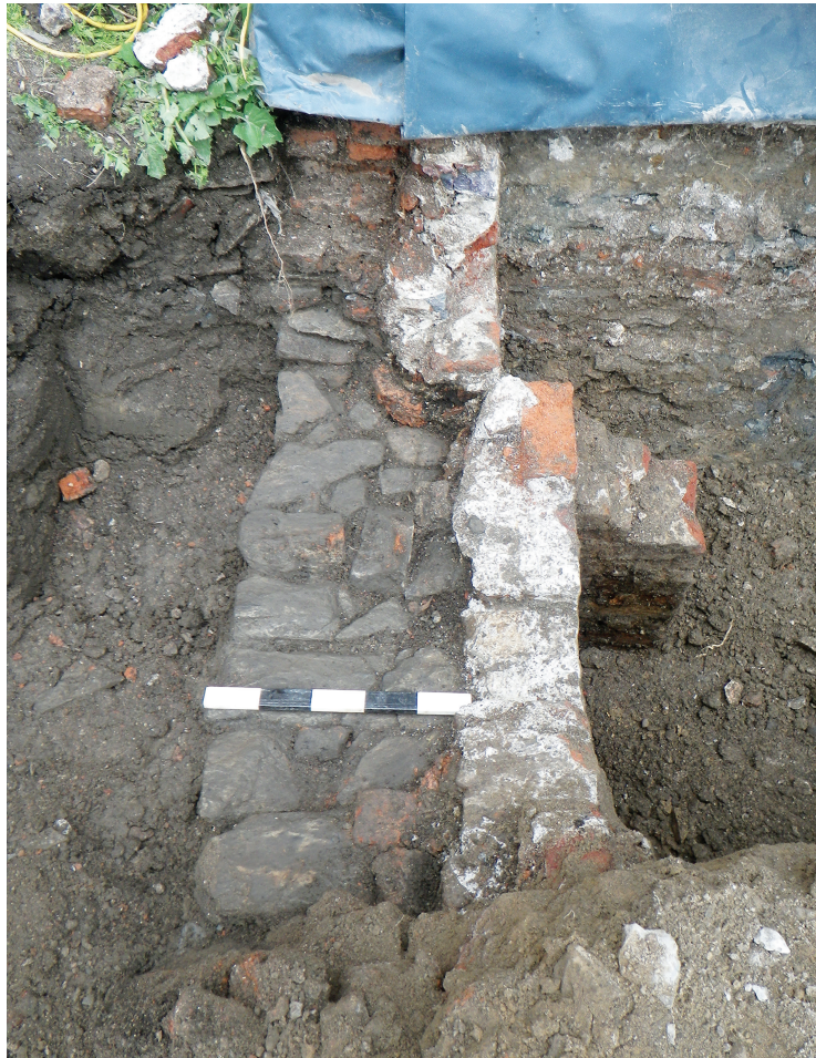
Fig. 10. Stone wall 417, with brick facings 418 and 419, viewed from the south (scale 0.50 m).
