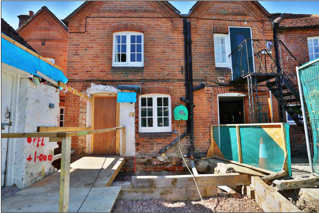
Plate 17: Exterior ground floor wall and openings (intervention 4)
