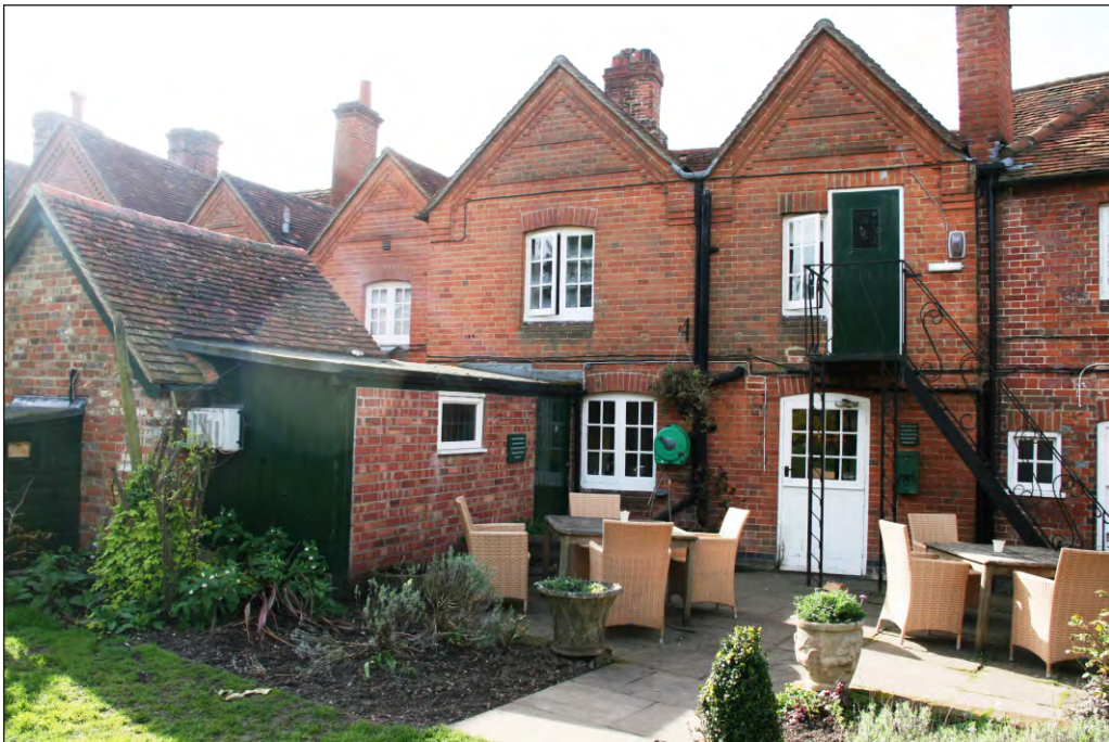
Plate 18: Connecting passage building (intervention 4)
