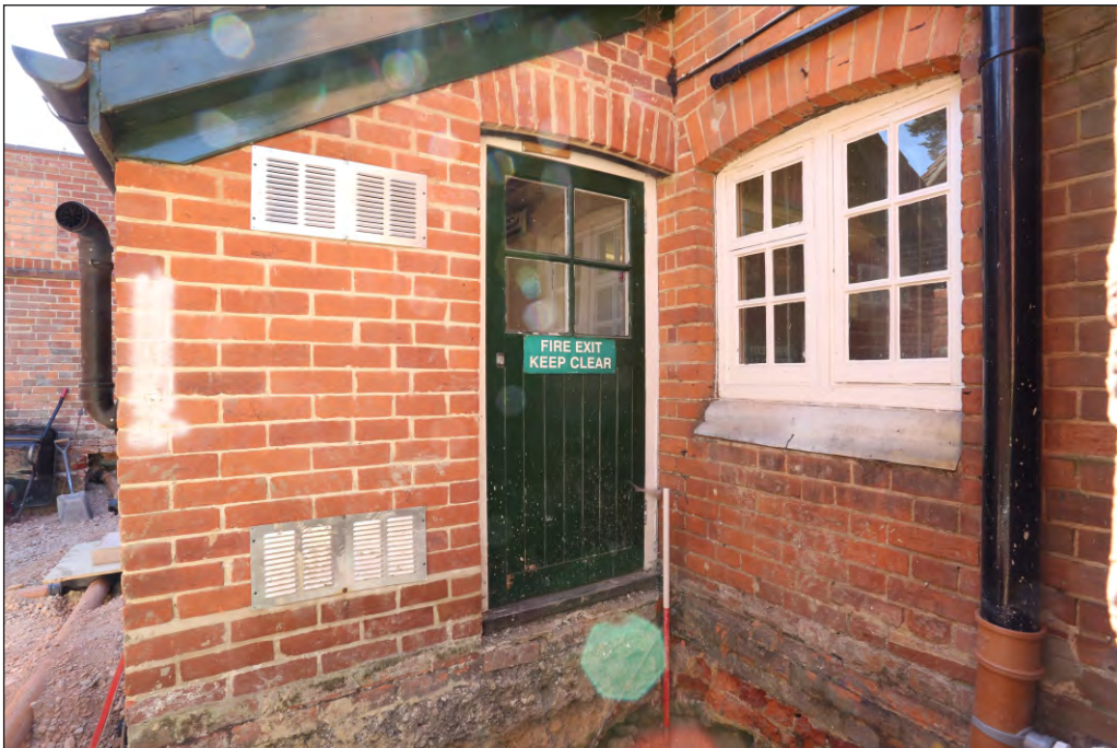
Plate 20: Outbuilding door and rear window (intervention 5)
