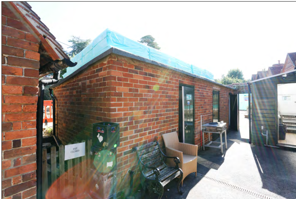
Plate 6: Outbuilding store (intervention 2) south front viewed from south-west
