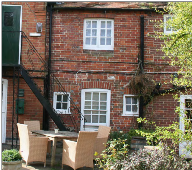
Plate 14: Exterior of ground floor toilets (intervention 3) viewed from north
