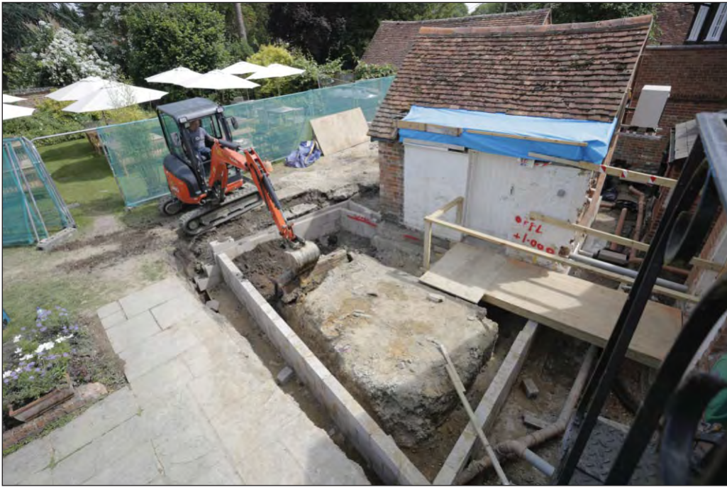
Plate 2: Trench 1 excavation of oversite
