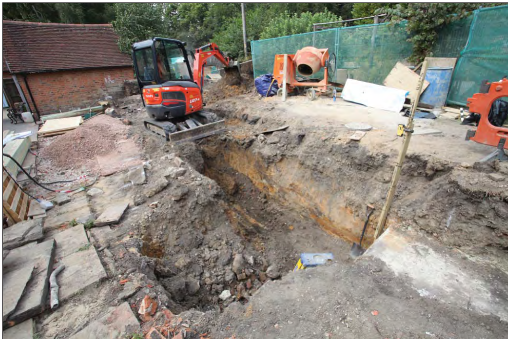
Plate 9: Trench 5 soil sequence and south extension exposing well
