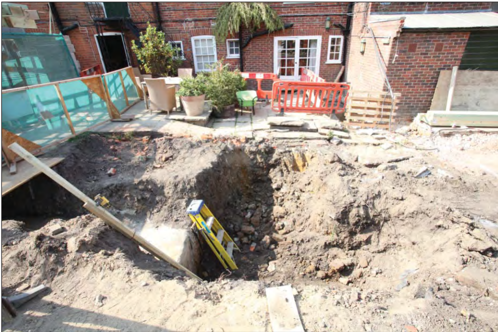
Plate 10: Trench 5 viewed from north showing disturbed rubble infill of old well
