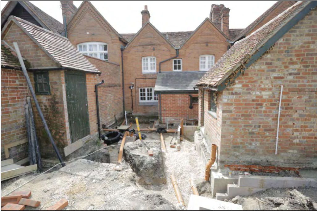
Plate 1: Trench 1 east area
