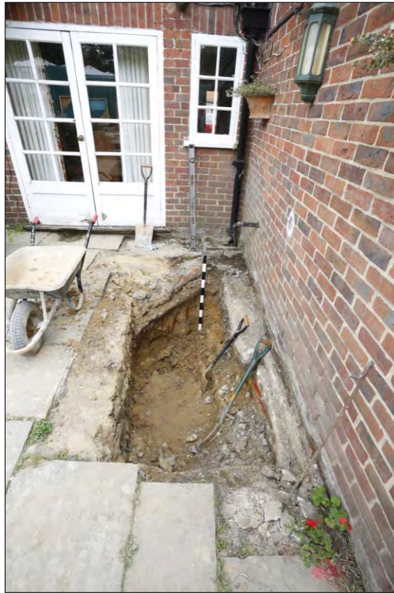
Plate 8: Trench 4 underpinning excavation
