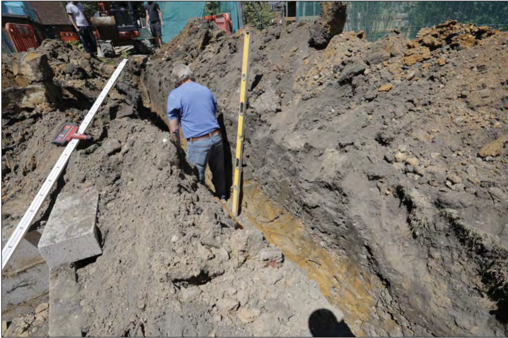
Plate 6: Trench 3 typical soil sequence
