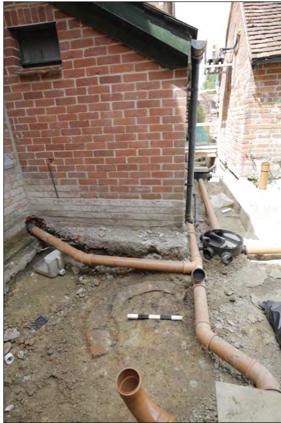
Plate 4: Trench 1 remains of infilled brick lined well
