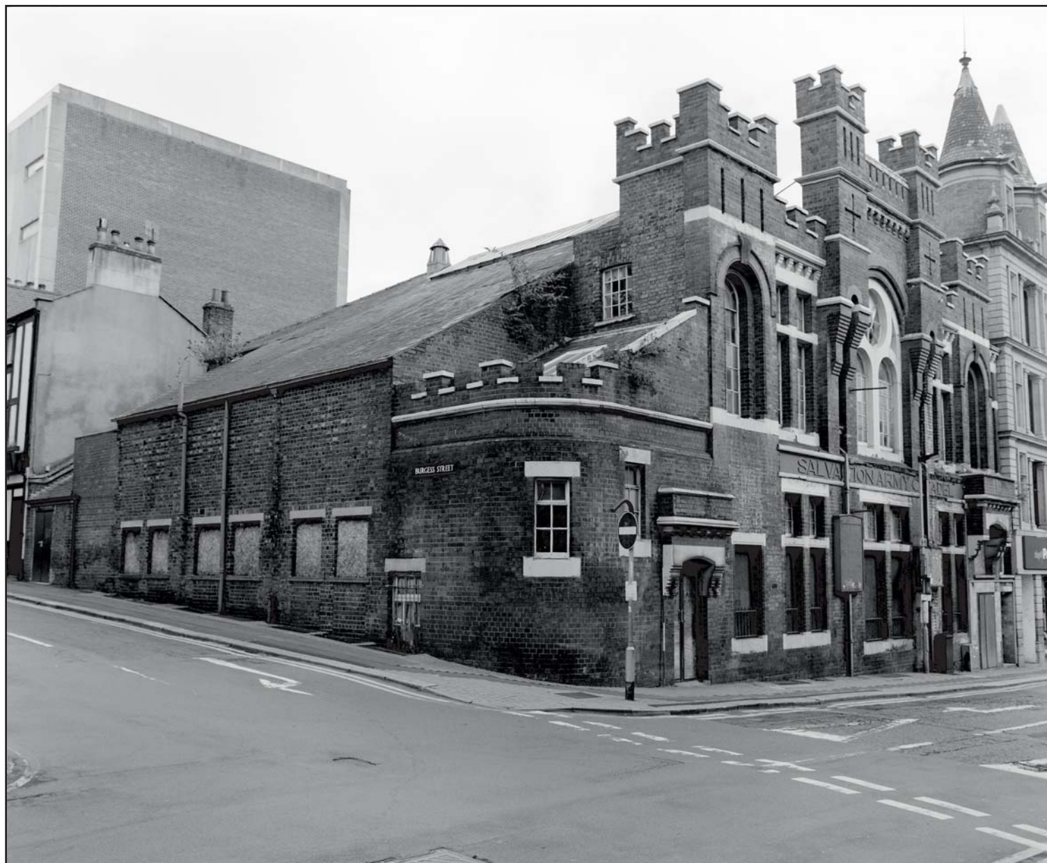
Plate 219: Oblique view of the principal south facing and west facing elevations of the Grade II Listed Building 'Salvation Army Citadel', at the junction of Cross Burgess Street and Burgess Street (ARCUS 2008)
