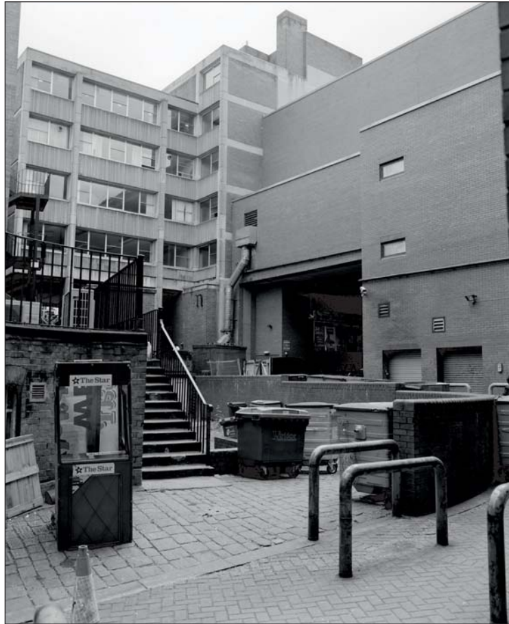
Plate 229: View of the rear elevations of Buildings 34 and 35 (ARCUS 2008)
