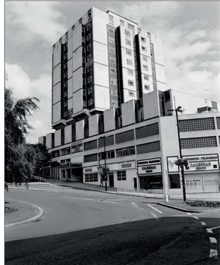
Plate 151: Oblique view of the west facing elevation of Building 23 showing multiple retail units at ground floor level with the 'Grosvenor Hotel' accommodation above, Charter Square (ARCUS 2008)
