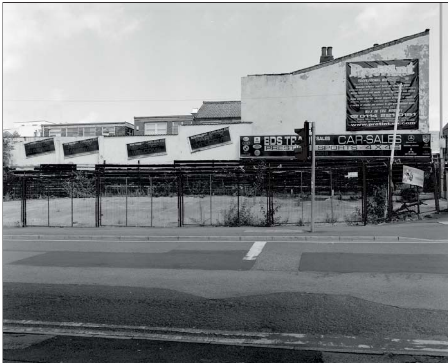
Plate 19: View of the south elevation of Building 7 with enclosed yard, looking north (ARCUS 2008)
