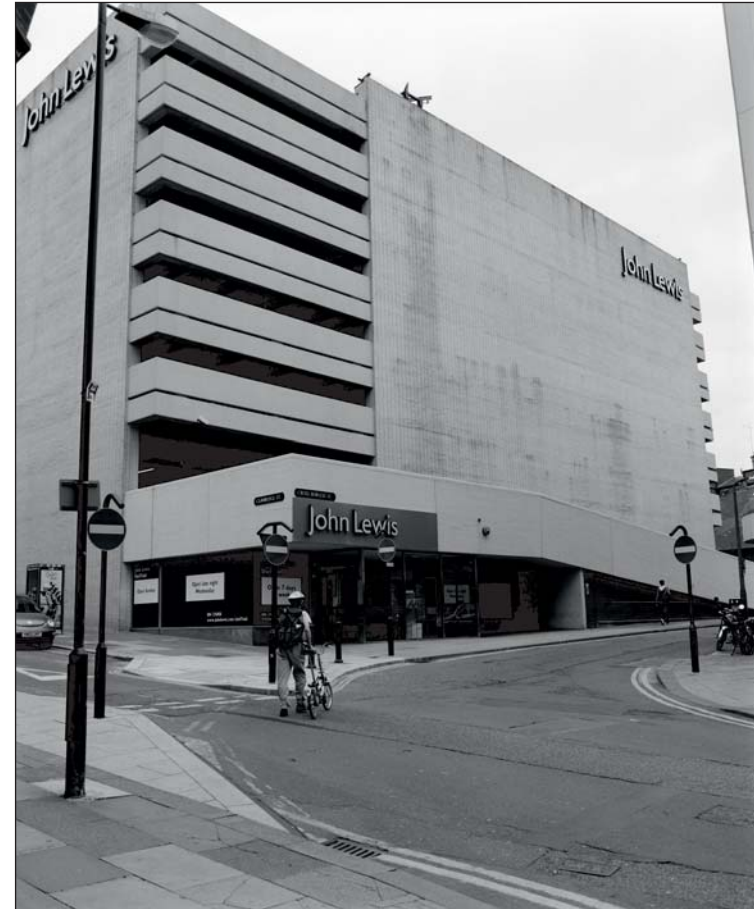
Plate 107: Oblique view of the south facing elevation of 'John Lewis', Building 33, Cross Burgess Street, looking north-east (ARCUS 2008)
