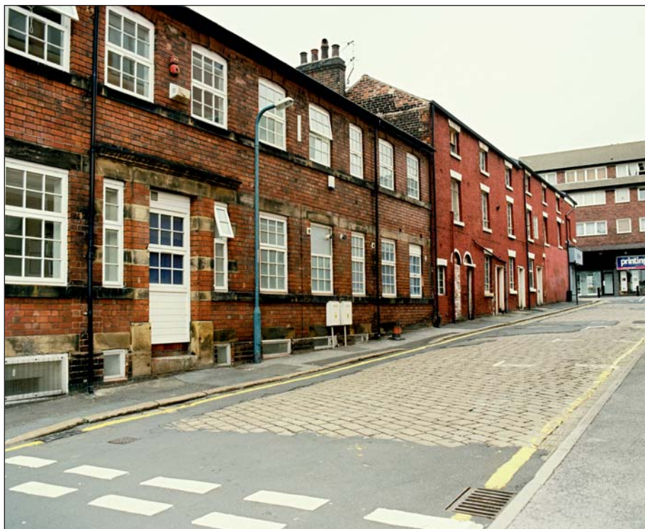
Plate 6: General view up Canning St, looking north (ARCUS 2008)
