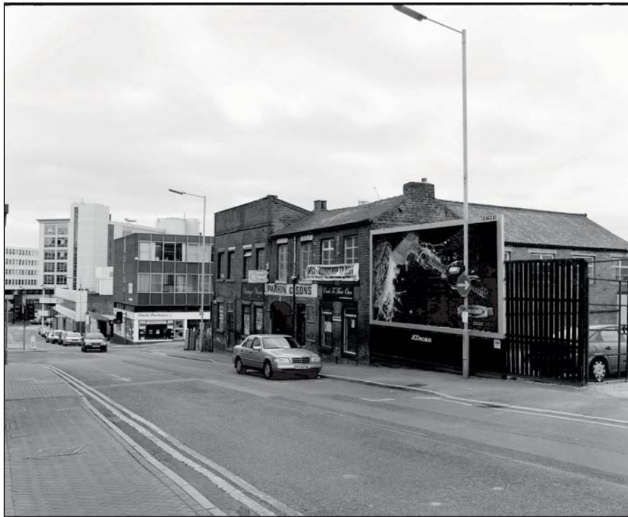
Plate 26: General view looking south down Rockingham Street showing Buildings 8 and 9 (ARCUS 2008)
