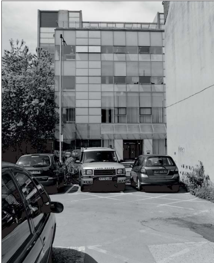
Plate 55: View of the east facing elevation of Building 41 (ARCUS 2008)
