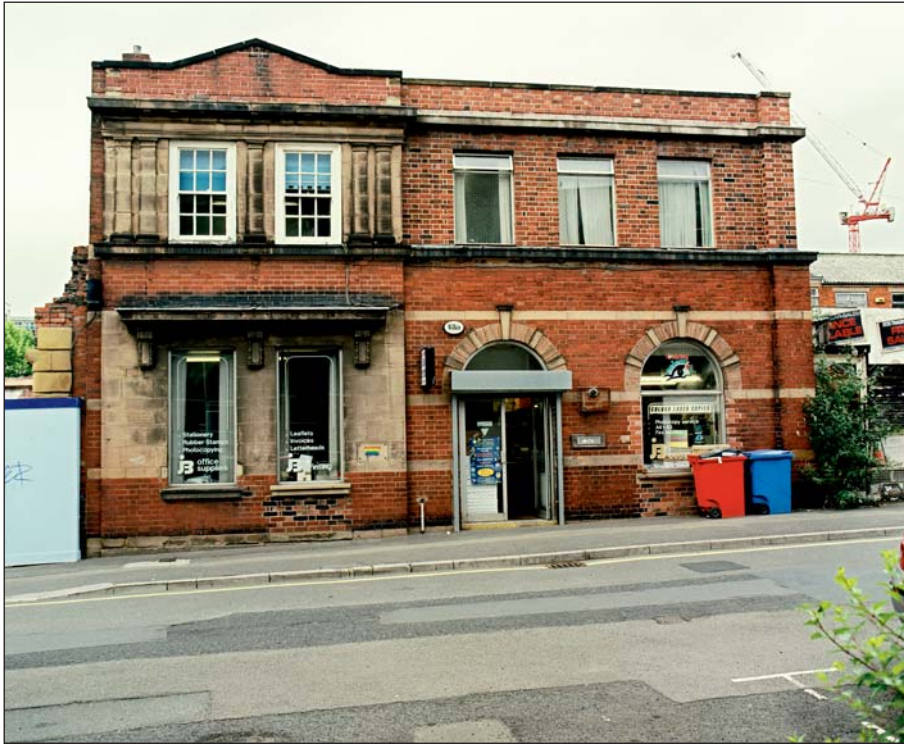
Plate 14: View of the principal south facing elevation Building 6, Wellington Street (ARCUS 2008)
