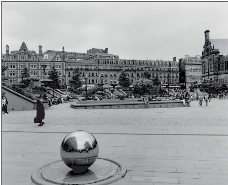
Plate 254: View of the principal east facing elevations of Buildings 37, 40 and 37, Pinstone Street from the Peace Gardens, looking west (ARCUS 2008)
