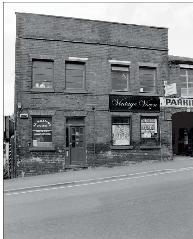
Plate 23: View of the principal east elevation of Building 7, looking west (ARCUS 2008)
