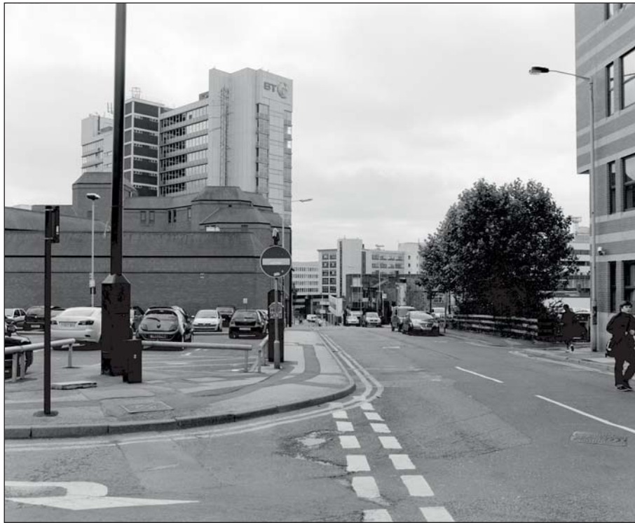
Plate 28: General view looking south down Rockingham Street showing Building 11 (ARCUS 2008)
