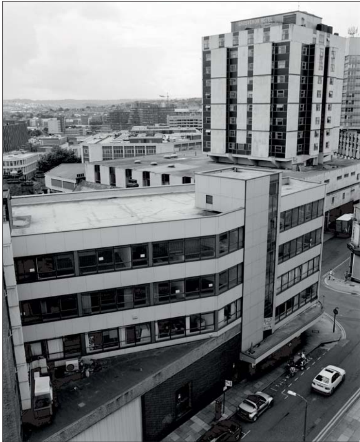
Plate 190: Elevated view of Building 27, Cross Burgess Street, with the 'Grosvenor Hotel', Building 23 beyond from the roof of 'John Lewis', Building 33 (ARCUS 2008)
