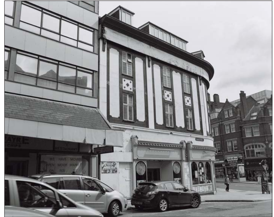
Plate 197: View of the south-west facing elevation of the 'Athol Hotel' Building 28, Charles Street (Wessex Archaeology 2016)
