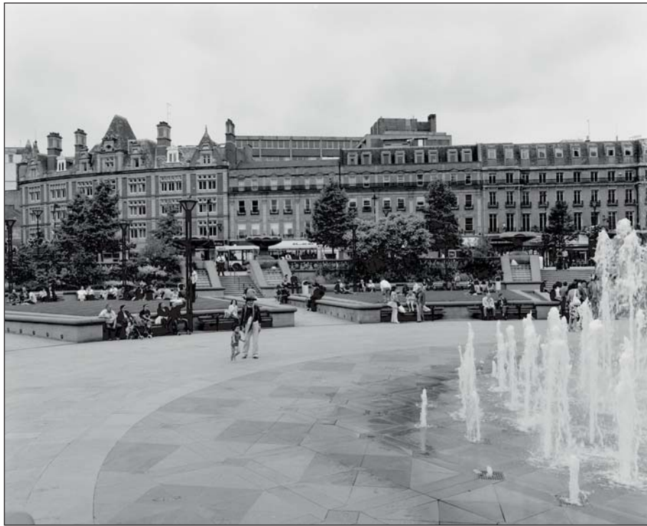
Plate 253: View of the principal east facing elevations of Buildings 38, 37 and 40, Pinstone Street from the Peace Gardens, looking west (ARCUS 2008)
