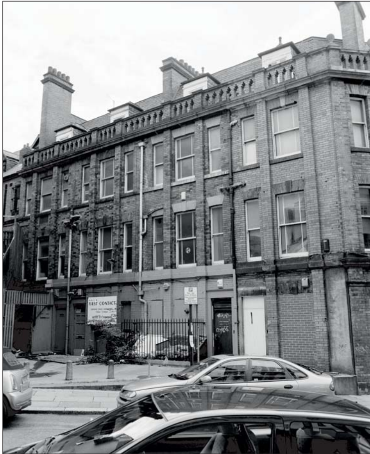
Plate 178: View of the rear north-west facing elevation of Building 25, Cambridge Street (ARCUS 2008)
