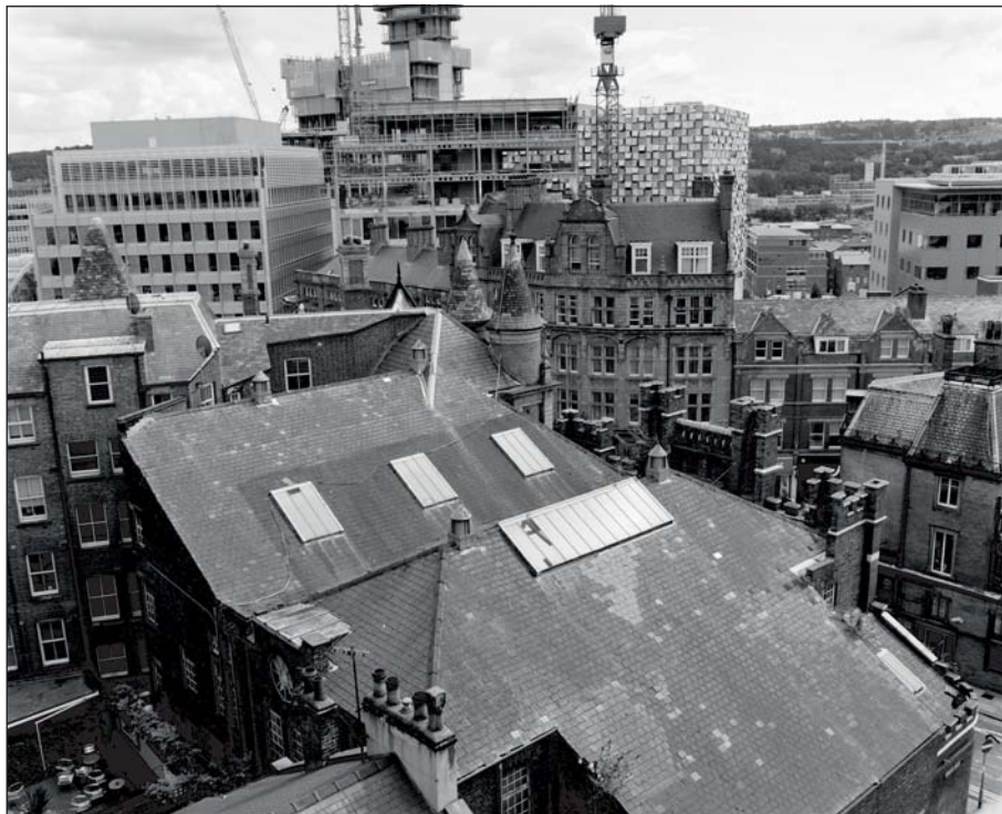
Plate 221: Elevated view of the rooftops of the Grade II Listed Building 'Salvation Army Citadel' and beyond from the roof of 'John Lewis', Building 33 (ARCUS 2008)
