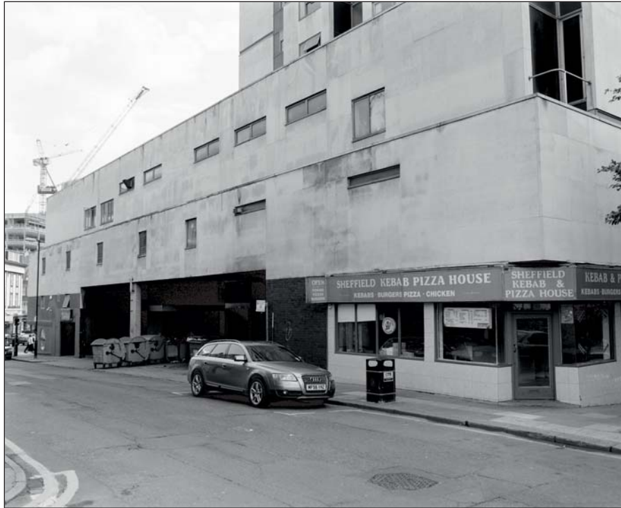
Plate 164: Oblique view of the north facing elevation of the 'Grosvenor Hotel' vehicular access and 'Sheffield Kebab Pizza House' within Building 23 at ground floor level, looking south-east (ARCUS 2008)
