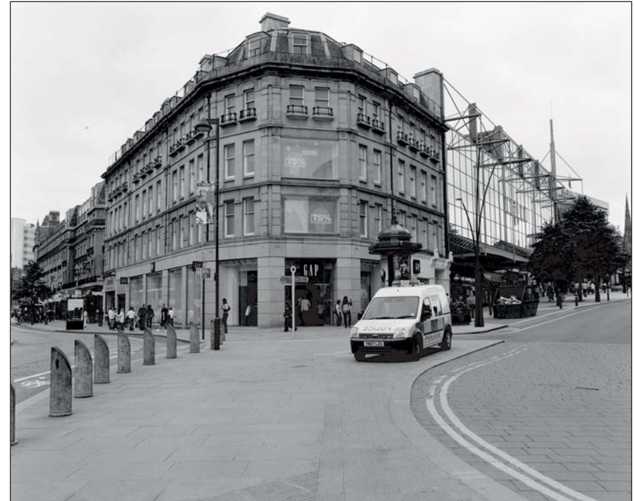
Plate 236: View of the junction of Barker's Pool and Pinstone Street showing Buildings 77, 40, 36 and 35, looking south-west (ARCUS 2008)
