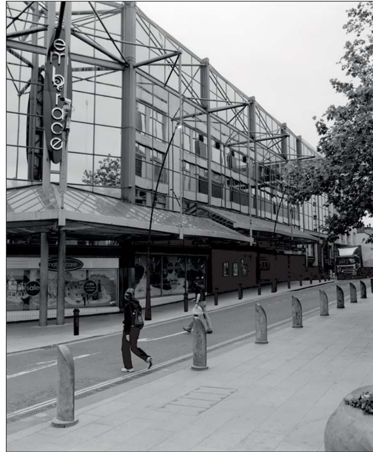
Plate 232: Oblique view of the west facing elevation of Building 35, Burgess Street, looking south-east (ARCUS 2008)
