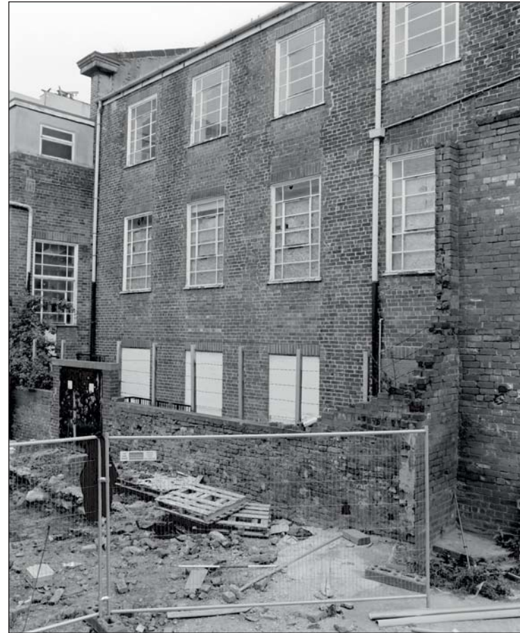
Plate 64: Oblique view of the north facing elevation of Building 17b (ARCUS 2008)
