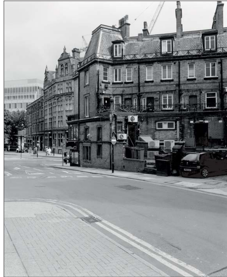
Plate 205: Oblique view of the rear north and north-west elevation of Building 30, Cross Burgess Street, with Pinstone Street beyond, looking south-east (ARCUS 2008)
