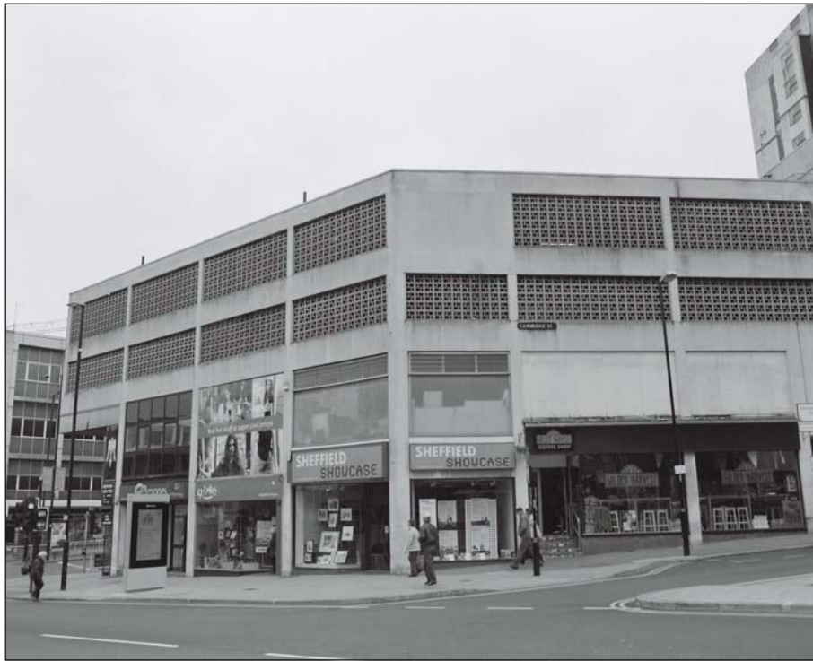
Plate 144: View of the south-east corner of Building 23 at the junction of Cambridge Street and Pinstone Street showing retail units (Wessex Archaeology 2016)
