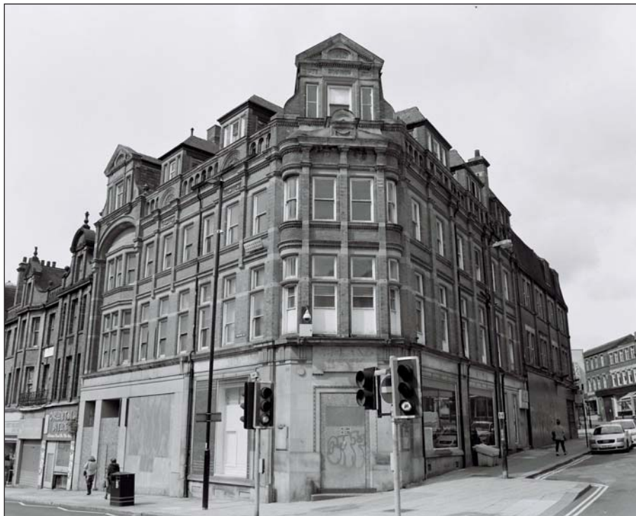
Plate 169: View of the east corner of the 'HSBC' Building 26 at the junction of Pinstone Street and Charles Street, looking west (Wessex Archaeology 2016)
