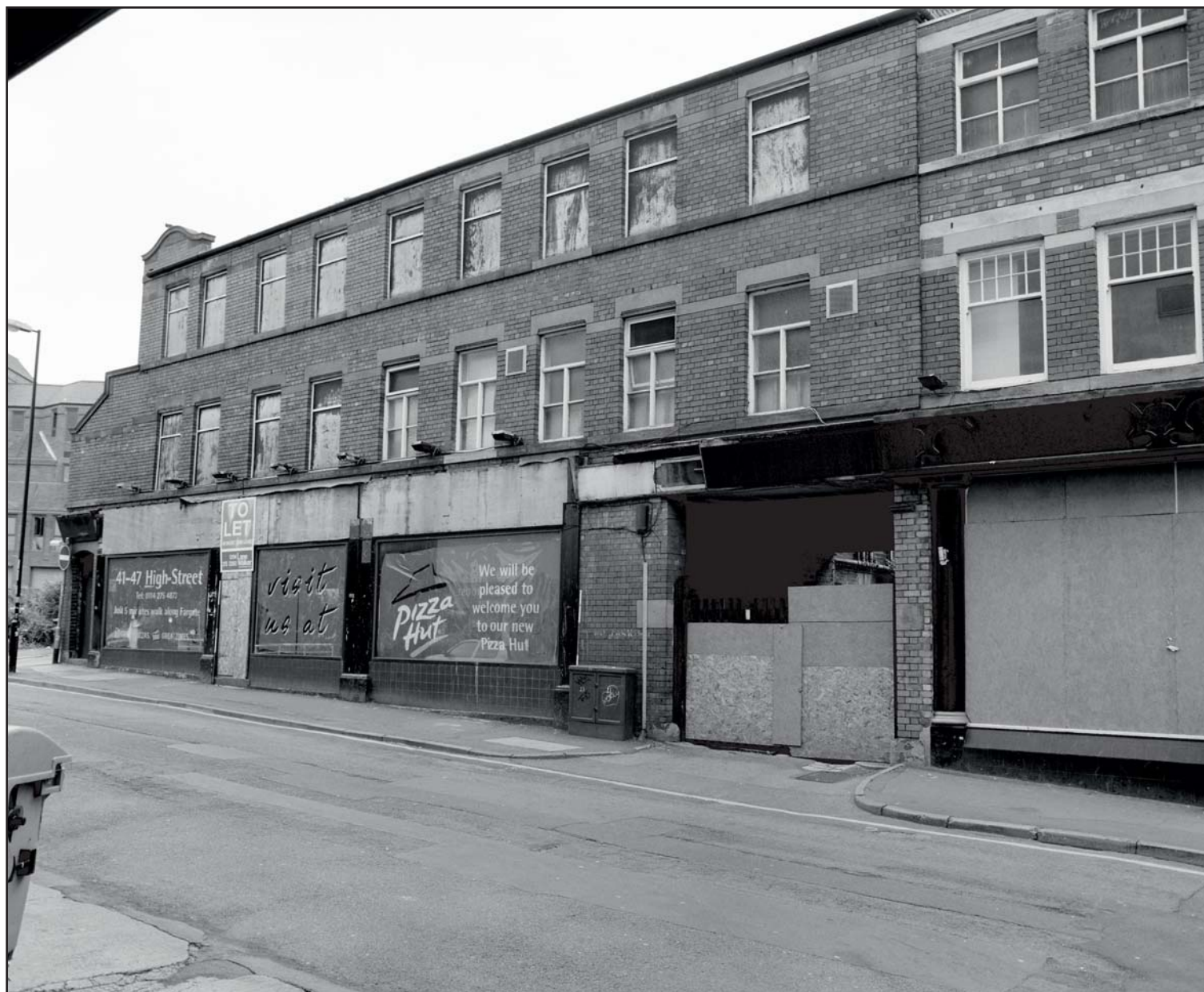
Plate 77: Oblique view of the south facing elevation of Building 22, looking north-west (ARCUS 2008)
