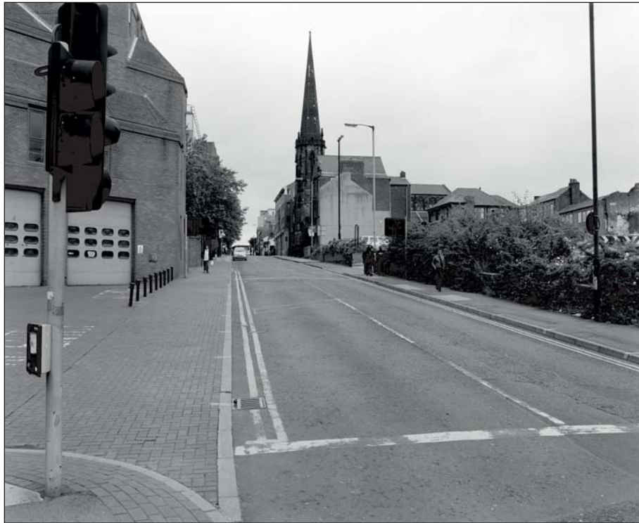
Plate 58: General view looking north up Carver Street (ARCUS 2008)
