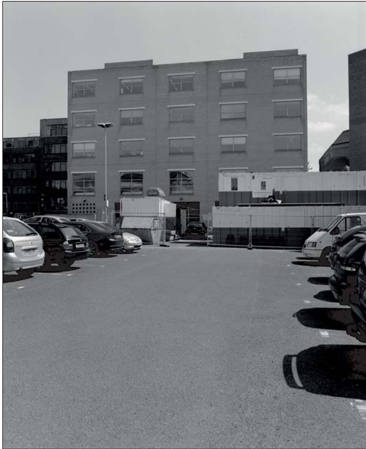
Plate 50: View of the west facing elevation of Building 41 (ARCUS 2008)
