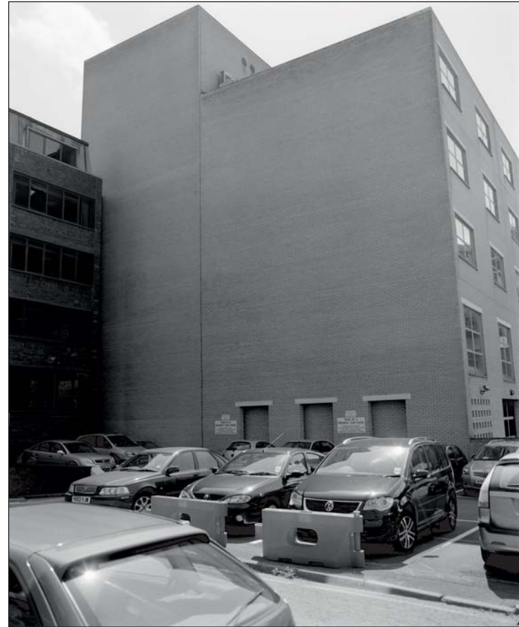
Plate 53: View of the north facing elevation of Building 41 (ARCUS 2008)
