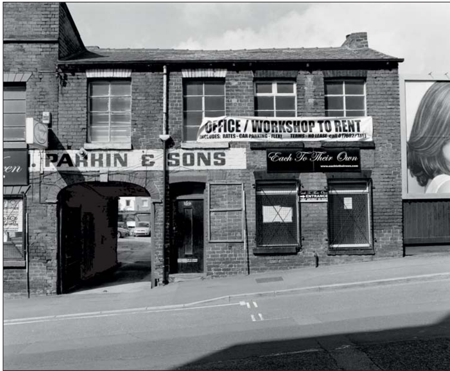
Plate 24: View of the principal east elevation of Building 8, looking west (ARCUS 2008)
