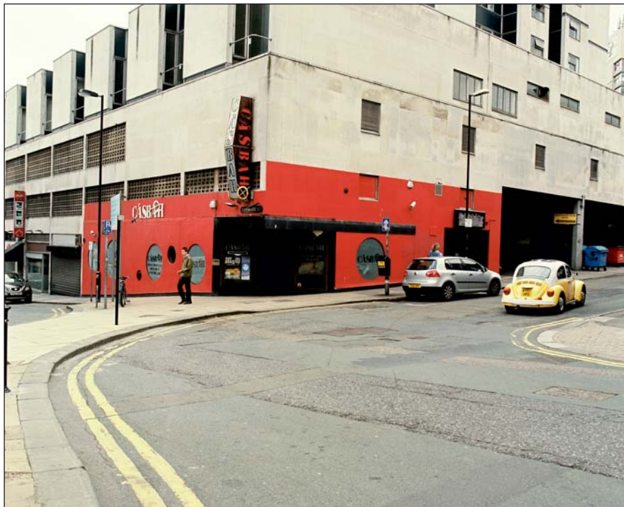
Plate 126: Oblique view of the north-east corner of Building 23, showing the 'Casbah' night club (ARCUS 2008)
