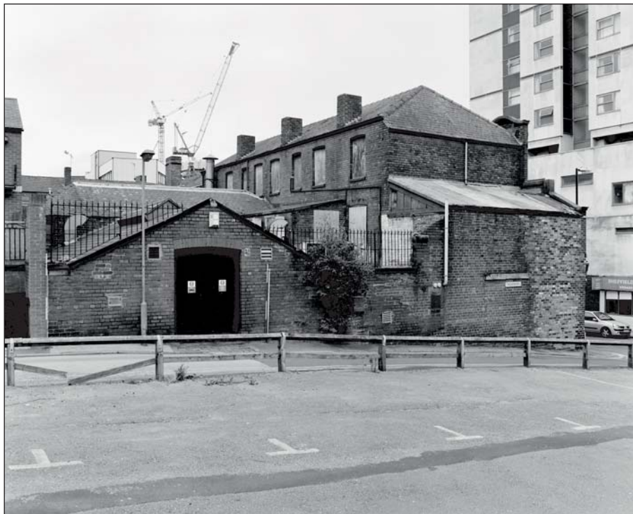
Plate 70: Oblique view of the west facing elevation of Building 22 showing north facing elevation of Building 21 at first floor level beyond (ARCUS 2008)
