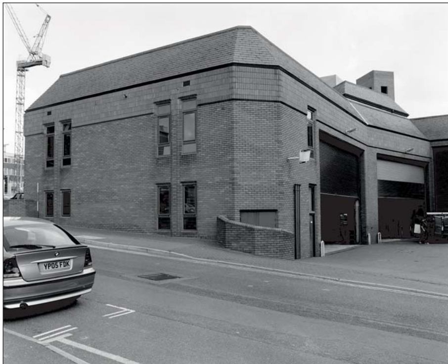
Plate 31: Oblique view of the south-west corner of Building 11 (ARCUS 2008)
