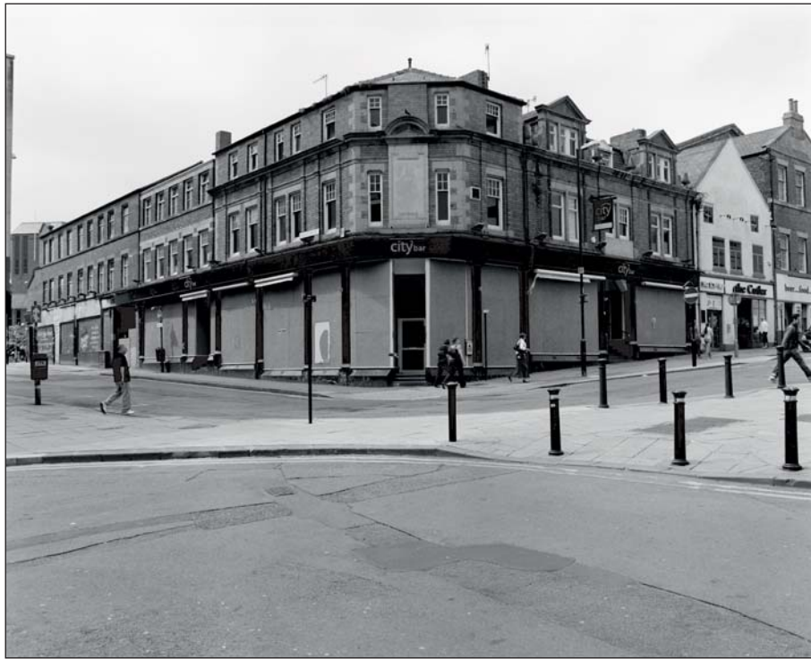
Plate 82: General view of the junction of Wellington Street and Cambridge Street showing the corner entrance of 'City Bar' comprising Buildings 21, 20b and 20a (ARCUS 2008)
