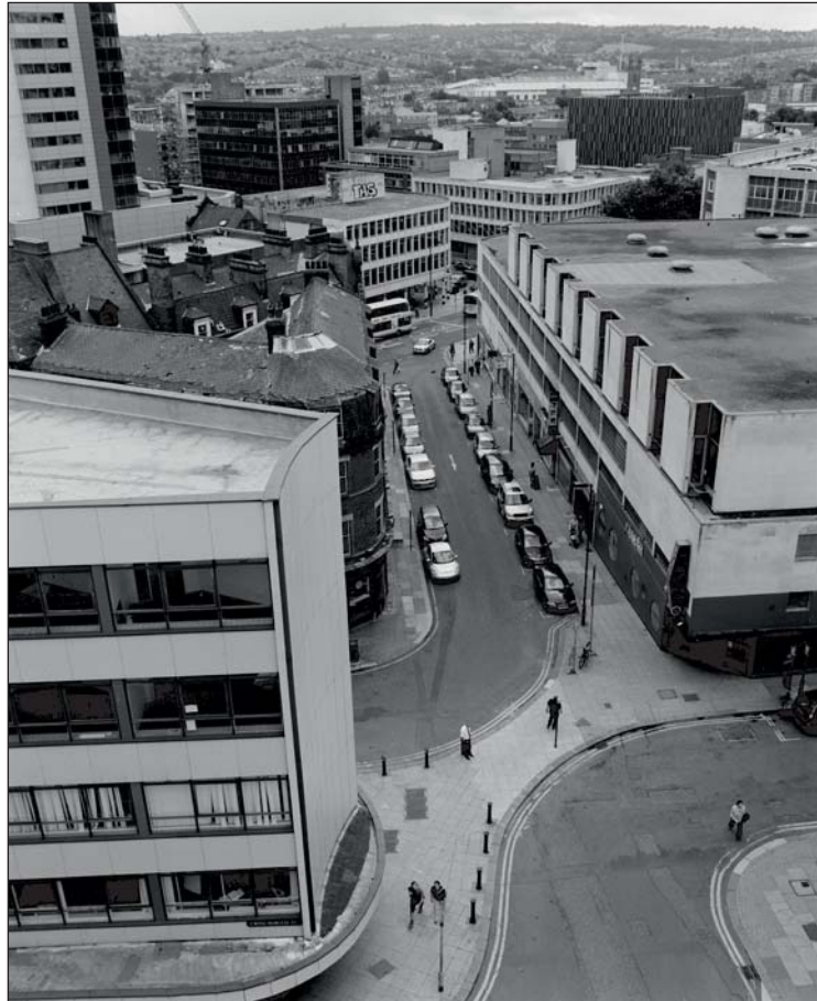
Plate 121: Elevated view of the south end of Cambridge Street showing the east facing elevation of Building 23, looking south-west from the roof of 'John Lewis', Building 33 (ARCUS 2008)
