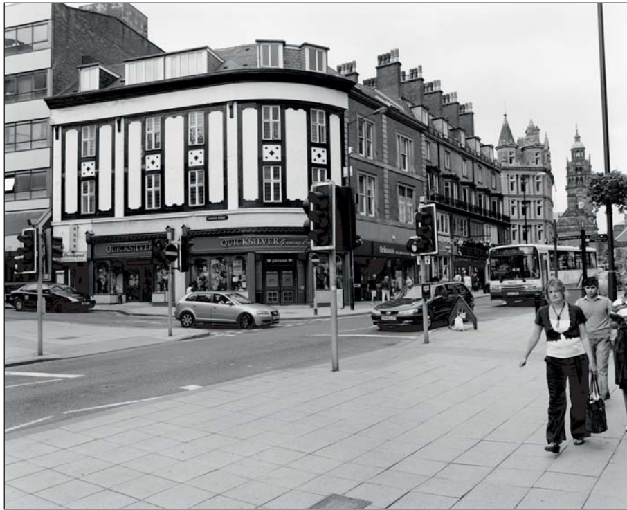
Plate 198: View of the 'Athol Hotel' Building 28, from the junction of Pinstone Street and Charles Street, with the south-east facing elevations of Buildings 29 and 30, Pinstone Street beyond, looking north (ARCUS 2008)
