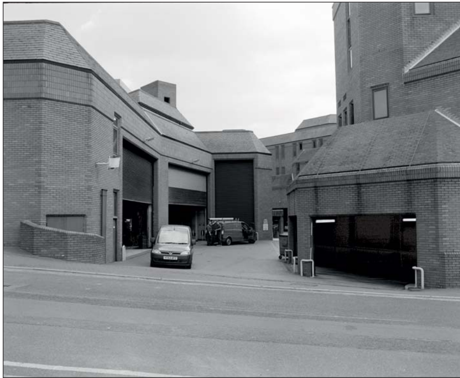
Plate 32: General view into yard of Fire Station, Buildings 11 and 12 looking east (ARCUS 2008)
