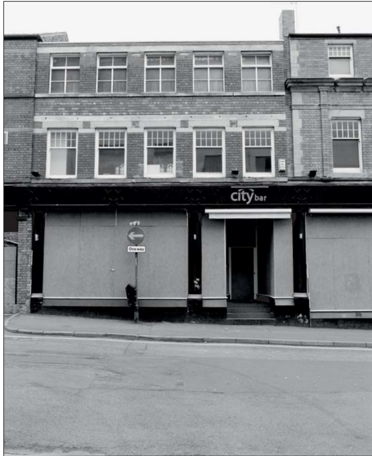
Plate 78: View of the south facing elevation of Building 22 (ARCUS 2008)
