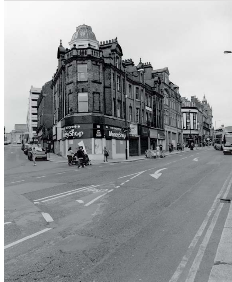
Plate 175: View of Building 25 at the junction of Cambridge Street and Pinstone Street, looking north (ARCUS 2008)
