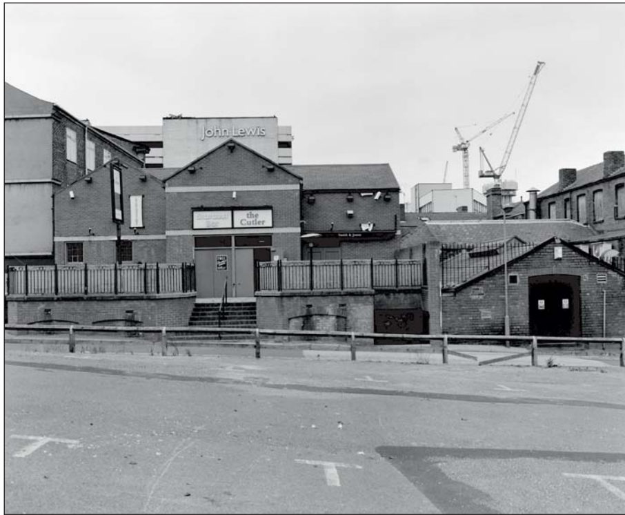
Plate 69: View of the west facing elevation of 'The Cutler' Building 19 from Backfields (ARCUS 2008)
