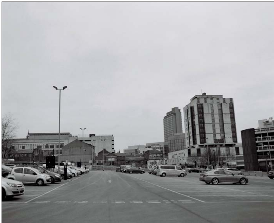
Plate 33: General view of the site of the former Fire Station, Buildings 11 and 12, now demolished, looking east (Wessex Archaeology 2016)
