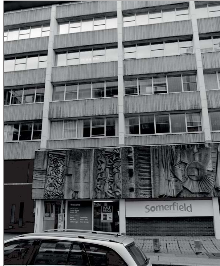
Plate 226: View of the principal west facing elevation of Building 34 at the central section, Burgess Street (ARCUS 2008)
