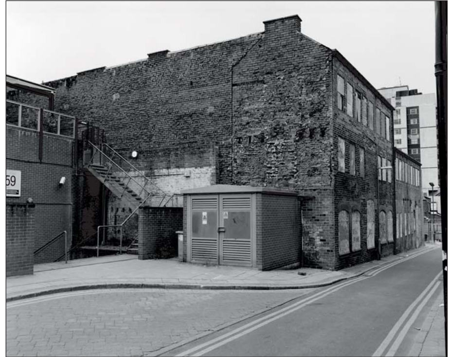
Plate 61: Oblique view of the north facing and west facing elevations of the Grade II* Listed Building 'Leahs Yard', Building 13 (ARCUS 2008)
