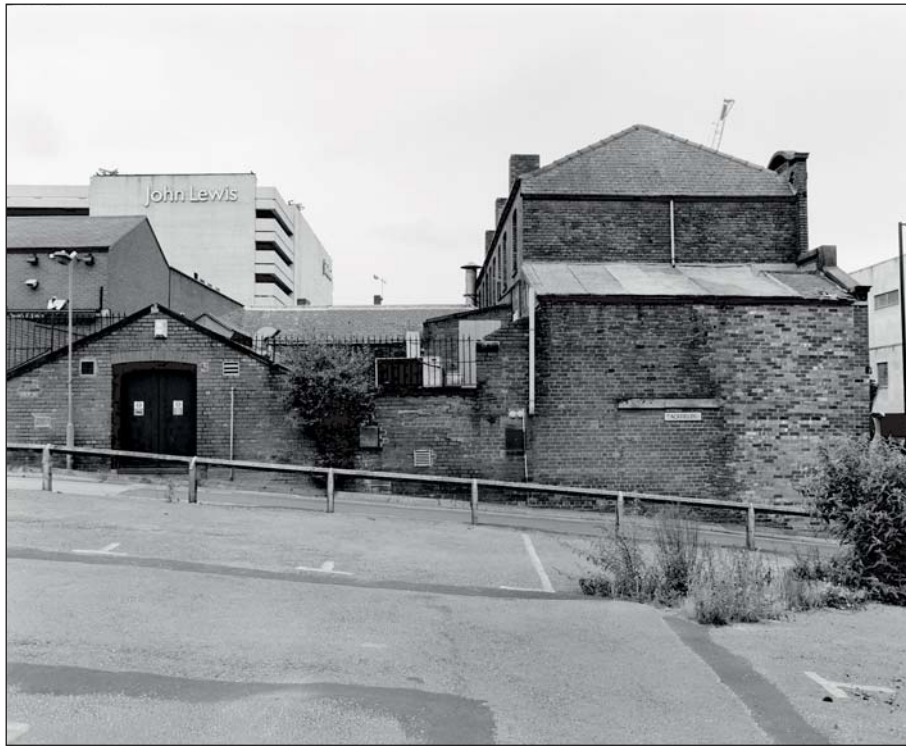
Plate 71: View of the west facing elevation of Building 22 from Backfields (ARCUS 2008)
