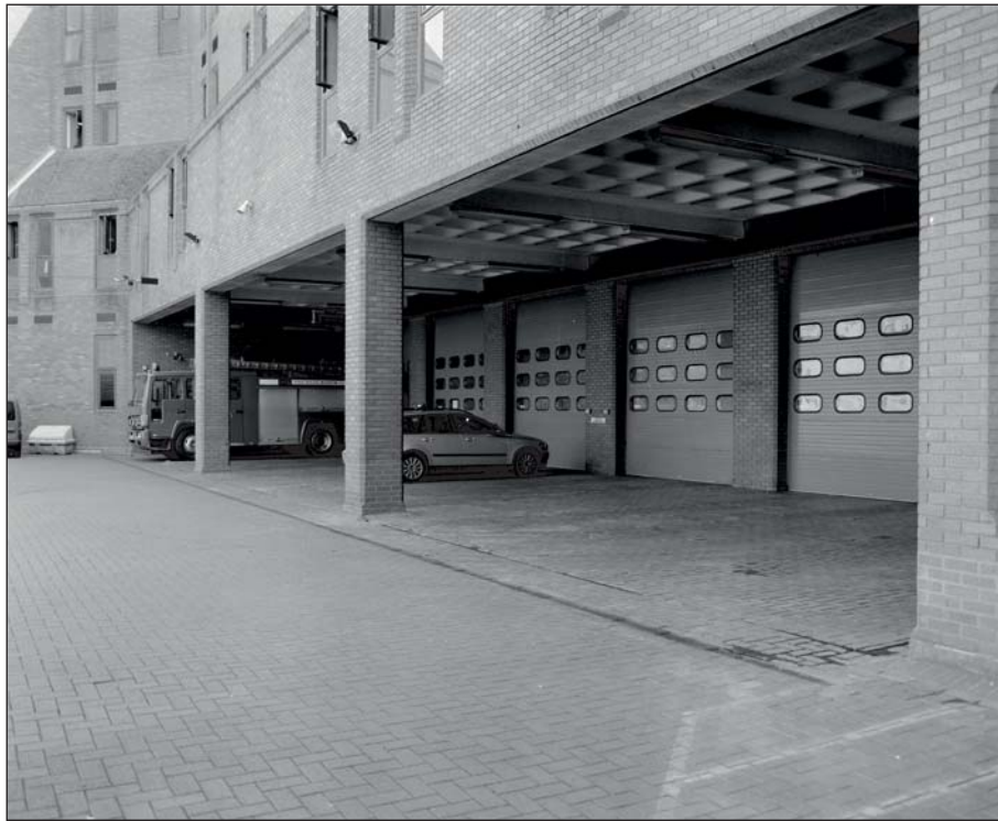
Plate 37: Detail of vehicular bays at Building 12 (ARCUS 2008)
