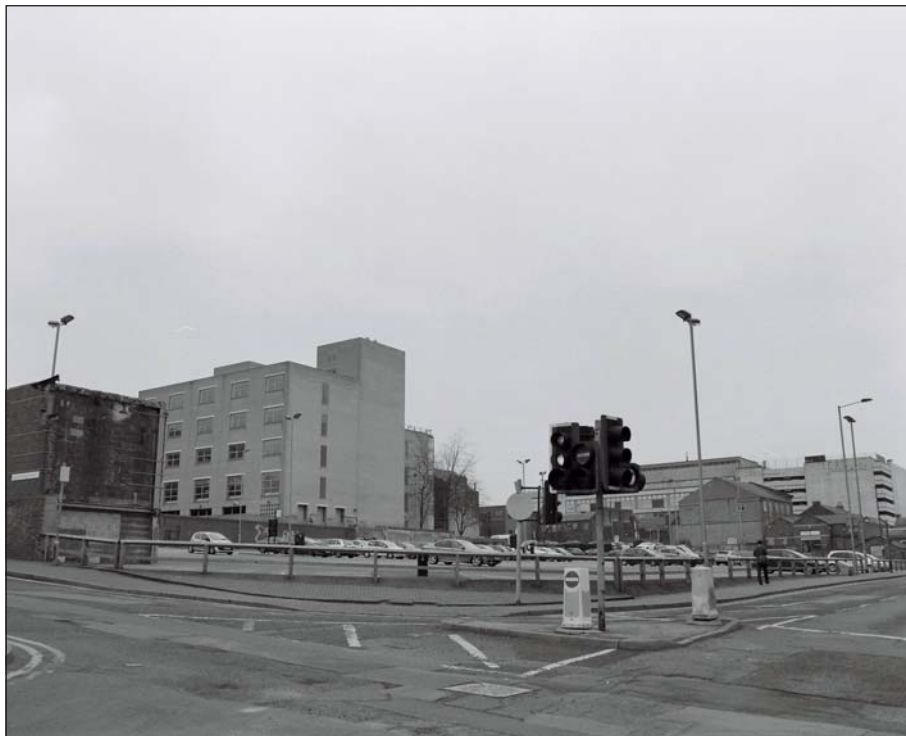
Plate 40: General view of the junction of Rockingham Street and Wellington Street showing the site of the former Fire Station, Building 12, now demolished (Wessex Archaeology 2016)
