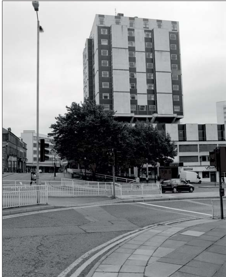
Plate 160: View of the west facing elevation of the 'Grosvenor Hotel' Building 23, Charter Square, with Wellington Street to the north, looking east (ARCUS 2008)
