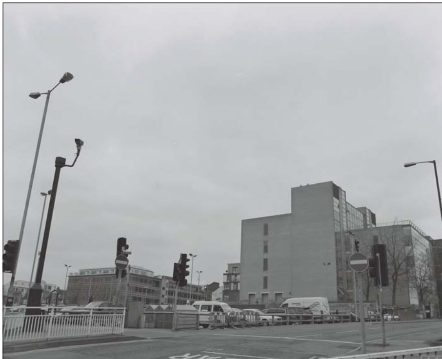
Plate 43: General view looking north-west up Carver Street from Charter Square showing the site of the former Fire Station, Building 12, now demolished with Building 41 beyond (Wessex Archaeology 2016)
