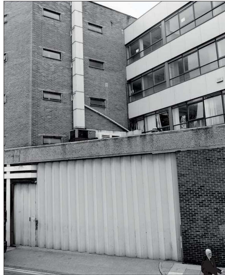
Plate 189: Oblique view of the north facing elevation of Building 27, showing vehicular entrance at street level, Cross Burgess Street (ARCUS 2008)
