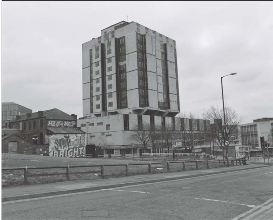
Plate 162: Distance view of Building 23, looking south-east (Wessex Archaeology 2016)
