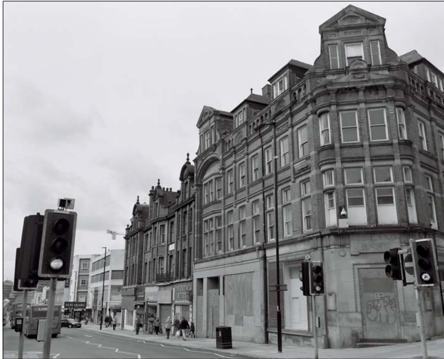
Plate 170: Oblique view of the south-east facing elevations of Buildings 25 and the 'HSBC' Building 26, Pinstone Street looking south-west with Building 23 beyond (Wessex Archaeology 2016)
