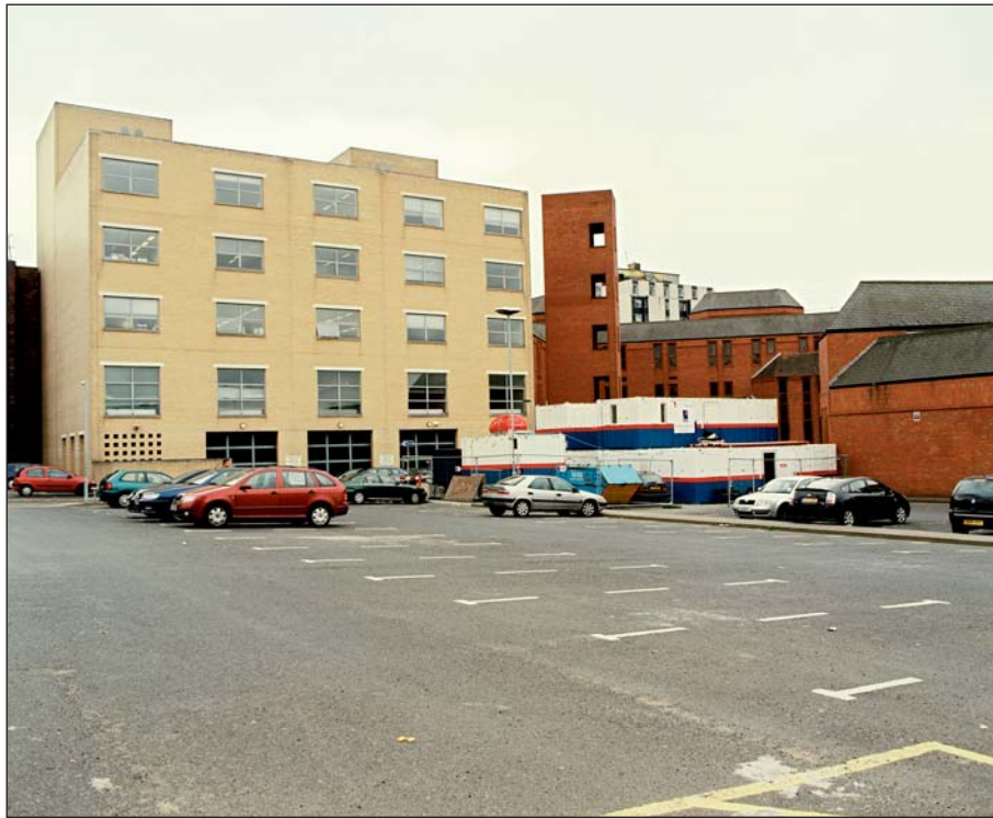
Plate 48: Oblique view of Buildings 41, 11, and 12, looking south-east (ARCUS 2008)
