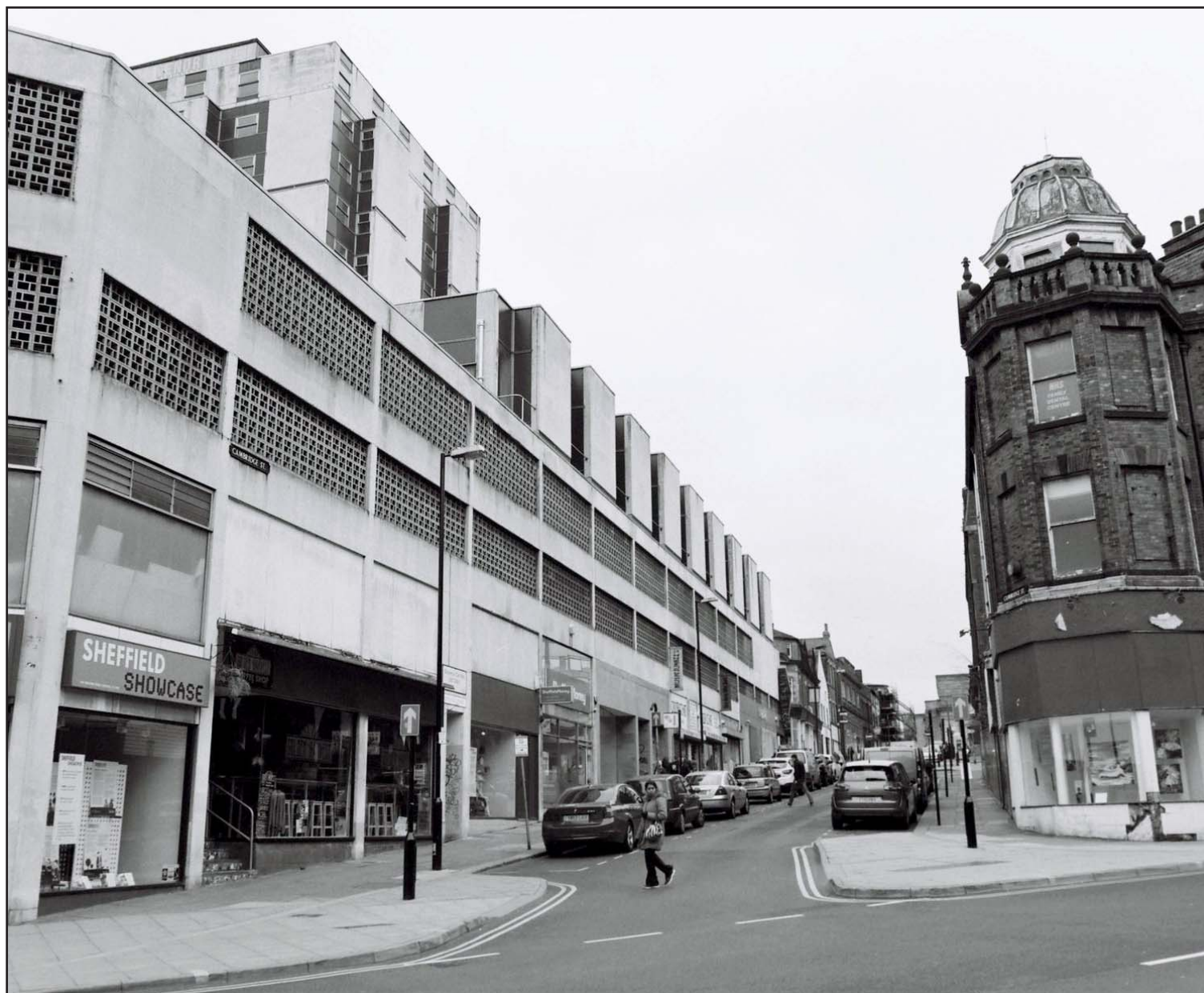
Plate 143: Oblique view of the east facing elevation of Building 23, Cambridge Street, looking north-west (Wessex Archaeology 2016)
