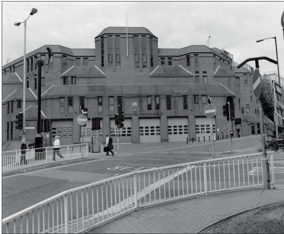
Plate 42: View of the south-east corner of Building 12, from Charter Square, looking north-west (ARCUS 2008)
