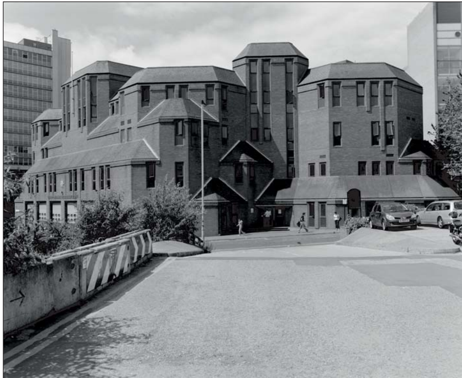
Plate 44: View of the east facing elevation of Building 12, Carver Street (ARCUS 2008)
