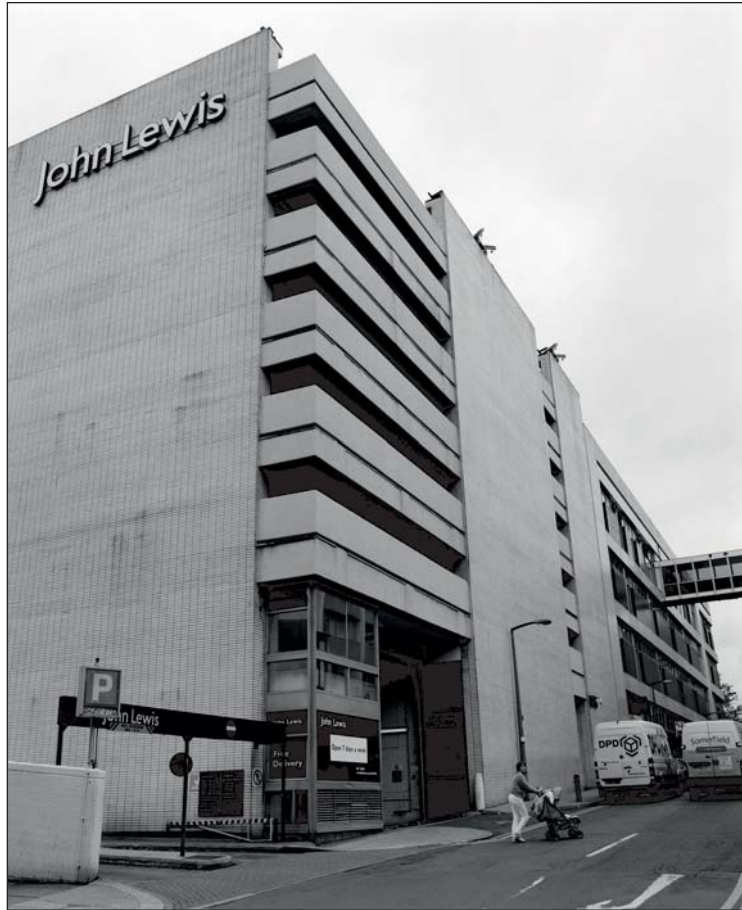
Plate 110: Oblique view of the east facing elevation of 'John Lewis', Building 33, Burgess Street, looking north-west (ARCUS 2008)
