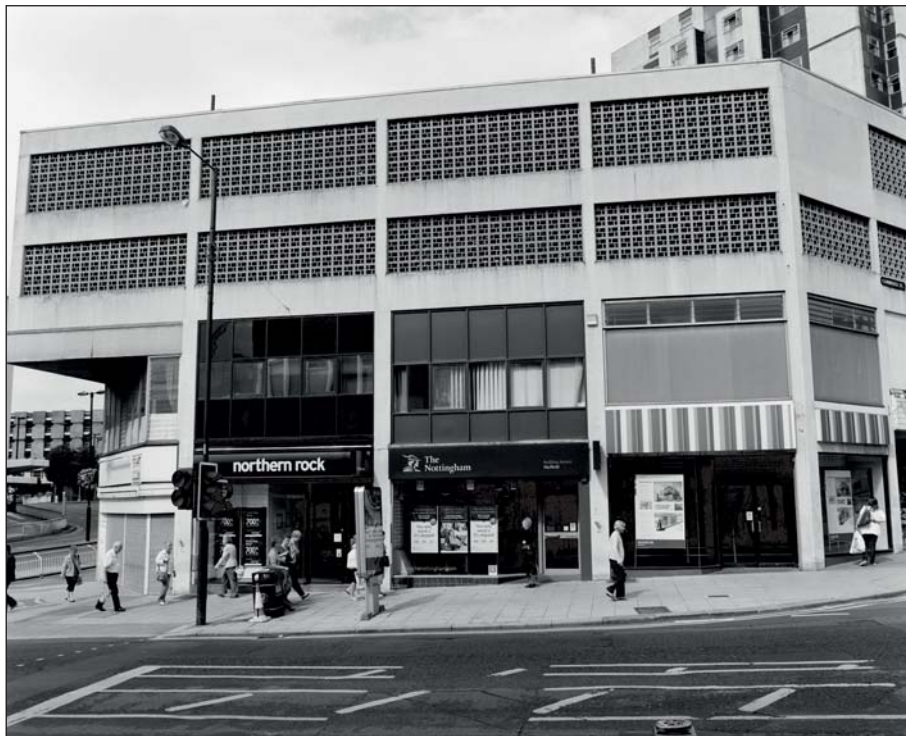
Plate 145: View of the south-east facing elevation of 'Northern Rock', 'The Nottingham' and other retails units, Building 23, Pinstone Street (ARCUS 2008)
