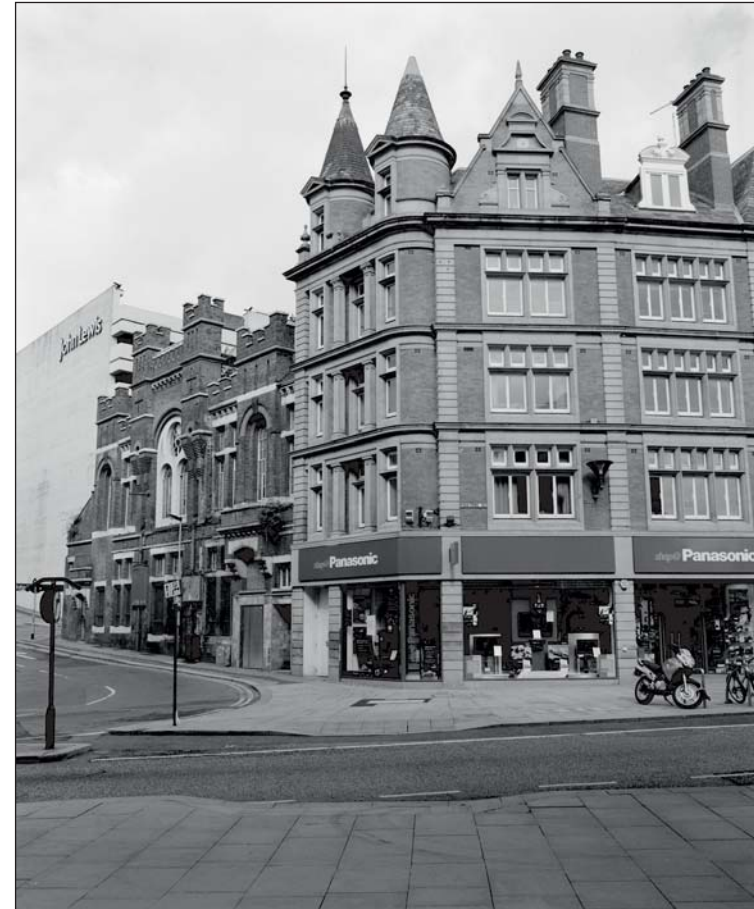
Plate 250: View of the principal east facing elevation of Building 38 at the south corner, Pinstone Street and the south facing elevation, Cross Burgess Street, looking west (ARCUS 2008)
