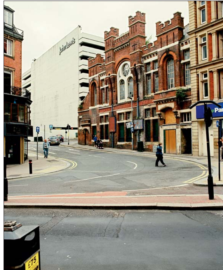
Plate 216: Oblique view of the principal south facing elevation of the Grade II Listed Building 'Salvation Army Citadel', Cross Burgess Street (ARCUS 2008)
