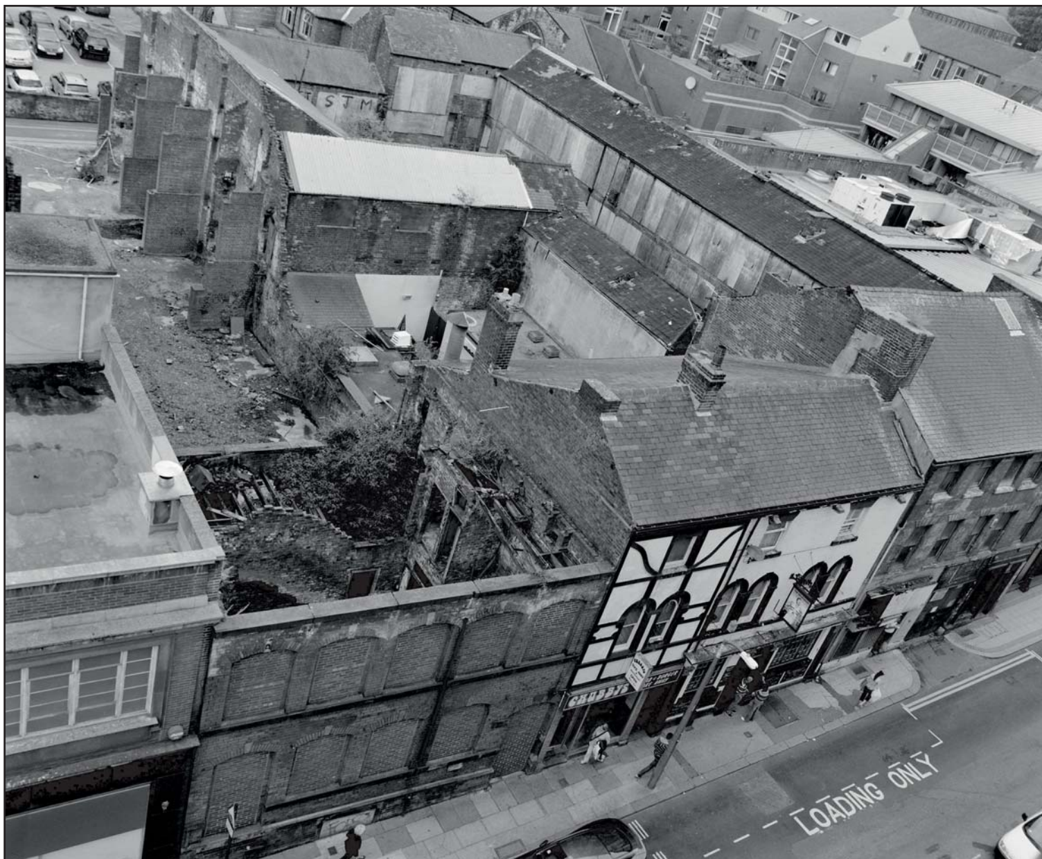
Plate 98: General elevated view across Buildings 16, 15, 14 and 13 showing some internal detail and yard space, looking north-west from the roof of 'John Lewis', Building 33 (ARCUS 2008)
