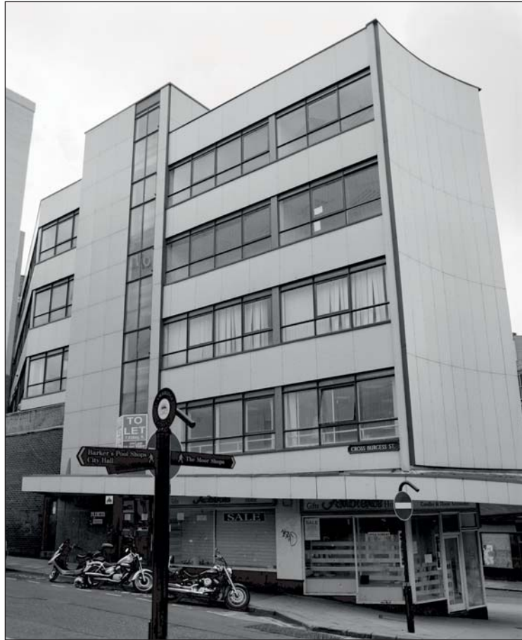
Plate 186: Oblique view of the north facing elevation of Building 27, Cross Burgess Street, looking south-east (ARCUS 2008)
