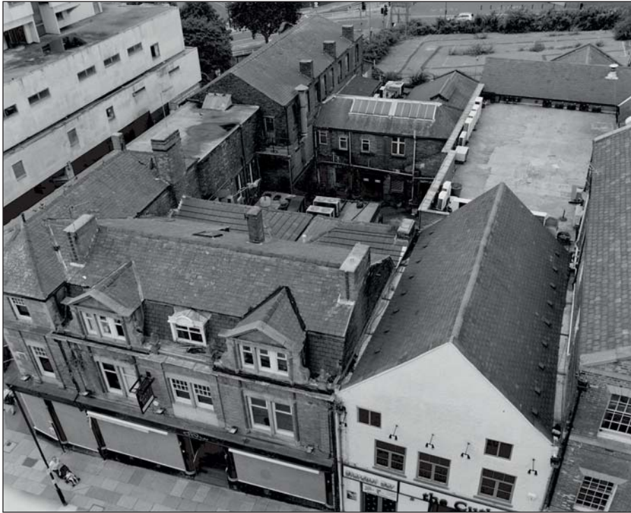
Plate 90: Elevated view of Buildings 20a, 20b and 19 showing enclosed rear yard with Building 22 beyond from the roof of 'John Lewis', Building 33 (ARCUS 2008)
