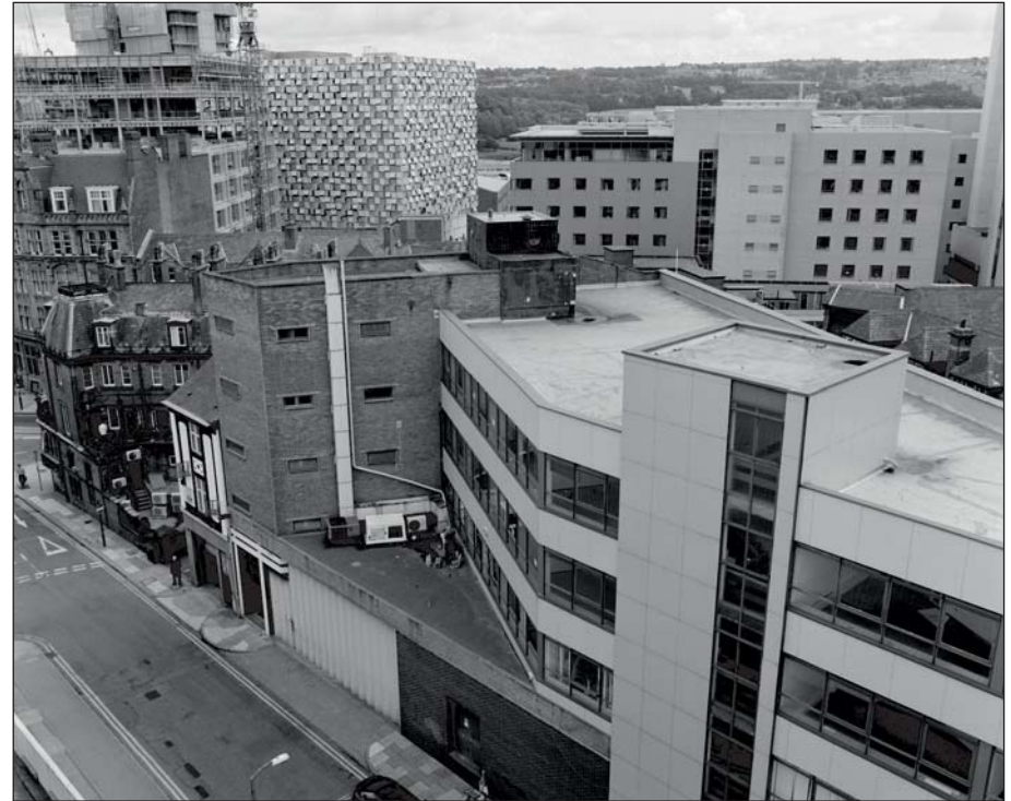
Plate 187: Elevated oblique view of the north facing elevations of Buildings 27, 28 and 30, Cross Burgess Street from the roof of 'John Lewis', Building 33 (ARCUS 2008)
