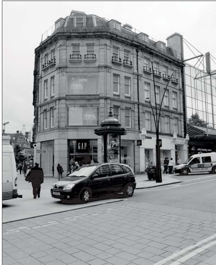
Plate 237: Oblique view of the north facing elevation of Building 36, Barker's Pool, looking south-west (ARCUS 2008)
