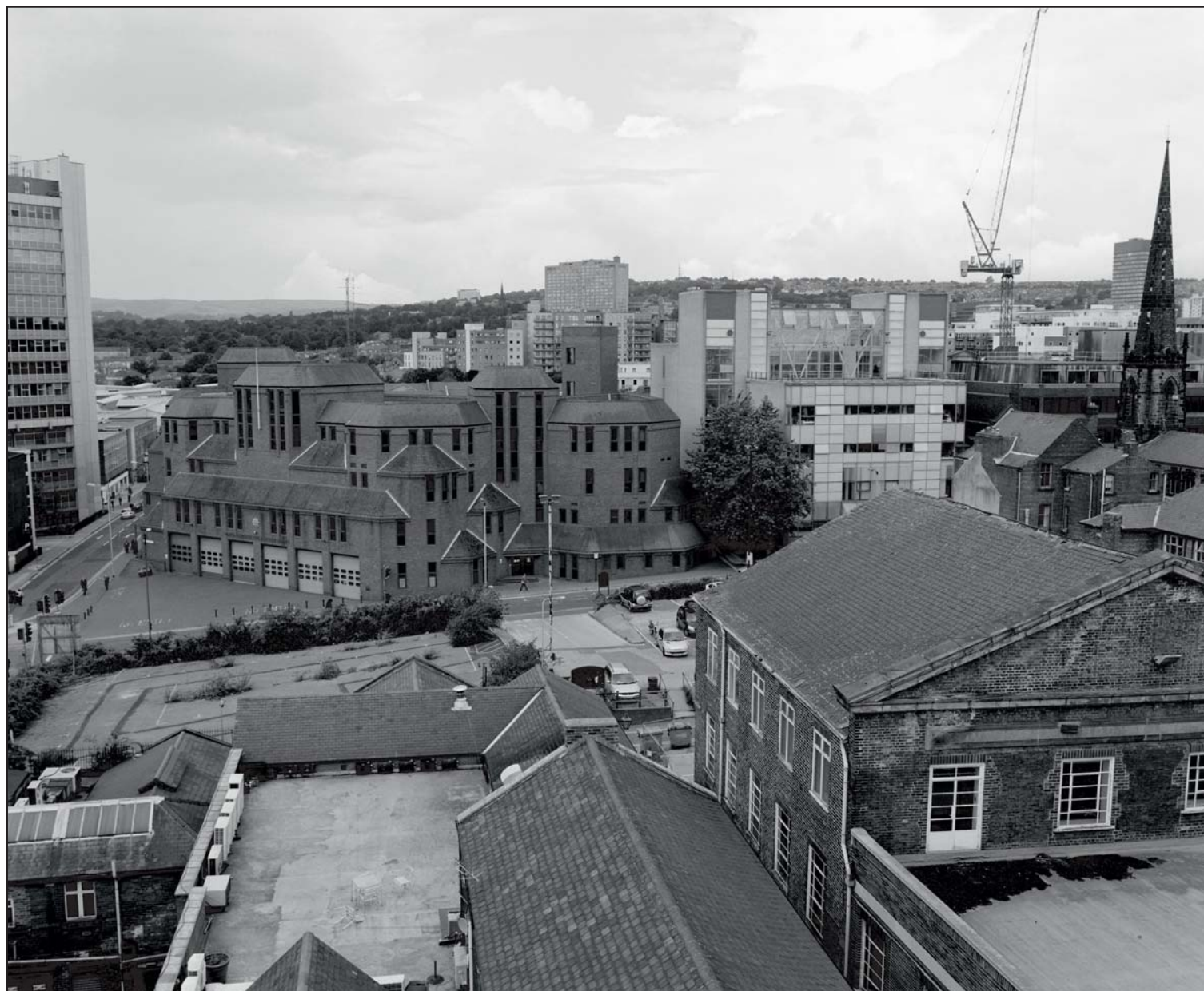
Plate 57: Elevated view of Buildings 11, 12 and 41 with Buildings 19 and 17b in the foreground from the roof of 'John Lewis', Building 33 (ARCUS 2008)
