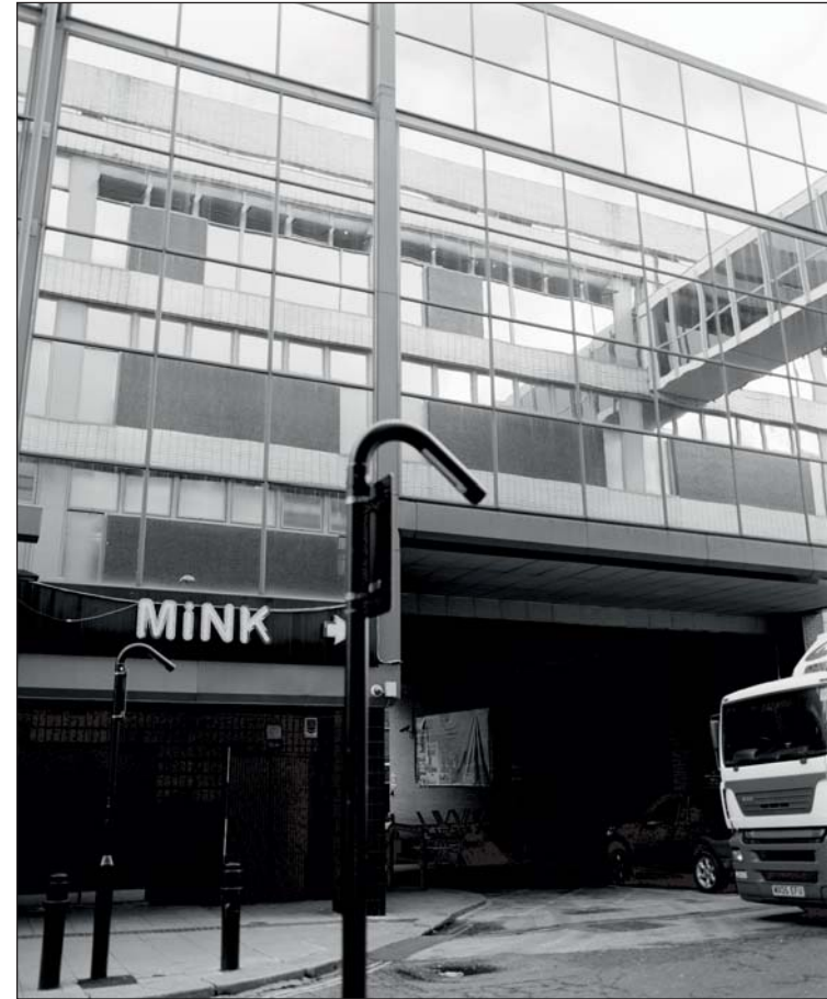
Plate 228: Oblique view of the west facing elevation of Building 35 at the south end, Burgess Street, showing vehicular access (ARCUS 2008)
