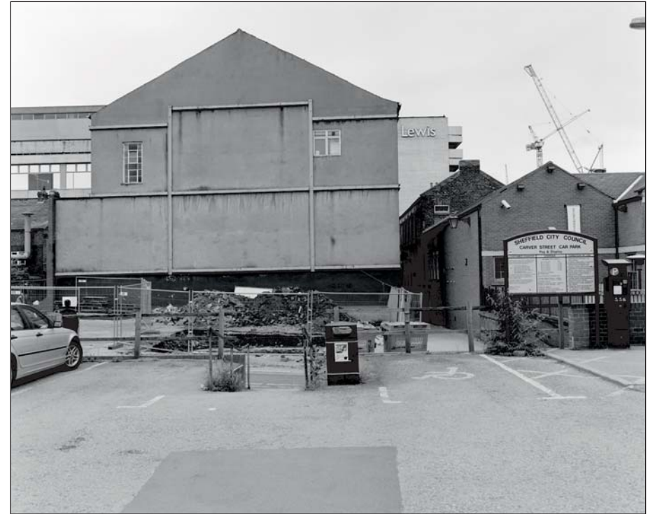
Plate 66: View of the west facing elevation of Building 17b showing Bethel Walk to the south (ARCUS 2008)
