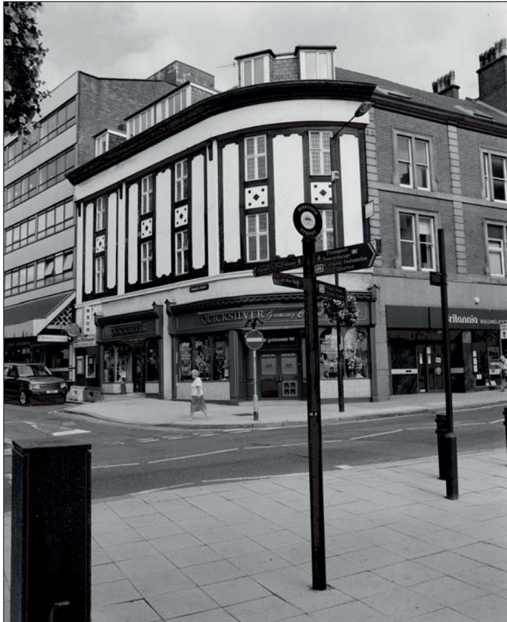
Plate 196: View of the south corner of the 'Athol Hotel' Building 28 at the junction of Pinstone Street and Charles Street, looking north (ARCUS 2008)
