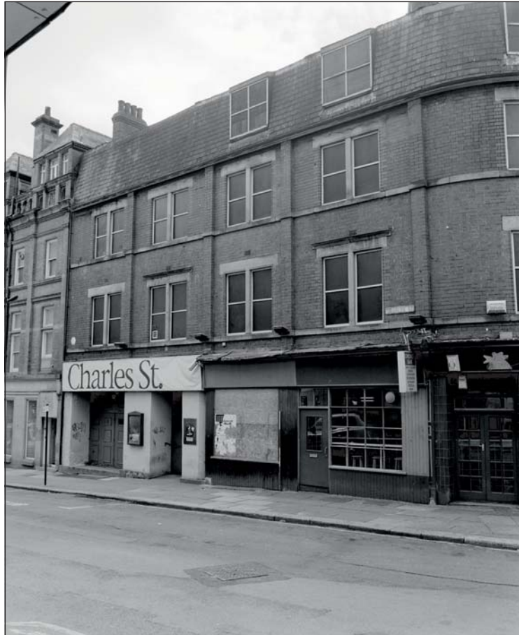
Plate 184: Oblique view of the north-east facing elevation of Building 24 showing various retail units, Charles Street, looking south (ARCUS 2008)
