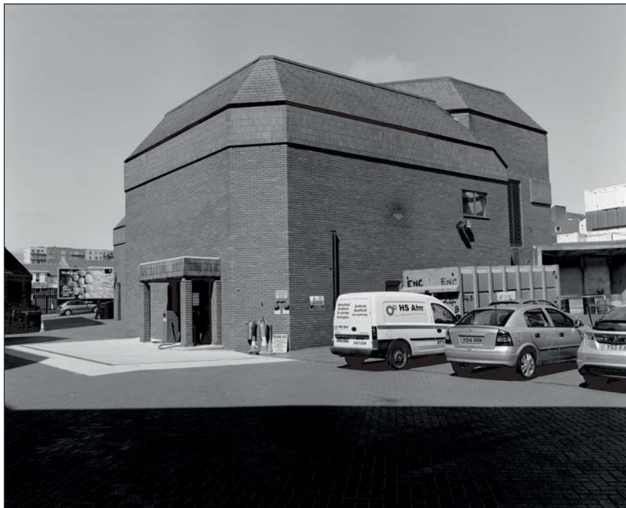
Plate 38: Oblique view of south and east facing elevations of Building 11 (ARCUS 2008)
