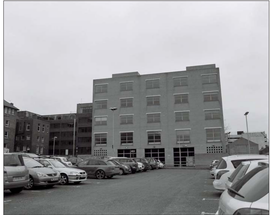
Plate 51: View of the west facing elevation of Building 41 (Wessex Archaeology 2016)
