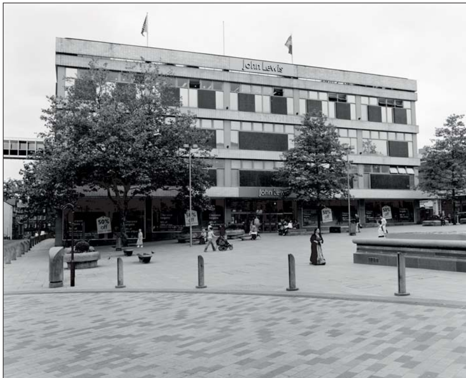
Plate 117: Oblique view of the principal north facing elevation of 'John Lewis', Building 33, Barker's Pool (ARCUS 2008)
