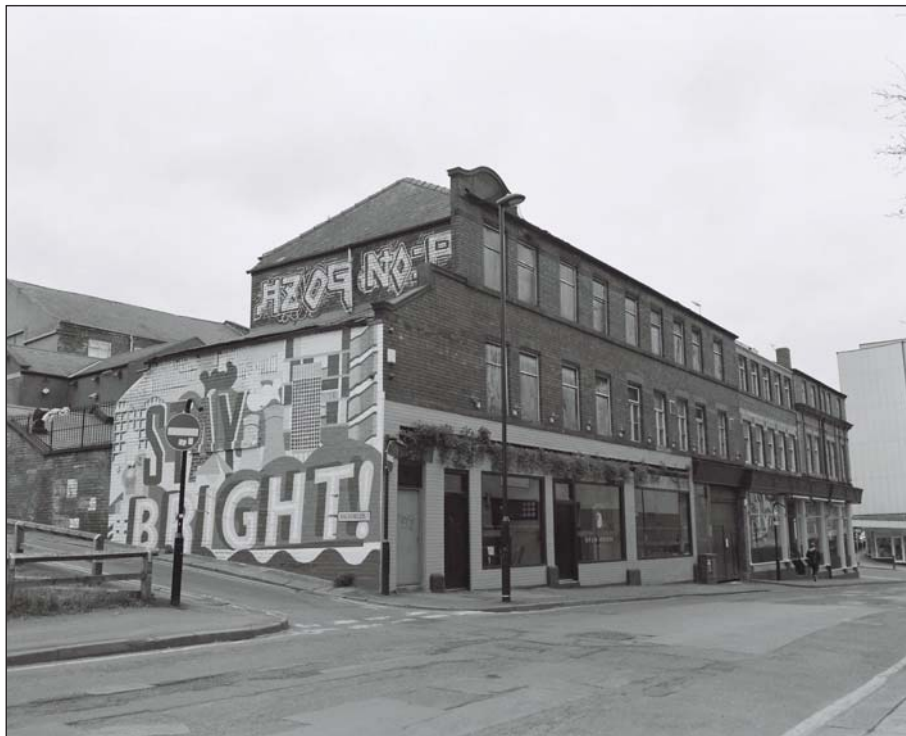
Plate 76: Oblique view of the south and west elevations of Building 22 showing Building 21 and 20b beyond (Wessex Archaeology 2016)
