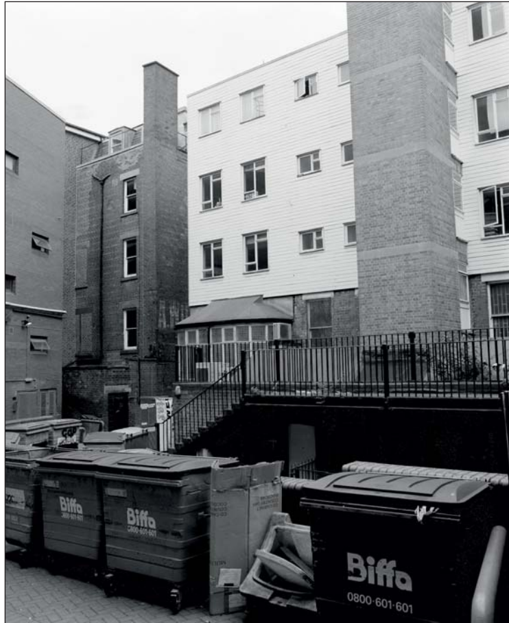
Plate 245: Oblique view of the rear elevations of Buildings 36 and 40, looking north-east (ARCUS 2008)
