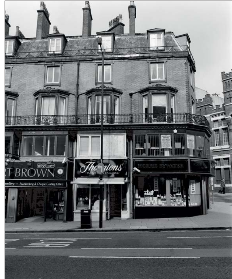
Plate 201: View of the south-east facing elevations of Building 30 showing various retail units, Pinstone Street (ARCUS 2008)
