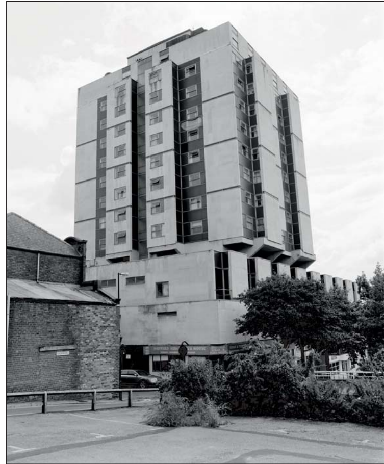
Plate 163: Oblique view of the north facing elevation of the 'Grosvenor Hotel' accommodation to Building 23, looking south-east (ARCUS 2008)
