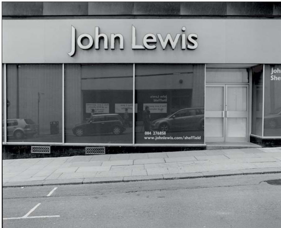
Plate 95: Detail of the principal entrance to 'John Lewis', Building 17a (ARCUS 2008)
