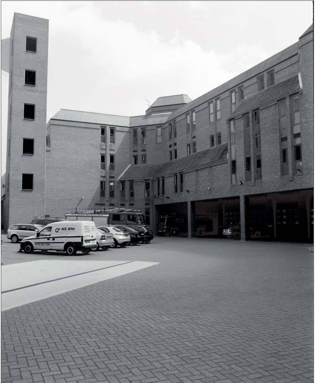
Plate 36: View of the south-west corner of Building 12, looking north-east (ARCUS 2008)
