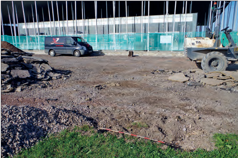
Plate 22: Area 6: Removal of temporary hardstanding
