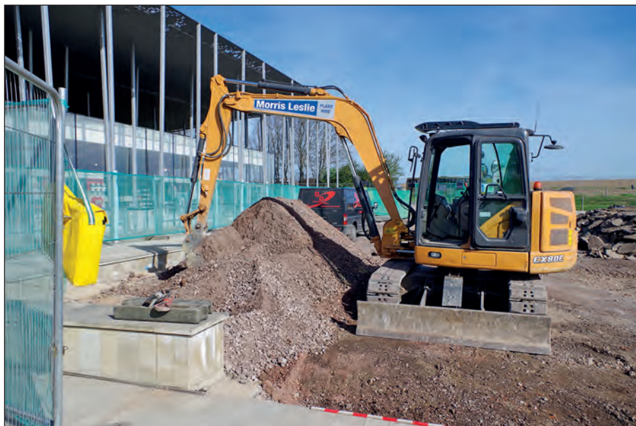
Plate 23: Area 6: Removal of temporary hardstanding
