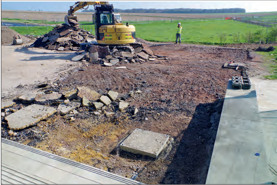
Plate 21: Area 6: Removal of temporary hardstanding
