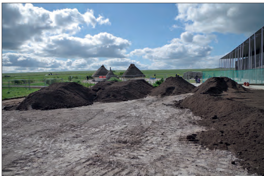
Plate 24: Area 6: Stored topsoil awaiting spread
