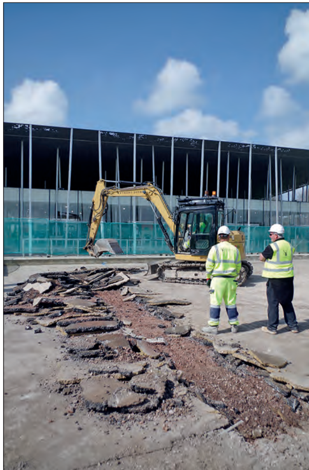
Plate 20: Area 6: Removal of temporary hardstanding
