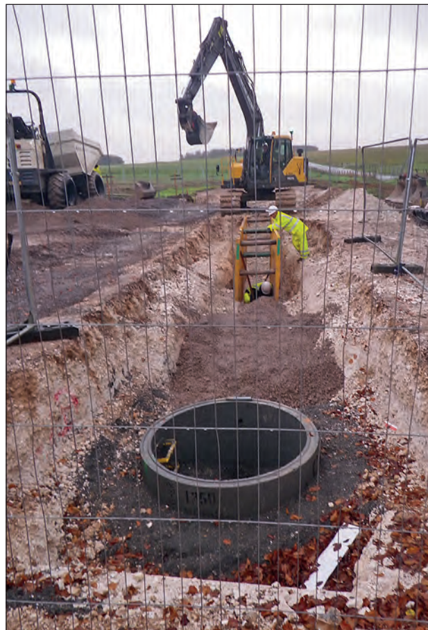
Plate 6: Area 2: Surface water drainage trenching
