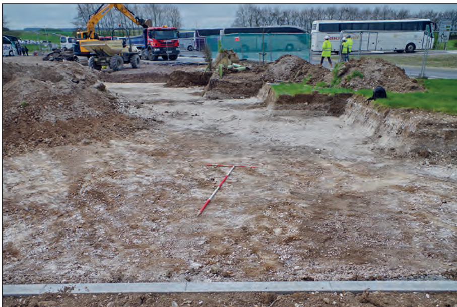
Plate 8: Area 2: Western edge of coach bays, showing made ground.
