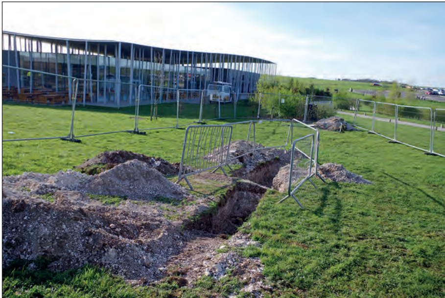
Plate 29: Area 10: Prospection for existing services
