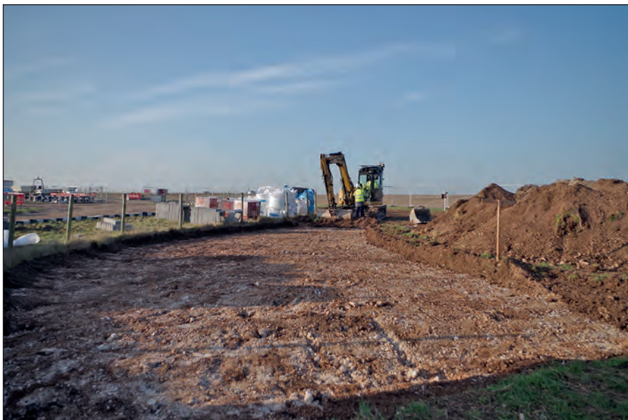
Plate 28: Area 8: Stripped area looking north
