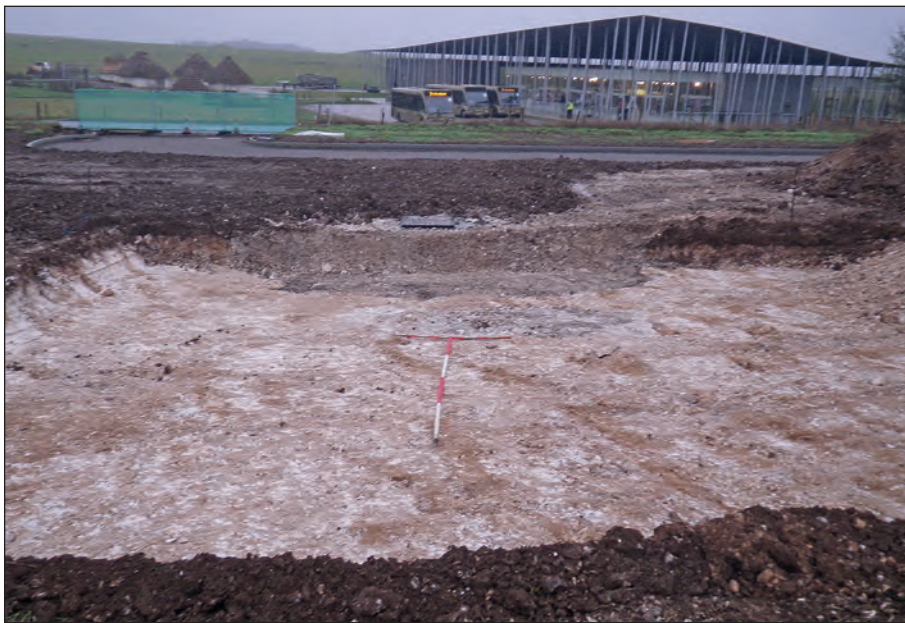
Plate 14: Area 3: Stripped area for tank
