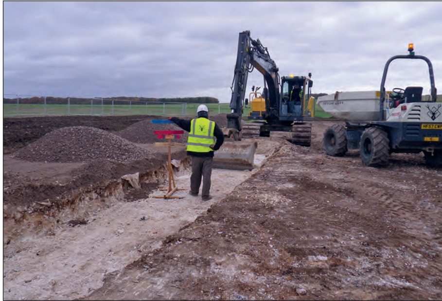
Plate 5: Area 2: Surface water drainage trenching
