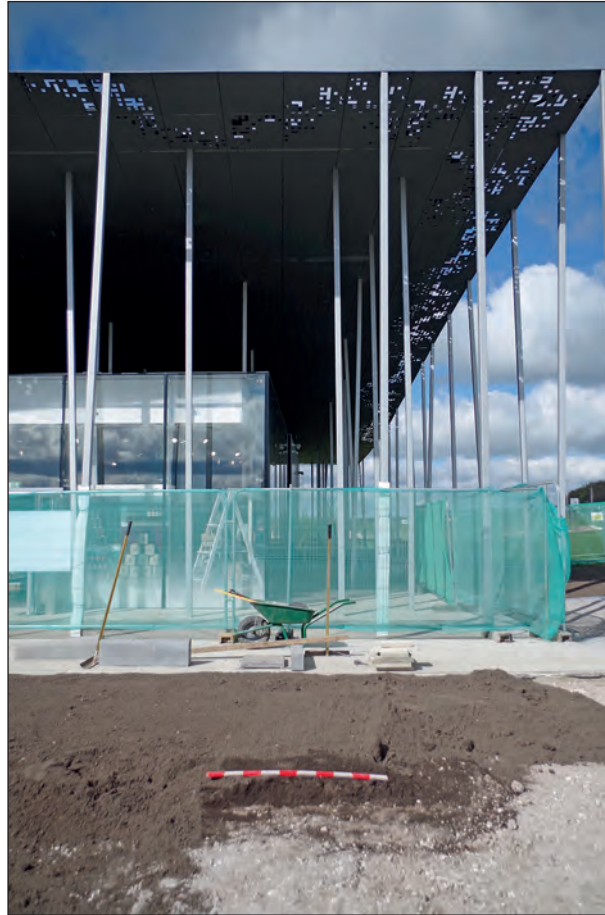
Plate 25: Area 6: Topsoil spreading
