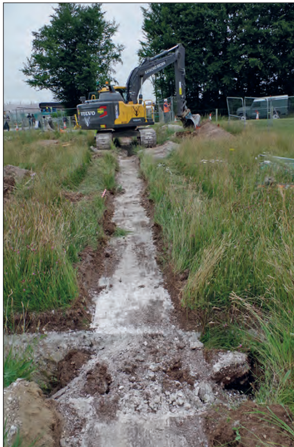
Plate 30: Area 10: Service trench strip
