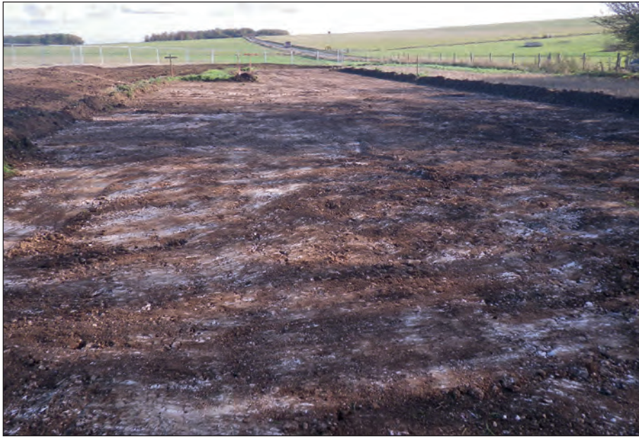
Plate 3: Area 2: General shot of stripping, facing east
