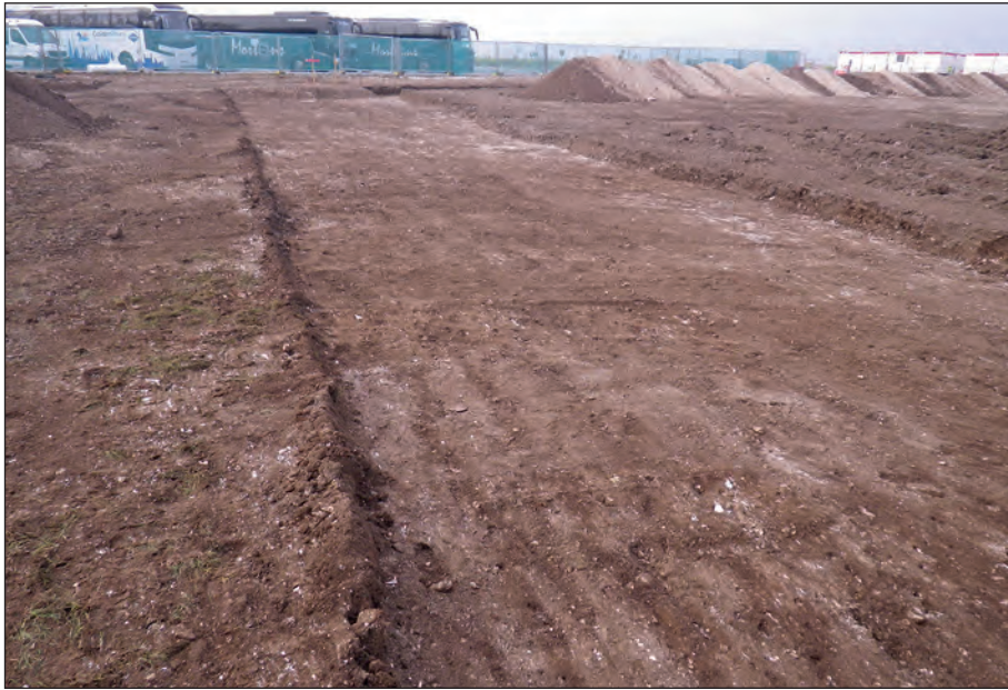
Plate 9: Area 3: Stripping to formation level
