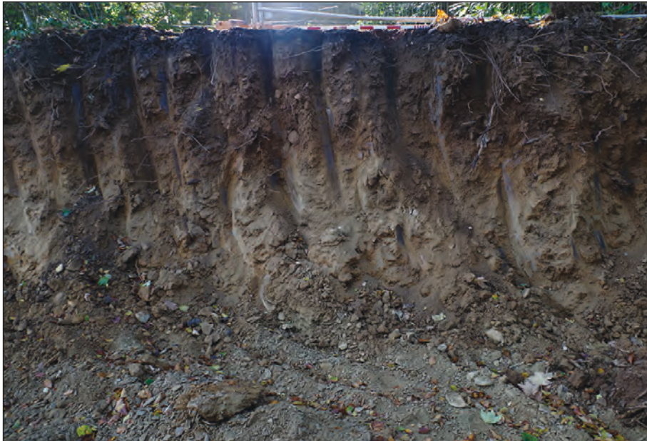
Plate 4: South-east facing view of deposits exposed in section within footprint of working platform / embankment (scale: 1 x 1 m)
