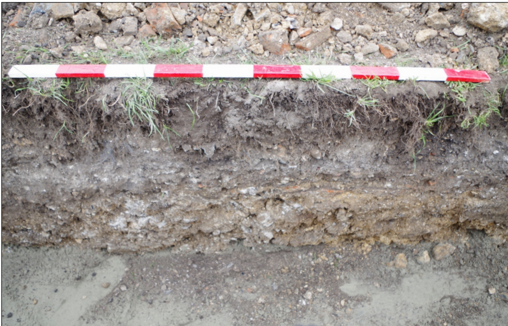
Plate 4: South facing representative section of made ground and soil sequence (1 x 1 m)
