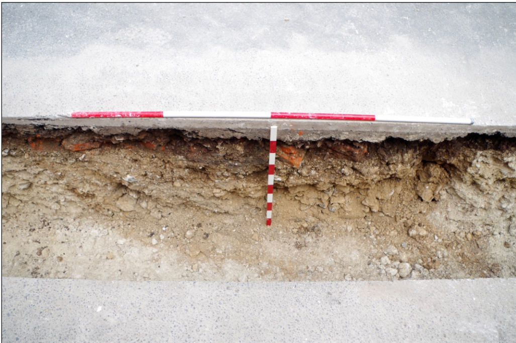
Plate 6: South-east facing section of wall footing 105 continuing into the base of trench (1 x 1 m, 1 x 2 m)
