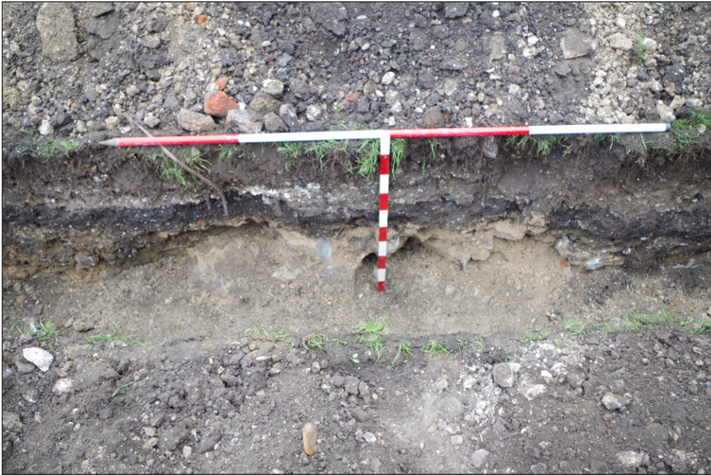
Plate 9: South-west facing section of wall footing 133 (1 x 1m, 1 x 2 m)
