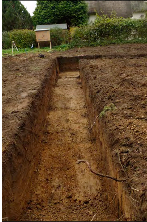
Plate 1: Southern foundation trench to formation level, view looking west.
