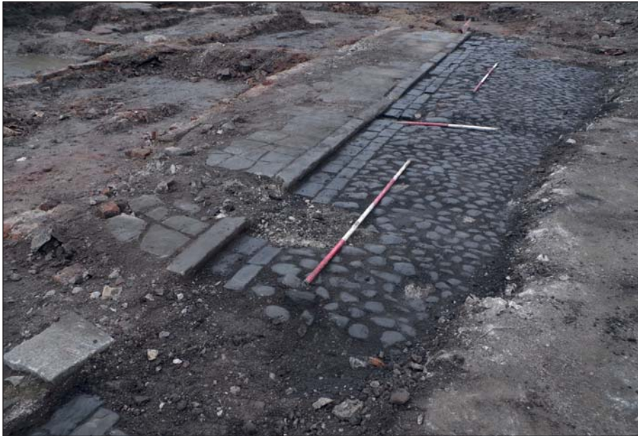
Plate 17: Cobble surface of Victor Road 1103 (constituent 126) with gutter 127, kerb 125 and pavement 124. View from north-west
