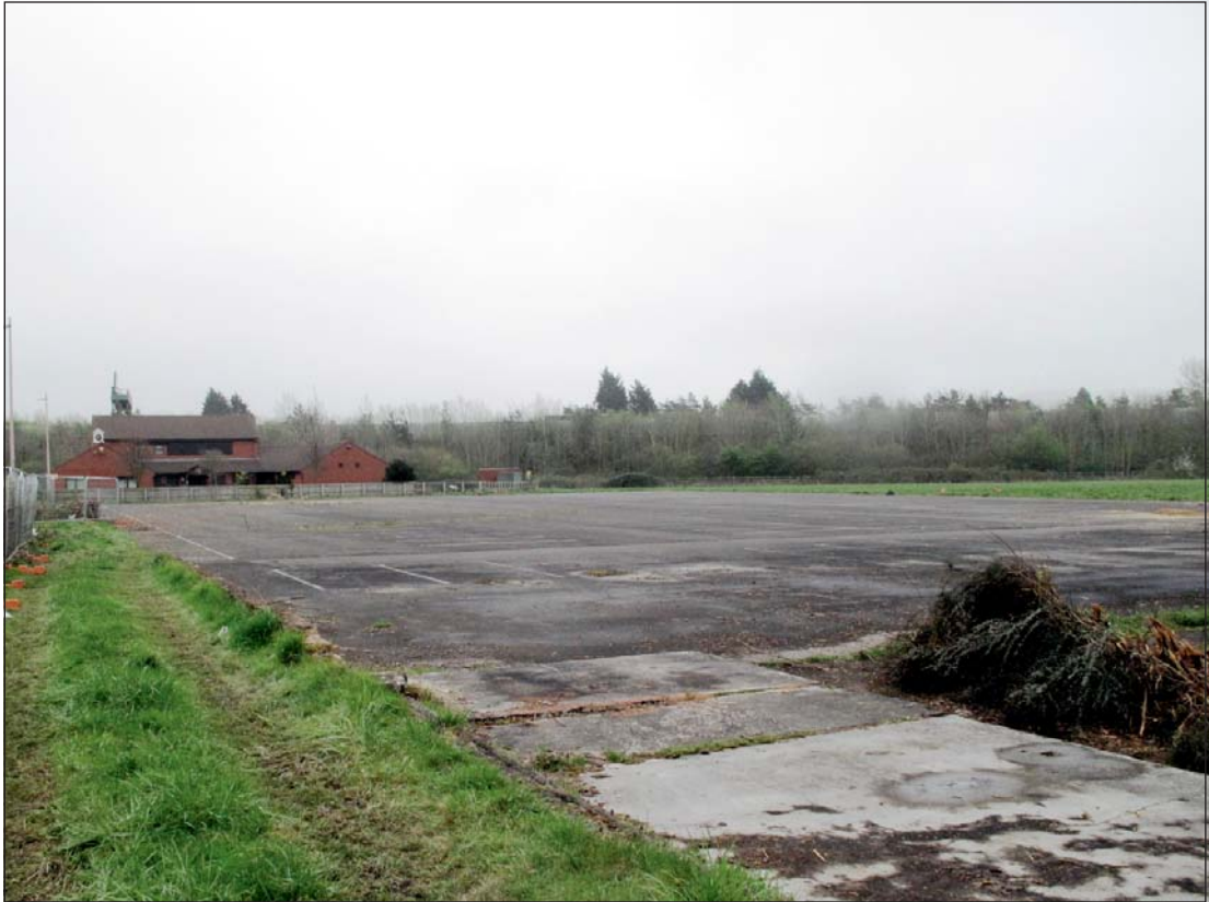
Plate 15: Area of hardstanding to the east - formerly a school playground and tennis courts
