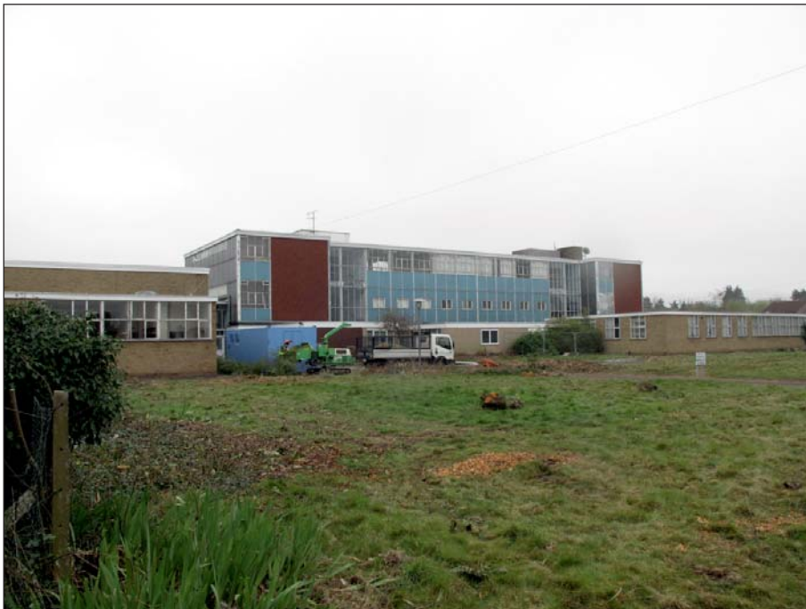
Plate 2: Hucclecote Centre viewed from the north-west
