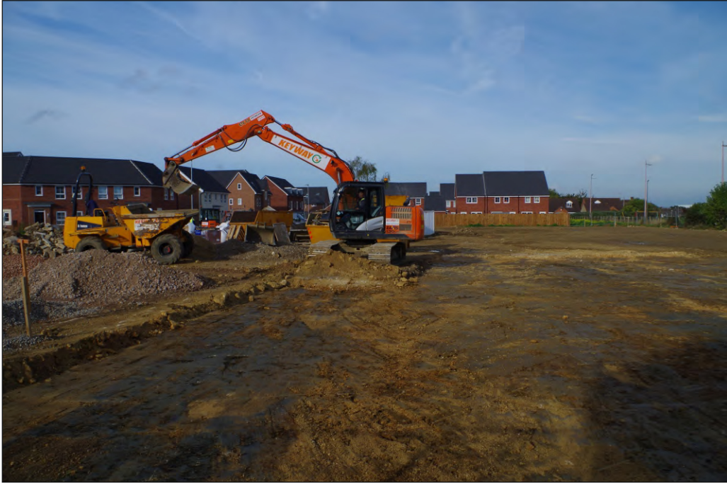
Plate 1: General view of ground reduction in the new rugby pitch area
