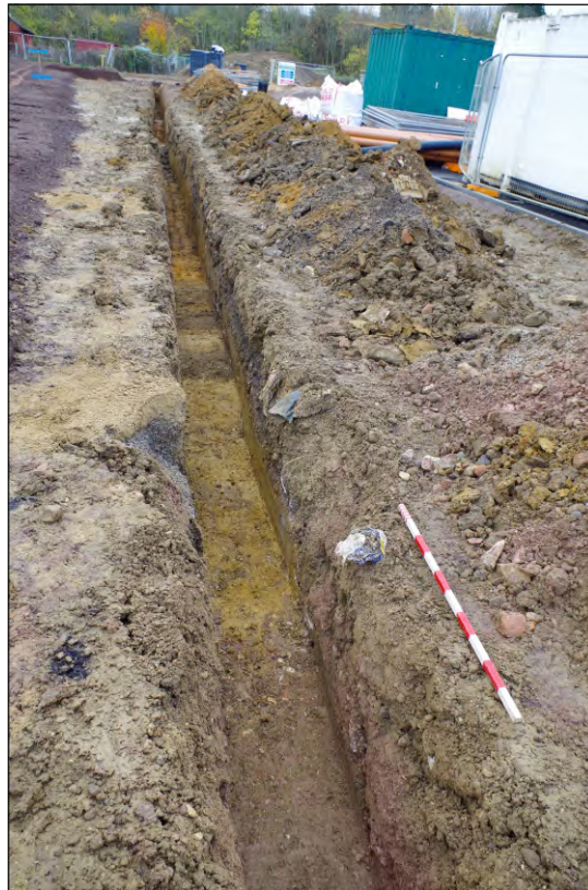
Plate 2: Drainage trench showing ditches 9002, 9004, 9006 and 9008, looking south-east
