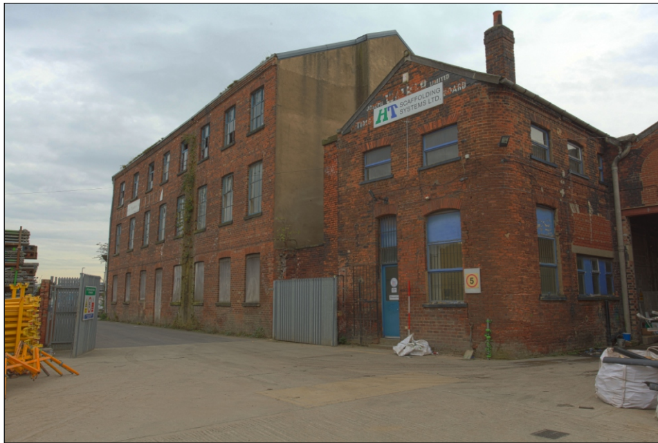
Plate 27: Oblique view of the north elevations of the north-east and central ranges, looking south-east (Film 4.02)
