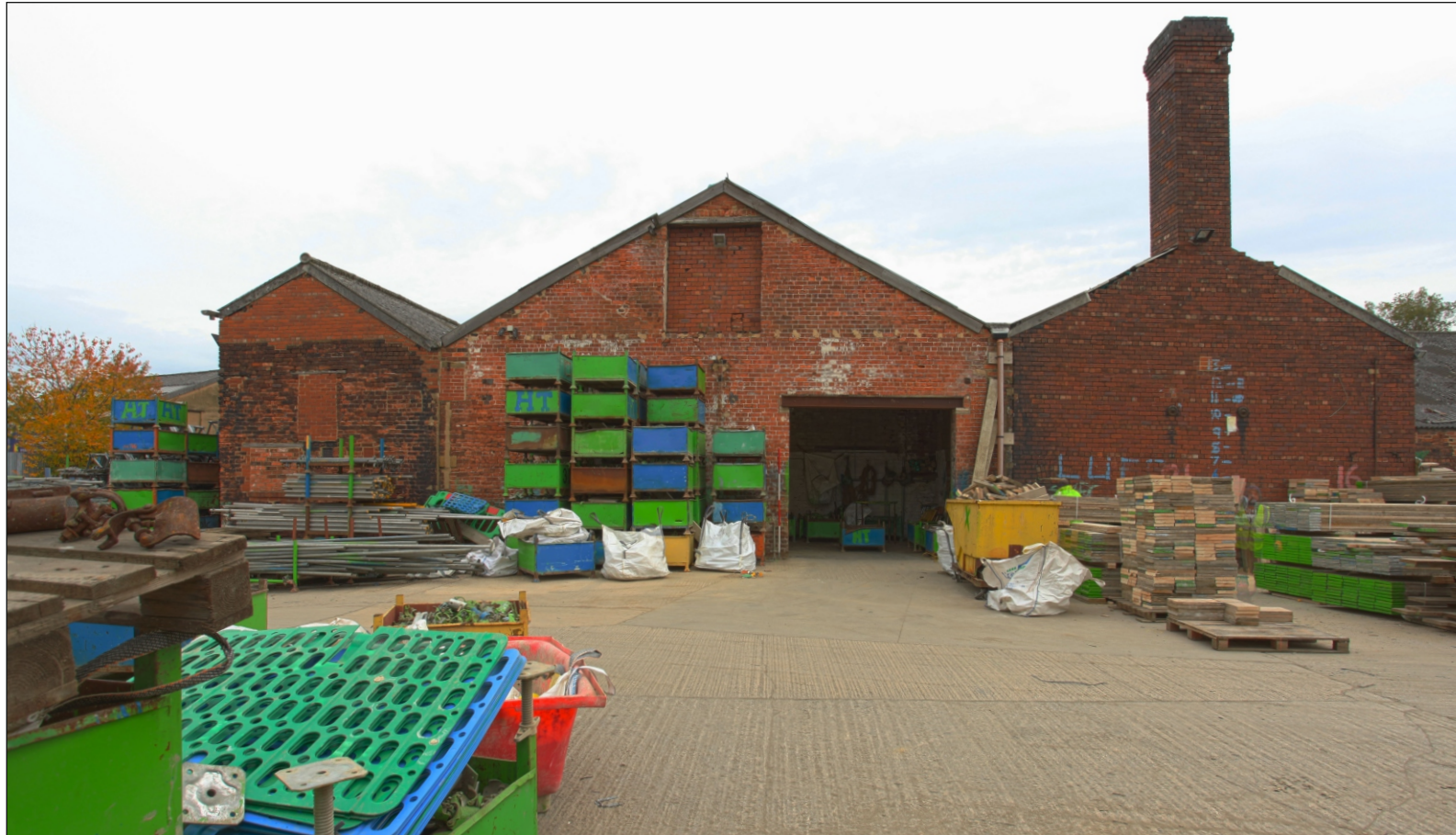
Plate 34: View of the west elevations of the west ranges (Film 4.07)
