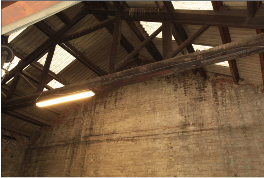
Plate 53: Detail of a queen post roof truss with princesses in G3 (Film 1.24)
