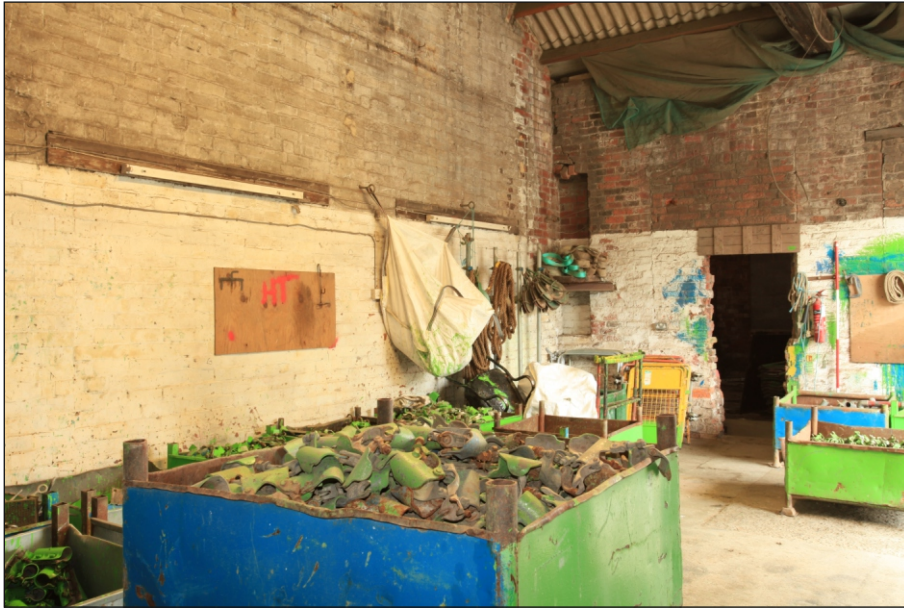
Plate 51: General view of G3, looking south-east (Film 5.06)
