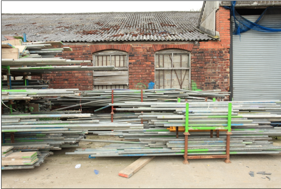
Plate 41: Detail of blocked windows in the west elevation of the south-west range (Film 1.27)
