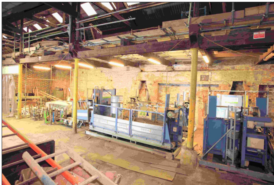
Plate 71: General view of the east aisle of G6, looking north-east (Film 6.03)
