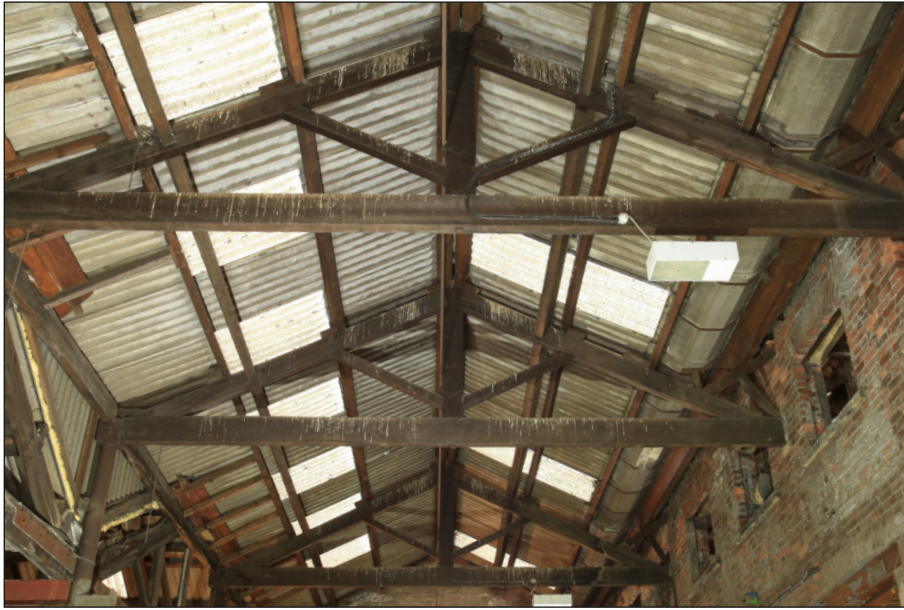
Plate 81: Detail of king post roof trusses in G6 (Film 2.26)
