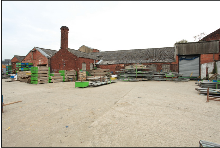
Plate 37: View of the west elevations of the west and south-west ranges (Film 4.09)
