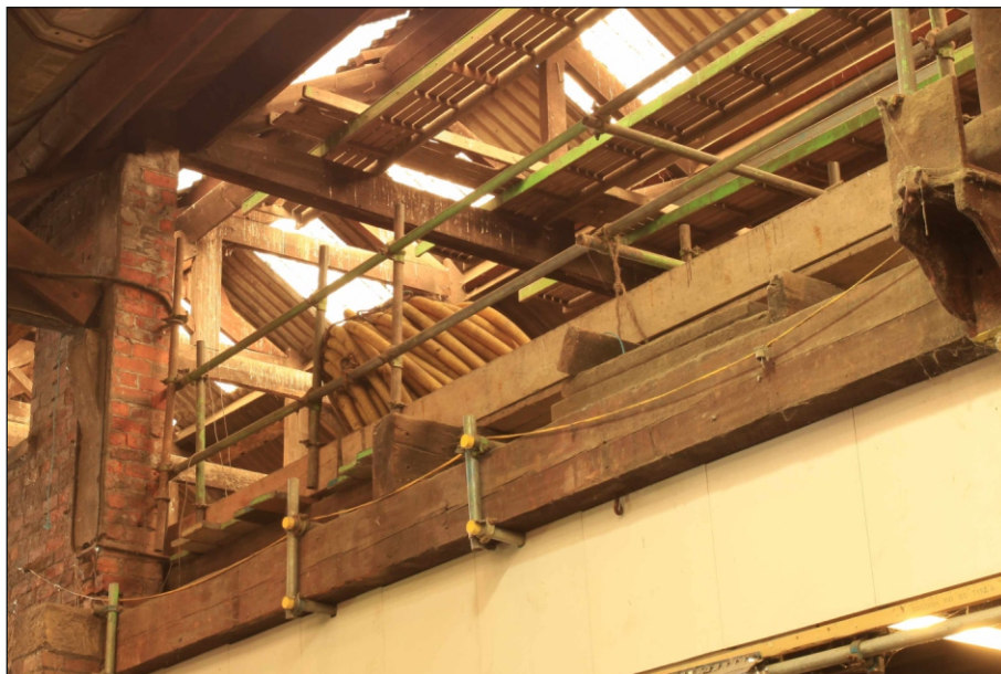
Plate 80: General view of FF6 above the G14, G15 and G6, showing queen post roof trusses, looking north-east (Film 2.32)
