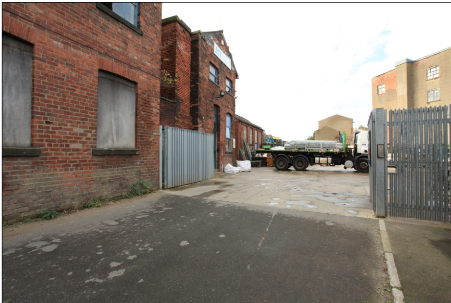
Plate 26: Oblique view of the north elevations of the central and west ranges, looking south-west (Film 2.08)
