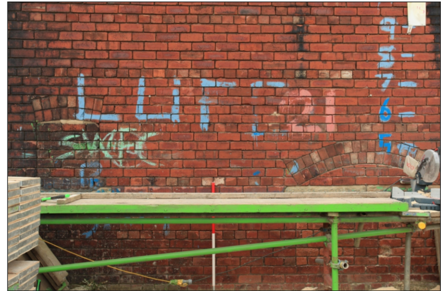
Plate 36: Detail of the west elevation of the west ranges at the south end, showing blockings (Film 1.25)
