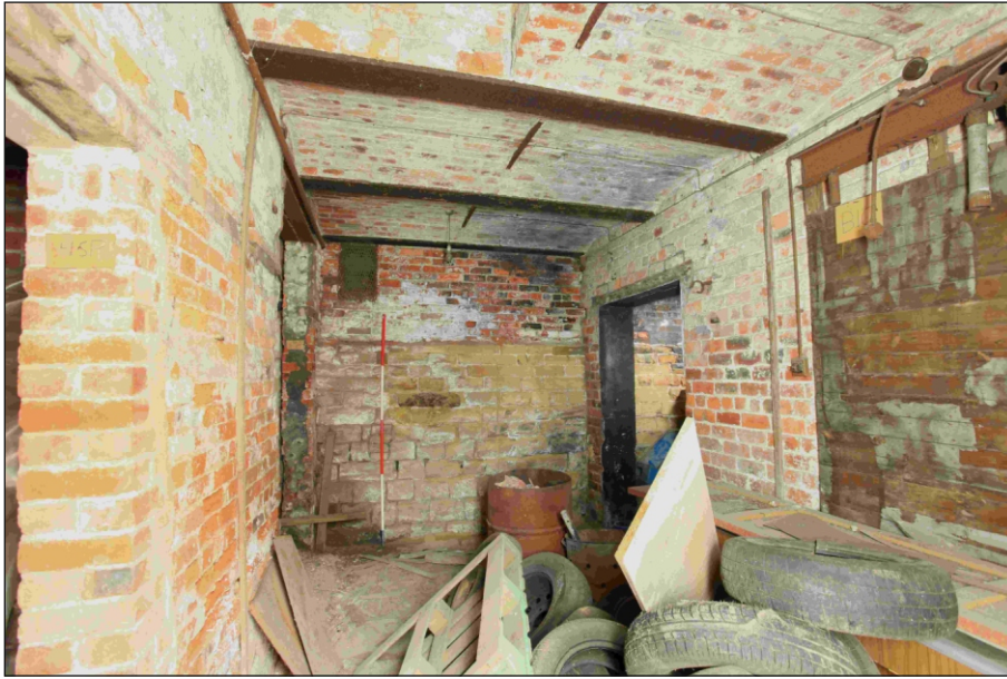
Plate 11: General view of G21, looking west (Film 1.30)
