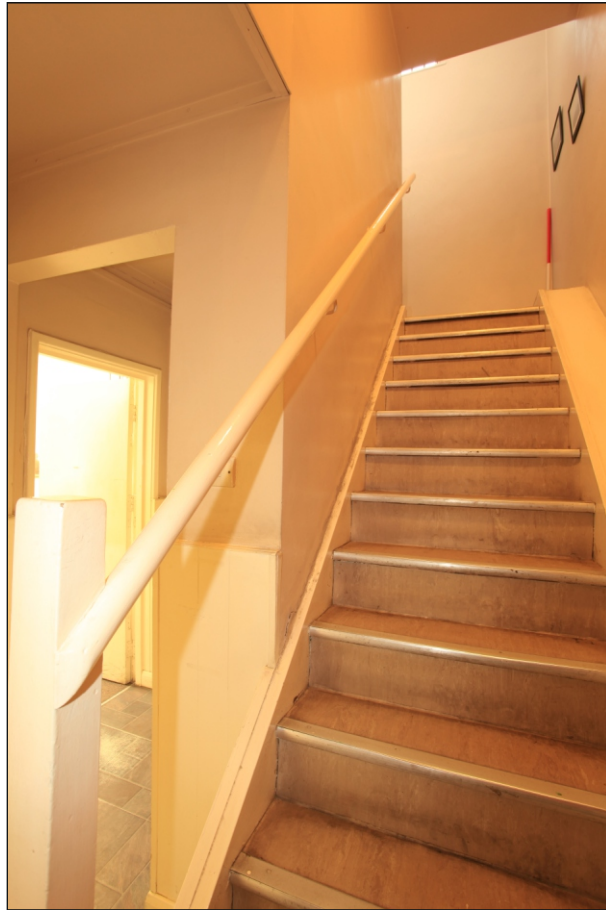
Plate 97: View of staircase in G9 leading to first floor level FF1, looking north (Film 7.04)
