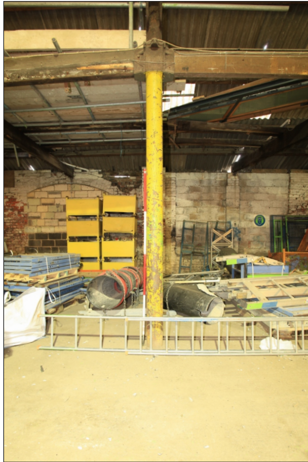
Plate 74: Detail of a typical cast-iron column in G6 (Film 2.29)
