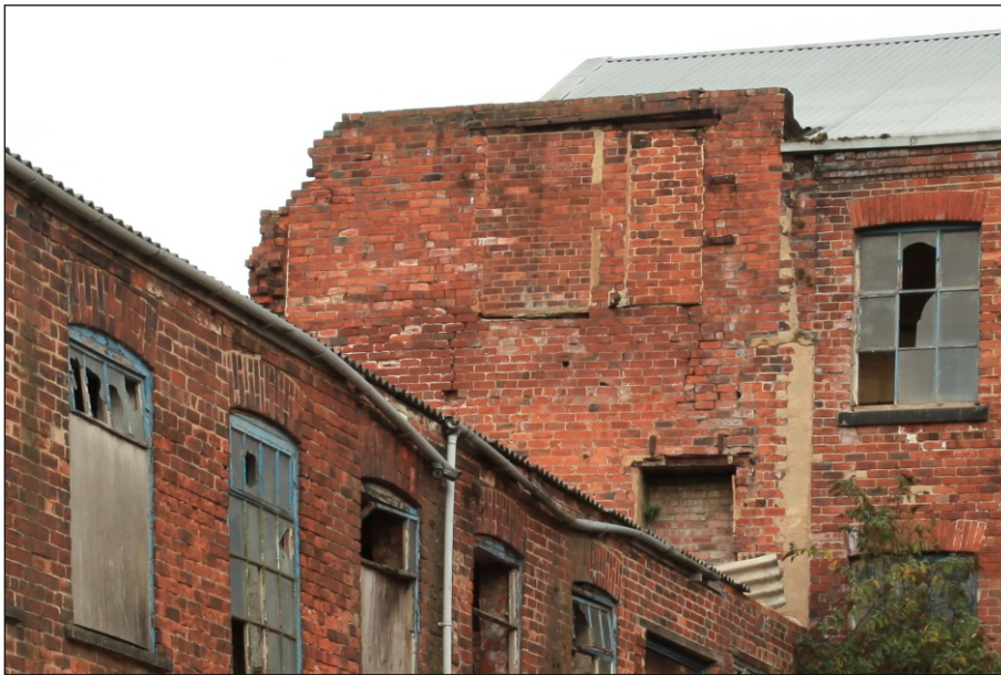
Plate 24: View of remains of the north wall to the second and third floors of the east range, since removed (Film 1.35)
