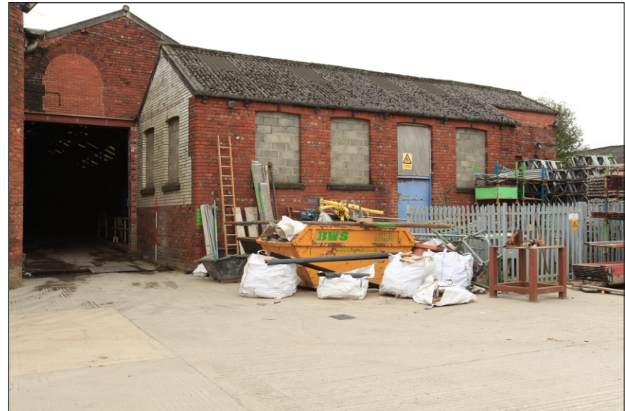
Plate 30: Oblique view of the north and east elevations of the north-west extension showing blocked opening and glazed brick detailing, looking south-west (Film 4.03)
