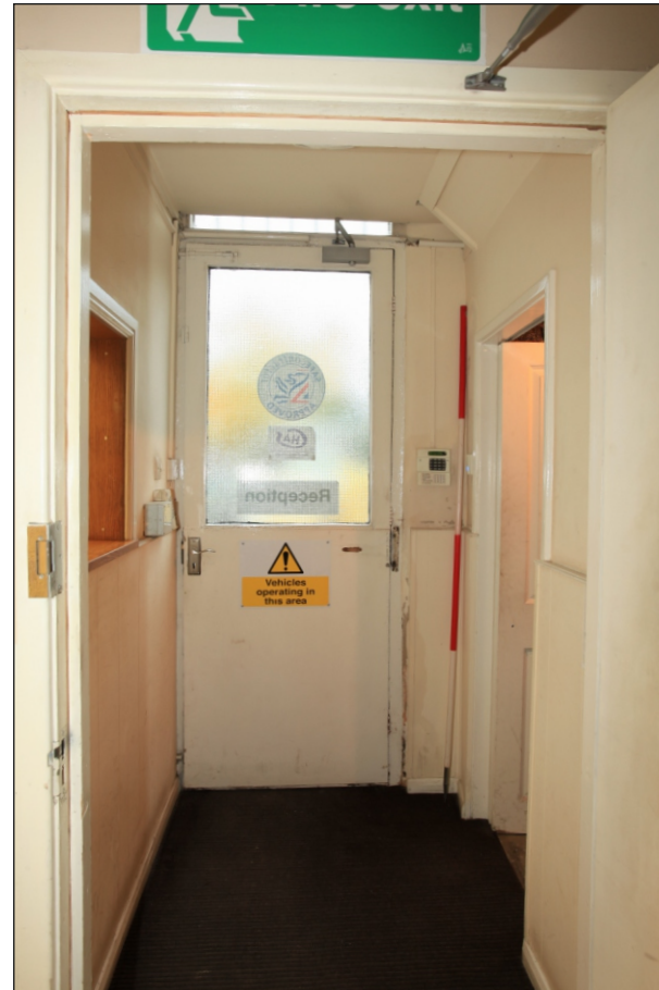
Plate 84: General view of porch to G9, looking north (Film 1.06)
