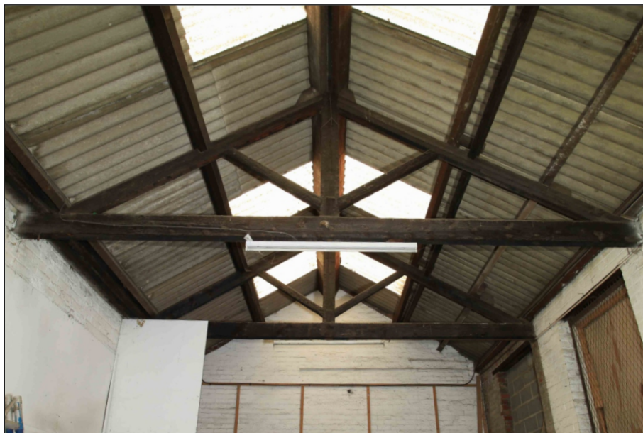
Plate 48: Detail of king post roof trusses in G2 (Film 1.22)
