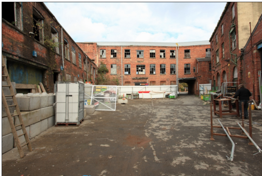
Plate 2: View of the central yard to the historic 'Low Hall Mills' looking north, showing the east range of the Site to the left of the picture (Film 2.10)
