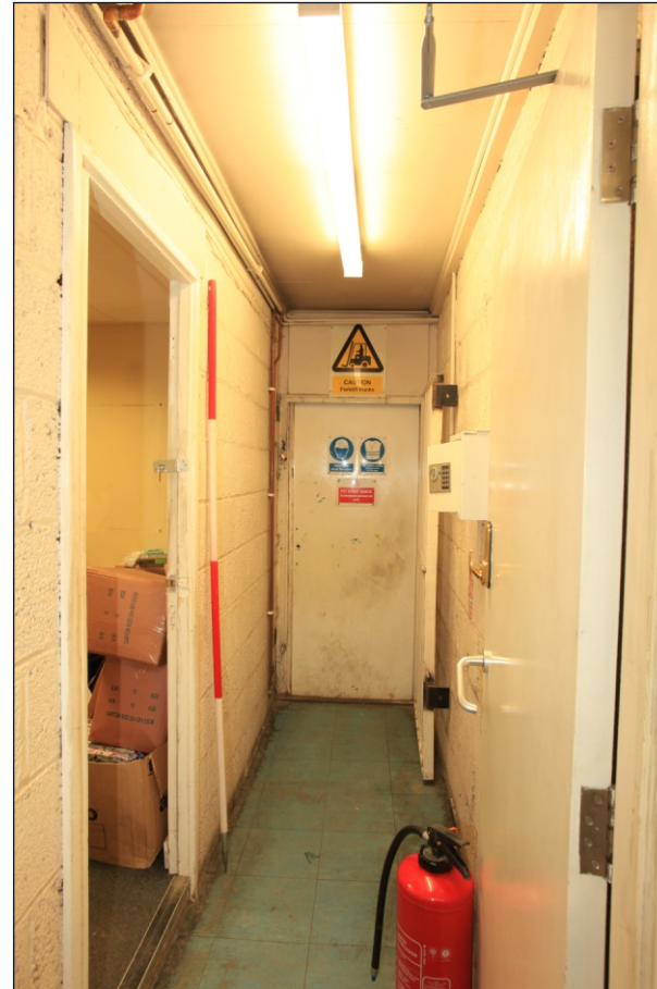
Plate 92: General view looking west of corridor leading from G13 to G6 (Film 1.02)
