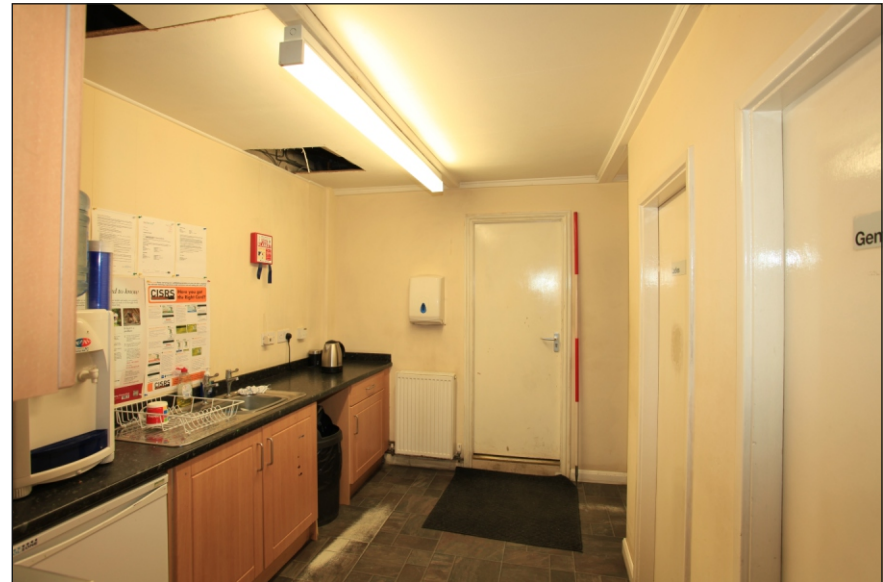
Plate 90: General view of kitchenette G13, looking south (Film 1.04)
