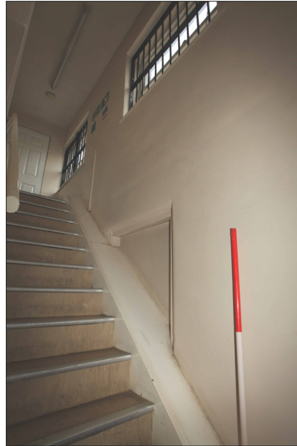
Plate 98: View of the staircase in FF1 at mezzanine level showing blocked transom light (Film 1.12)
