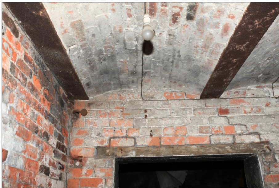
Plate 14: Detail of profile of jack-arched ceiling in G21 (Film 1.33)
