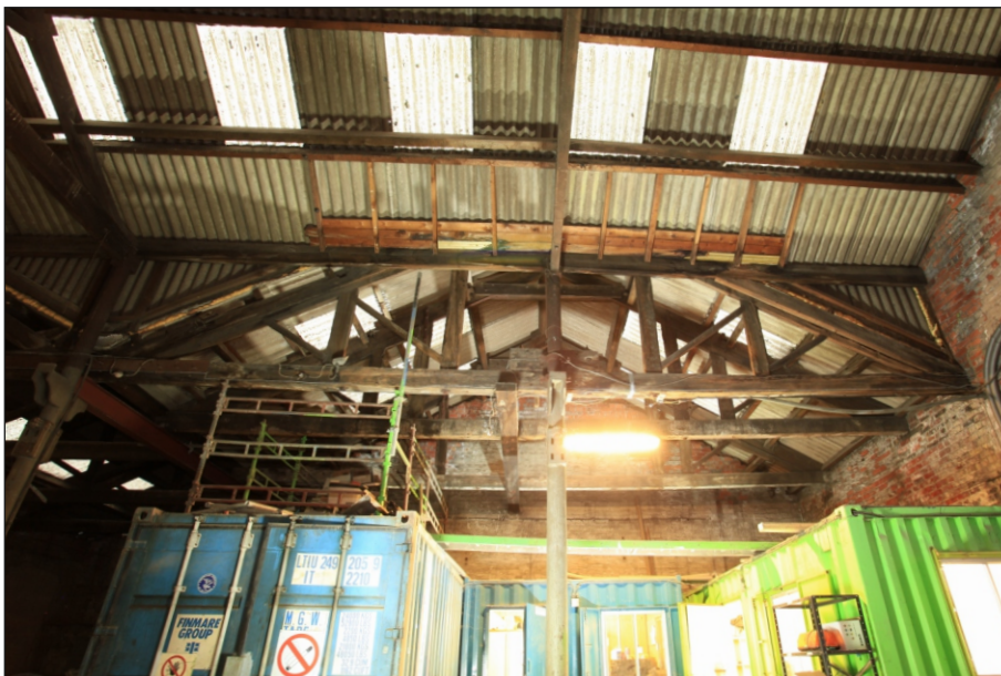
Plate 61: Detail of queen post roof trusses with princesses in G4 (Film 2.25)
