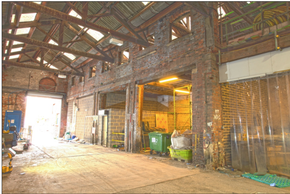
Plate 62: Oblique view of the former west elevation of the central range at the north end of G6 showing extensive alteration (Film 6.08)
