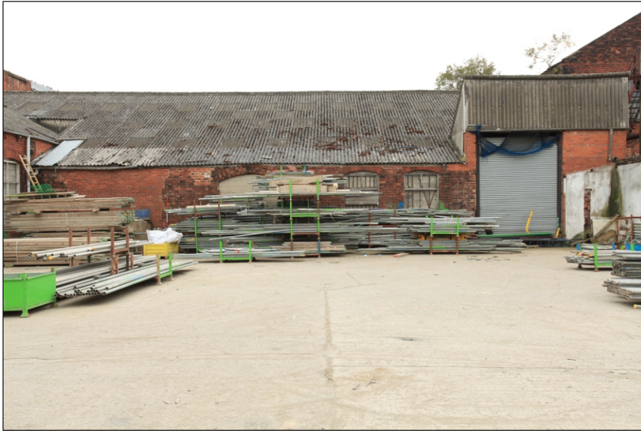
Plate 39: View of the west elevation of the south-west range (Film 4.08)
