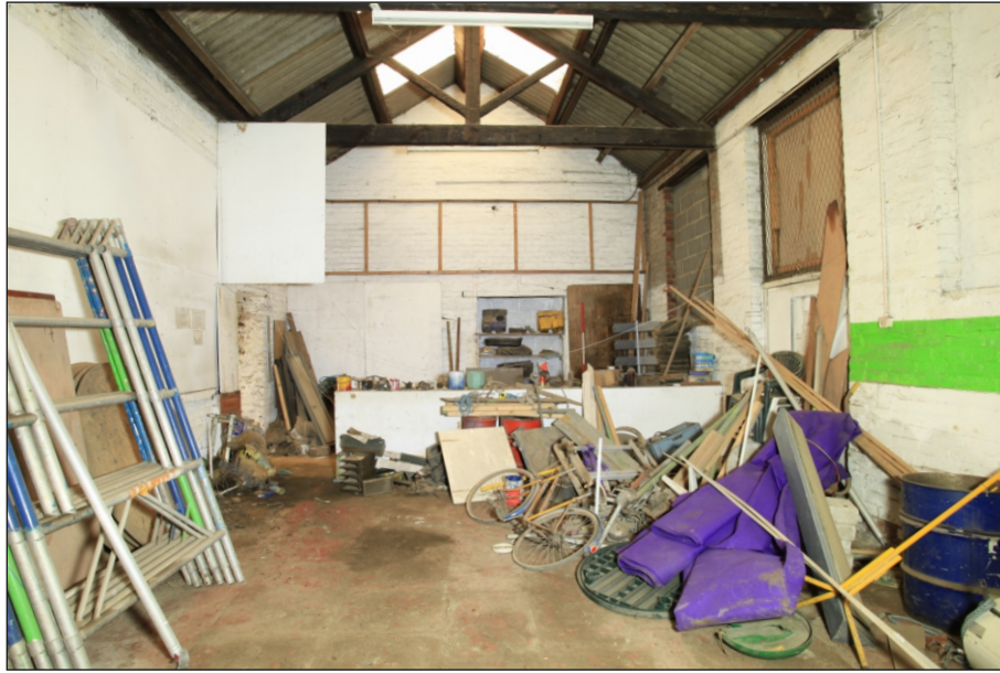
Plate 47: General view of G2, looking north-west (Film 5.08)
