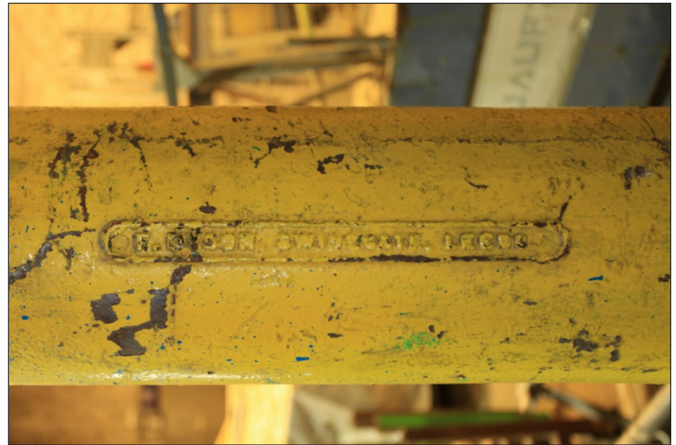
Plate 75: Detail of makers mark 'F. DYSON SWINEGATE, LEEDS' on cast-iron column in G6 (Film 2.30)
