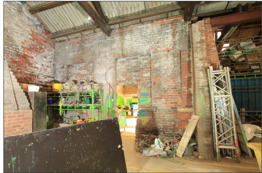
Plate 56: Detail of the north wall of G5 showing blockings (Film 1.19)
