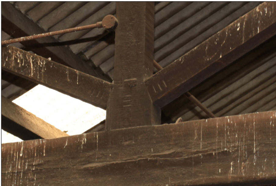
Plate 82: Detail of carpenters marks in king post roof trusses in G6 (Film 2.02)
