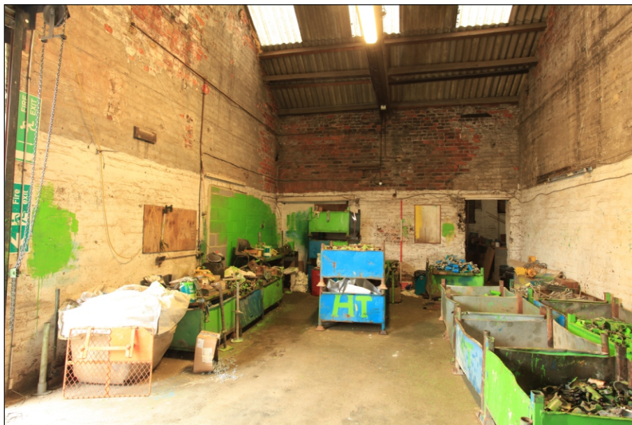
Plate 50: General view of G3, looking north-west (Film 5.05)
