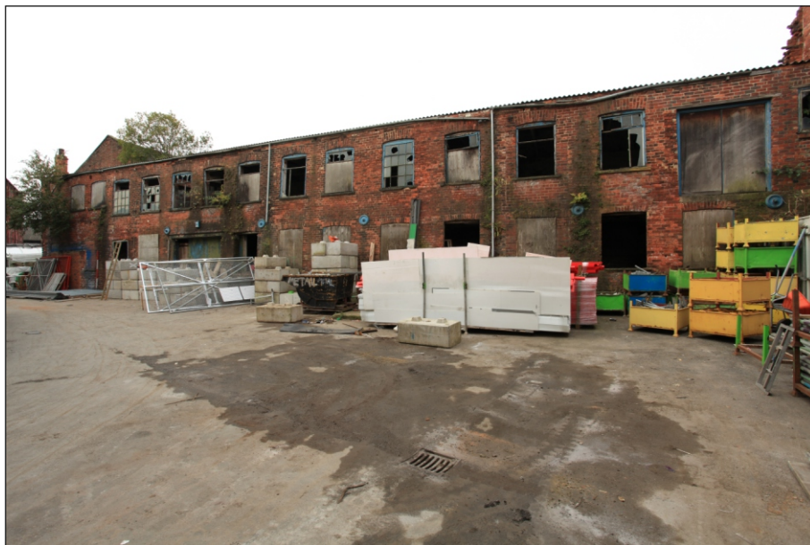
Plate 4: Oblique view of the east elevation of the east range (Film 3.03)
