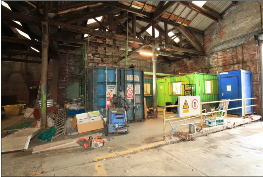
Plate 60: General view of G4, looking west (Film 6.09)
