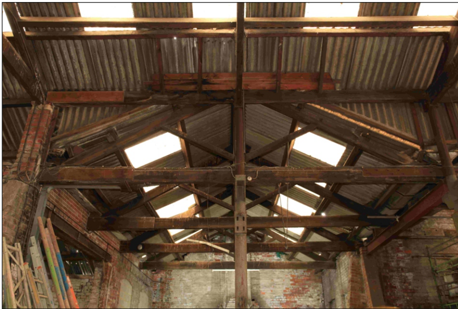
Plate 58: Detail of king post roof trusses in G5 (Film 1.20)
