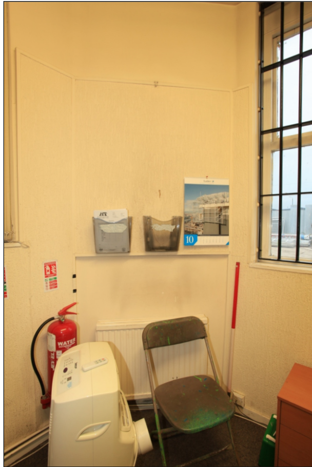
Plate 87: Detail of blocked corner fireplace in G7 (Film 1.08)
