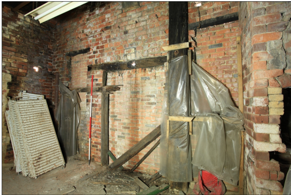
Plate 9: Oblique view of the east wall of G23 showing blockings (Film 1.31)
