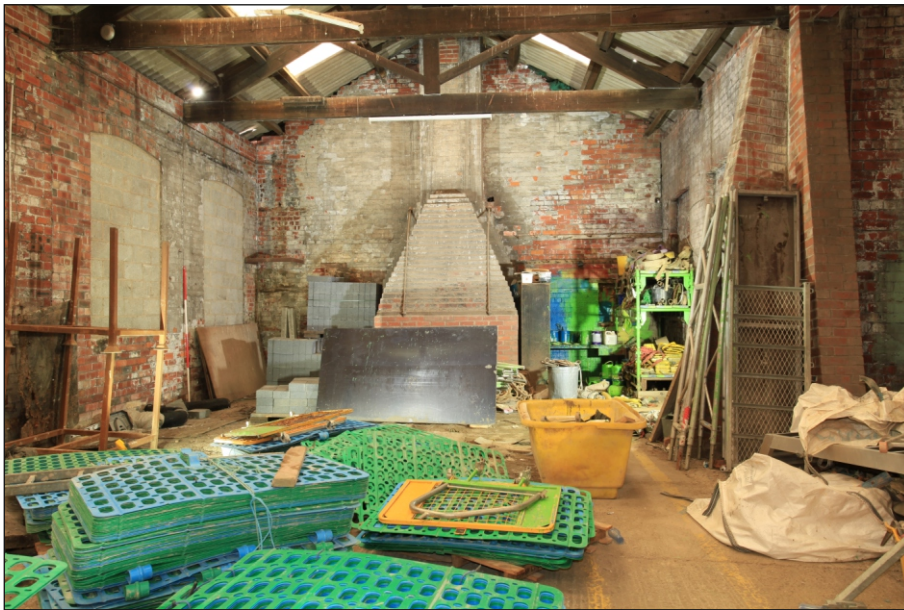
Plate 54: General view of G5, looking west (Film 5.9)
