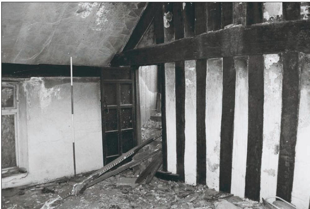
Plate 202: General view of F3, Building 2, showing close stud partition (Film 05.29)
