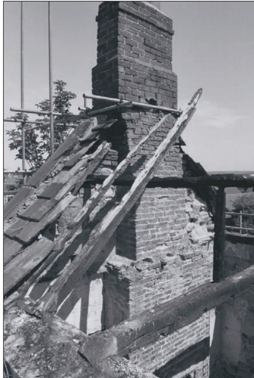
Plate 326: Detail of chimney stack, north end of Building 4 (Film 25.32)
