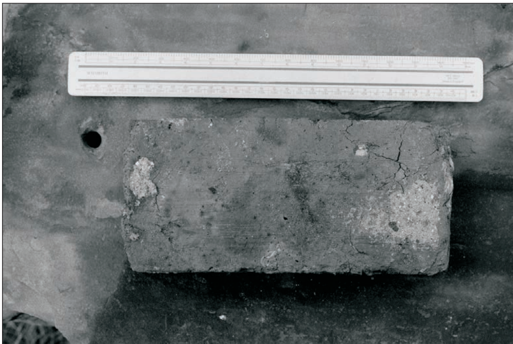
Plate 355: Detail of hand made brick from gable of Building 4 (Film 27.16)
