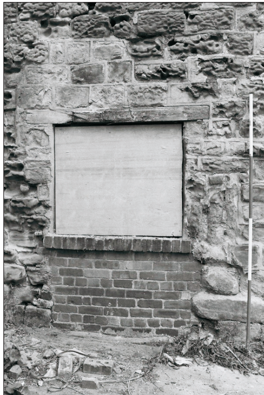
Plate 13: Detail of altered door to window, west elevation of barn, Building 1 (Film 02.11)
