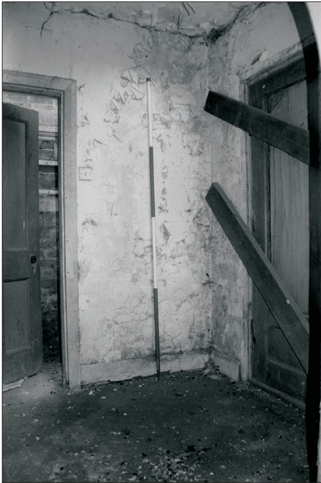
Plate 290: General view of room G5, Building 3 (Film 28.05)
