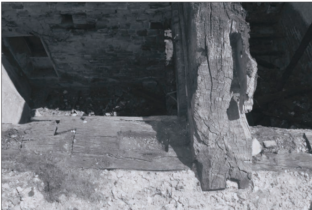
Plate 325: Detail of wall head, west wall of Building 4, showing scarf joint and tie beam (Film 25.30)
