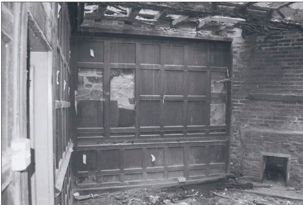
Plate 273: General view of room G3, Building 4 (Film 35.10)
