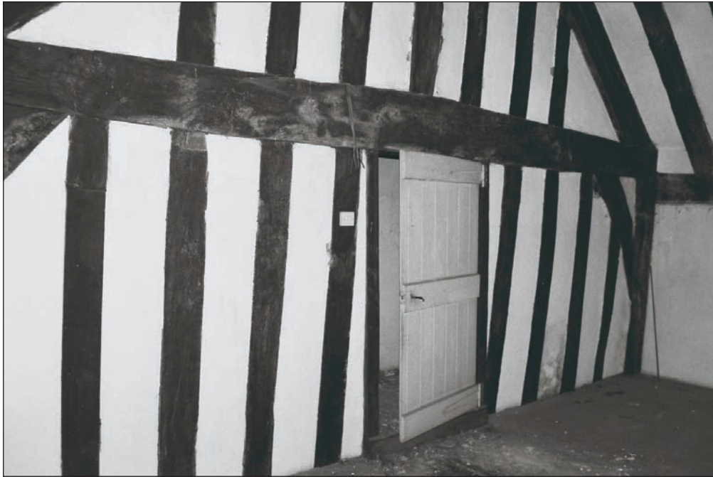
Plate 187: General view of F1, showing close stud partition, Building 2 (Film 06.02)
