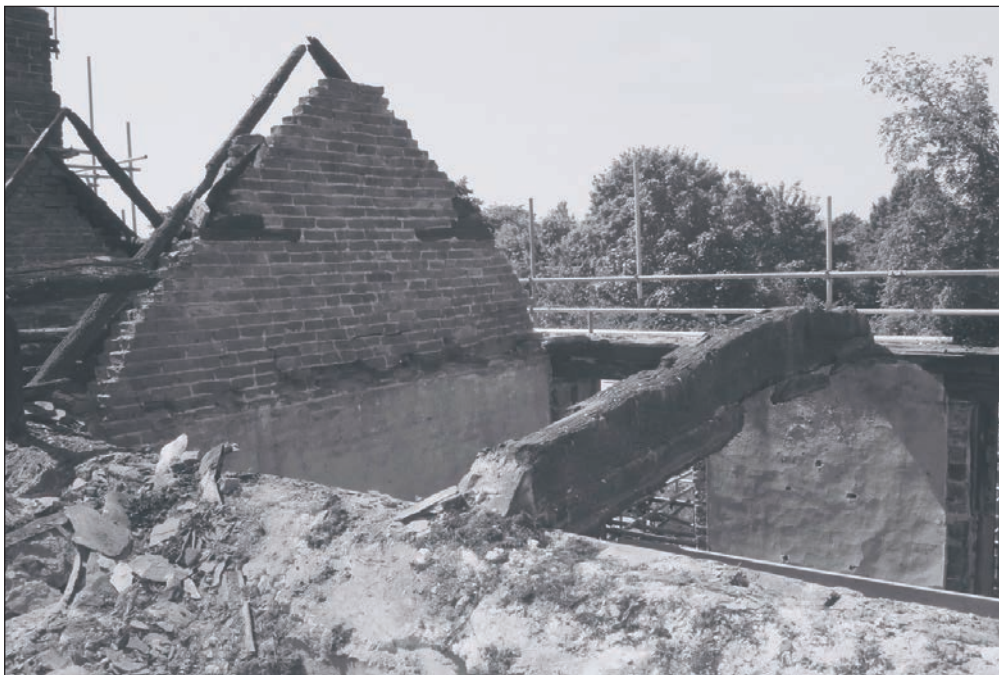
Plate 345: General view of central brick gable and tie beam, Building 4 (Film 26.34)
