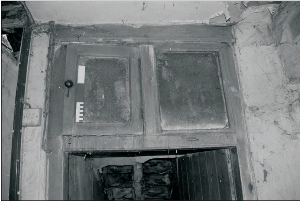
Plate 256c: Detail of upper gauze cupboards above doorway to cellar, G8, Building 3 (Film 28.19)
