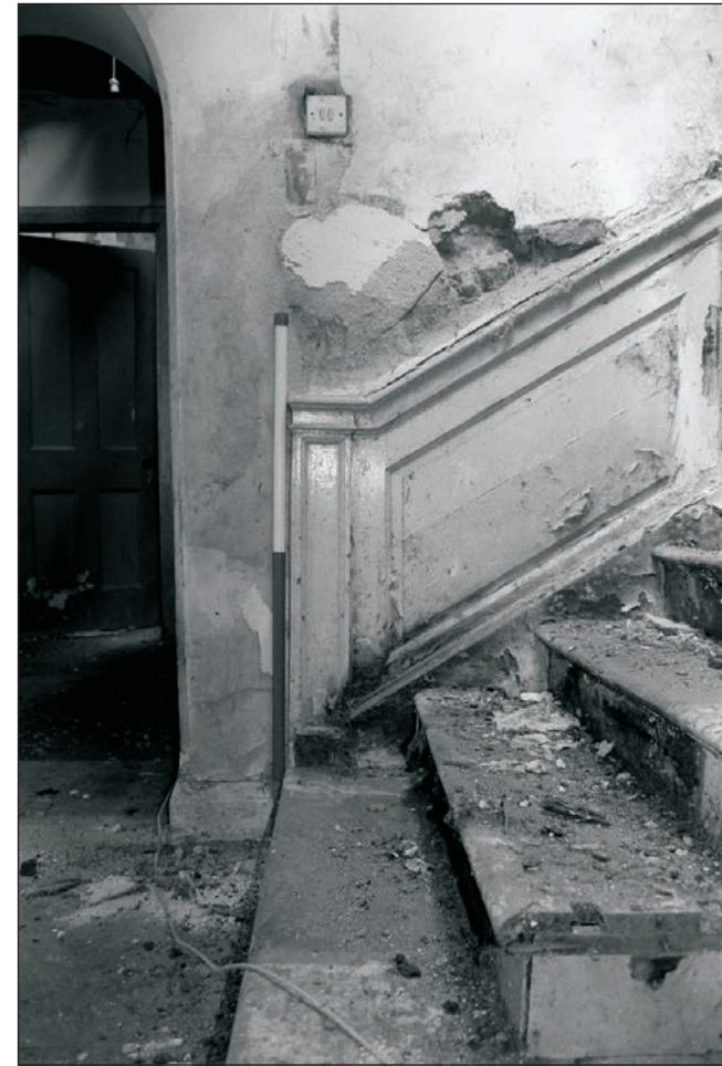
Plate 287: Detail of staircase, G6, Building 3 (Film 28.02)
