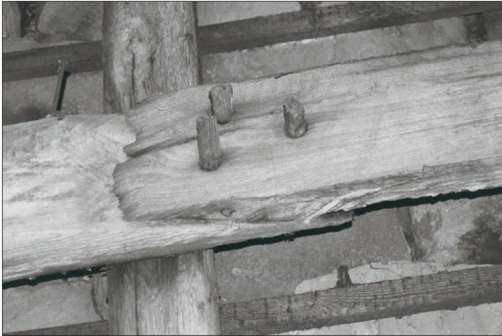
Plate 85: Detail of pegged purlins, F1 and F2, Building 1 (Film 03.08)
