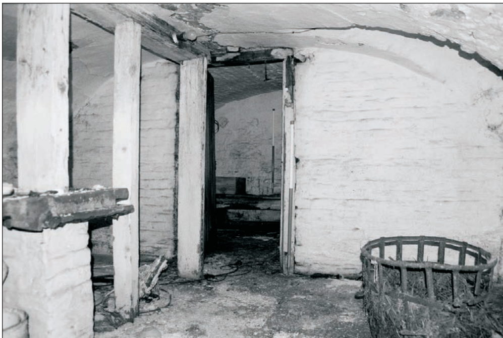
Plate 259: General view of room C2, Building 4 (Film 28.23)
