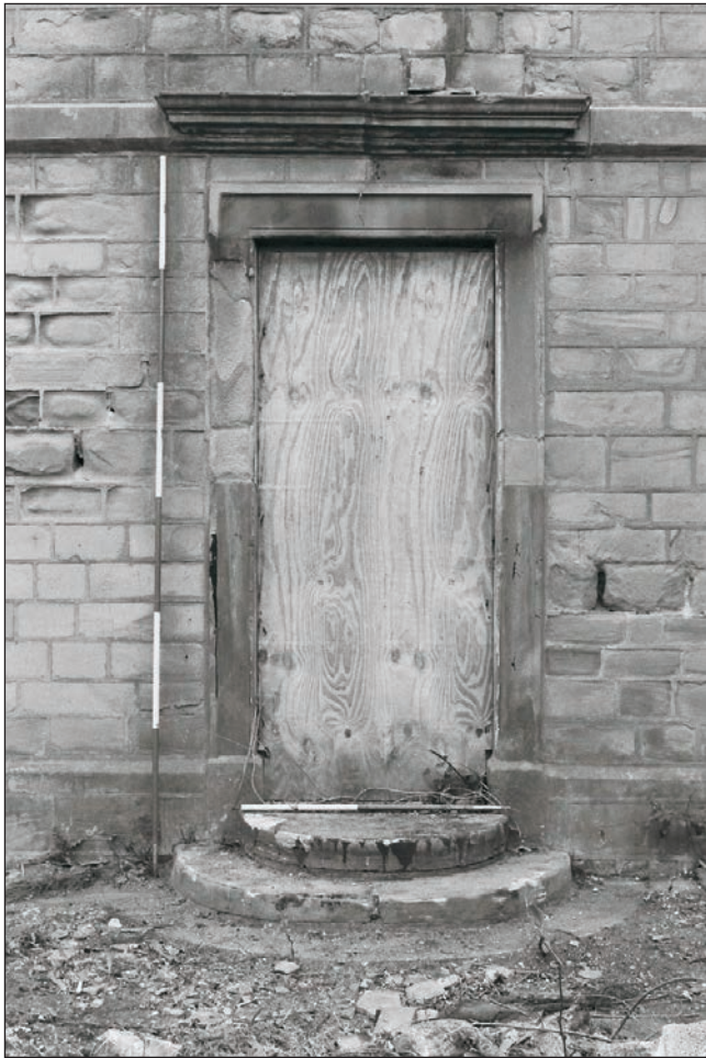
Plate 244: Detail of main entranceway, west elevation of Building 4 (Film 06.21)
