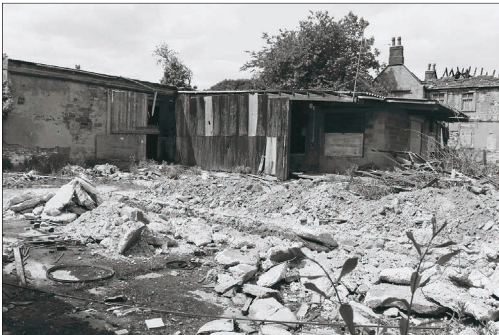
Plate 357: General view of Building 5 looking northwest (Film 02.29)
