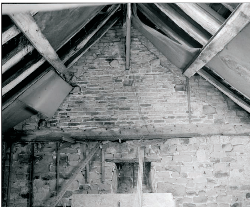
Plate 52: View of raised roof, south gable of F1, Building 1 (Film 20.02)
