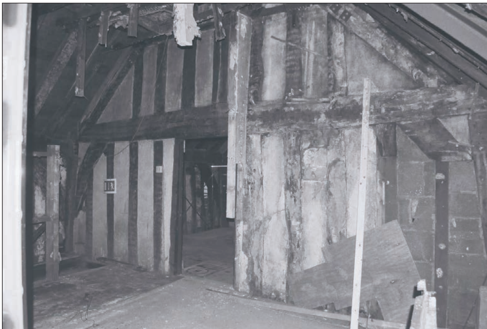
Plate 179: General view of landing F2 and room F3 after the removal of modern partitions, showing primary central close stud partition, Building 2 (Film 43.01)
