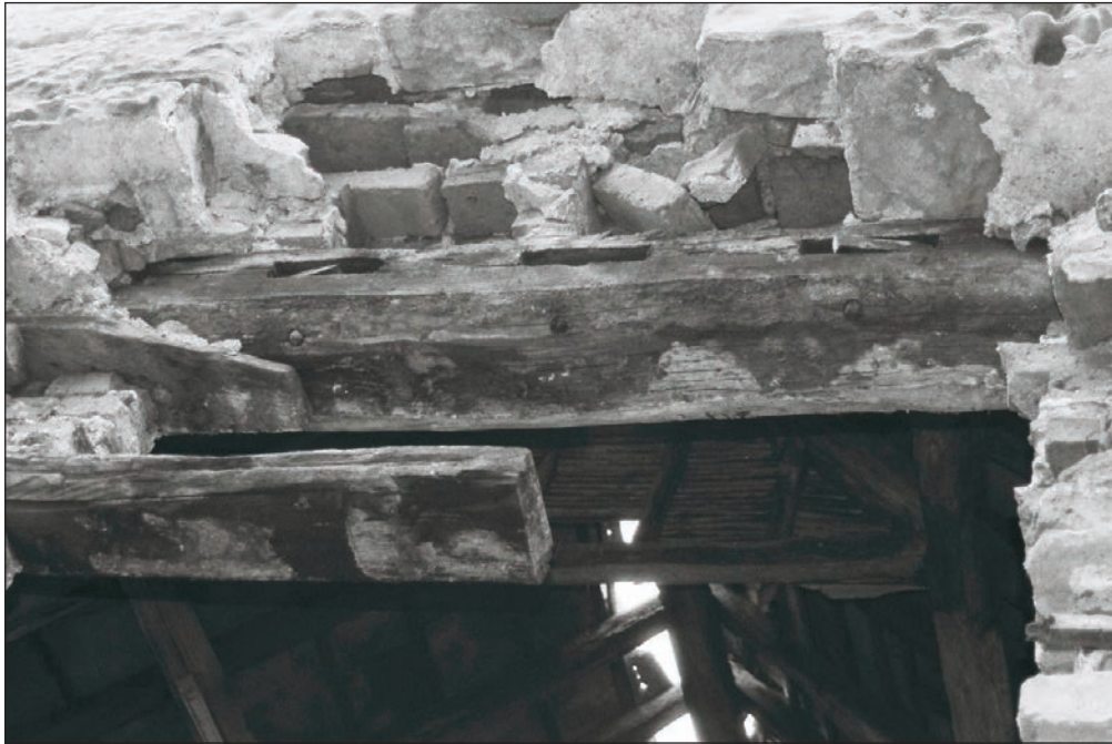
Plate 81: Detail of reused (and rotated) tie beam within the north gable of the dovecote, F2, Building 1 (Film 03.29)
