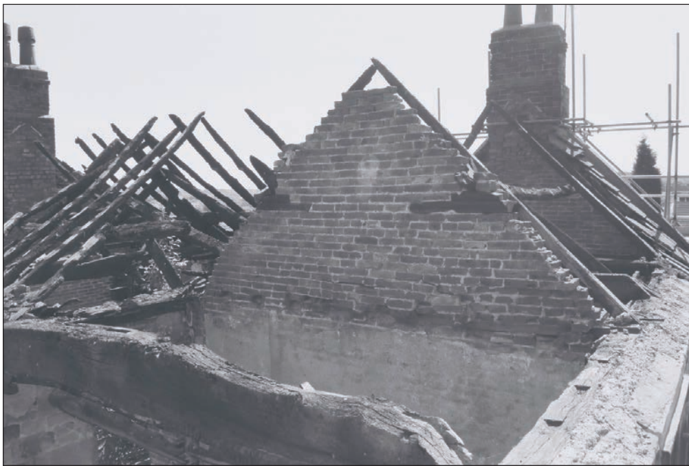
Plate 323: General view of brick gable, Building 4 (Film 25.27)
