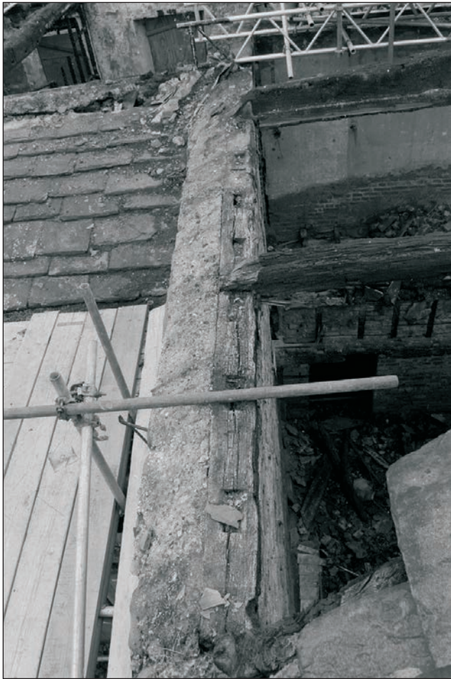
Plate 346: General view of wall head, east wall of building 4 (Film 27.17)
