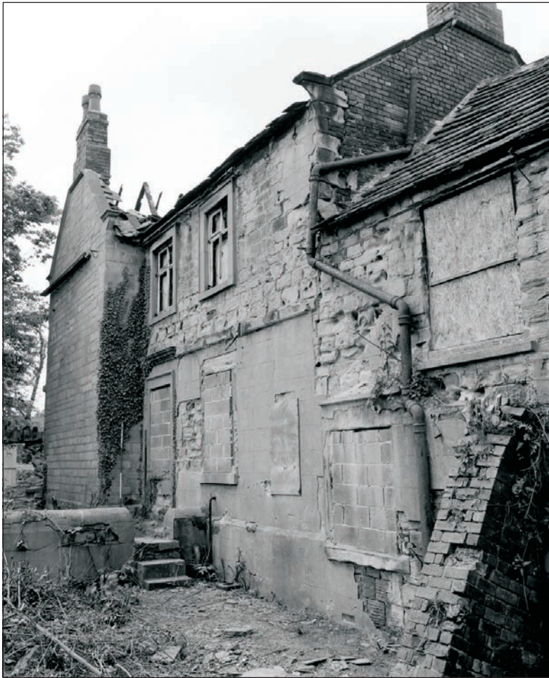
Plate 234: General view of the south elevation of Building 3 and 4 (Film 10.10)
