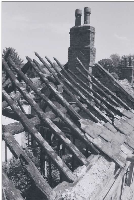
Plate 315: General view of roof timbers, Building 3 (Film 25.11)
