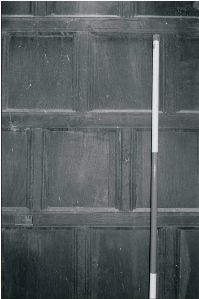
Plate 280: Detail of the Type 3 oak panelling on the east wall of room G3, Building 4 (Film 29.15)
