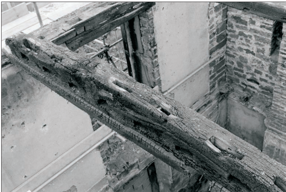
Plate 349: Detail of redundant mortices within tie beam, Building 4 (Film 27.24)
