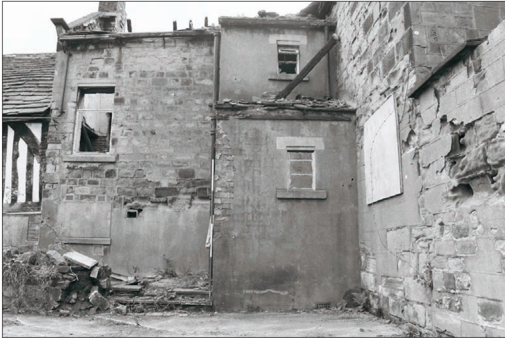
Plate 248: General view of the north elevation of Building 3 (Film 01.02)
