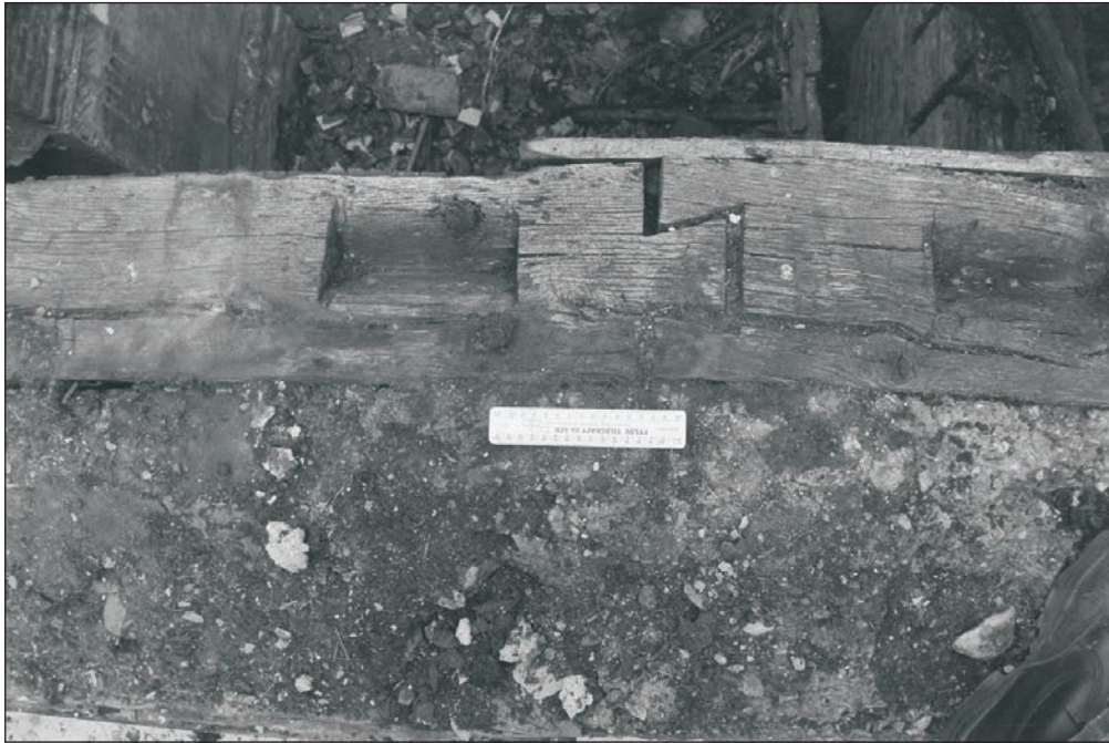
Plate 354: Detail of scarf joint, west wall plate, Building 4 (Film 27.33)
