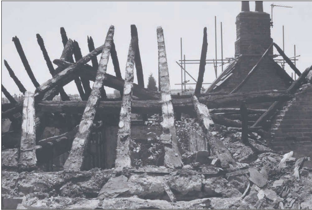
Plate 340: General view of roof timbers, Building 3 (Film 26.24)
