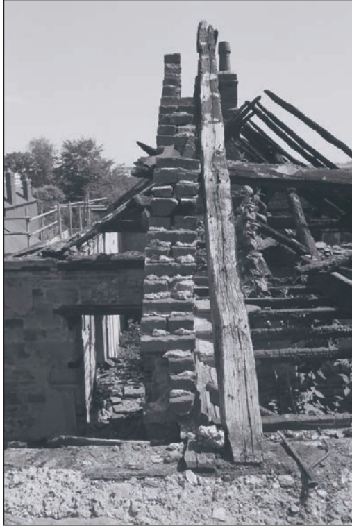
Plate 322: Detail along gable and truss from west wall of Building 4 (Film 25.24)
