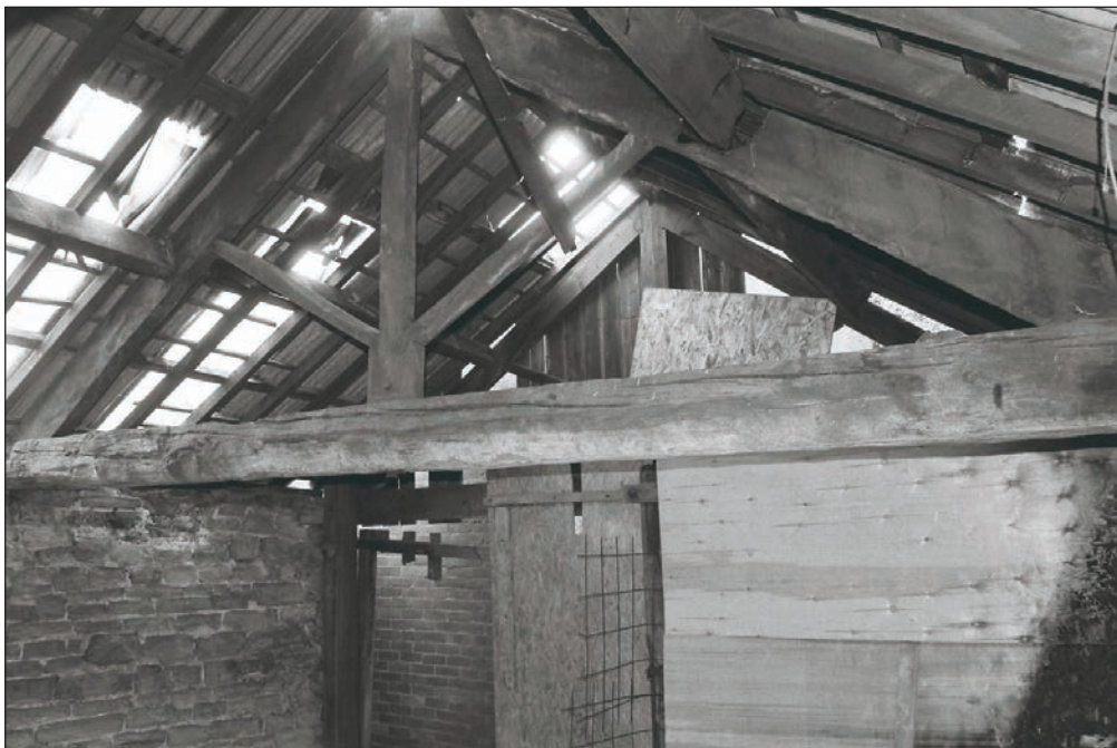
Plate 365: Detail of timber King-Post roof trusses within Building 5 (Film 06.32)
