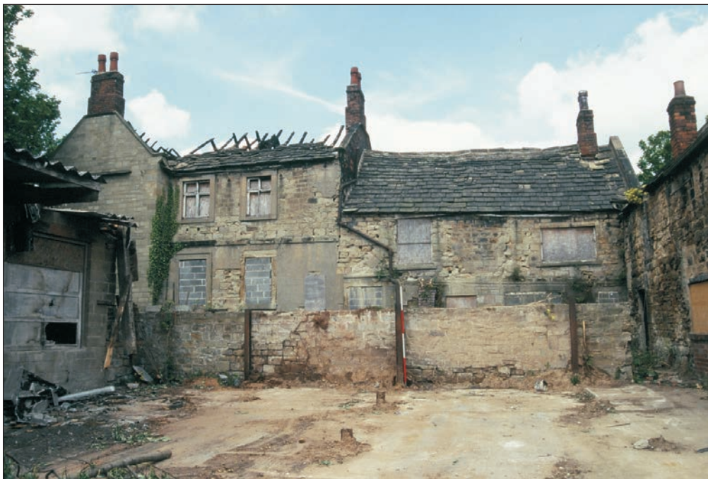
Plate 2: General view of the south elevation of Hanson House (Buildings 2-4) (Colour Slide 06)
