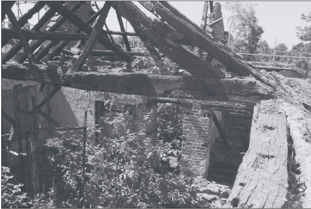
Plate 336: General view of roof timbers, Building 3 (Film 26.17)
