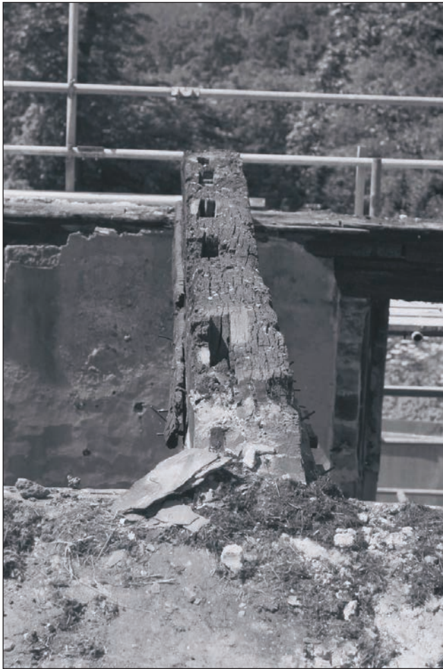
Plate 330: Detail of re-used tie beam, Building 4 (Film 26.04)
