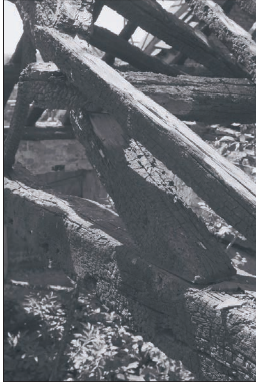
Plate 334: Detail of truss, Building 3 (Film 26.12)
