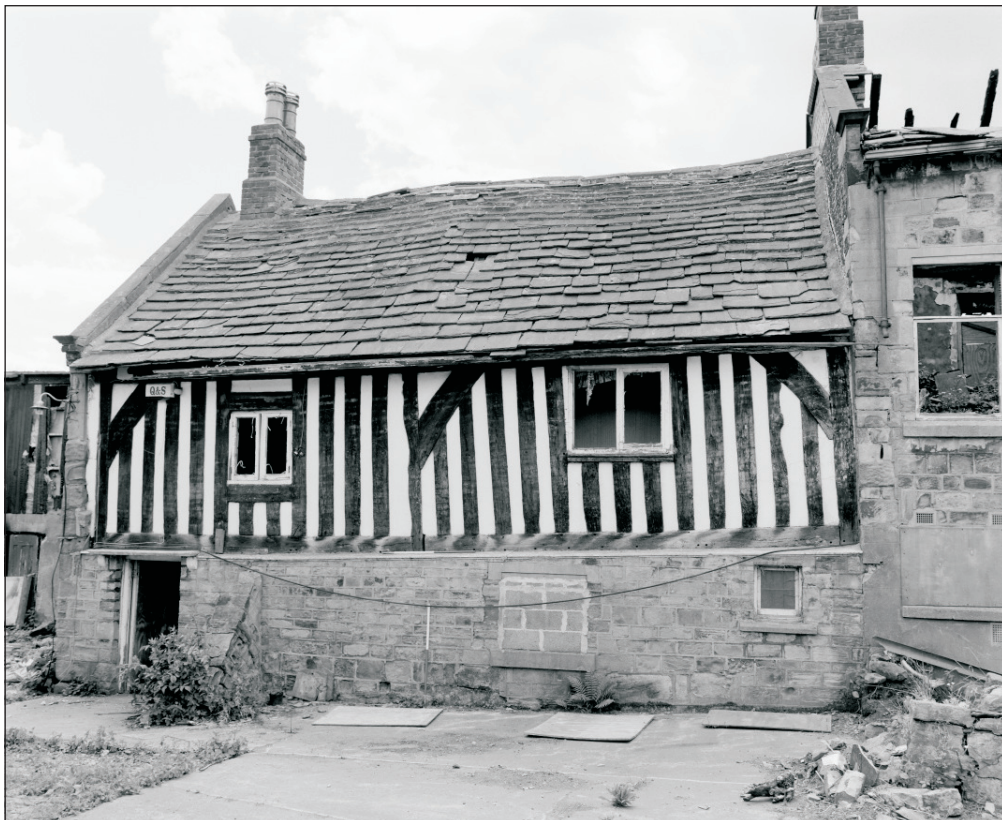
Plate 107: General view of the north elevation of Building 2 (Film 13.02)
