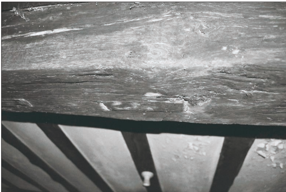
Plate 139: Detail of mortice holes on underside of beam, G1, Building 2 (Film 04.16)
