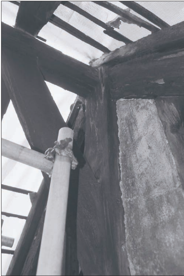
Plate 215: Detail of King-Post and ridge brace, F1, Building 2 (Film 41.03)
