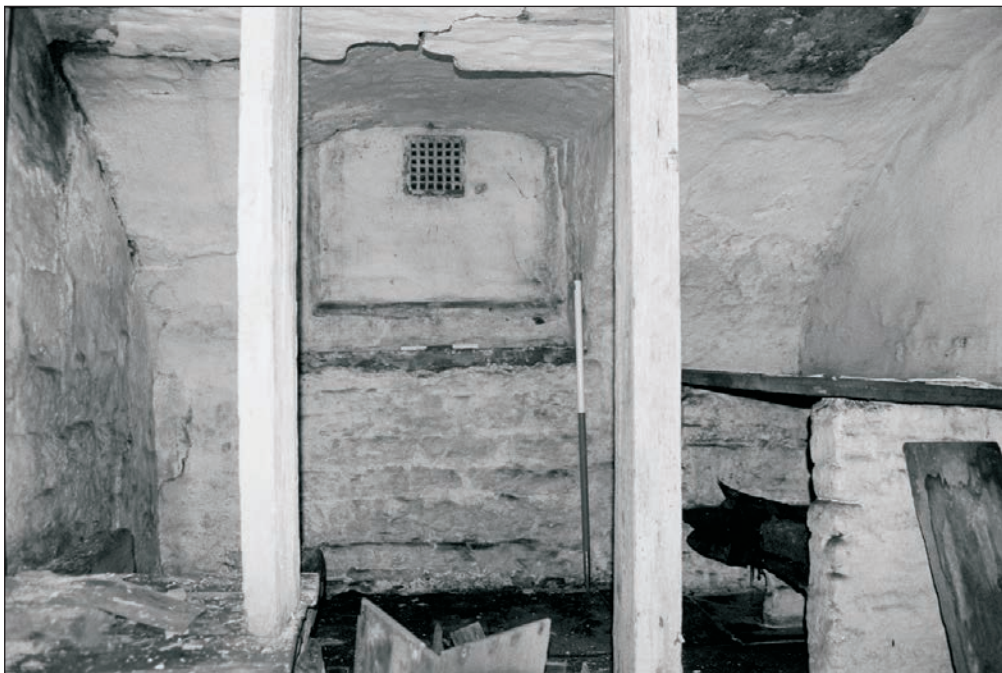
Plate 263: General view of room C1, Building 4 (Film 28.25)
