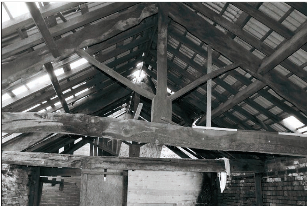
Plate 363: Detail of timber King-Post roof trusses within Building 5 (Film 02.24)
