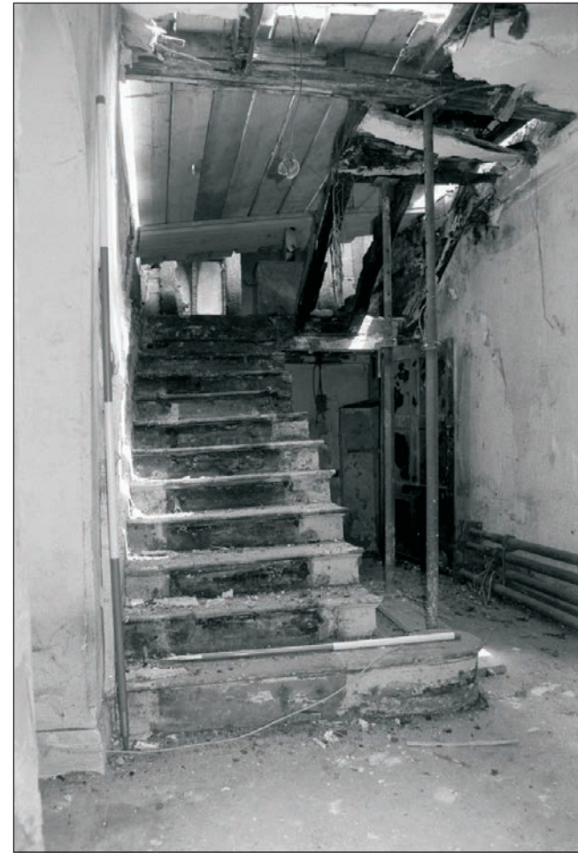
Plate 285: General view of staircase and hallway G6, Building 3 (Film 28.11)
