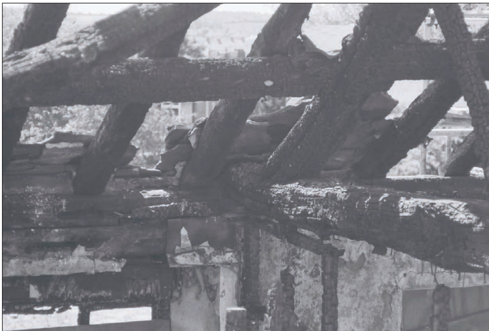
Plate 335: Detail of truss, Building 3 (Film 26.15)
