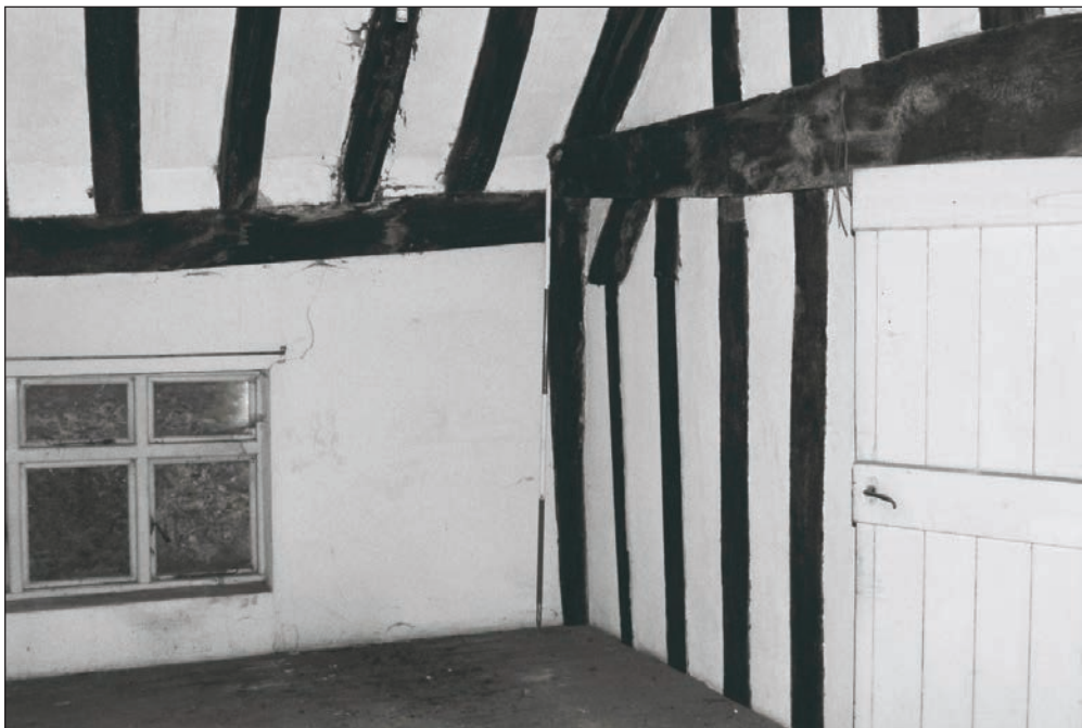
Plate 184: General view of F1, showing close stud partition, Building 2 (Film 05.30)
