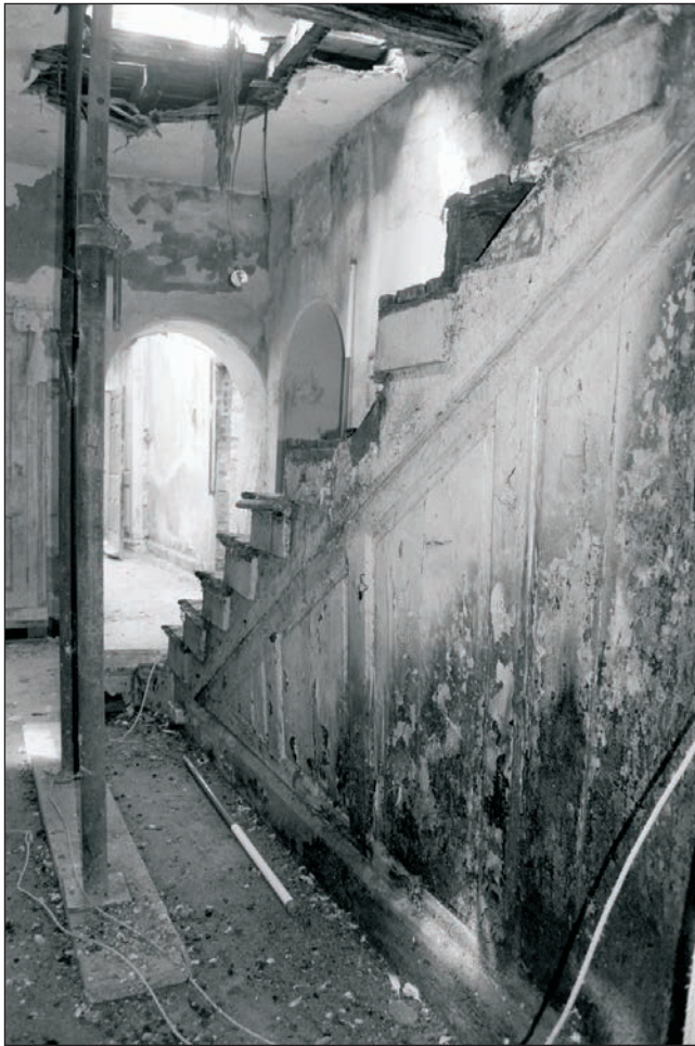
Plate 288: General view of staircase and hallway G6, Building 3 (Film 28.13)
