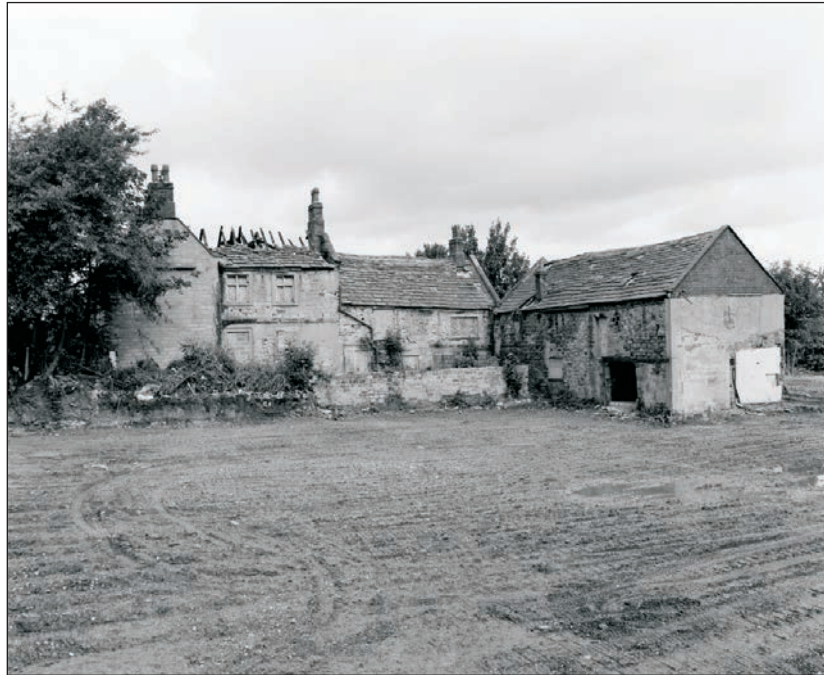
Plate 5: General view of Hanson House and barn (Buildings 1-4) after the demolition of Buildings 5 and 6 (Film 22.01)
