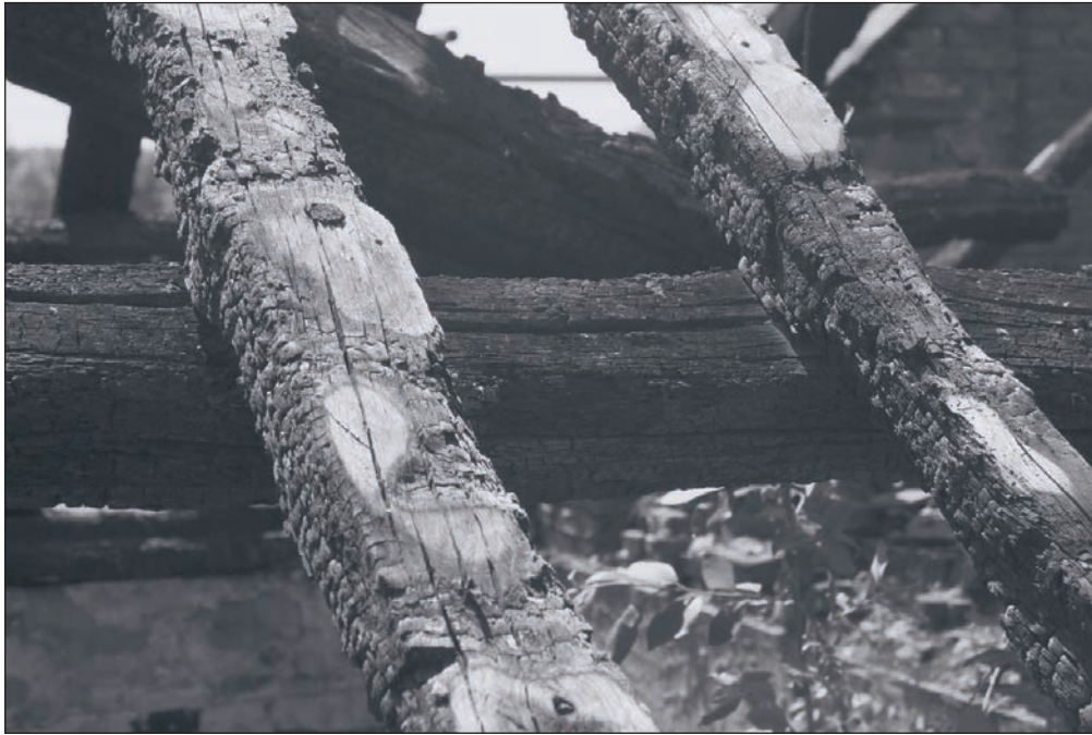
Plate 332: Detail of rafters and pegged purlin, Building 3 (Film 26.08)
