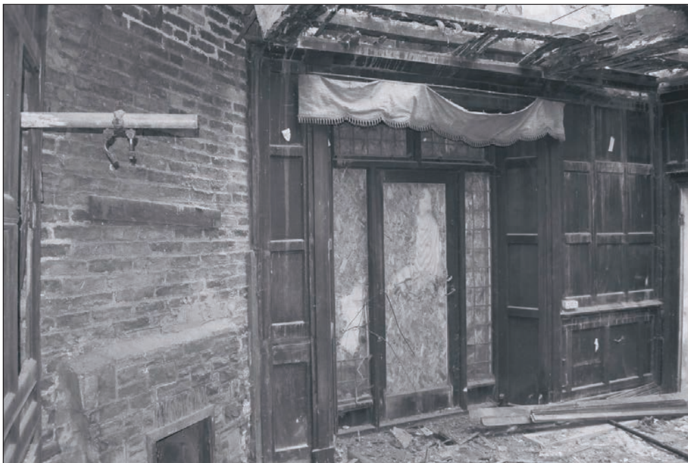
Plate 275: General view of room G3, Building 4 (Film 35.15)
