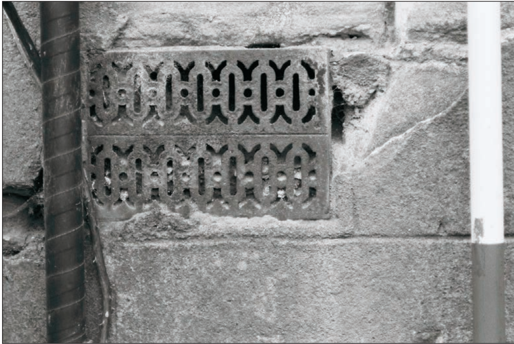
Plate 238: Detail of cast iron vent, south elevation of Building 3 (Film 05.02)
