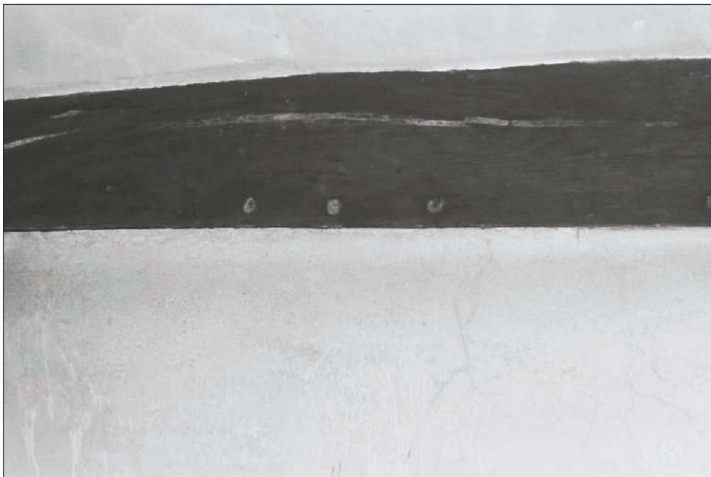
Plate 212: Detail of empty pegs from removed timber framing, wall plate to south wall of F3, Building 2 (Film 05.12)
