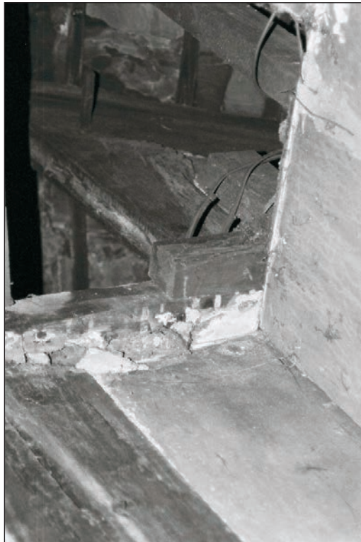
Plate 182: Detail of close studding partition above ceiling within F2, Building 2 (Film 04.01)
