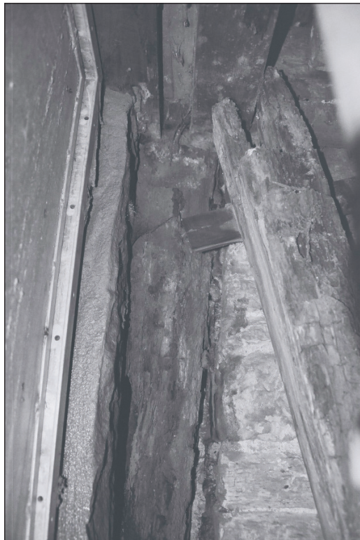
Plate 171: Detail of exposed south-west original timber post, G4, Building 2 (Film 42.12)
