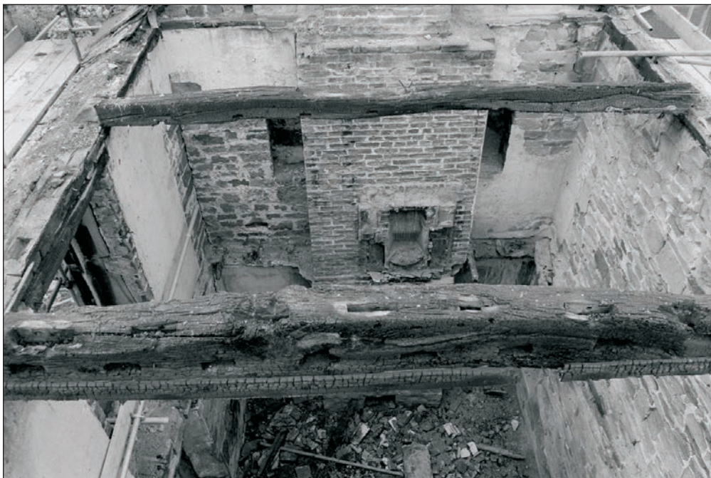
Plate 351: View into former room F1, showing brick chimney breast, flanking windows and tie beams, Building 4 (Film 27.25)
