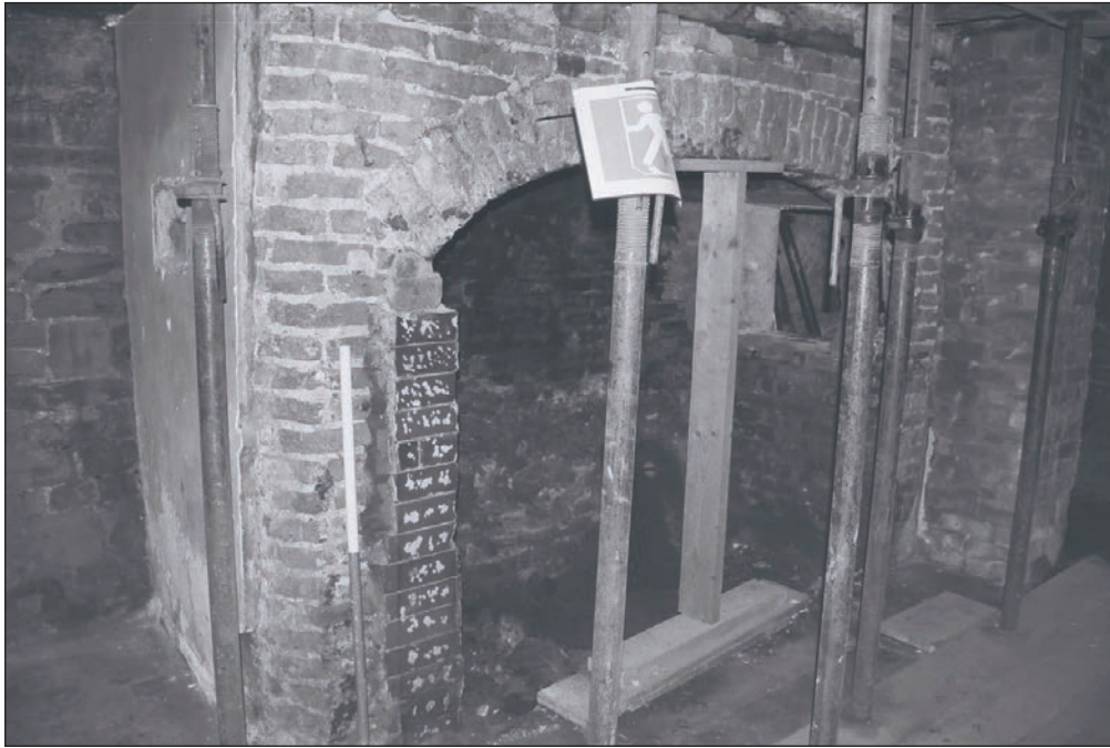
Plate 132: Detail of exposed fireplace and chimney breast during watching brief, G1, Building 2 (Film 42.30)
