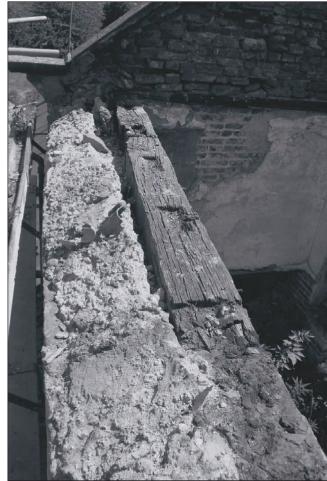
Plate 331: Detail of wall plate, west wall, Building 4 (Film 26.06)
