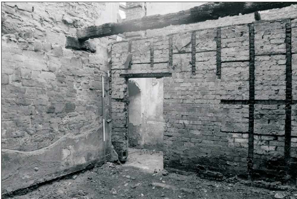
Plate 267: General view of room G1, Building 4 (Film 29.05)
