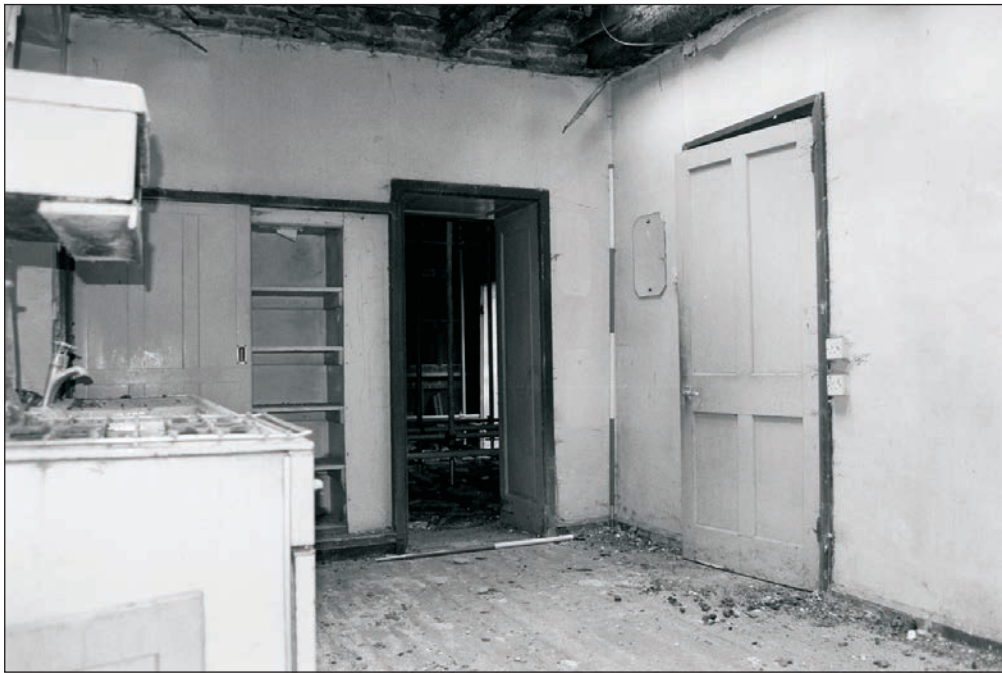
Plate 292: General view of room G7, Building 3 (Film 29.26)
