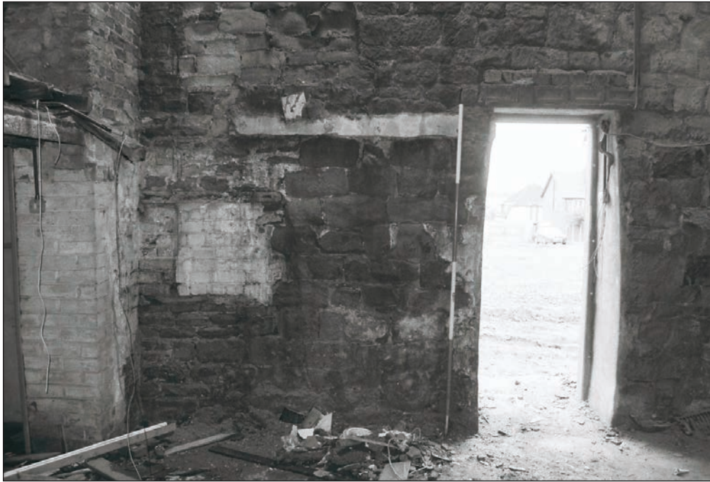
Plate 39: Internal view of the inserted door and blocked window, east wall of G1, Building 1 (Film 24.10)
