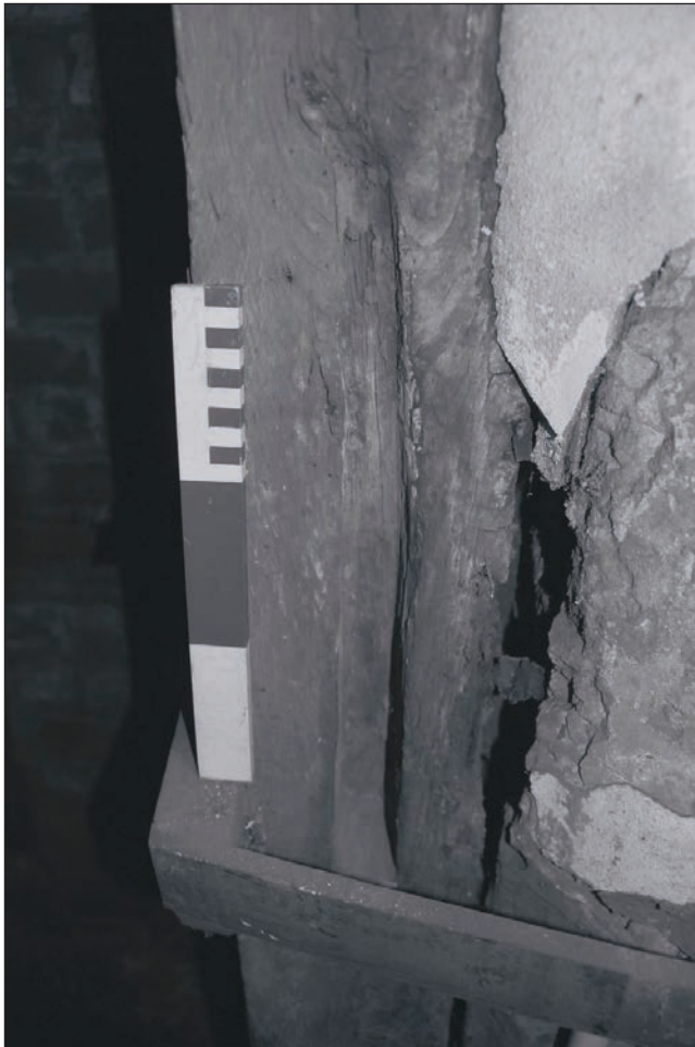
Plate 158: Detail of groove within the exposed south post, G4, Building 2 (Film 30.13)
