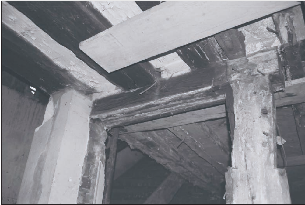
Plate 166: Detail of doorway between G3 and G1 showing primary timber framing with empty mortices, truncated cross beam, and inserted brick pier, Building 2 (Film 42.04)
