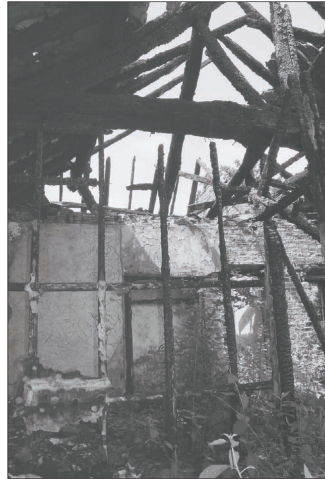
Plate 307: View of rooms F5 and F6, Building 3, from F3, Building 2 (Film 12.24)
