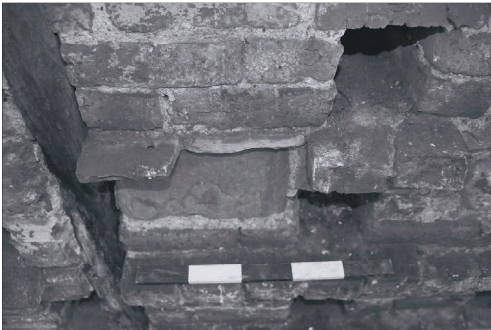
Plate 80: Detail of reused roof tile within dovecote, F2, Building 1, during watching brief (Film 39.33)
