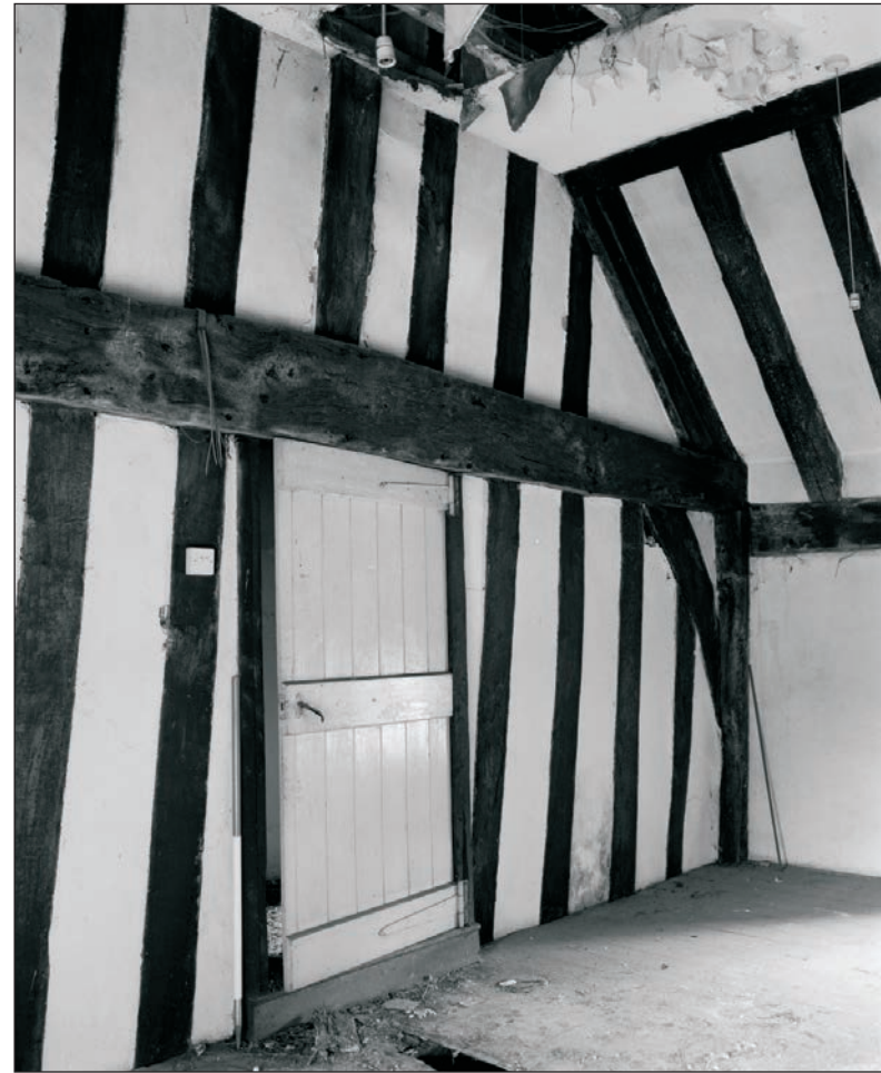
Plate 186: General view of F1, showing close stud partition, Building 2 (Film 16.07)
