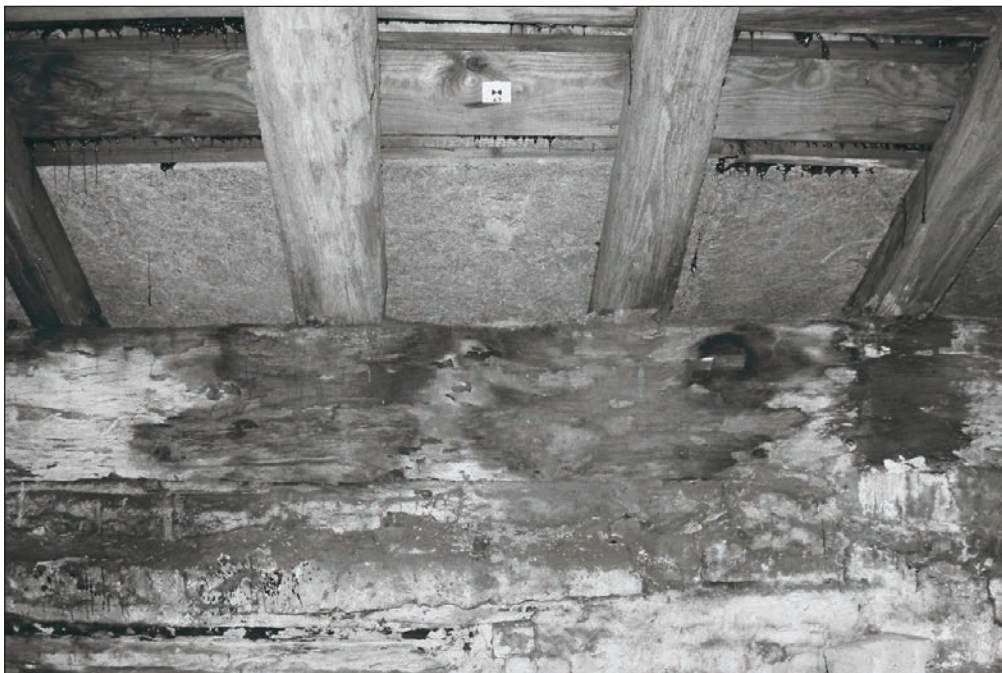
Plate 84: Detail of common rafters and wall plate, F2, Building 1 (Film 06.10)
