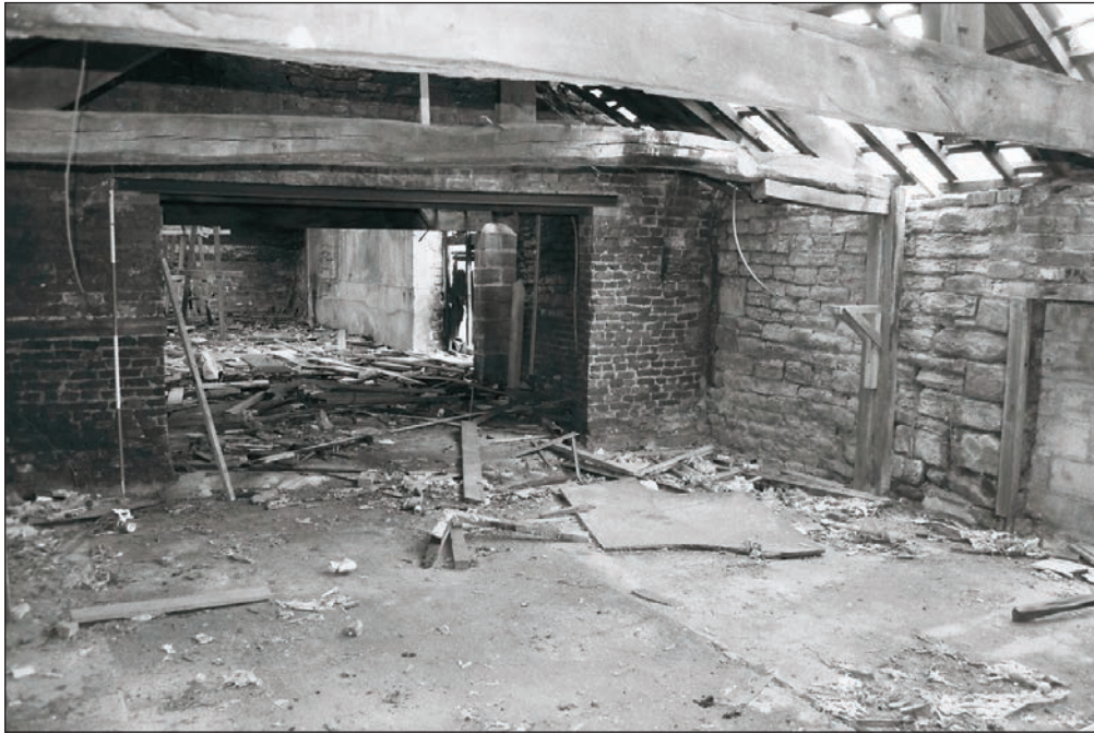
Plate 362: General internal view of Building 5 (Film 06.29)
