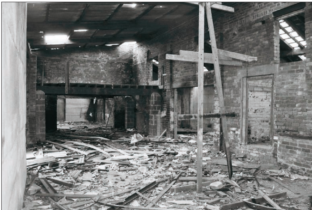
Plate 361: General internal view of Building 5 (Film 06.35)
