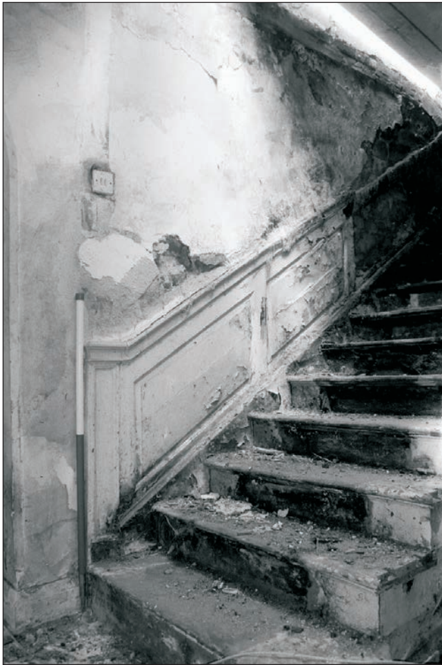
Plate 286: Detail of staircase, G6, Building 3 (Film 28.01)
