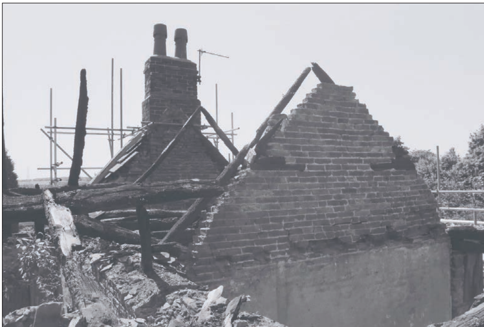
Plate 343: General view of central brick gable, Building 4 (Film 26.31)
