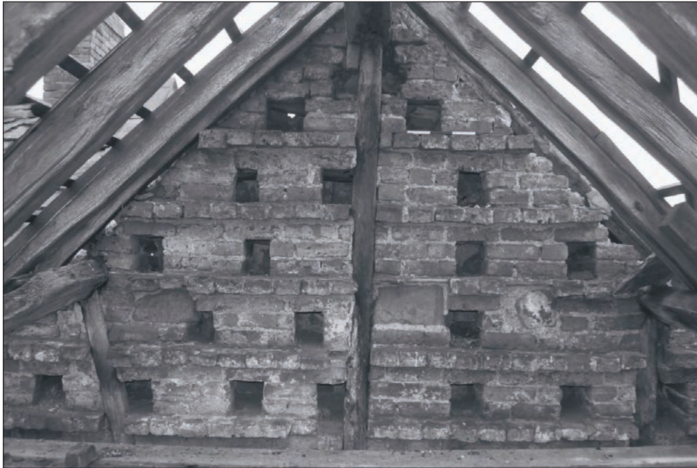
Plate 79: Detail of the upper dovecote north gable, F2, Building 1, during the watching brief (Film 39.35)
