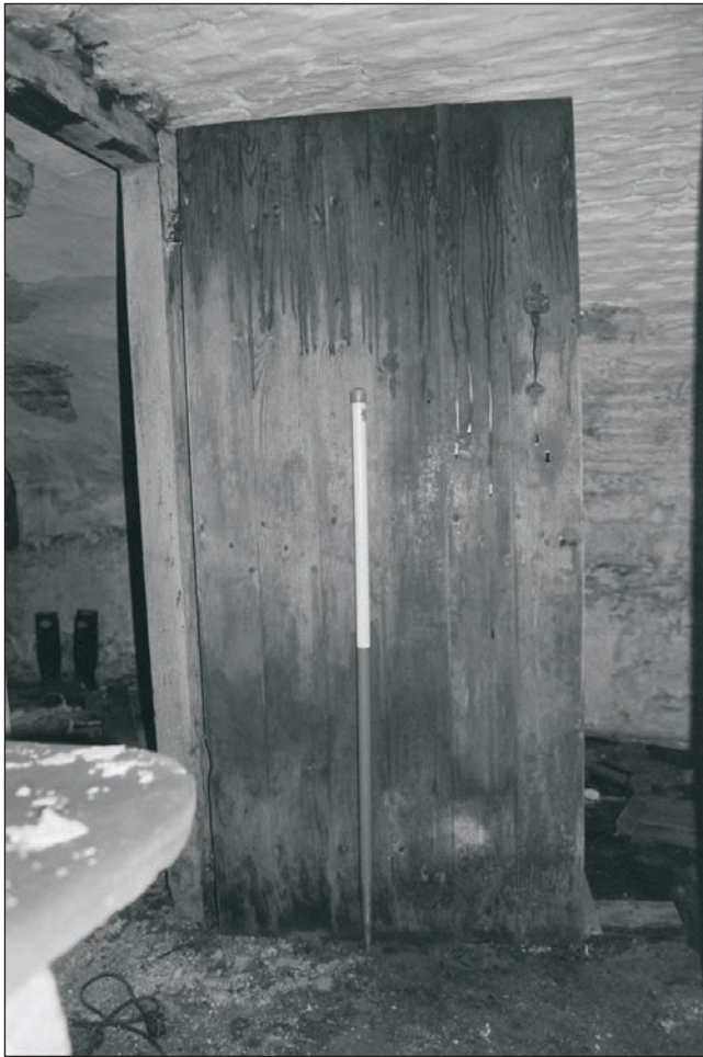
Plate 264: Detail of timber doorway between room C1 and C2, Building 4 (Film 28.26)
