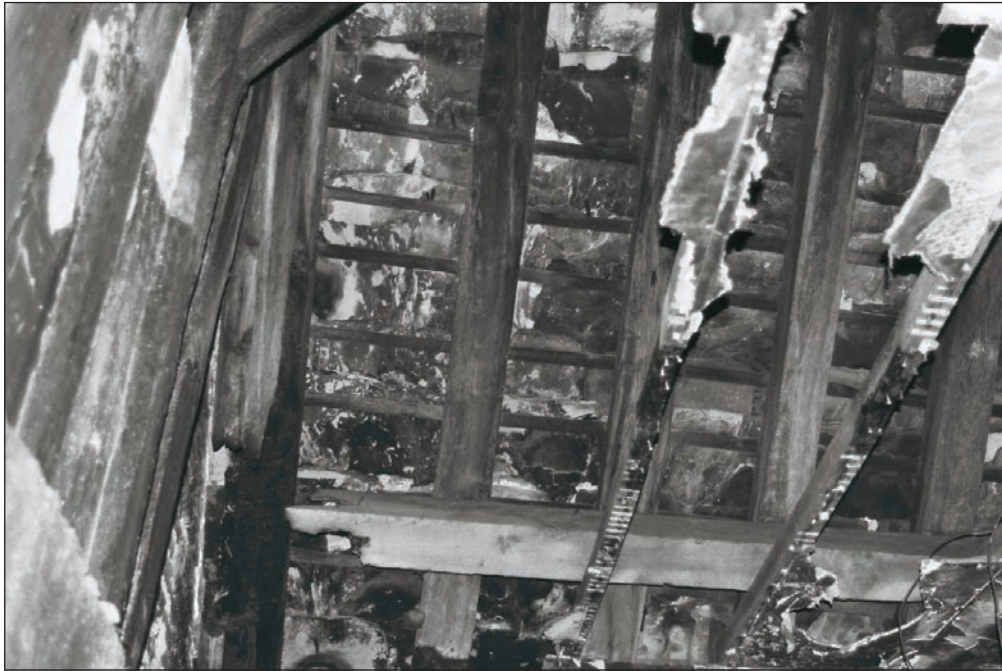
Plate 211: Detail of former ceiling and roof structure above, F3, Building 2 (Film 05.22)
