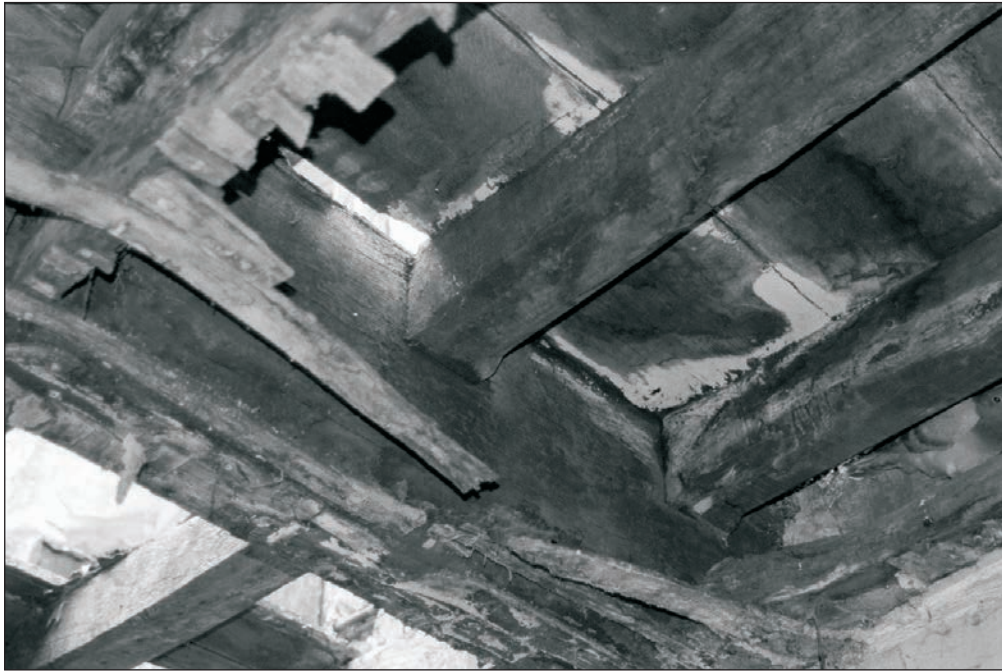
Plate 298: Detail of ceiling beam and joists, room G7, Building 3 (Film 29.25)
