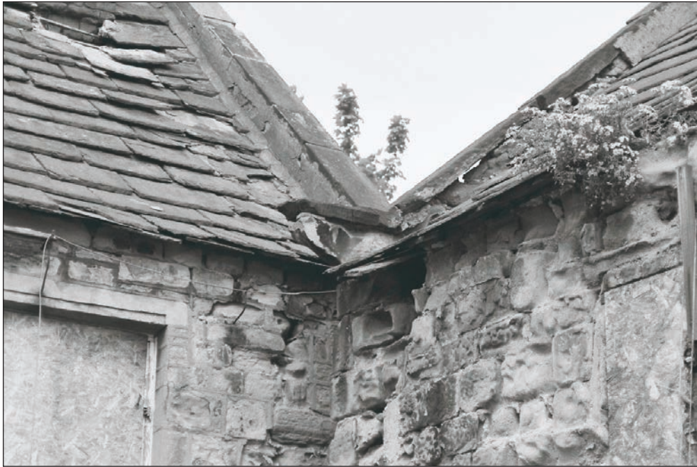
Plate 18: Detail of stone kneeler, north end of the west elevation of the barn, Building 1 (Film 02.10)
