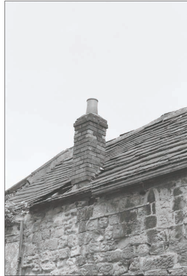
Plate 17: Detail of brick chimney, west elevation of the barn, Building 1 (Film 02.14)
