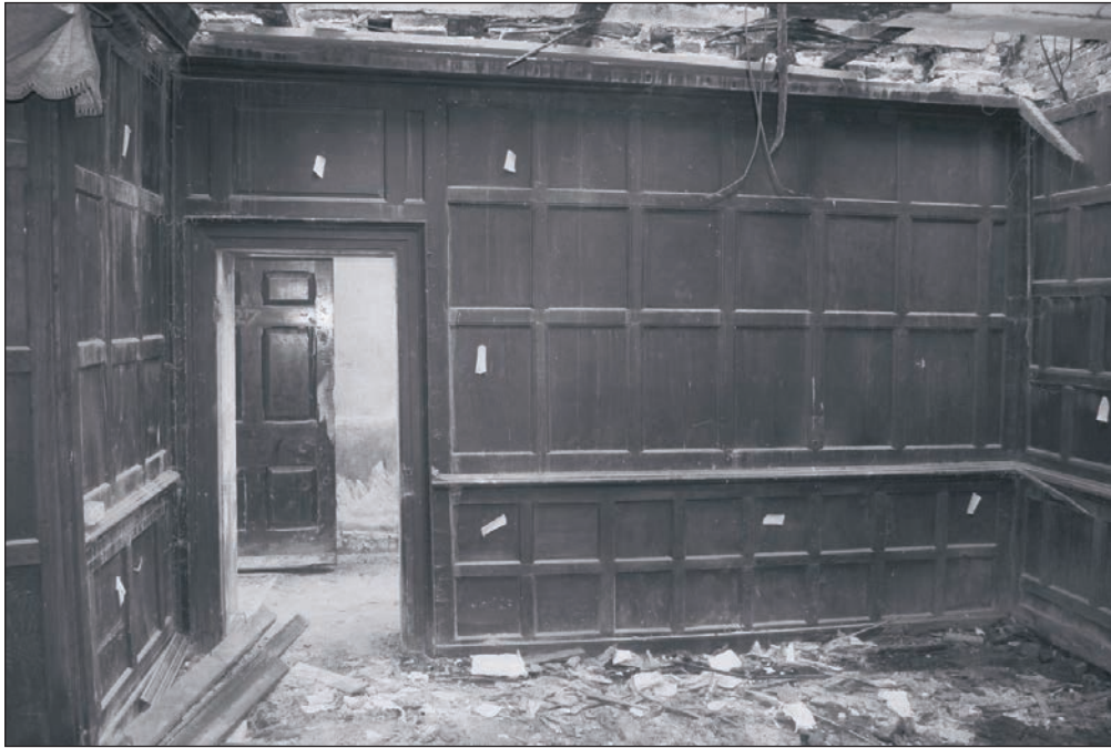
Plate 276: General view of room G3, Building 4 (Film 35.17)
