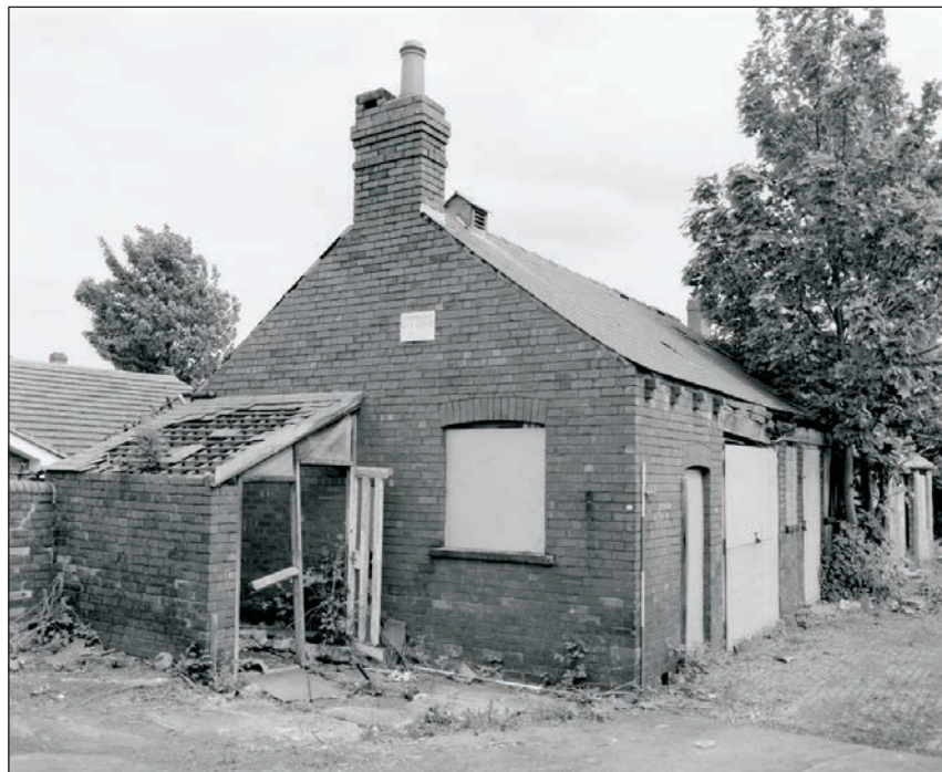
Plate 369: General view of the west and south elevations of Building 7 (Film 08.04)
