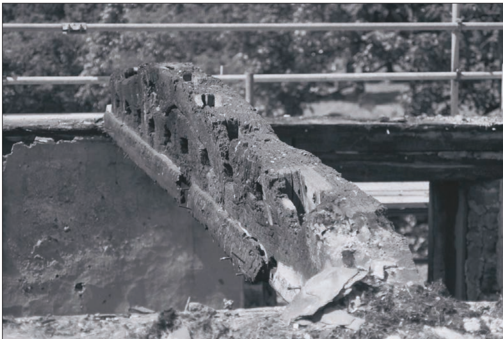
Plate 329: Detail of re-used tie beam, Building 4 (Film 26.02)
