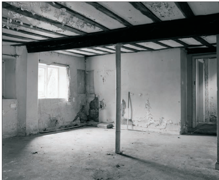
Plate 121: General view of G1, Building 2 (Film 14.02)
