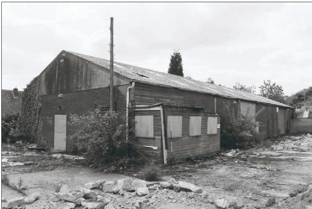
Plate 367: General view of Building 6, looking southwest (Film 02.32)
