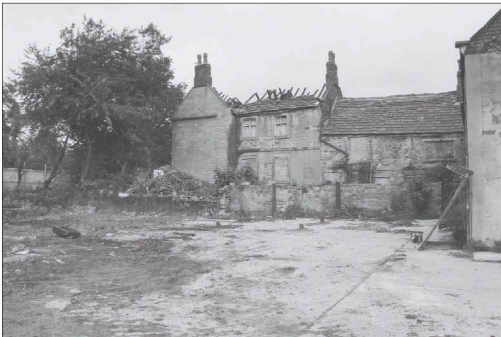
Plate 4: General view of Hanson House (Buildings 2-4) after the demolition of Buildings 5 and 6 (Film 18.23)
