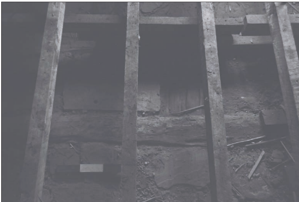
Plate 230: Detail of reused roof tiles on limeash floor beneath removed timber floor, F1, Building 2 (Film 40.07)
