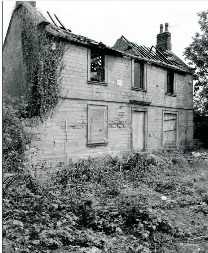
Plate 241: General view of the west elevation of Building 4 (Film 11.05)
