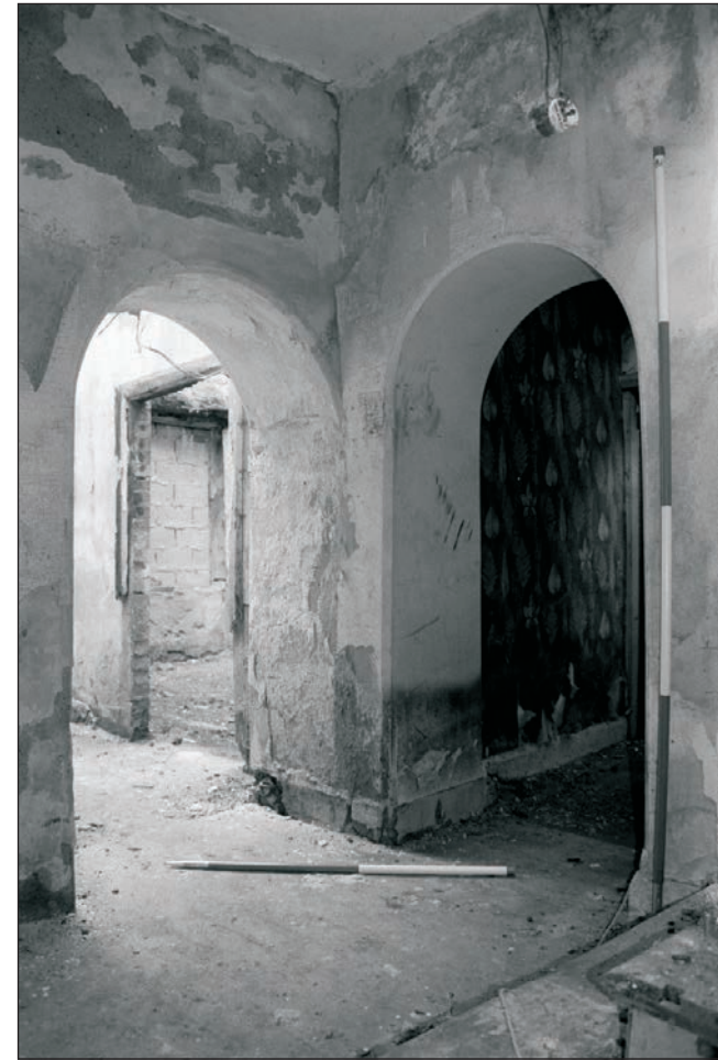
Plate 289: General view of hallway G6, Building 3, showing arched doorways to G2 and G5 (Film 28.09)
