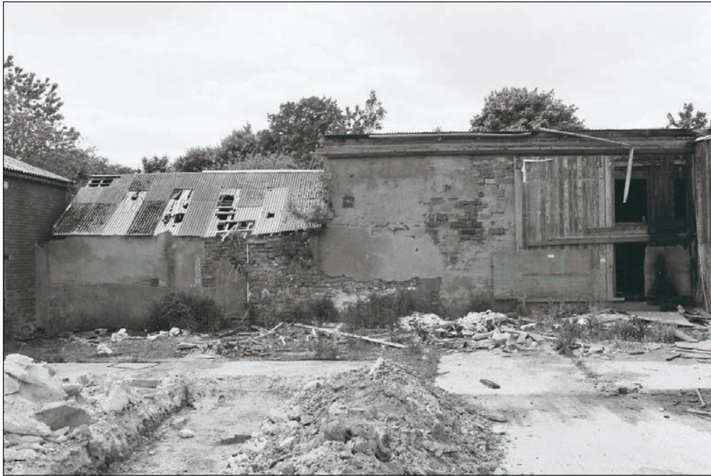
Plate 356: General view of the east elevation of Building 5 (Film 02.27)
