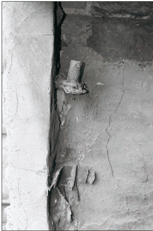
Plate 46: Detail of bolt hinges, doorway reveal of G3, Building 1 (Film 03.31)
