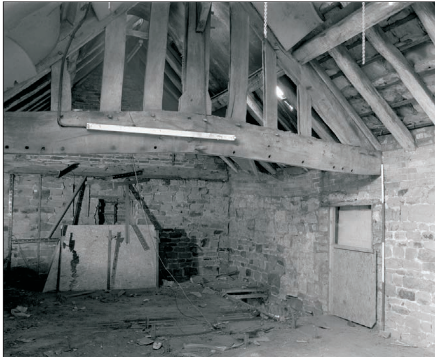
Plate 48: General view of F1, Building 1 (Film 19.04)
