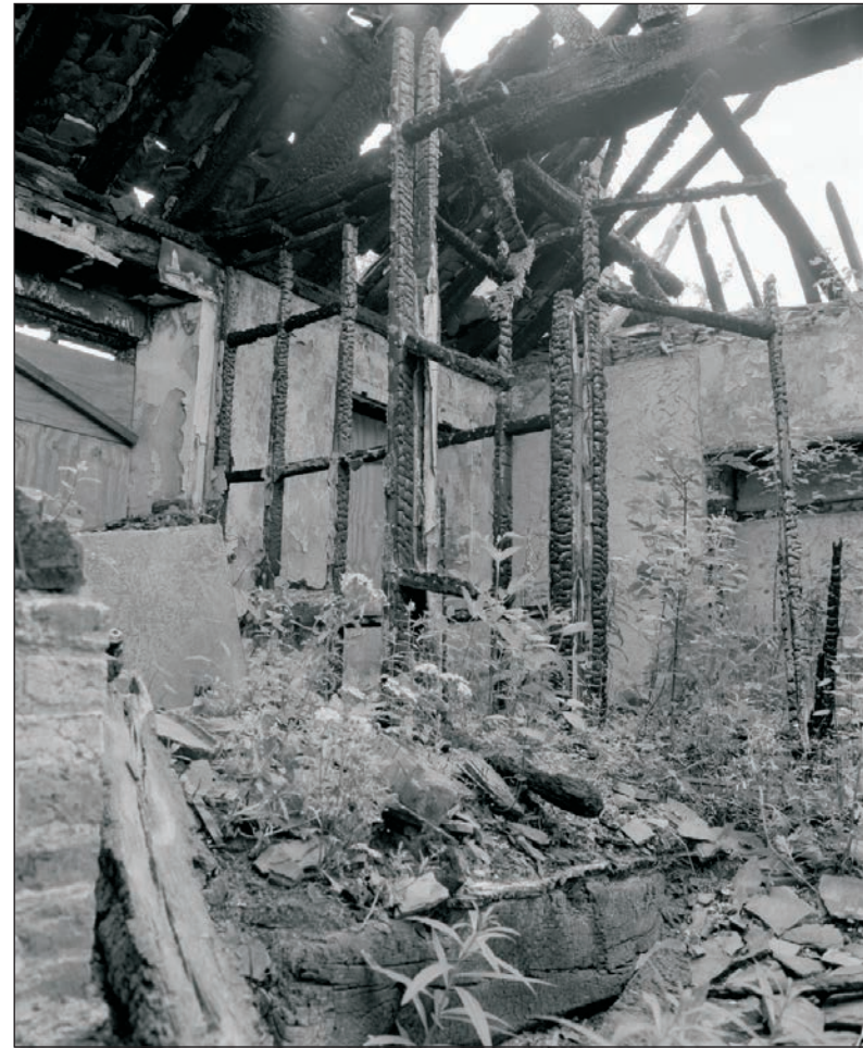
Plate 305: View of rooms F5 and F6, Building 3, from F3, Building 2 (Film 16.01)
