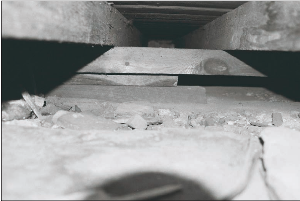
Plate 223: View beneath floorboards, F1, Building 2 (Film 06.01)
