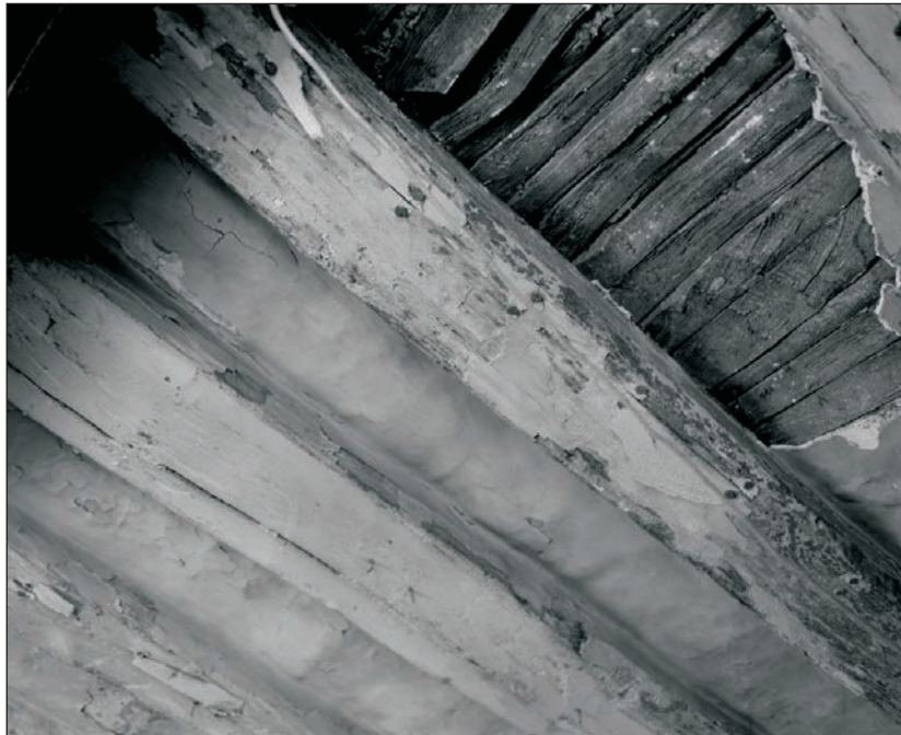
Plate 145: Detail of joists with lath and plaster infills of ceiling, G1, Building 2, during watching brief (Film 31.10)
