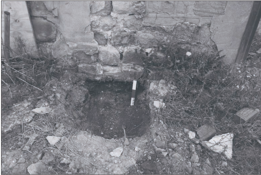
Plate 95: General view of Test Pit 2, against the west elevation of Building 1 (Film 36.04)
