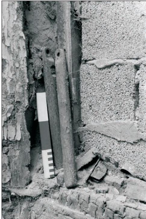
Plate 272: Detail of sash window weights, room G1, Building 4 (Film 29.01)
