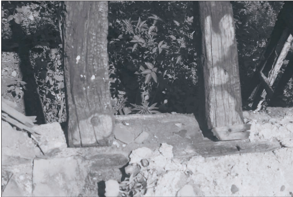
Plate 314: Detail of south wall plate, Building 3 (Film 25.08)
