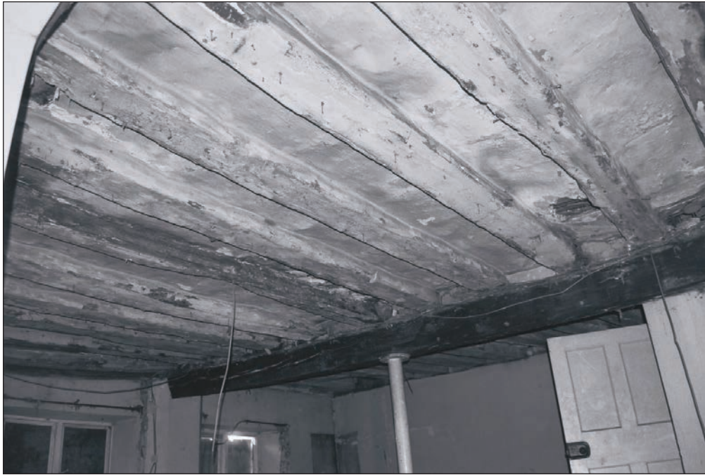
Plate 140: View of exposed ceiling of G1, Building 2, during watching brief (Film 30.03)
