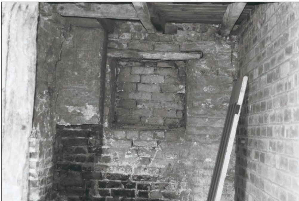
Plate 40: General internal view of G3, Building 1, showing blocked window and flue (Film 03.32)
