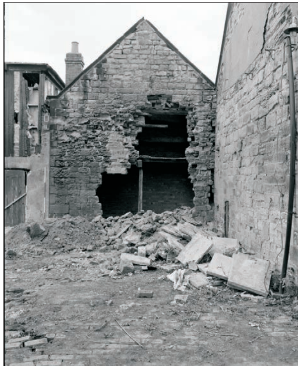
Plate 21: General view of the north elevation of the barn, Building 1 (Film 07.08)
