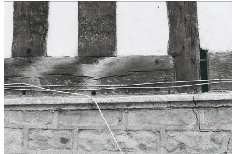
Plate 115: Detail of mid-rail, north elevation, Building 2 (Film 04.23)
