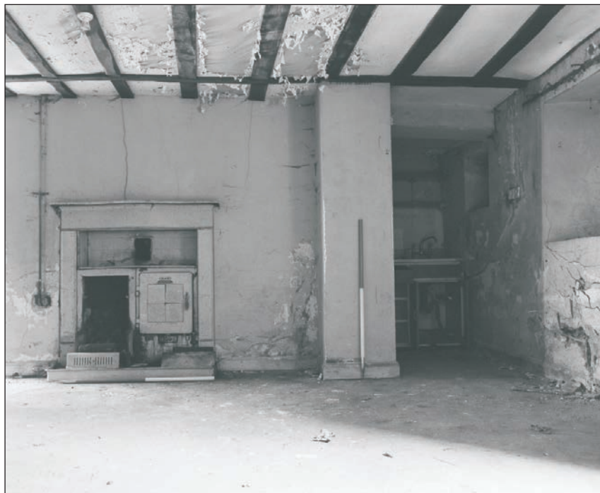
Plate 123: General view of G1, Building 2, showing fireplace and kitchen (Film 14.04)
