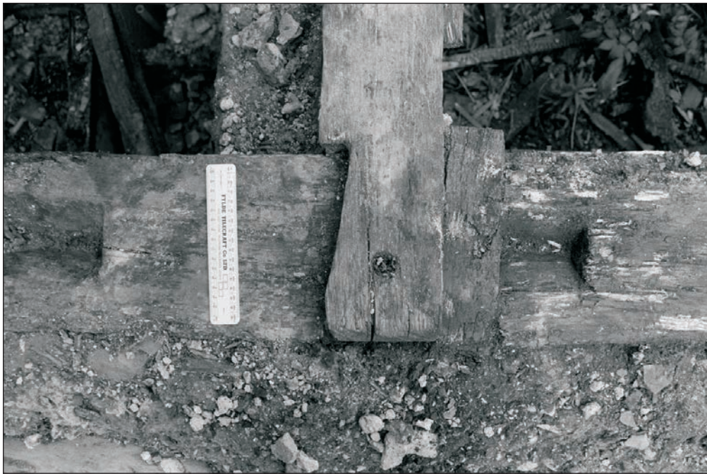
Plate 352: Detail of pegged joint, west wall plate, Building 4 (Film 27.29)
