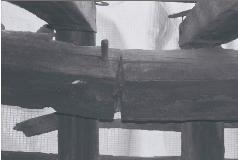
Plate 221: Detail of join in purlins, F1, Building 2 (Film 41.15)
