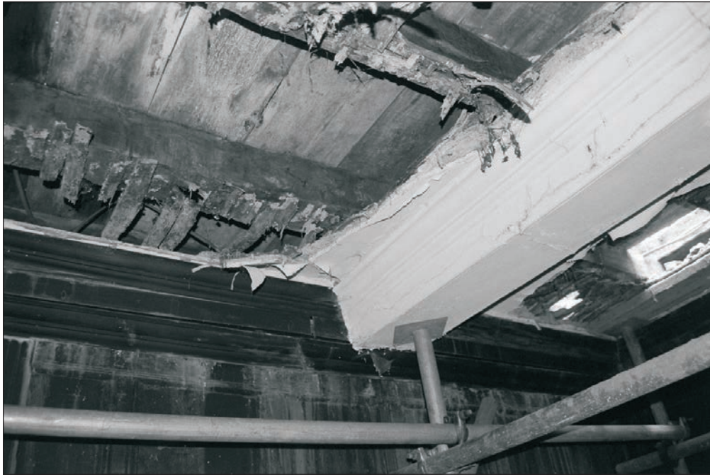
Plate 282: View of moulded ceiling beams, room G3, Building 4 (Film 29.21)
