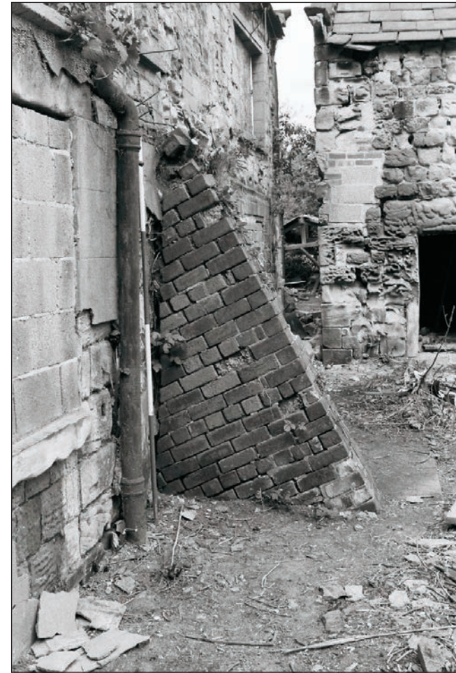
Plate 101: View of brick buttress, south elevation of Building 2 (Film 05.01)
