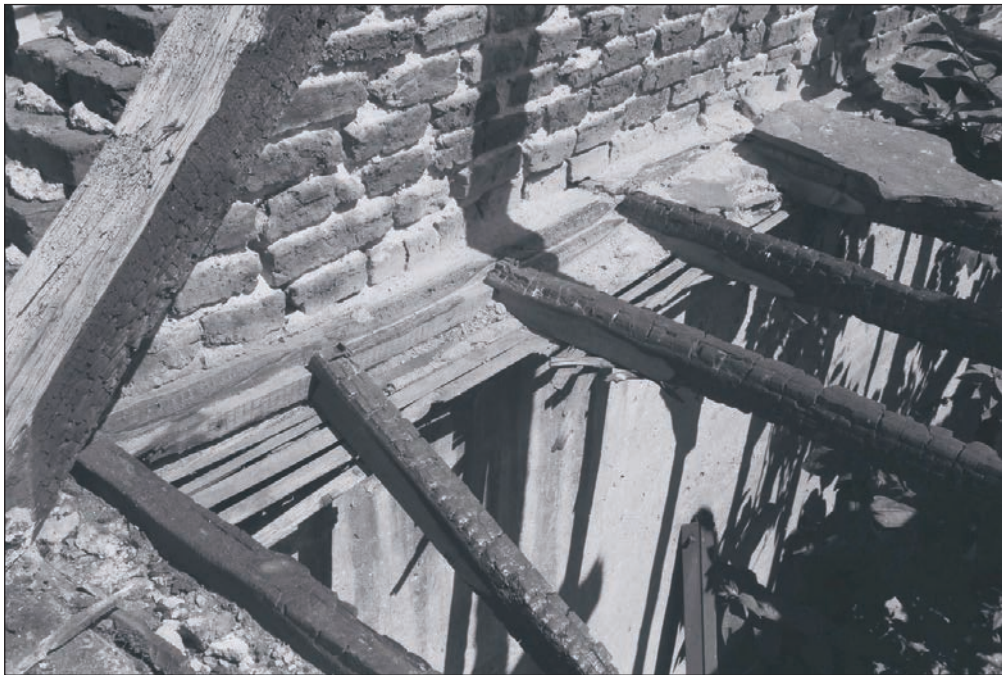
Plate 320: Detail of ceiling joists, south end of Building 4 (Film 25.20)
