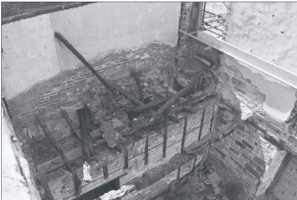
Plate 341: General view of first floor joists (F1), Building 4 (Film 26.27)
