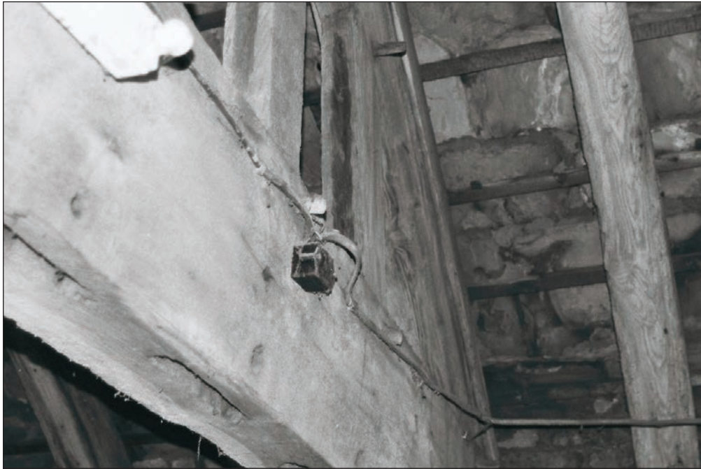
Plate 63: Detail of timber truss, F1, Building 1 (Film 03.11)
