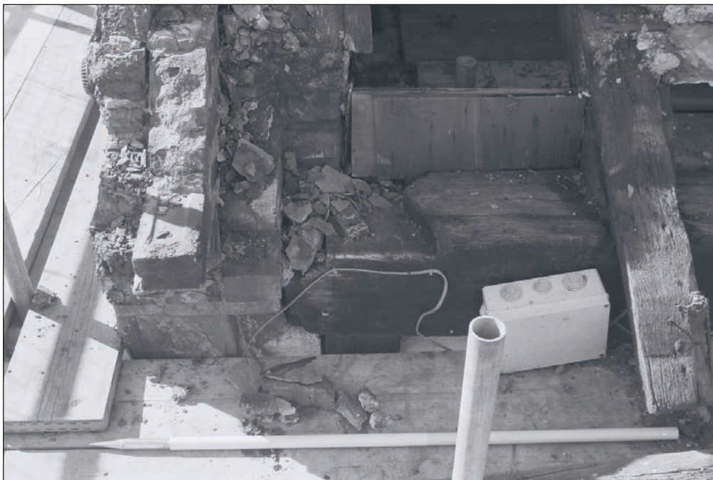
Plate 222: Detail of wall plate showing joint of removed principal rafter at east end of Building 2 (Film 41.07)
