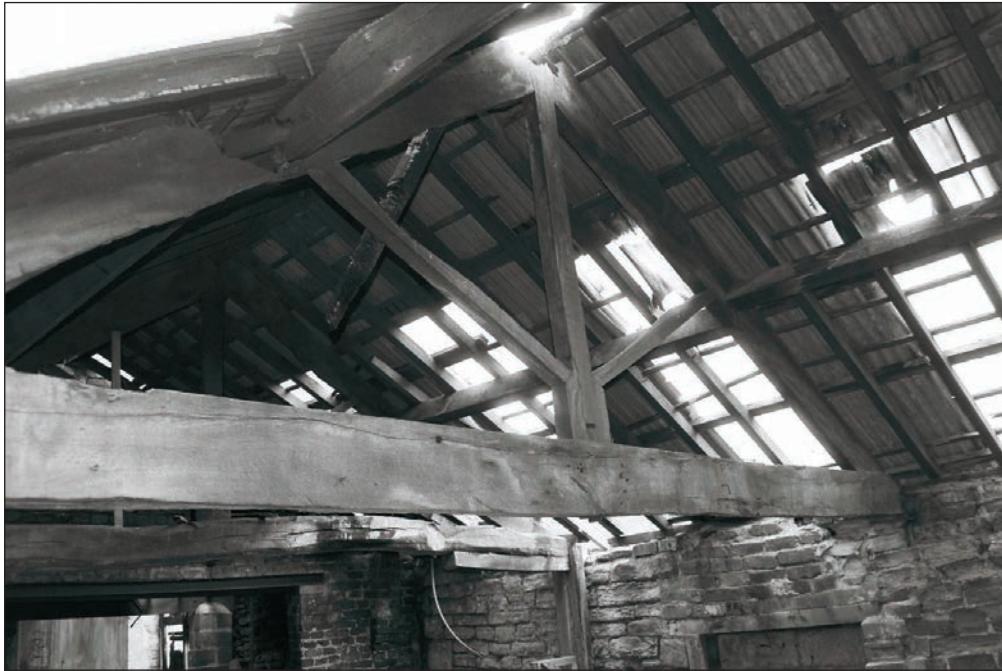
Plate 364: Detail of timber King-Post roof trusses within Building 5 (Film 06.31)
