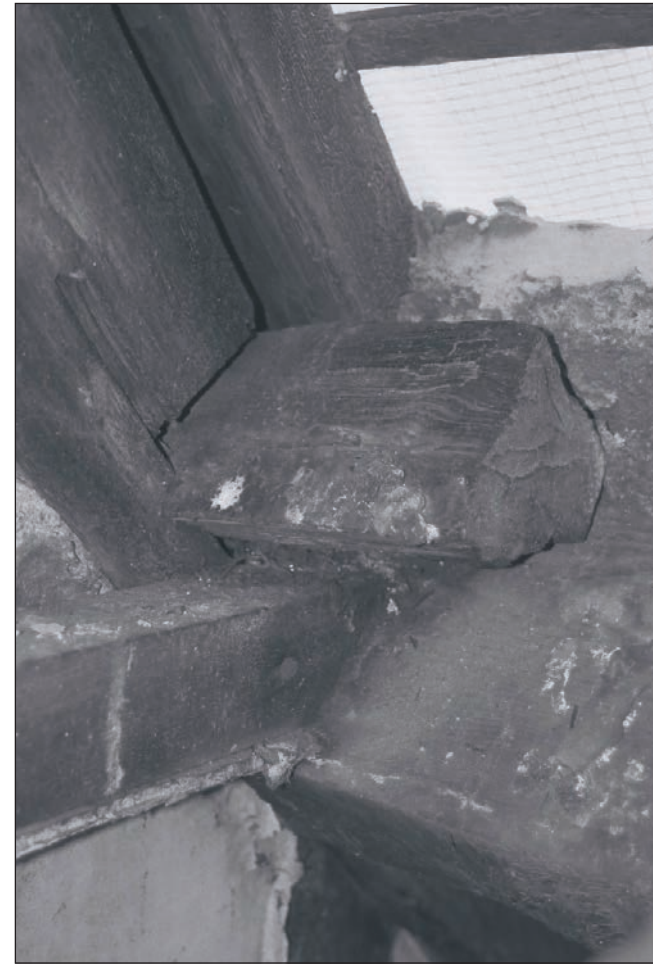
Plate 216: Detail of purlin and principal rafter, F1, Building 2 (Film 41.05)
