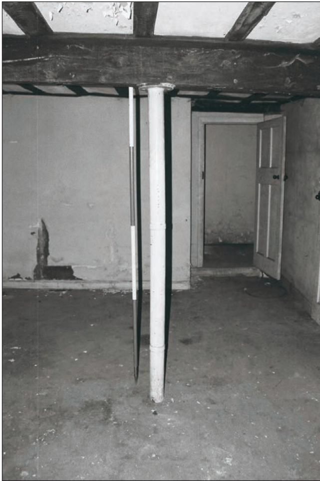
Plate 128: Detail of cast iron column, G1, Building 2 (Film 04.18)
