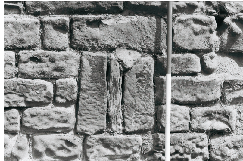
Plate 15: Detail of blocked breather slit, west elevation of the barn, Building 1 (Film 02.05)
