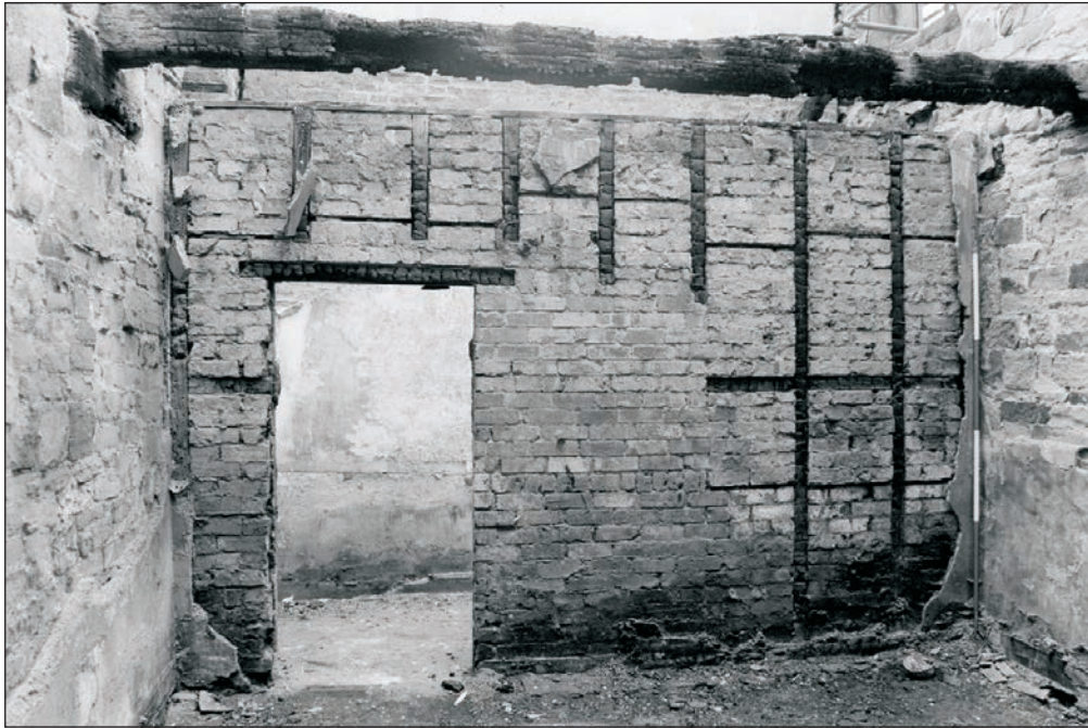
Plate 268: General view of room G1, showing altered south wall, Building 4 (Film 29.09)
