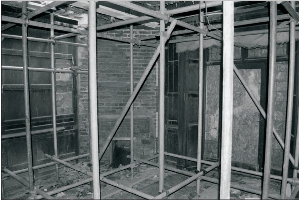
Plate 278: General view of room G3, Building 4 (Film 29.22)
