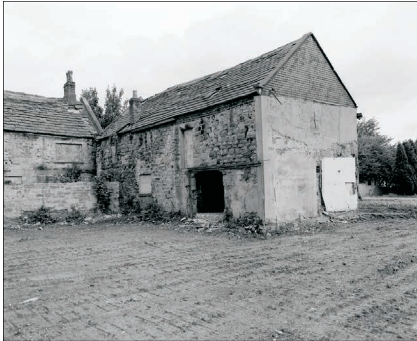
Plate 8: General view of the barn, Building 1 (Film 22.04)
