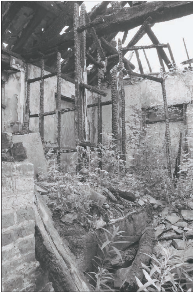
Plate 304: View of rooms F5 and F6, Building 3, from F3, Building 2 (Film 12.10)
