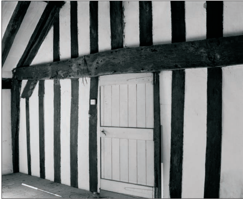
Plate 183: General view of F1, showing close stud partition, Building 2 (Film 16.05)
