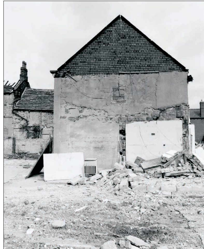
Plate 27: General view of the south elevation of the barn, Building 1, after the demolition of the extensions (Film 20.03)
