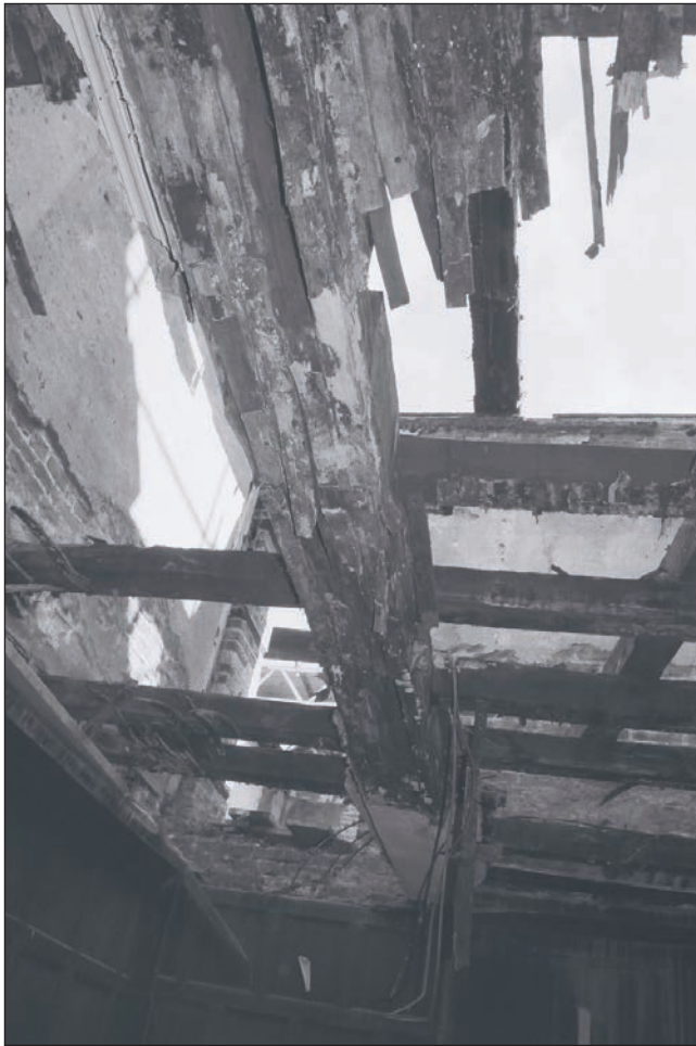
Plate 284: View of moulded ceiling beam and joists, room G3, Building 4 (Film 35.20)
