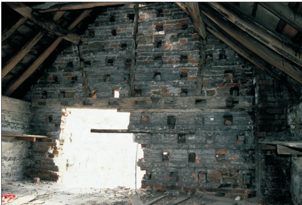
Plate 78: General view of Dovecote, F2, Building 1 (Colour Slide 10)
