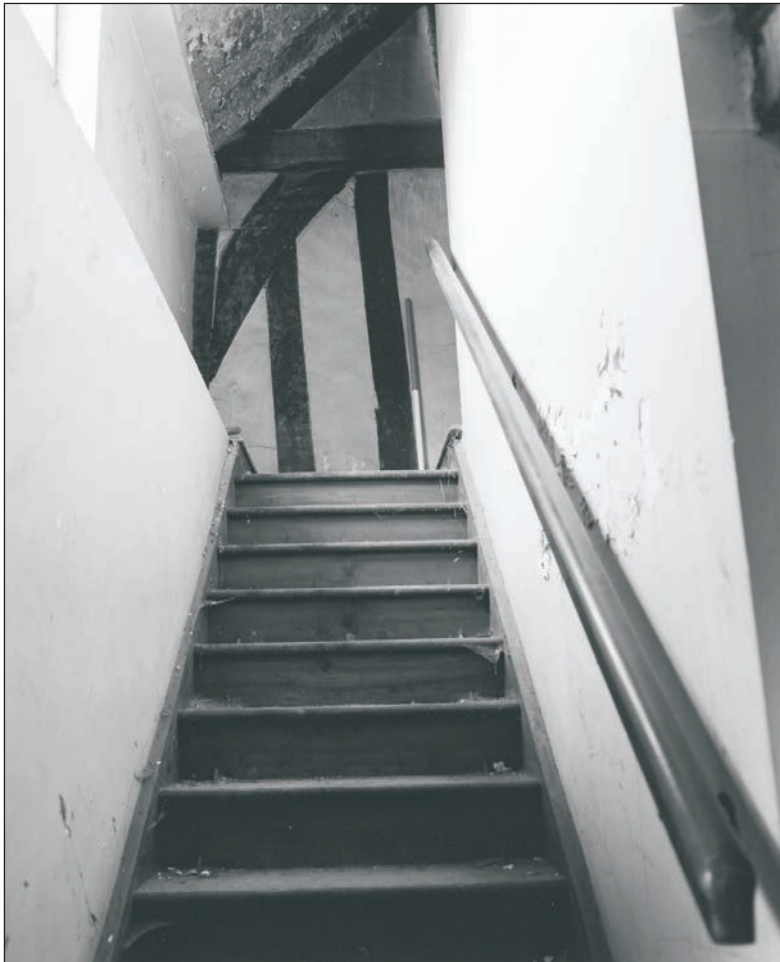
Plate 150: General view up staircase to first floor from G3, Building 2 (Film 15.02)
