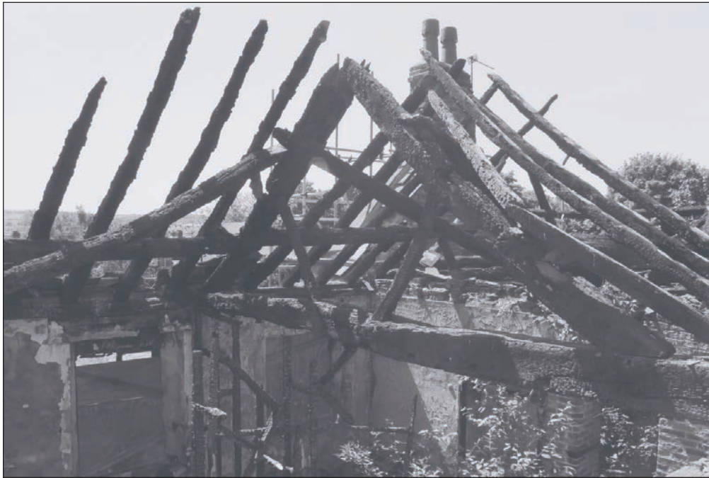
Plate 337: General view of roof timbers, Building 3 (Film 26.19)
