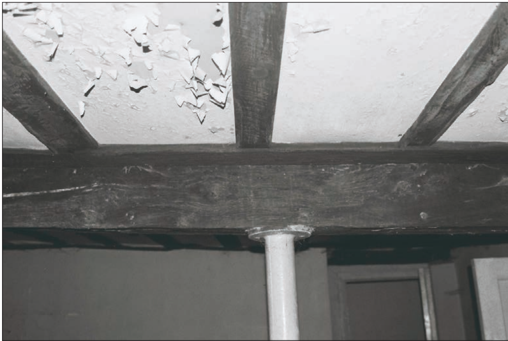
Plate 138: Detail of cast iron column and timber beam, G1, Building 2 (Film 06.07)
