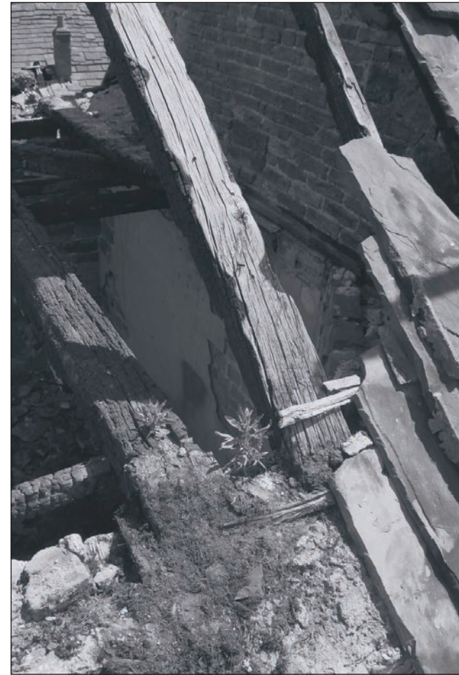
Plate 319: Detail of tie beam and rafter, west wall, Building 4 (Film 25.19)
