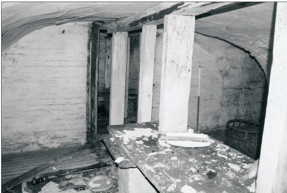
Plate 261: General view of room C2, Building 4 (Film 28.30)
