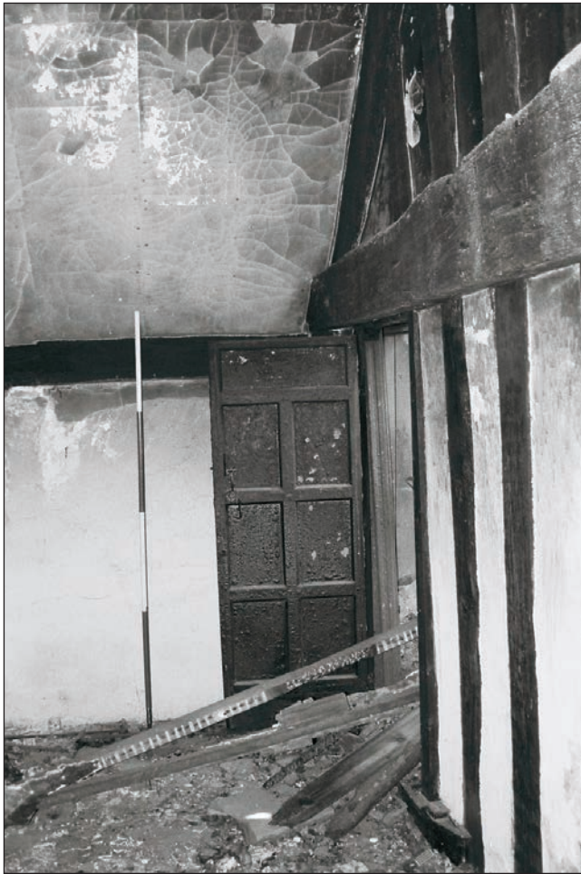
Plate 209: View of timber partition and inserted door, F3, Building 2 (Film 05.17)
