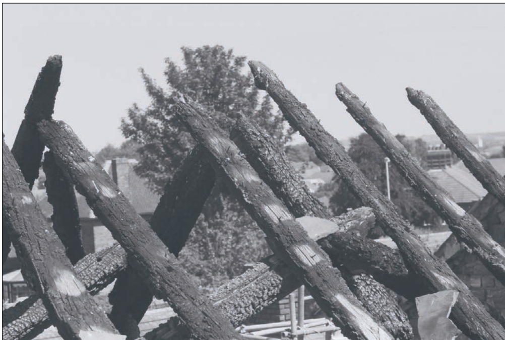
Plate 313: General view of common rafters and ridge of Building 3 (Film 25.07)
