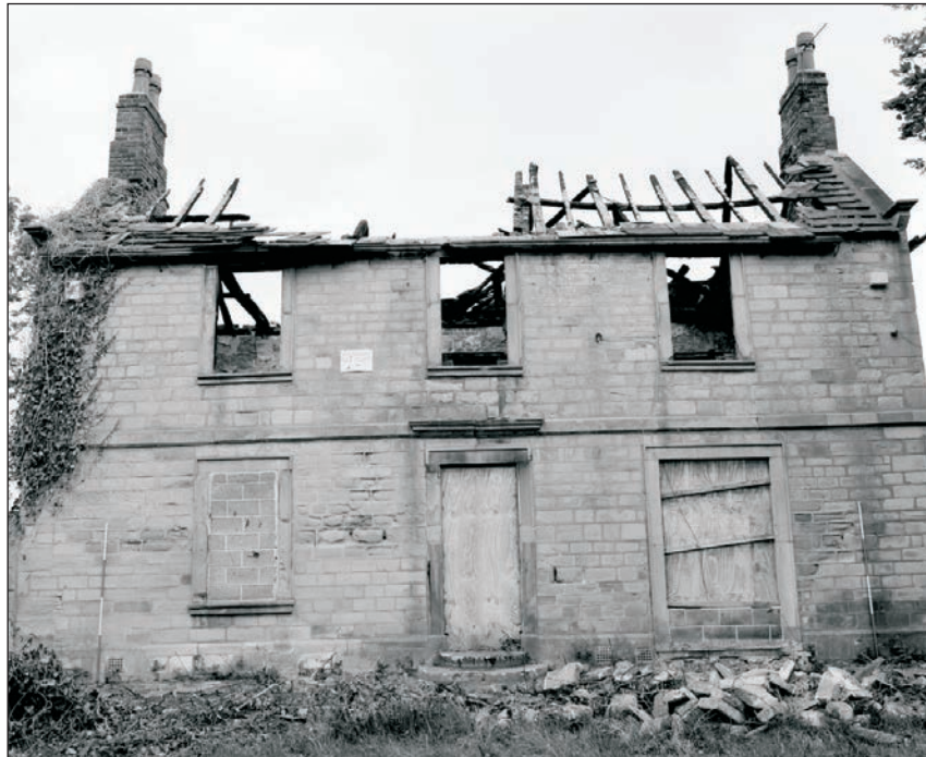
Plate 239: General view of the west elevation of Building 4 (Film 11.01)
