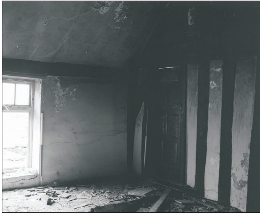
Plate 203: General view of F3, Building 2, showing close stud partition (Film 15.08)
