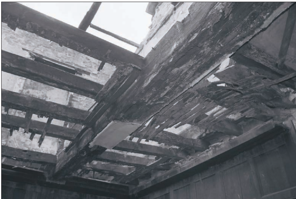
Plate 283: View of moulded ceiling beam and joists, room G3, Building 4 (Film 35.18)
