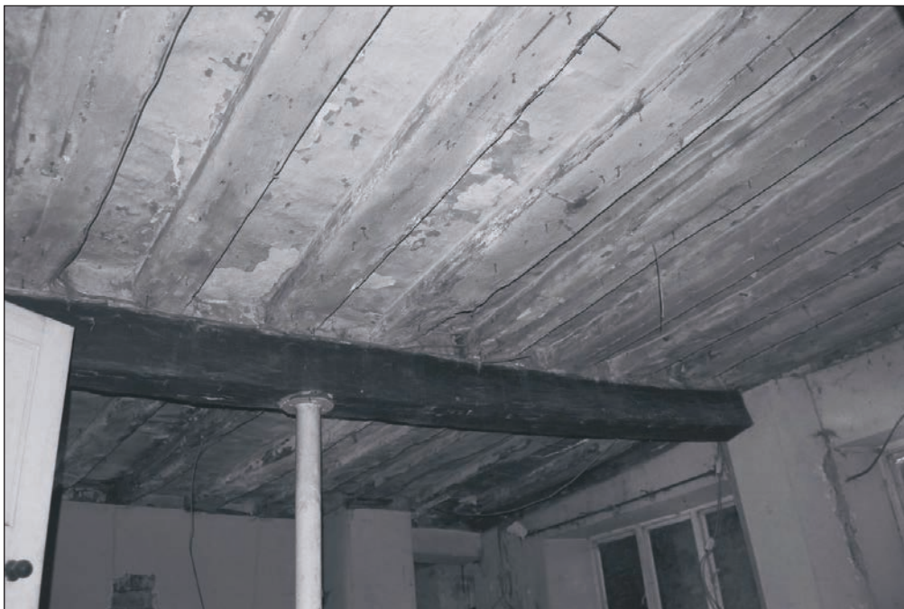
Plate 141: View of exposed ceiling of G1, Building 2, during watching brief (Film 30.04)
