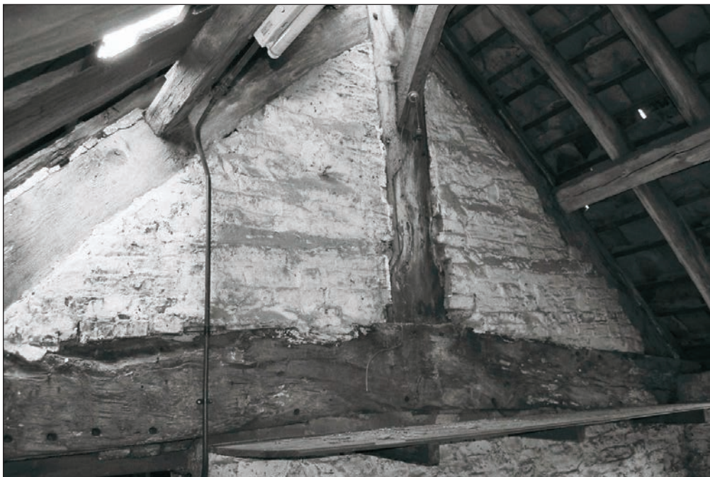
Plate 82: Detail of timber truss with later brick infill, F2, Building 1 (Film 06.09)
