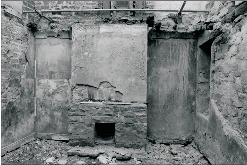
Plate 270: General view of room G1, showing altered fireplace, Building 4 (Film 29.13)
