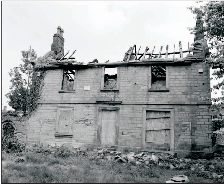
Plate 240: General view of the west elevation of Building 4 (Film 11.07)
