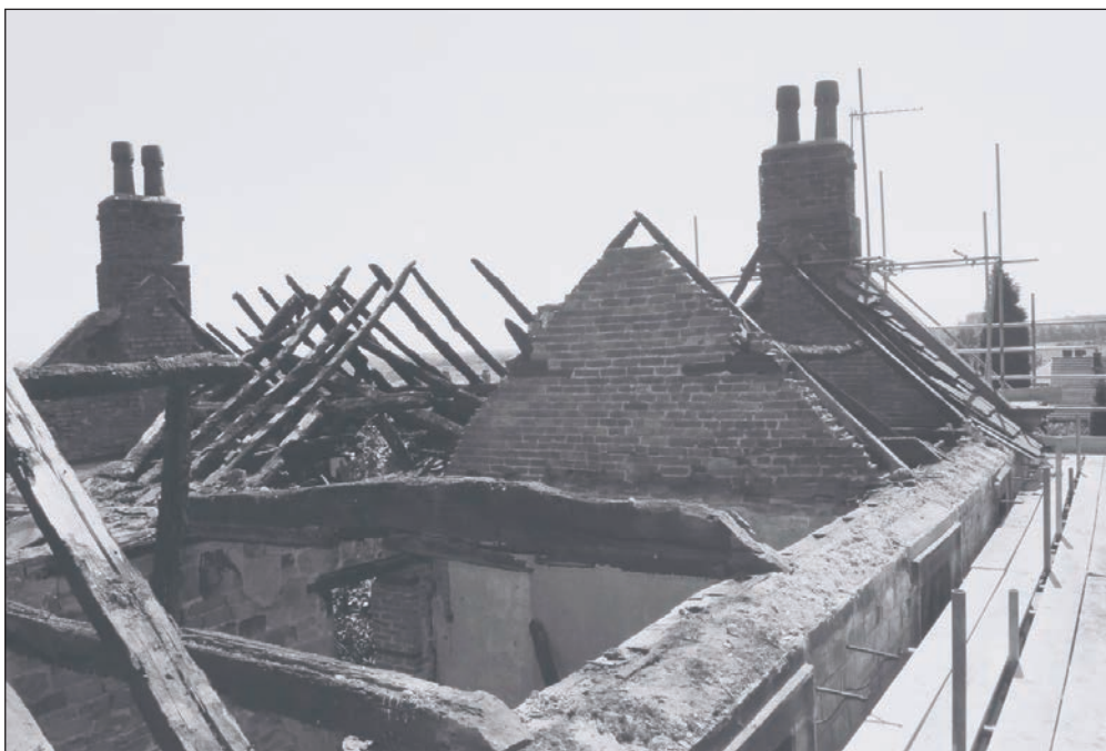
Plate 327: General view along roof of Building 4 (Film 25.35)
