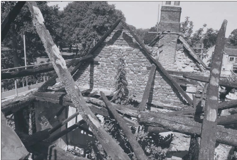
Plate 316: General view of roof timbers, Building 4 (Film 25.12)
