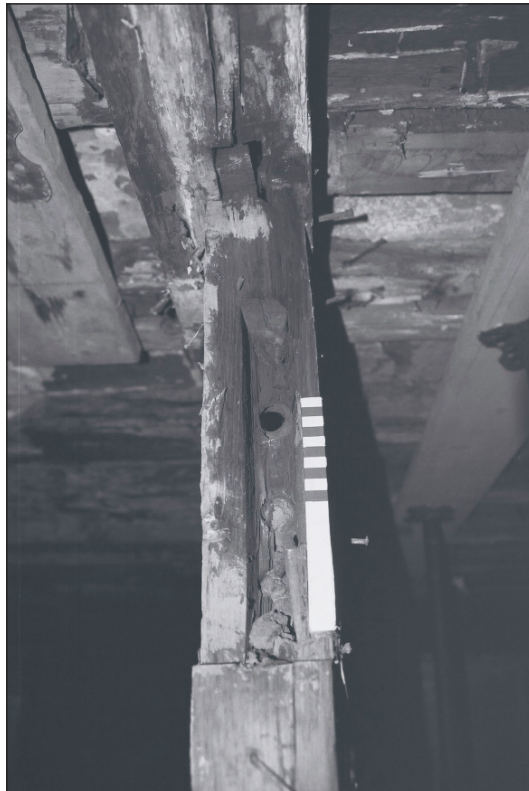
Plate 167: Detail of empty pegged mortice hole in post of primary timber framed partition in southeast corner of G3/north wall of G4, Building 2 (Film 42.01)
