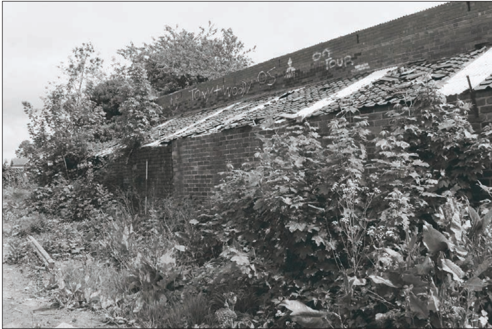
Plate 358: General view of the west elevation of Building 5 (Film 06.26)
