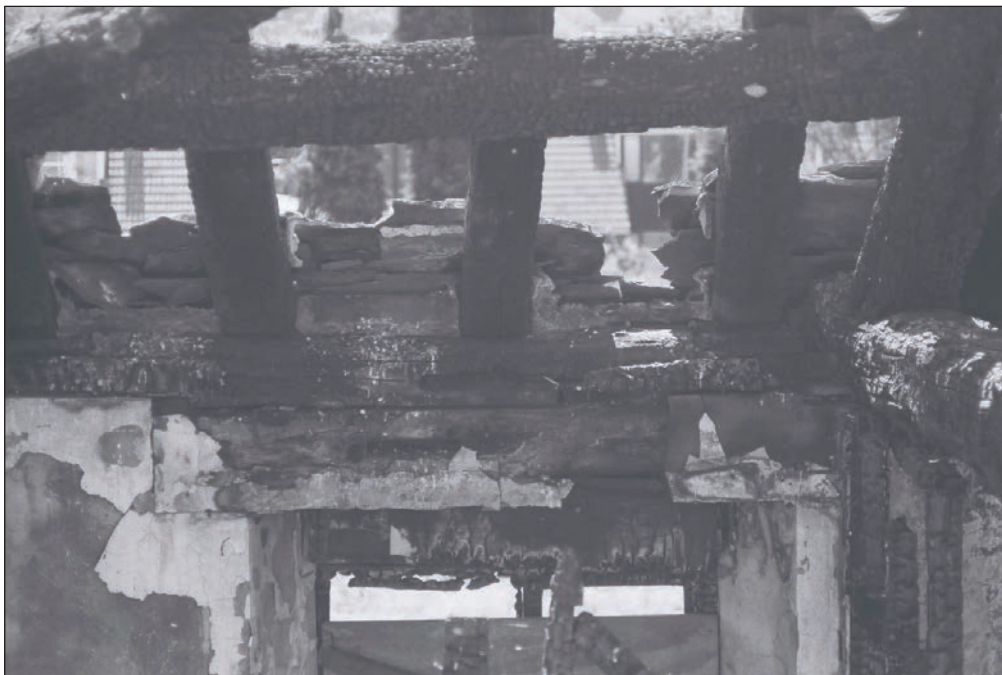
Plate 333: Detail of wall head, south wall of Building 3 (Film 26.10)
