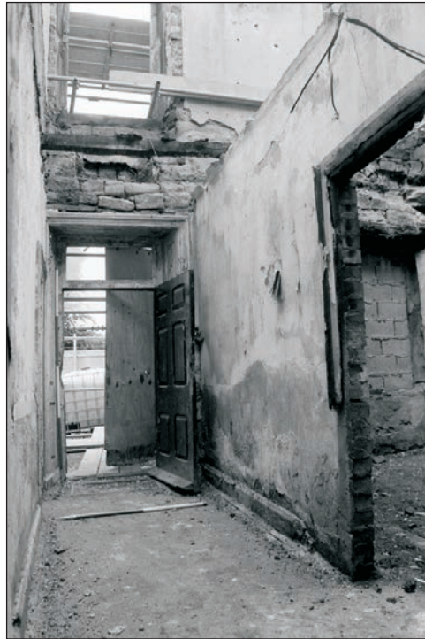
Plate 266: General view of hallway G2, showing main entrance, Building 4 (Film 29.33)
