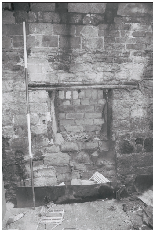
Plate 51: Detail of blocked window, east wall of F1, Building 1 (Film 18.34)
