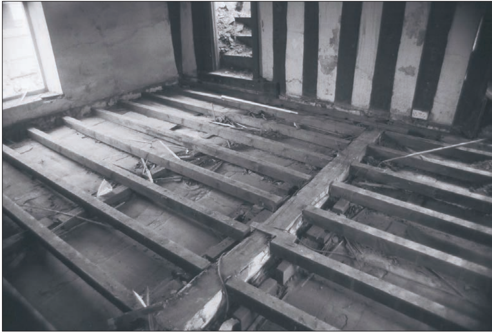
Plate 227: General view of lifted floor boards, F3, Building 2 showing limeash floor beneath (Film 40.01)
