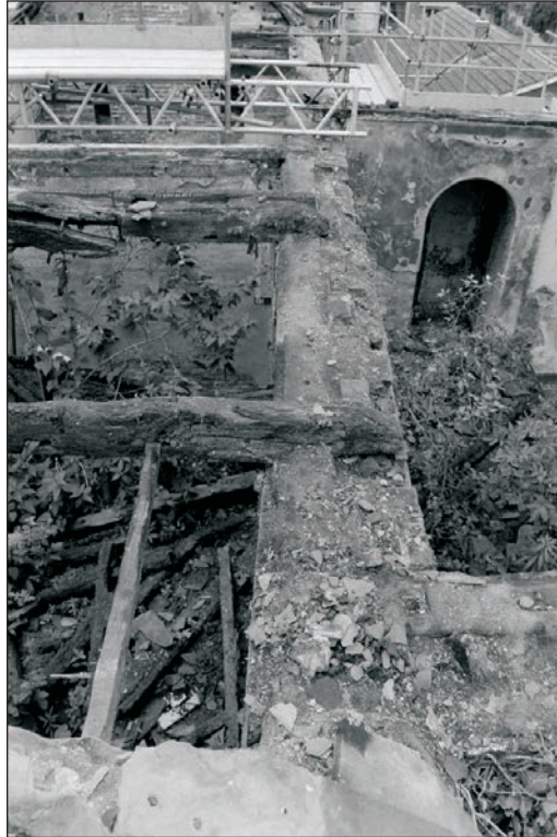
Plate 350: View along wall head, east wall, Building 4 (Film 27.28)
