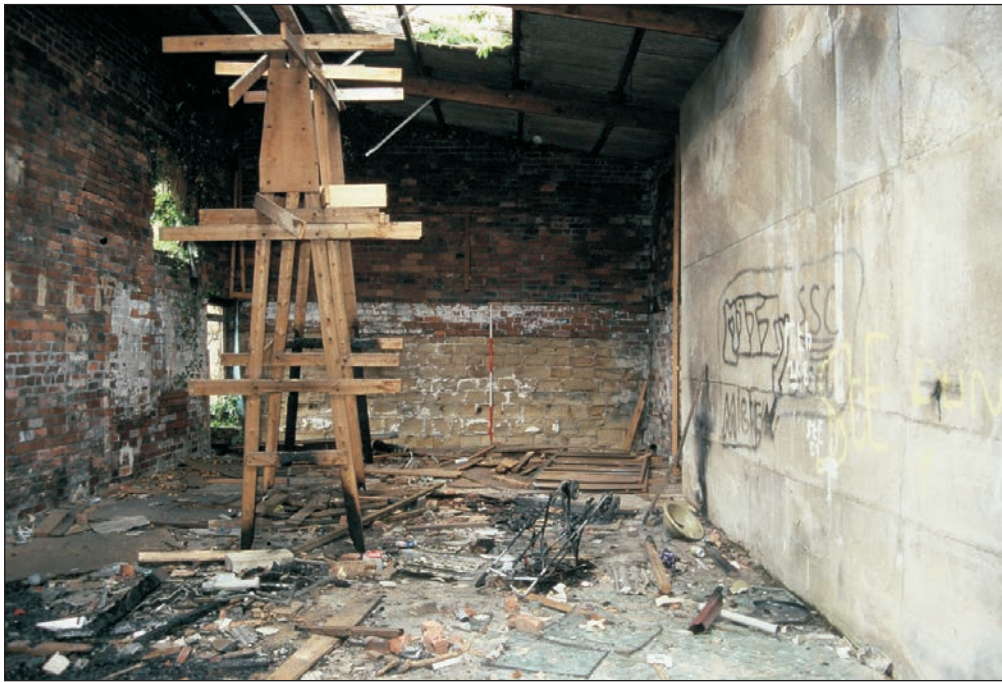
Plate 360: General internal view of Building 5 (Colour Slide 08)
