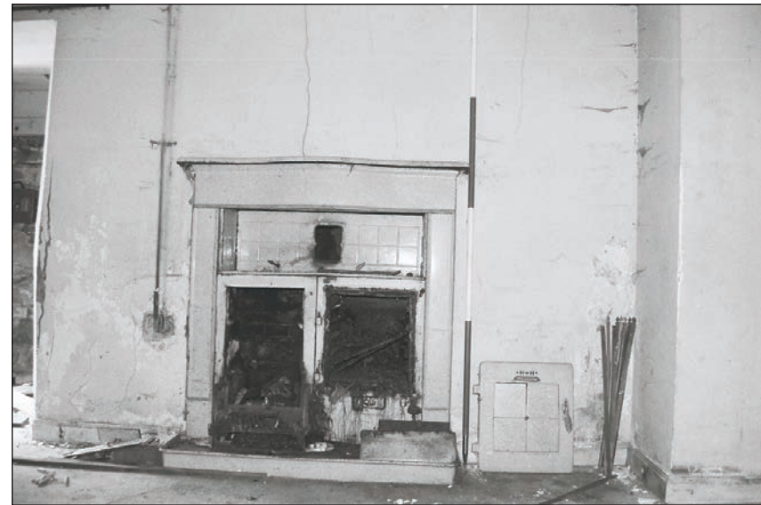
Plate 129: Detail of fireplace, G1, Building 2 (Film 04.20)
