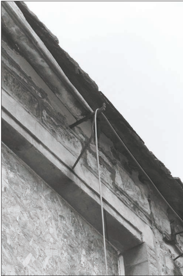
Plate 102: Detail of gutter bracket, south elevation of Building 2 (Film 04.33)
