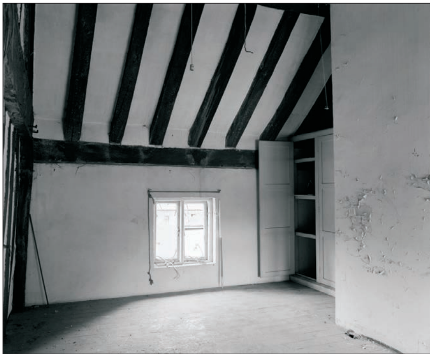
Plate 188: General view of F1, showing window to the north, Building 2 (Film 17.01)
