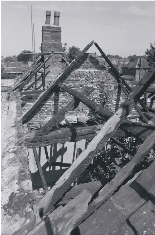
Plate 318: View along wall head, west wall of Building 4 (Film 25.17)
