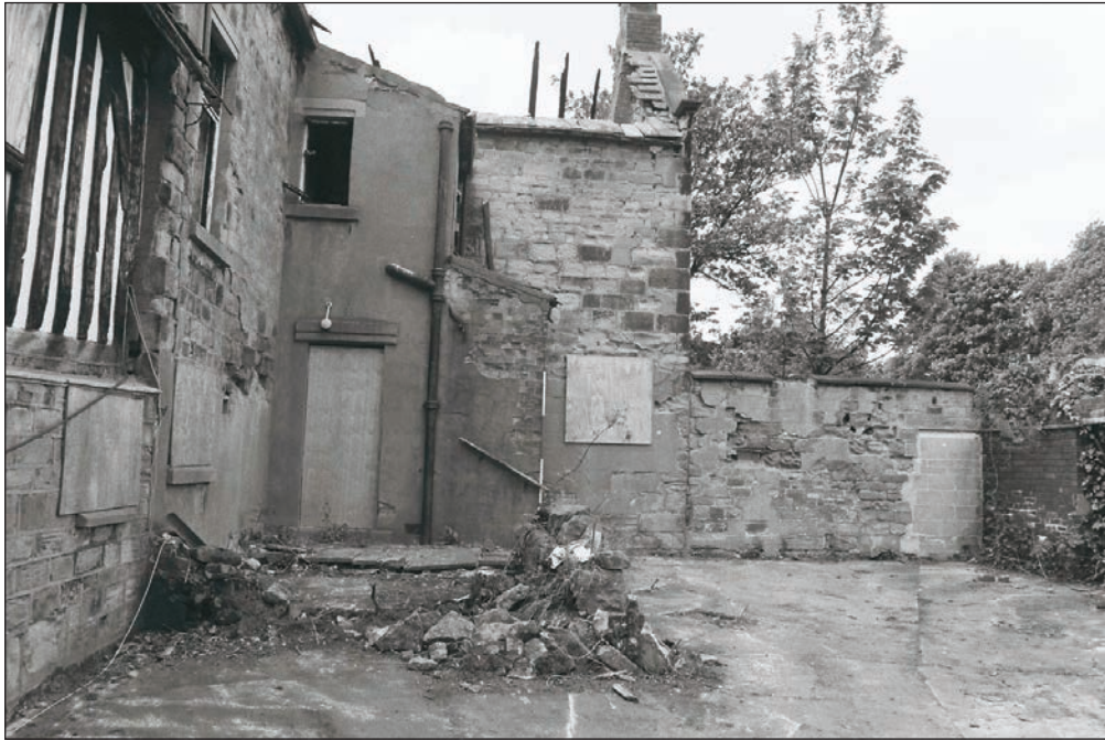
Plate 246: General view of the east elevation of Building 4 (Film 01.05)
