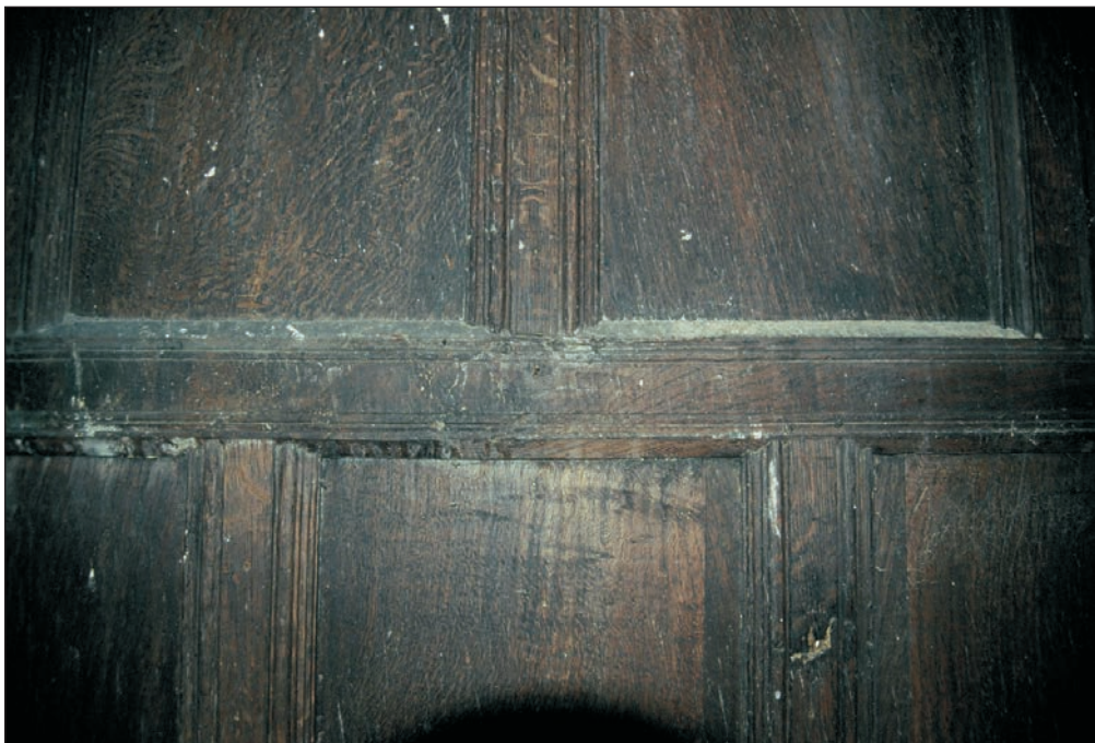
Plate 279: Detail of the Type 3 oak panelling on the east wall of room G3, Building 4 (Colour Slide 50)
