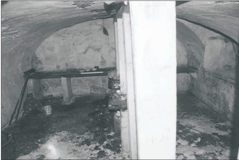
Plate 260: General view of room C2, Building 4 (Film 28.29)
