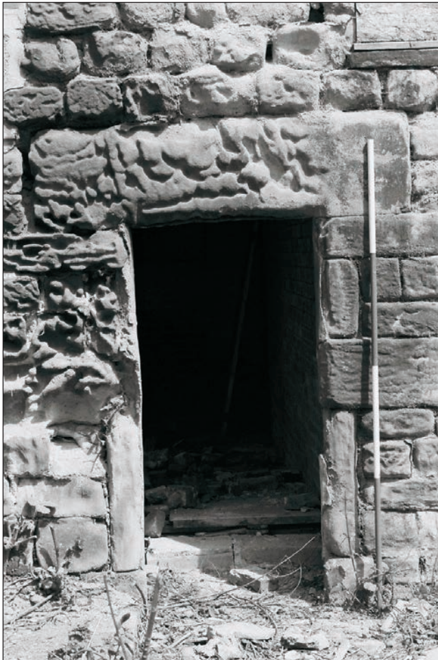
Plate 14: Detail of doorway, west elevation of the barn, Building 1 (Film 02.03)
