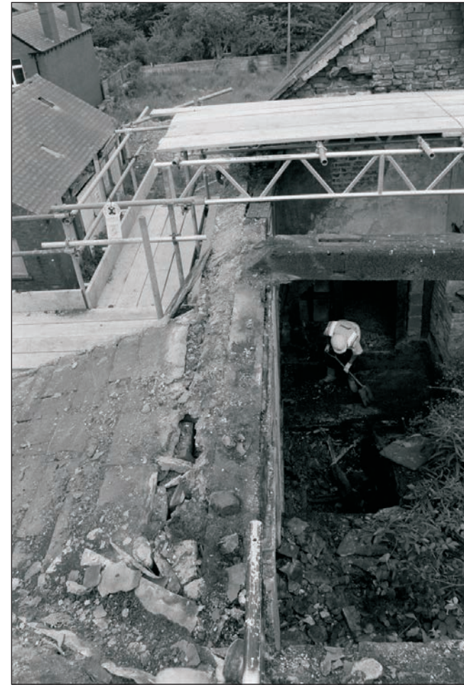
Plate 347: General view along wall head, north wall, Building 3 (Film 27.20)
