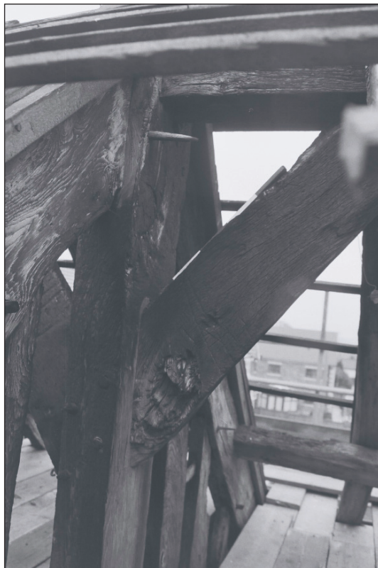
Plate 72: Detail of King-Post and ridge braces during watching brief, Building 1 (Film 39.19)
