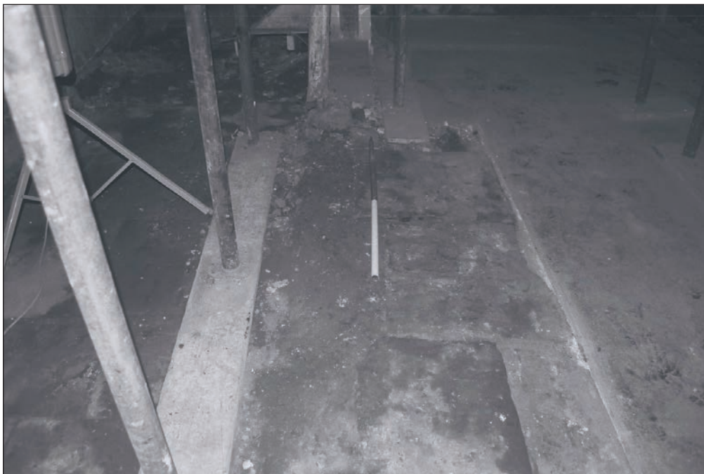
Plate 163: Detail of stone flagged surface showing position of removed primary timber partition, watching brief, G4, Building 2 (Film 42.08)
