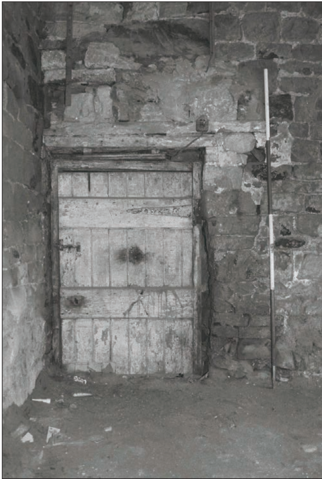
Plate 37: Detail of doorway in the south wall of G1, Building 1 (Film 24.07)
