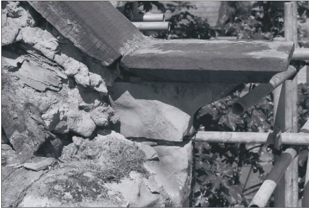
Plate 328: Detail of north gable east kneeler, Building 4 (Film 26.01)
