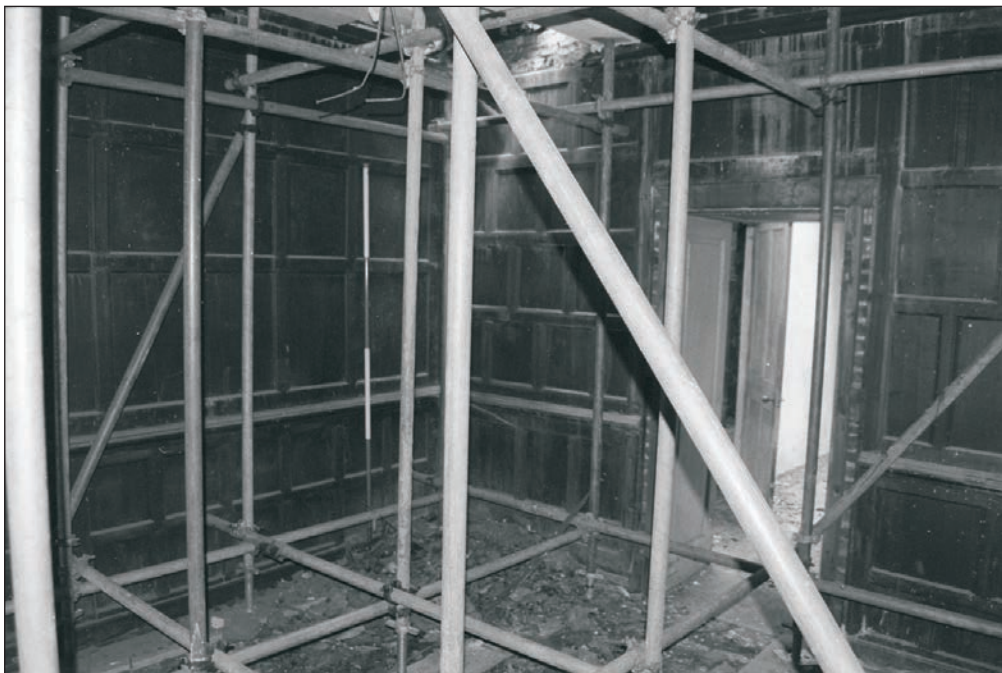
Plate 277: General view of room G3, Building 4 (Film 29.19)
