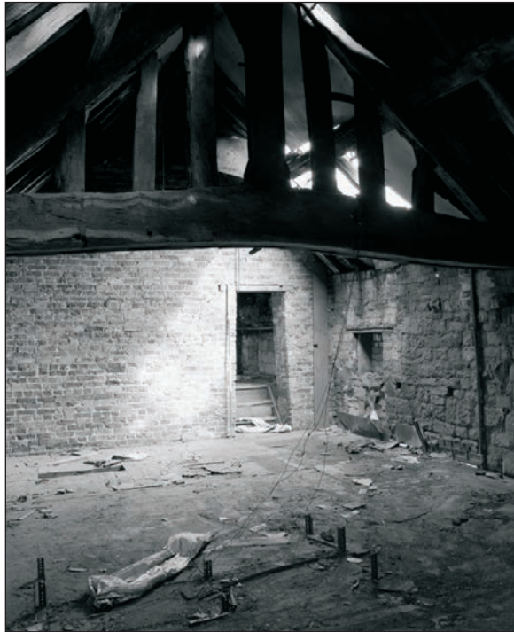
Plate 47: General view of F1, Building 1 (Film 19.02)
