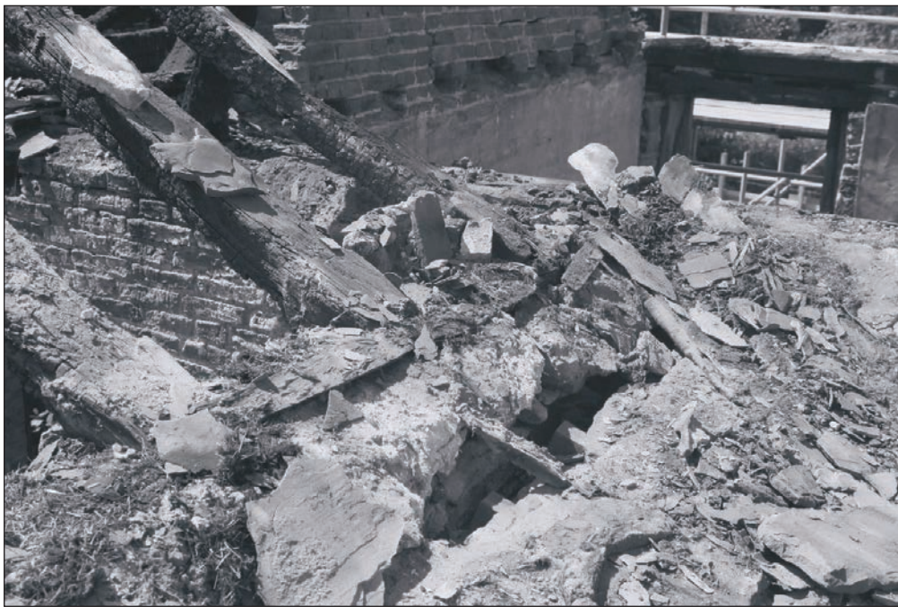
Plate 339: Detail of wall head and rafters, north wall of Building 3 (Film 26.23)
