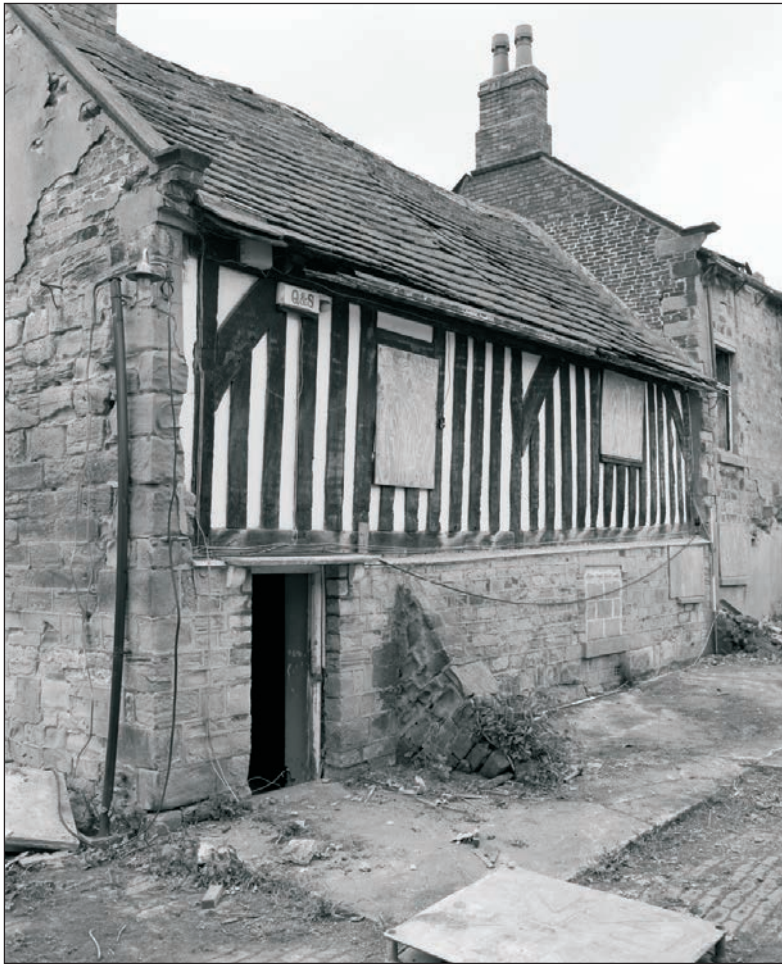
Plate 108: General view of the north elevation of Building 2 (Film 09.03)
