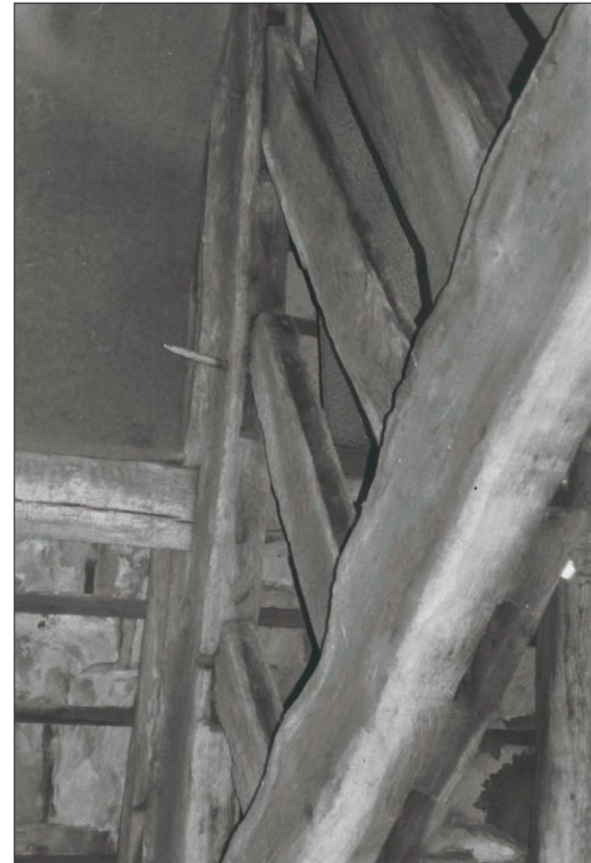
Plate 60: Detail of timber truss, F1, Building 1 (Film 24.20)
