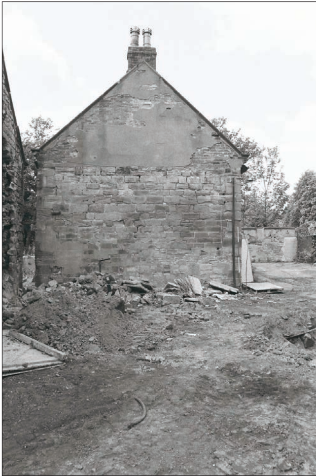
Plate 104: General view of the east elevation of Building 2 (Film 01.13)
