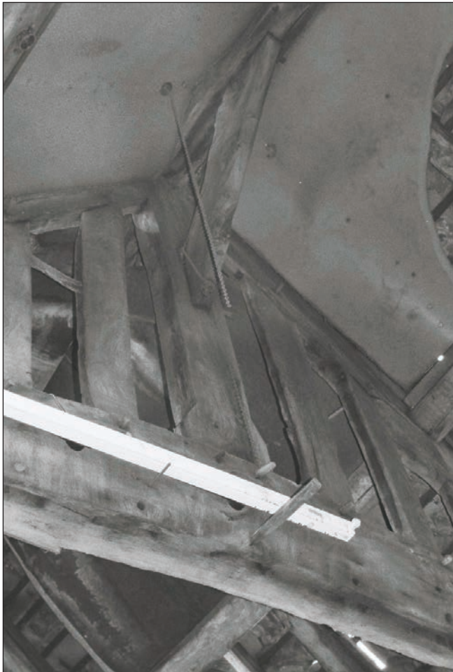
Plate 59: Detail of timber truss, F1, Building 1 (Film 24.12)
