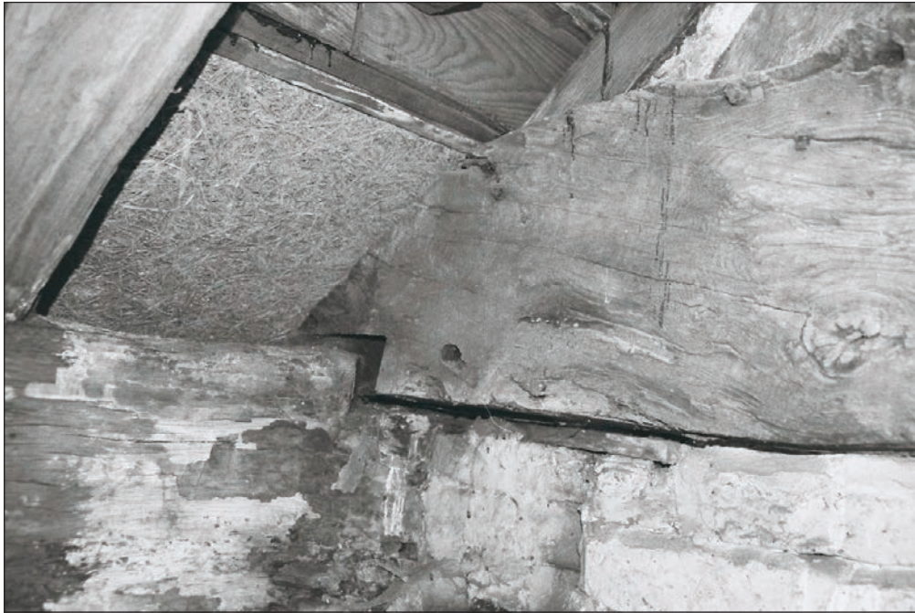
Plate 83: Detail of tie beam and wall plate, F2, Building 1 (Film 03.04)
