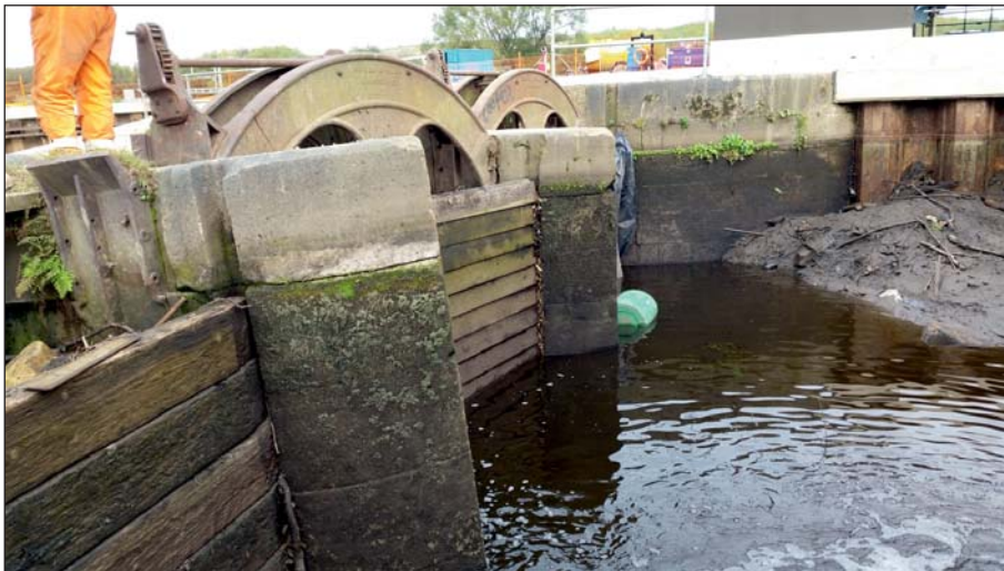
Plate 38: View of the sluices from upstream post-piling (Client Digital 38)
