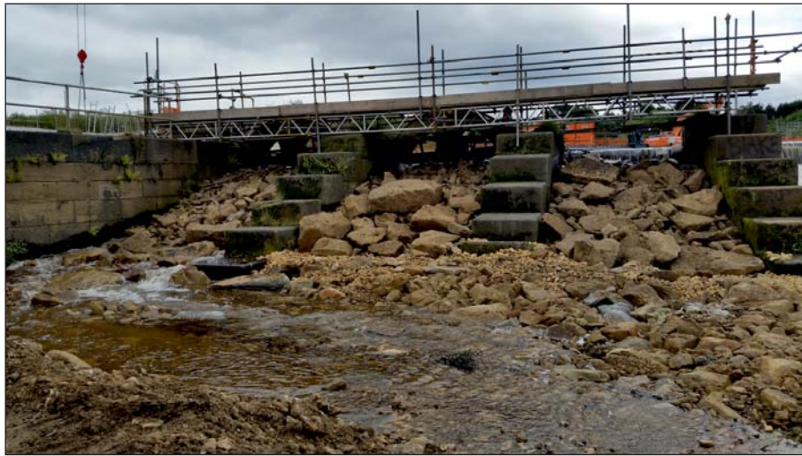
Plate 35: View of the sluices and piers from downstream post-piling (Client Digital 35)
