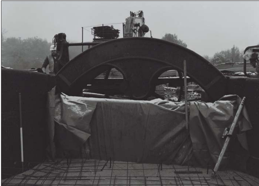
Plate 51: Detail of central sluice from upstream (Film 2.10)
