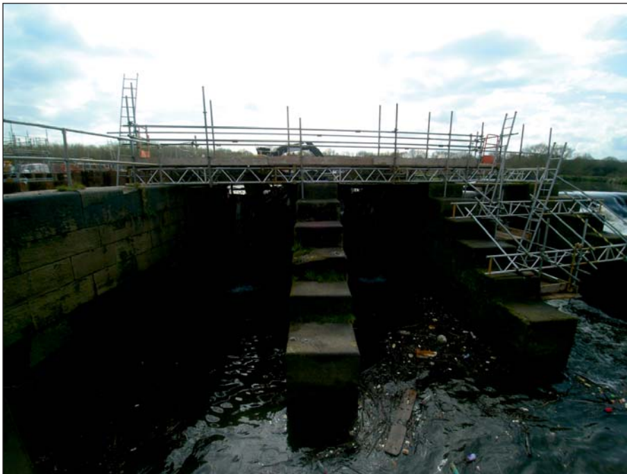
Plate 16: General view of sluices from downstream during works (Client Digital 16)
