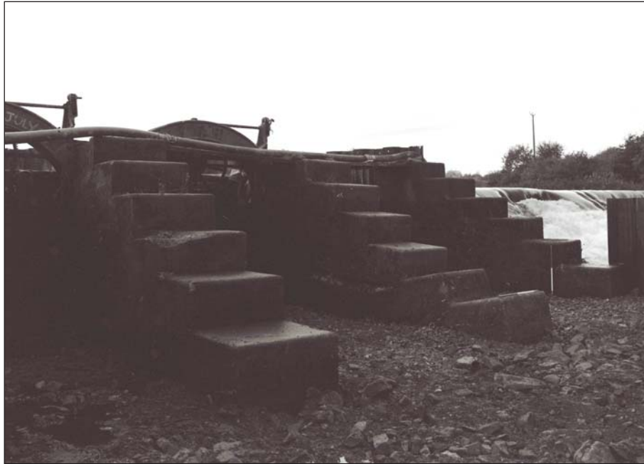
Plate 53: General view of sluices and piers from downstream (Film 3.2)
