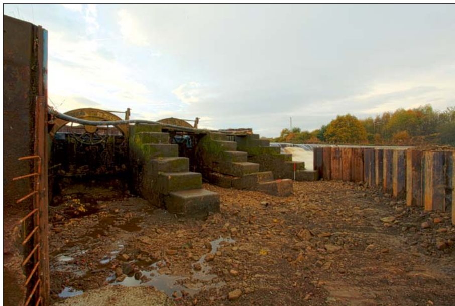
Plate 54: General view of sluices and piers from downstream (Digital IMG_0219)
