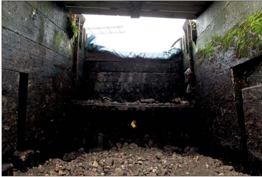
Plate 67: Detail view of the downstream westernmost sluice, showing arched opening (Digital IMG_0238)
