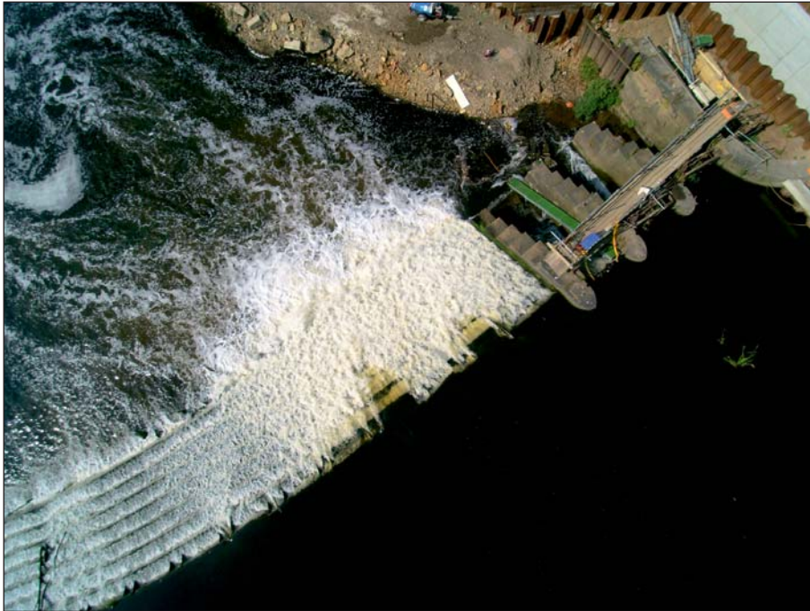
Plate 19: Aerial view of sluices and weir during works (Client Digital 19)
