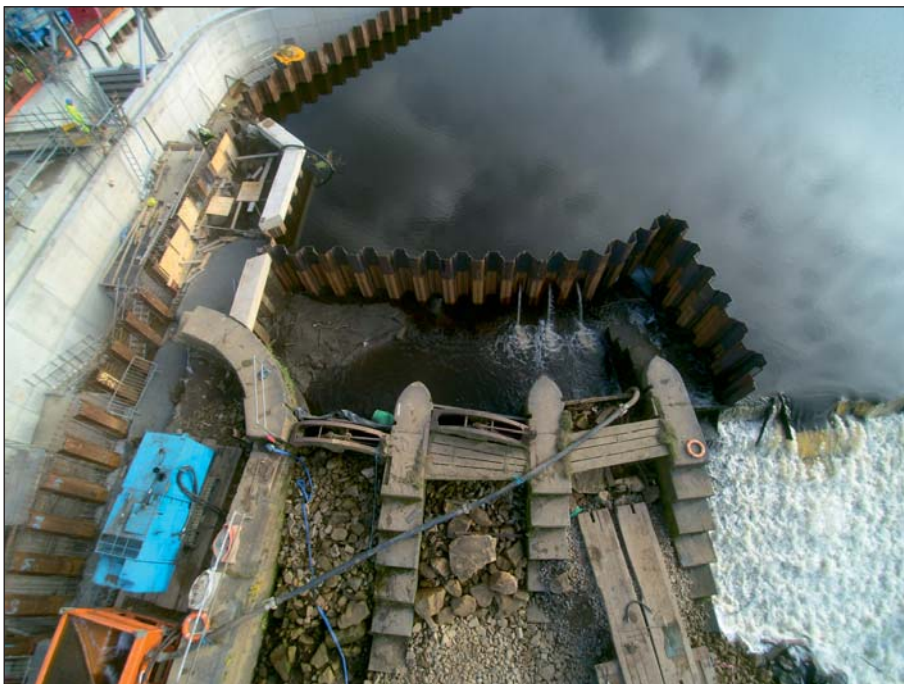
Plate 34: Aerial view of wingwall and sluices post-piling (Client Digital 34)
