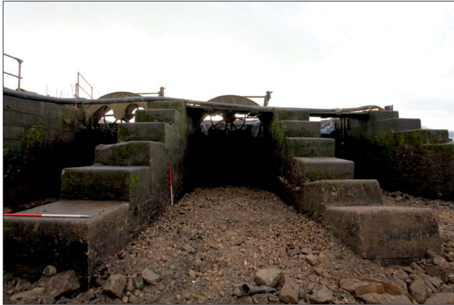
Plate 61: View of the downstream central sluice (Digital IMG_0229)
