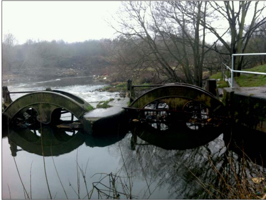
Plate 5: View of sluices from upstream prior to works (Client Digital 5)
