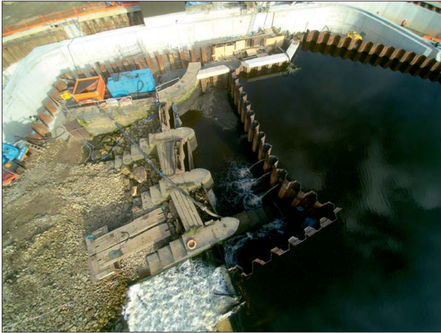
Plate 31: Aerial view of wingwall and sluices post-piling (Client Digital 31)
