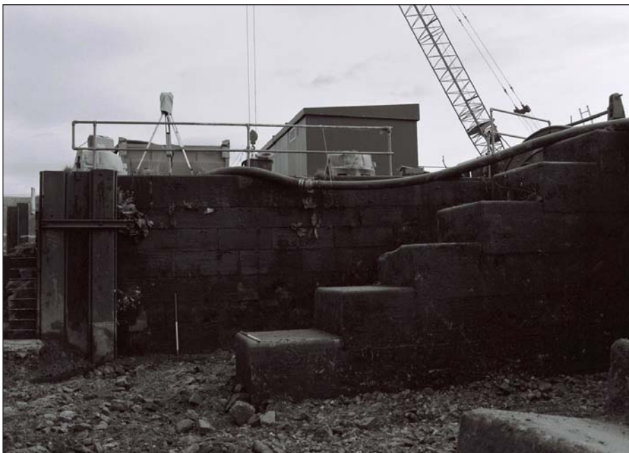
Plate 56: General view of the downstream easternmost sluice pier and wingwall (Film 4.3)
