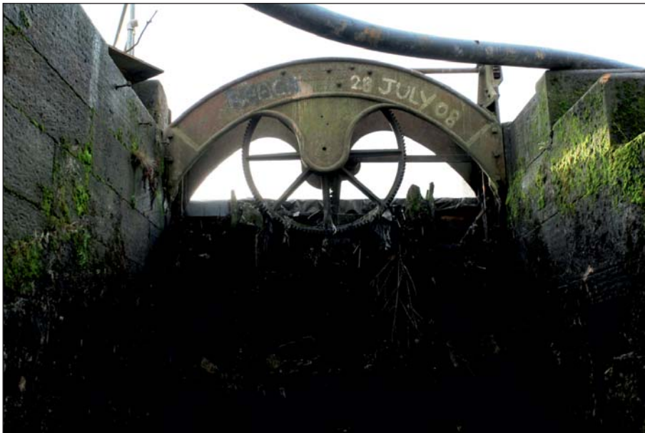
Plate 60: View of the downstream easternmost sluice (Digital IMG_0261)
