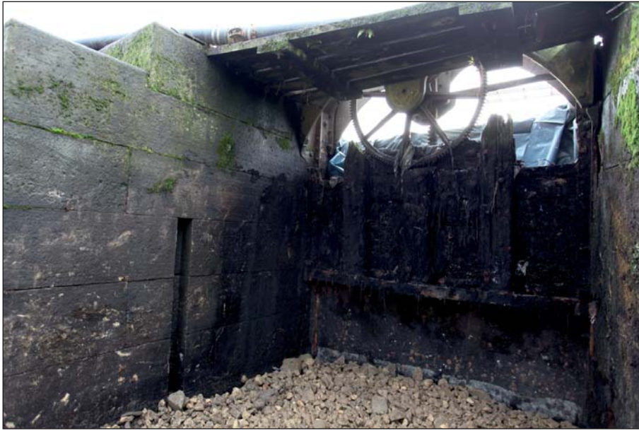
Plate 63: Detail view of the downstream central sluice (Digital IMG_0251)
