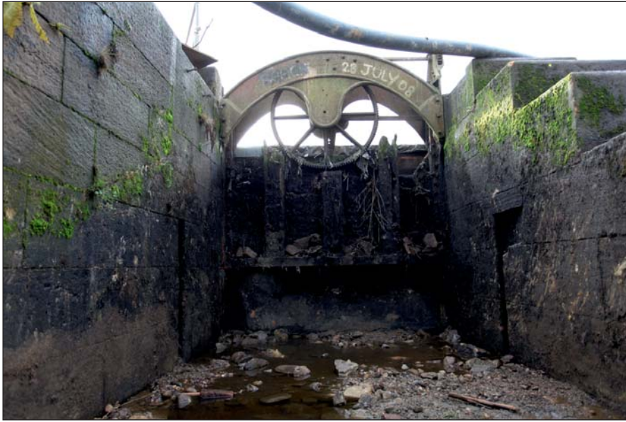
Plate 59: View of the downstream easternmost sluice (Digital IMG_0263)
