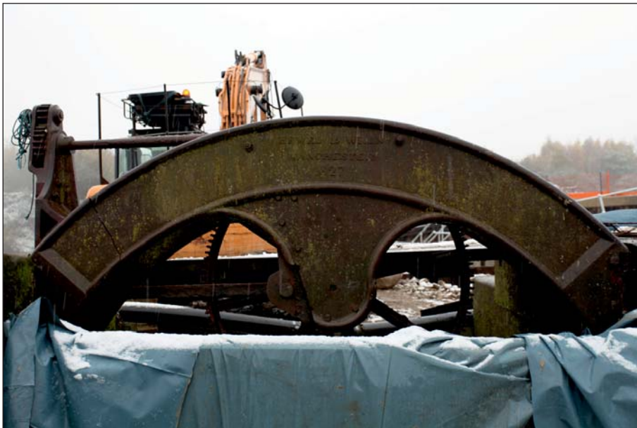
Plate 52: Detail of central sluice cast iron mechanism from downstream (Digital IMG_0211)
