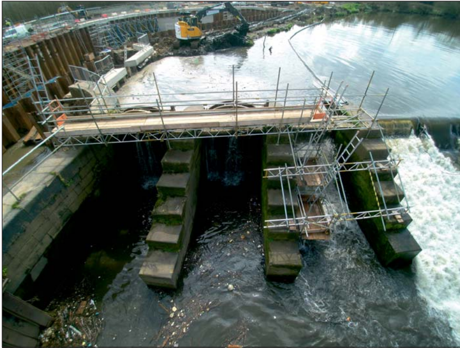
Plate 17: Aerial view of sluices during works (Client Digital 17)
