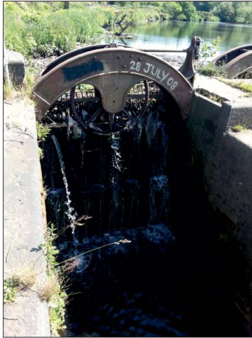
Plate 11: Detail of easternmost sluice and mechanism from downstream, prior to works (Client Digital 11)
