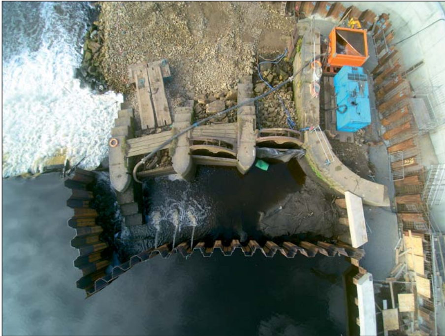
Plate 33: Aerial view of wingwall and sluices post-piling (Client Digital 33)
