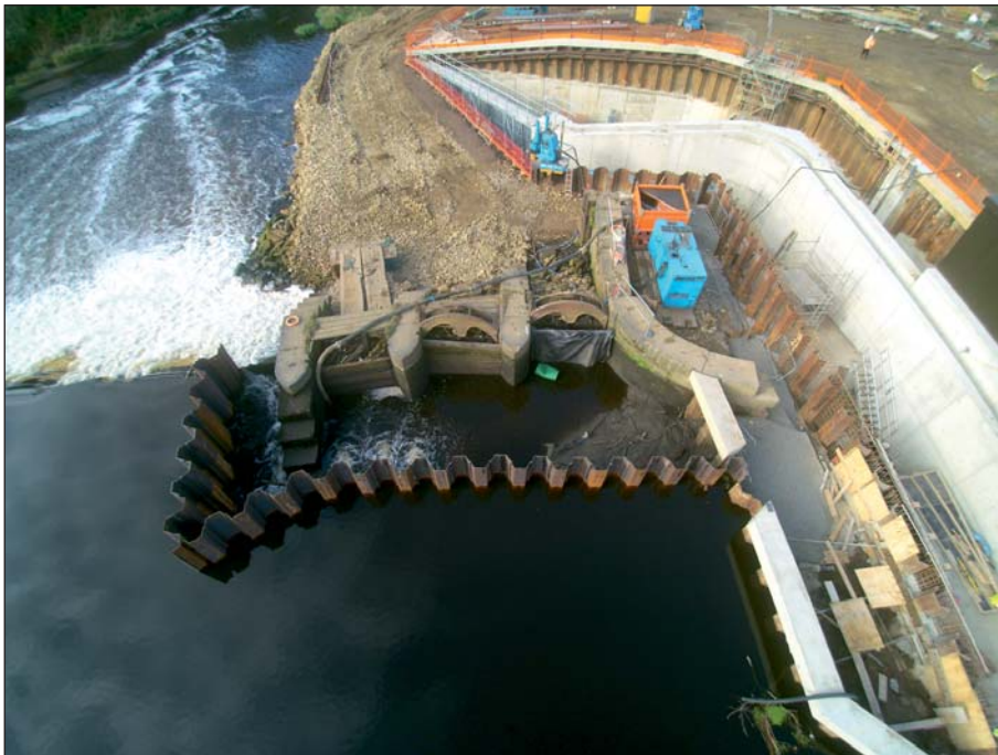
Plate 32: Aerial view of wingwall and sluices post-piling (Client Digital 32)
