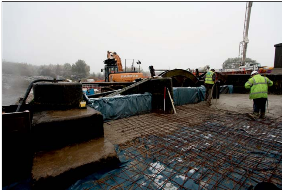
Plate 48: General view of sluices from upstream (Digital IMG_0207)
