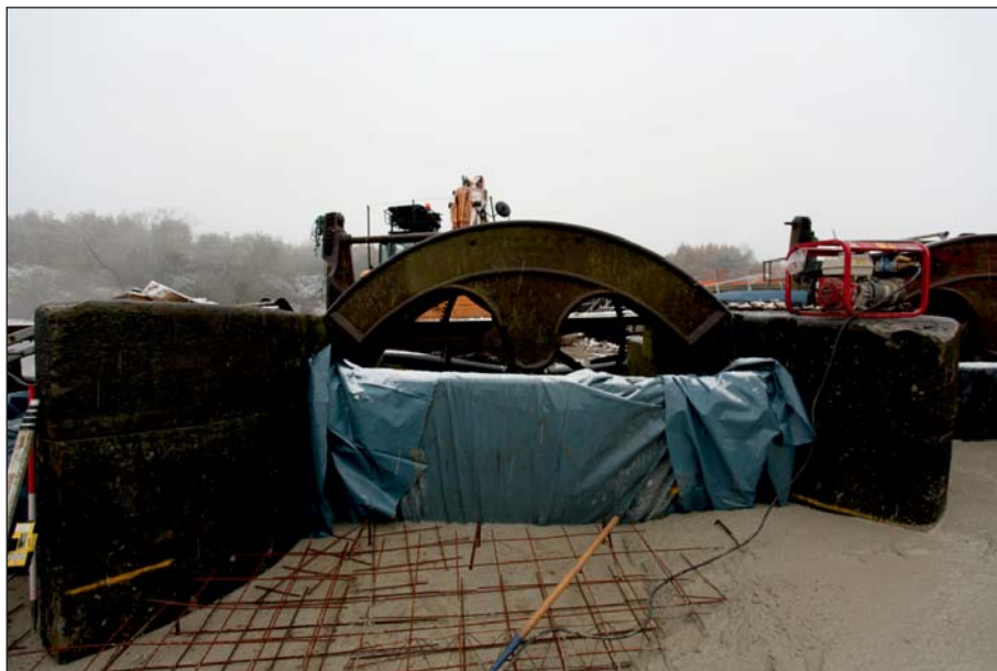
Plate 50: General view of sluices from upstream (Digital IMG_0212)
