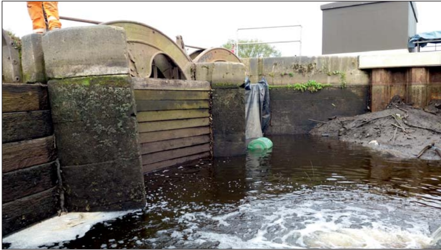
Plate 37: View of the sluices from upstream post-piling (Client Digital 37)
