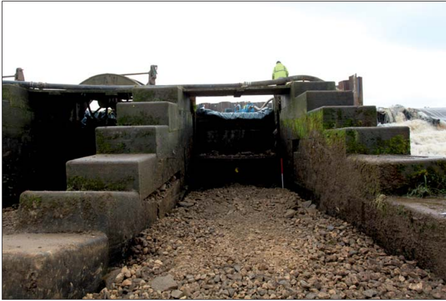
Plate 65: Detail view of the downstream westernmost sluice (Digital IMG_0231)
