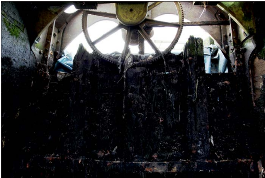
Plate 64: Detail view of the downstream central sluice (Digital IMG_0255)
