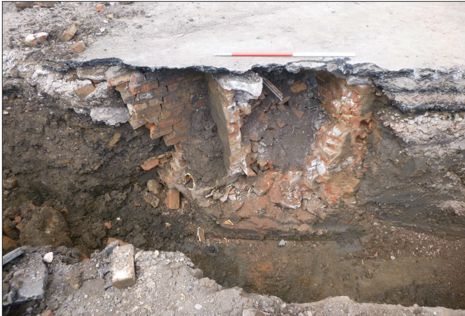
Plate 8: Trench 17, drainage structure 1710
