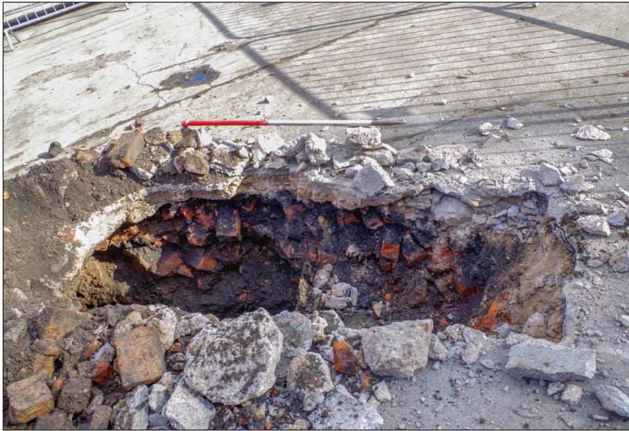
Plate 1: Test pit 1, concrete foundation and modern brick floor
