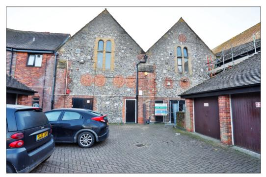
Plate 4: West elevation of north buildings showing flint walls, lancet windows and brick oculus
