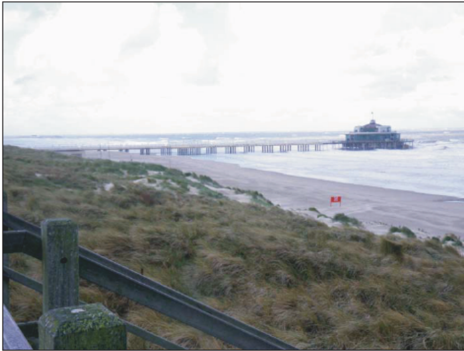
Plate 9: Blankenberge pier – photo taken from top of dunes
