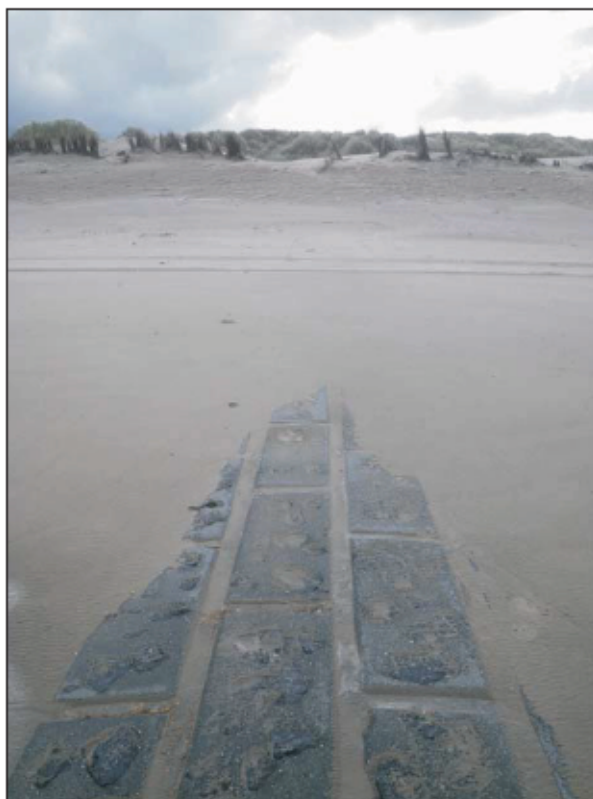
Plate 16: Example of a modern breakwater dating from the 1960's, near Blankenberge, facing dyke/dune systems
