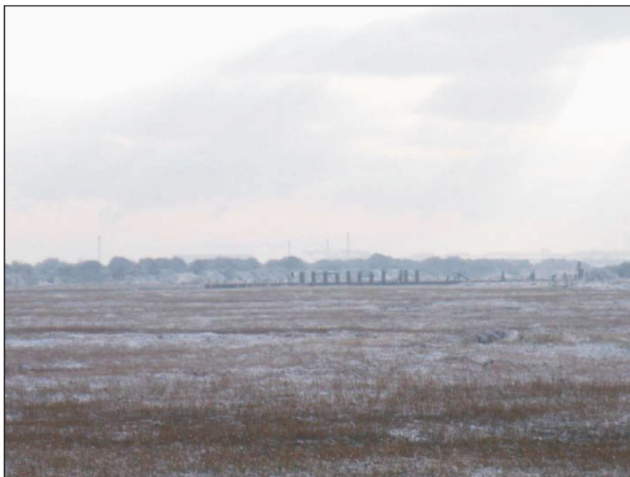
Plate 8: Remains of WWI train ferry (WA1043), photo taken facing south across intertidal area
