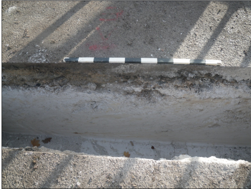
Plate 1: Representative section of the trench, 1m scale, looking east
