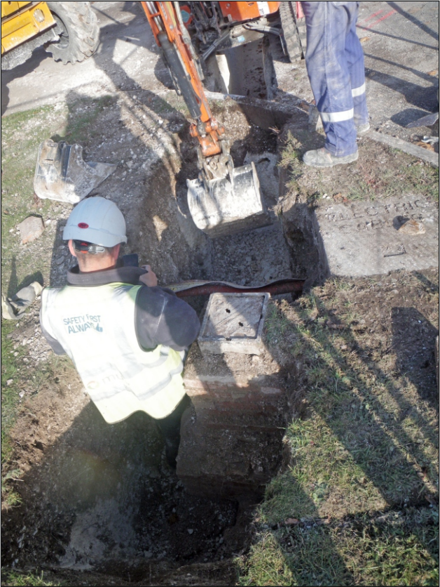
Plate 4: Southern end of the pipe trench, showing disturbance, looking south
