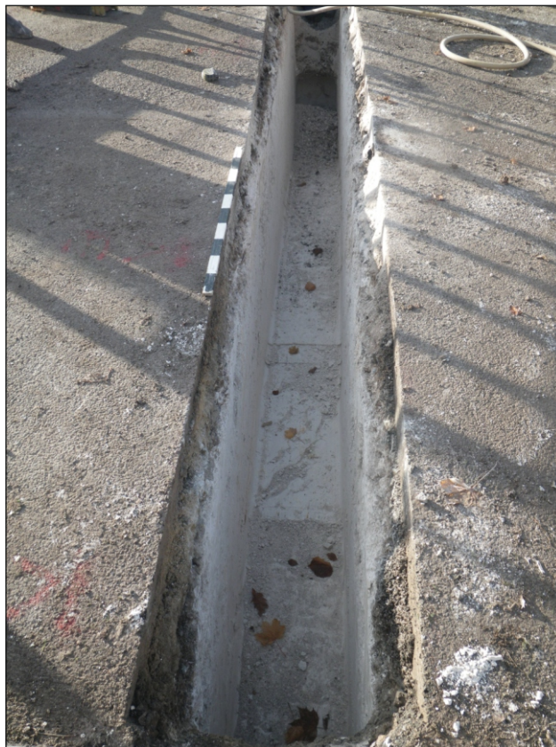
Plate 2: General shot of the pipe trench, 1m scale, looking north
