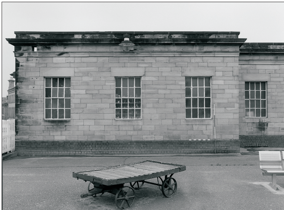
Plate 9: General view of west elevation of Building 2, north end (film 1.1)
