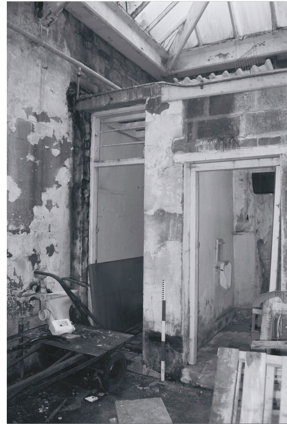
Plate 24: View of former toilet cubicles, north-west corner of G1, Building 1 (film 7.34)
