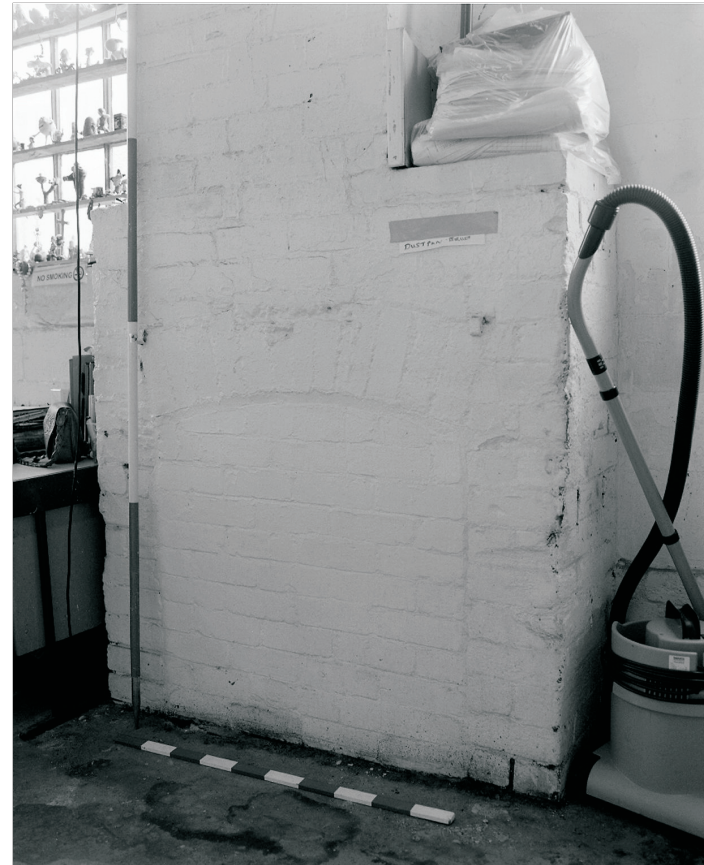
Plate 39: Detail of blocked fireplace, west wall of G5, Building 2 (film 3.7)
