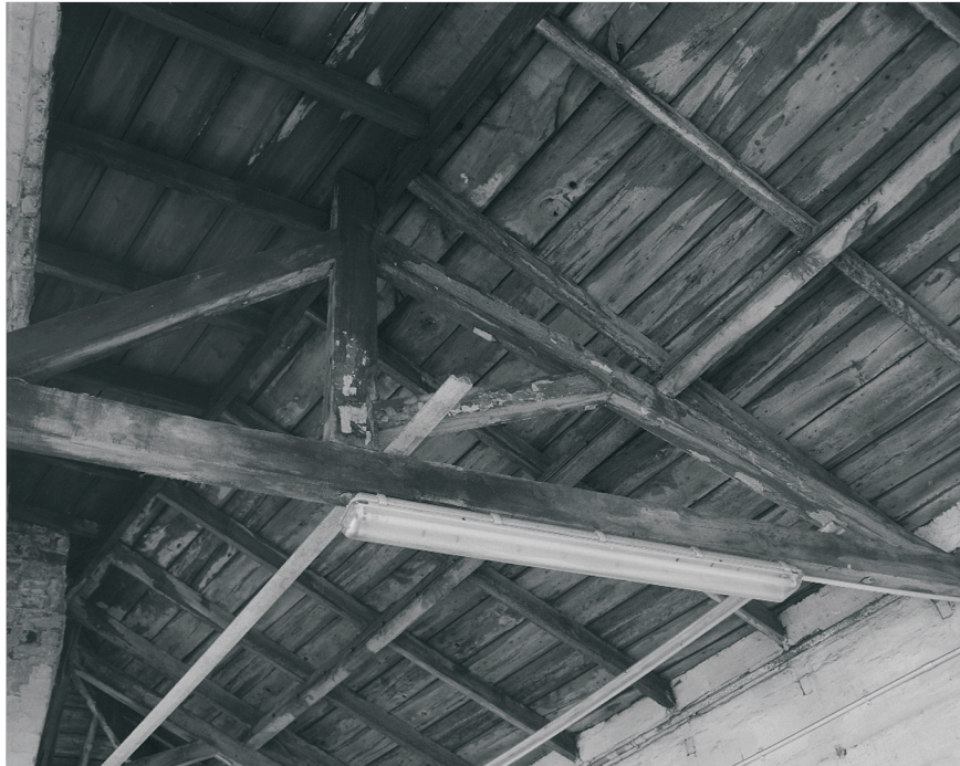
Plate 40: Detail of timber truss, G5, Building 2 (Film 3.10)
