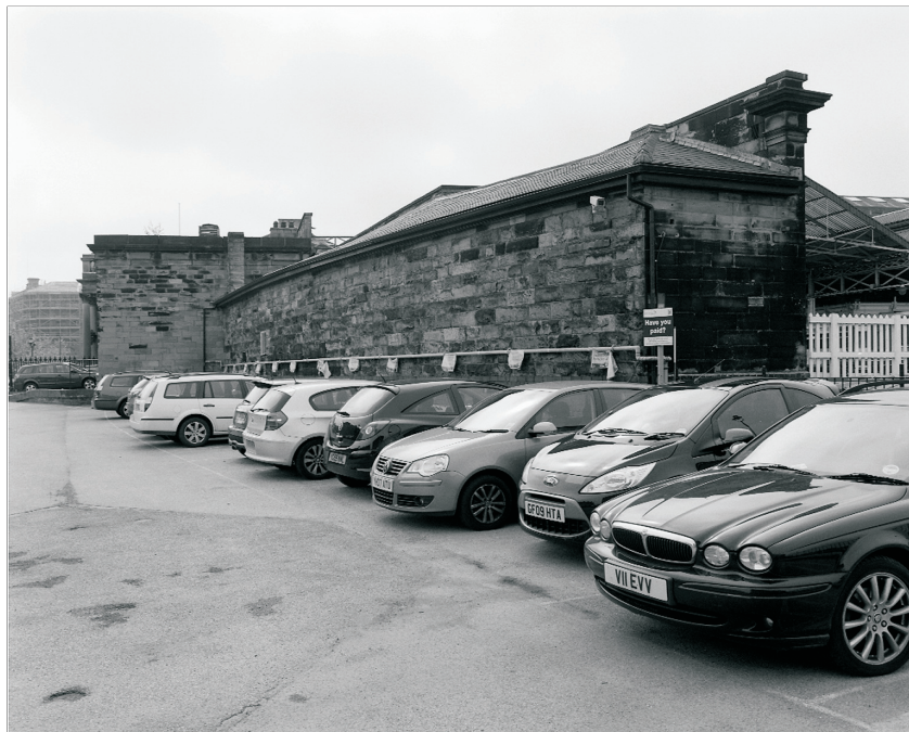
Plate 17: View of north and east elevations of Building 2 (film 5.1)
