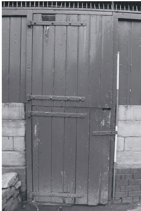
Plate 16: Detail of dutch door to G2, west elevation of Building 2 (film 7.25)
