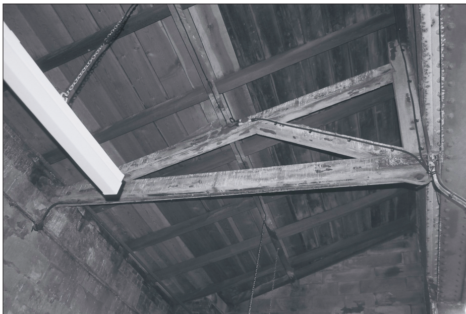
Plate 33: Detail of timber truss, G2, Building 2 (film 7.22)
