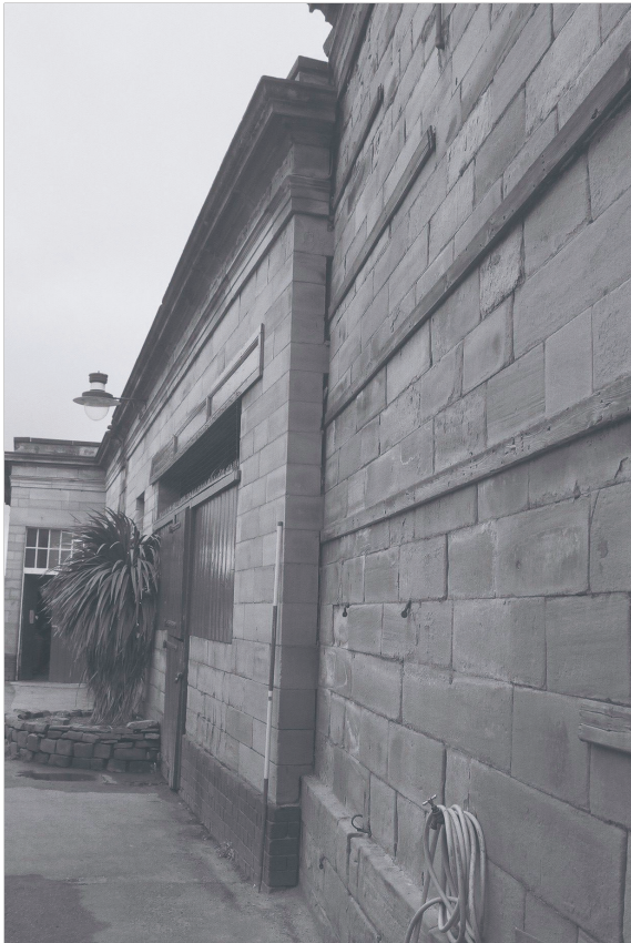
Plate 12: Detail of join in west elevation between Buildings 1 and 2 (film 7.27)
