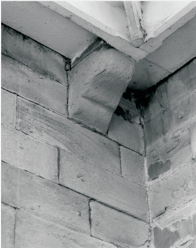
Plate 27: Detail of stone corbel supporting roof guttering, G1, Building 1 (film 6.10)
