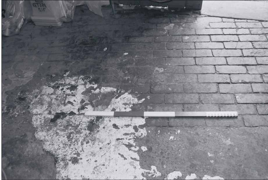
Plate 42: Detail of brick and concrete flooring, G5, Building 2 (film 7.12)
