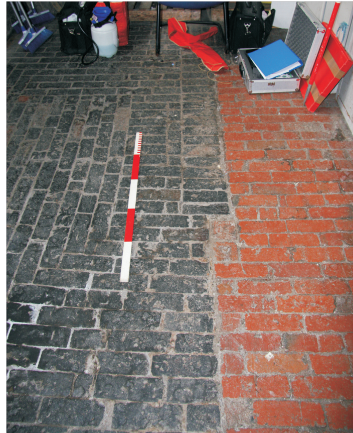
Plate 32: Detail of brick flooring in G2, Building 2 (film 8.9)
