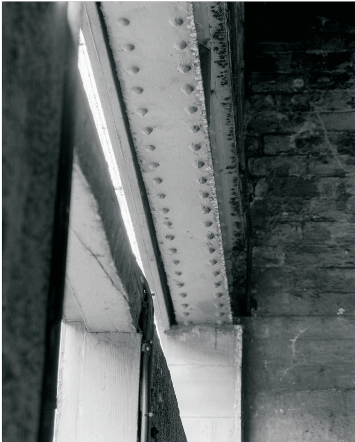
Plate 31: Detail of riveted I-section lintel, west wall of G2, Building 2 (film 2.5)
