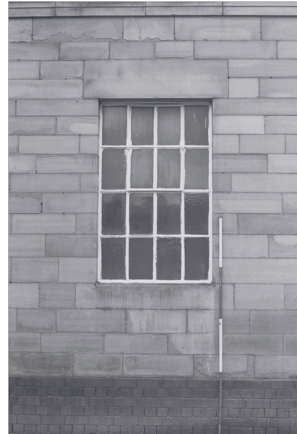
Plate 13: Detail of multi-paned metal framed window, west elevation of Building 2 (film 7.15)
