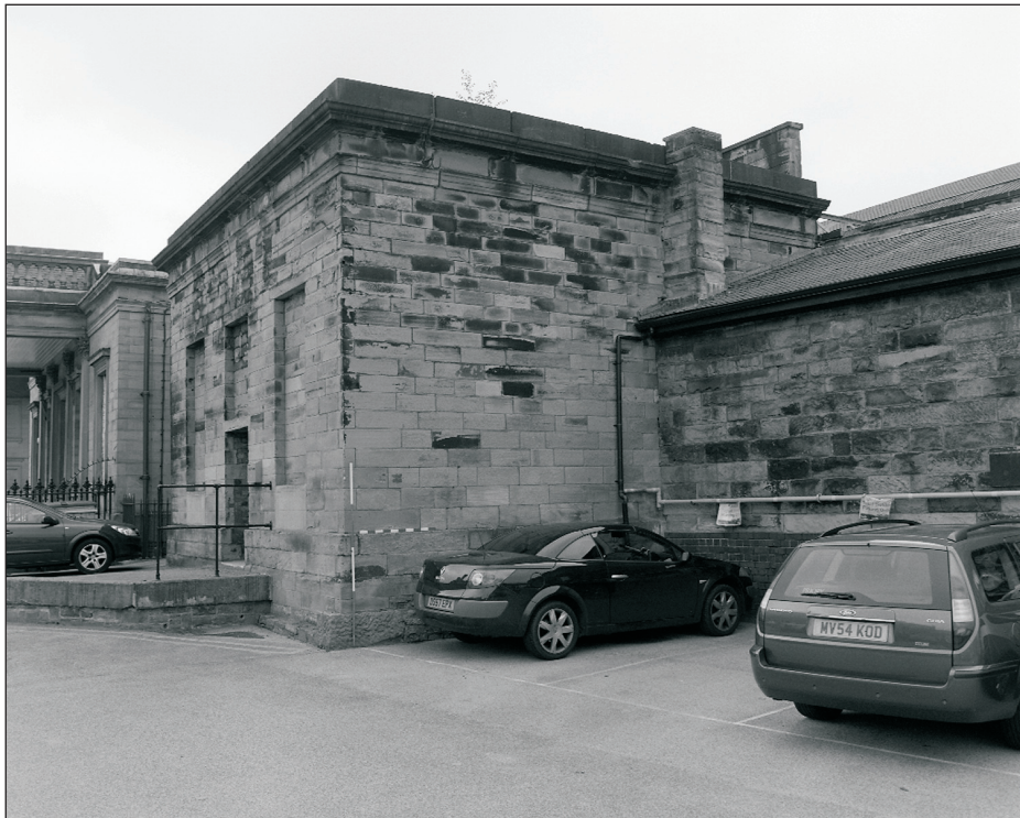
Plate 7: General view of north elevation of Building 1, showing added chimney stack (film 4.5)
