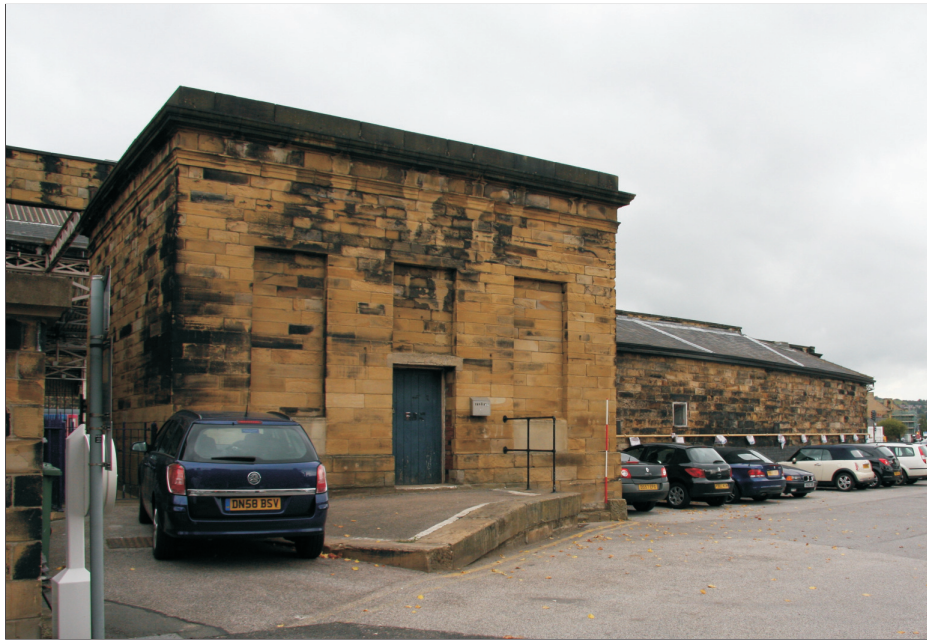
Plate 1: General view of east elevation of Buildings 1 and 2 (film 8.1)
