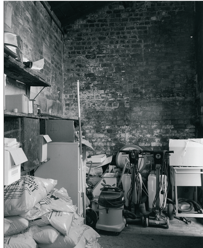
Plate 35: General view of G4, Building 2 (film 2.10)
