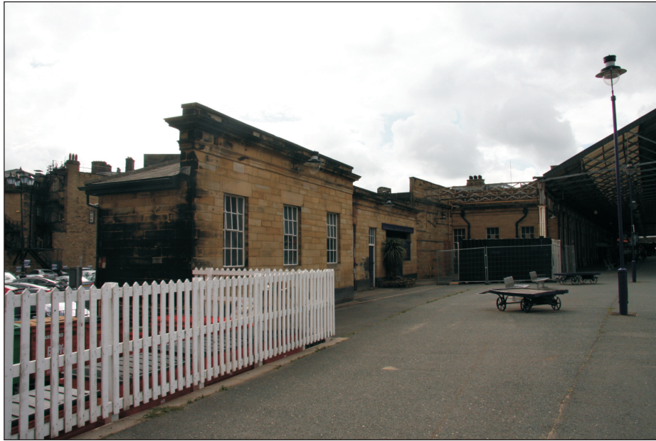
Plate 8: General view of west elevation of Building 2, fronting platform 1 (film 8.3)
