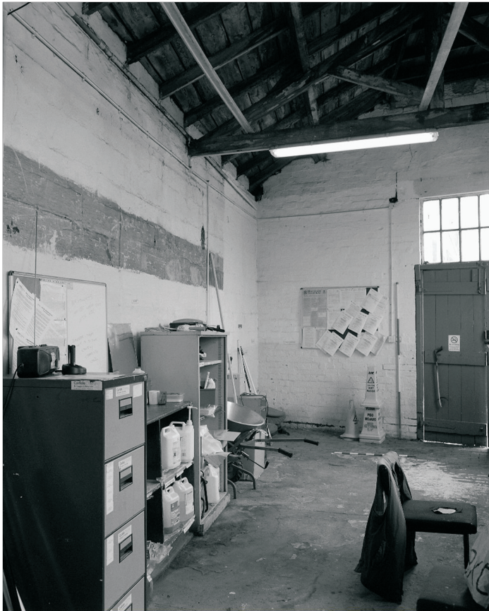
Plate 38: General view of G5, Building 2 (film 3.5)
