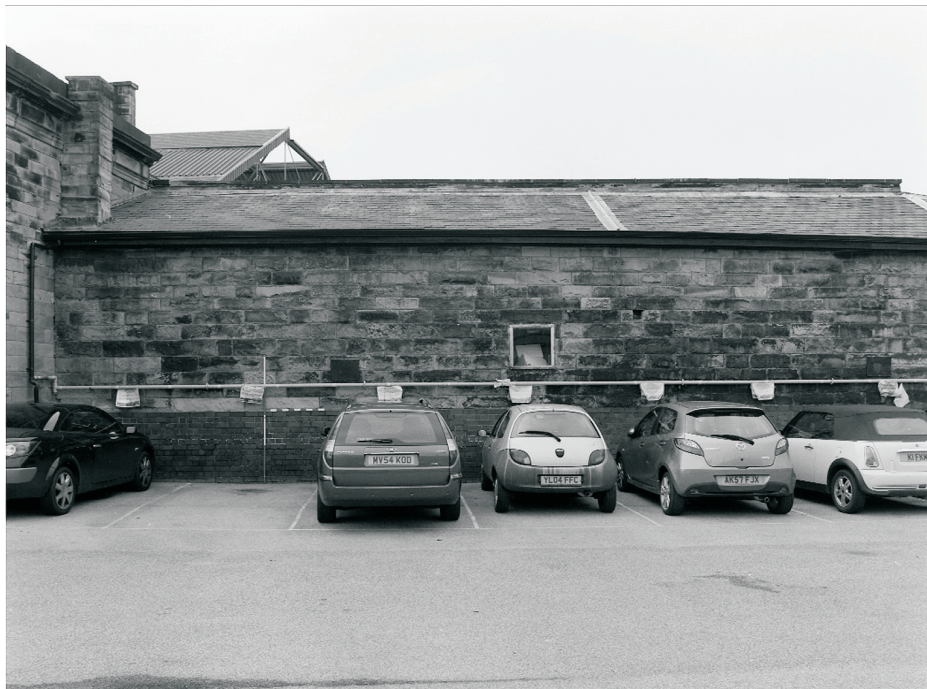
Plate 19: General view of the south end of the east elevation of Building 2, note inserted window (film 4.7)
