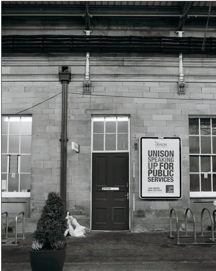
Plate 21: View of primary doors and windows, west elevation of South Wing (film 2.10)
