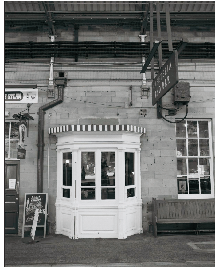
Plate 14: View of added bay window, south end of South Wing, west elevation (film 1.10)
