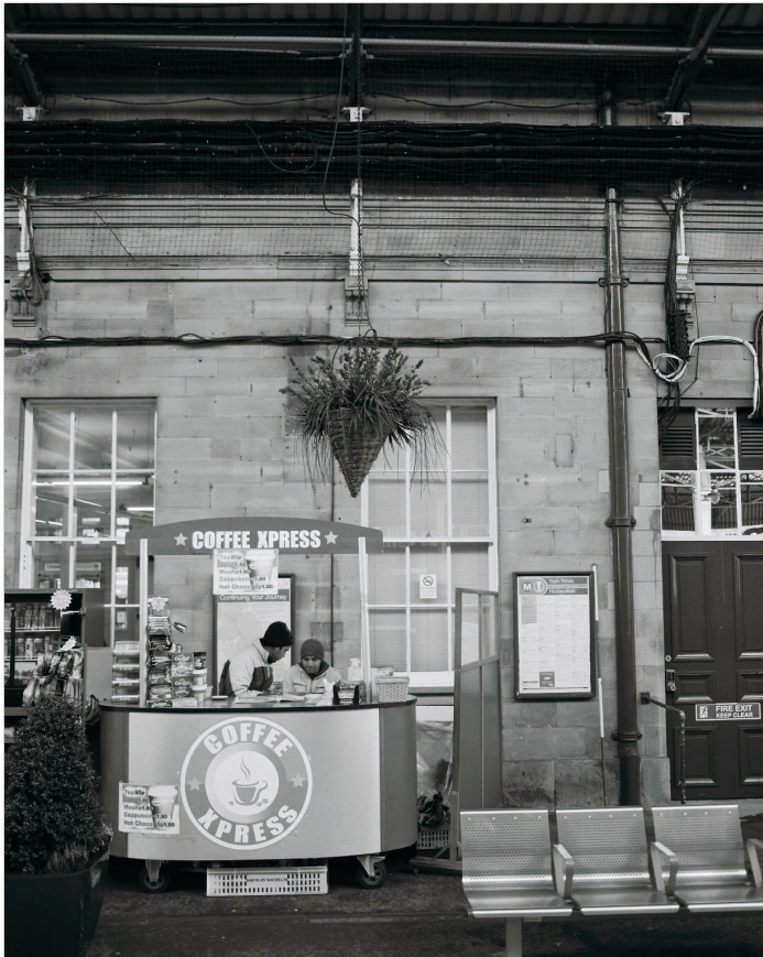
Plate 27: View of windows and door, west elevation of Central Block (film 3.6)
