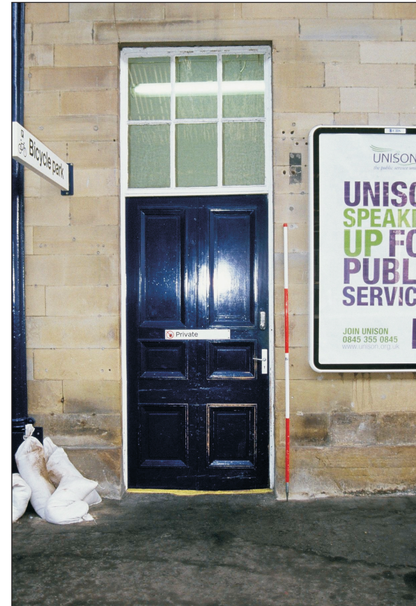
Plate 22: Detail of primary door, west elevation of South Wing (film 7.7)
