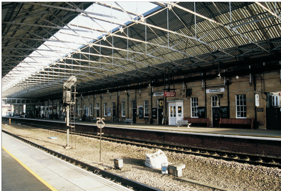
Plate 2: General view of west elevation of Booking Hall from south-west (film 7.2)
