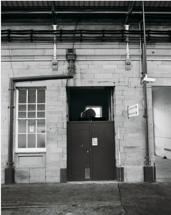
Plate 37: View of altered opening, west elevation of North Wing (film 4.10)
