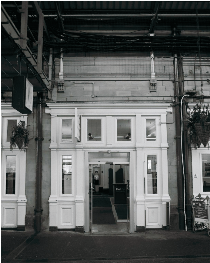
Plate 29: View of central double door main entrance from Booking Hall to platforms, west elevation of Central Block (film 3.10)
