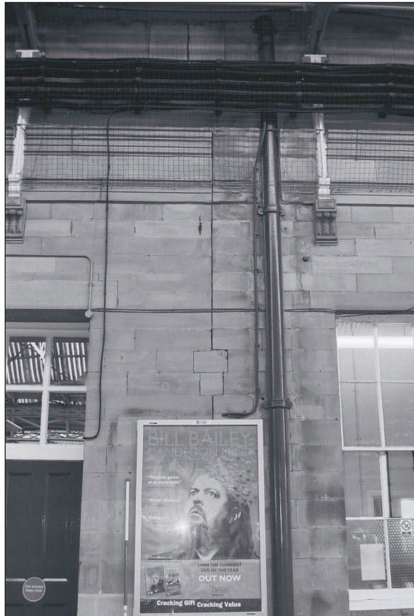
Plate 25: Detail of vertical joint in stonework delineating join between Central Block and South Wing (film 6.18)
