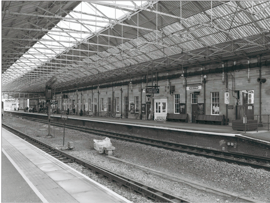
Plate 1: General view of west elevation of Booking Hall from south-west (film 5.8)
