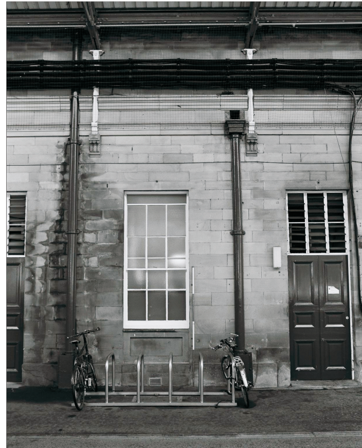
Plate 16: View of door and window, west elevation of South Wing (film 2.3)
