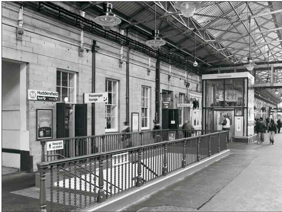
Plate 9: General view of west elevation of Booking Hall from north (film 5.2)
