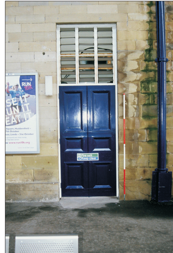
Plate 18: Detail of primary door with louvered over-light, west elevation of South Wing (film 7.6)
