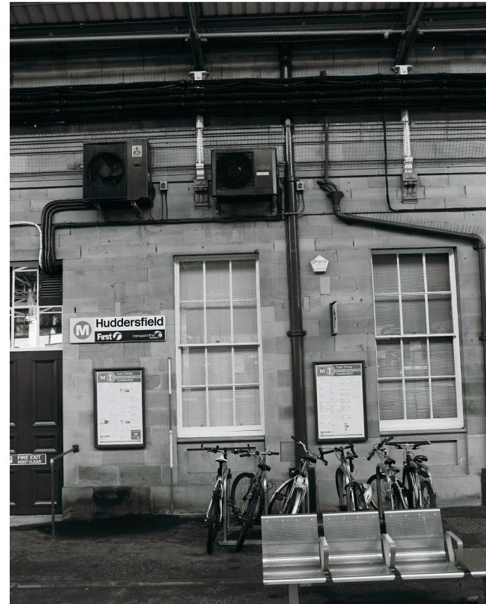
Plate 26: View of altered doors to windows, west elevation of Central Block (film 3.3)
