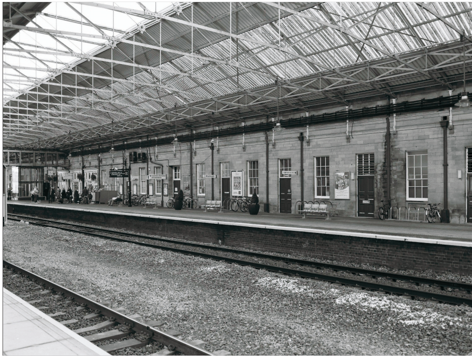
Plate 3: General view of west elevation of Booking Hall from south-west (film 5.6)
