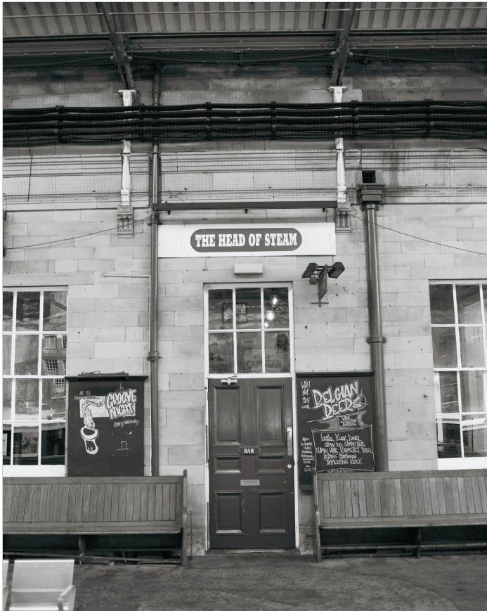
Plate 13: View of doorway to pub at south end of South Wing, west elevation (film 1.8)
