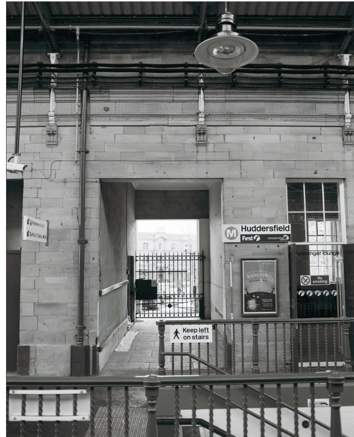
Plate 36: View of inserted passageway, west elevation of North Wing (film 4.8)
