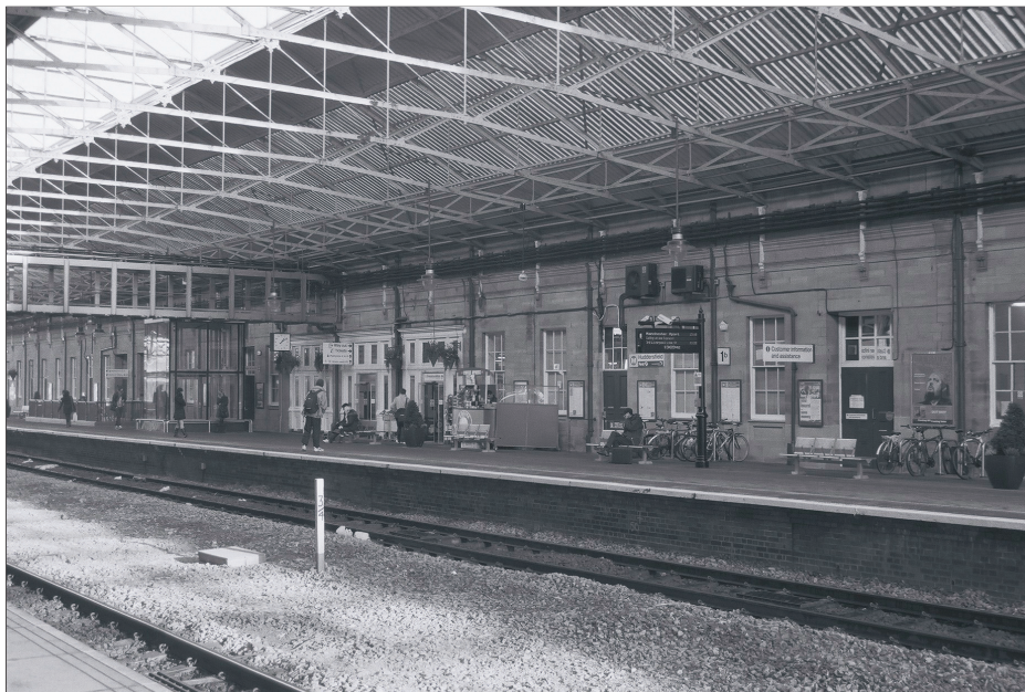
Plate 4: General view of west elevation of Booking Hall from south-west (film 6.10)
