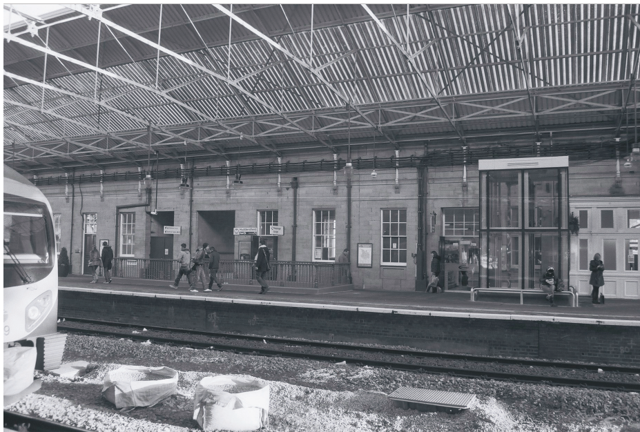
Plate 8: General view of west elevation of Booking Hall from west (film 6.4)
