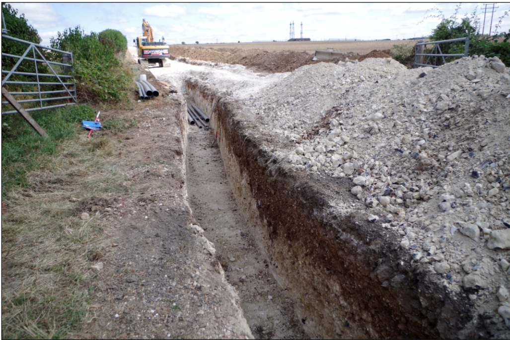
Plate 2: General view of cable trench
