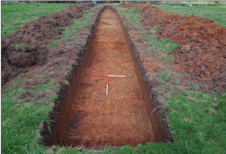
Plate 2: Trench 2 looking north-east
