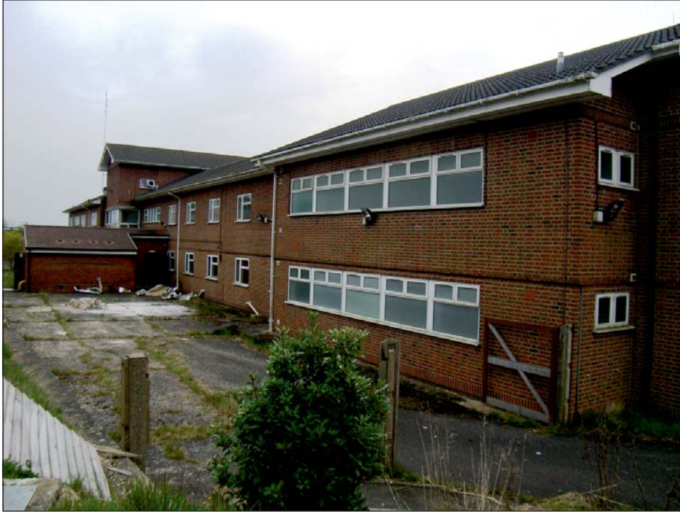
Plate 5: Building 7 Sergeants Mess viewed from north-west
