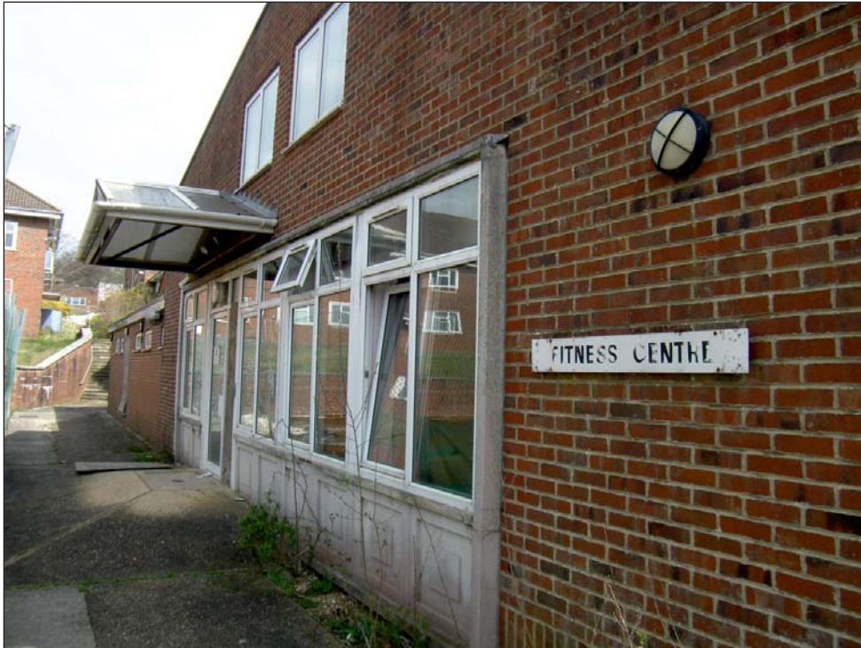
Plate 15: Building 17 Fitness centre west entrance viewed from south
