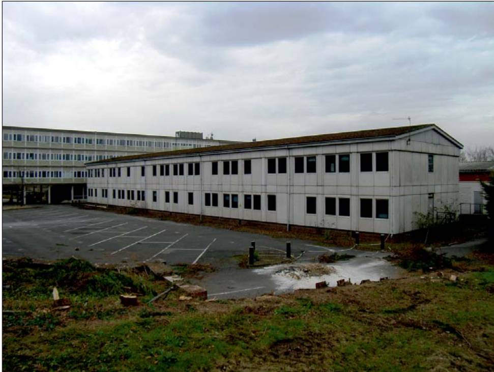
Plate 13: Building 16 Headquarters centre extension viewed from north
