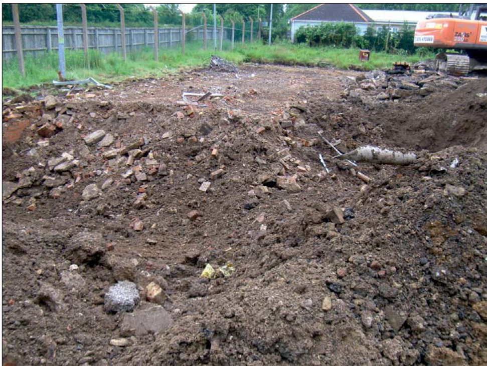
Plate 22: Removal of drainage in area of gatehouse building showing made ground
