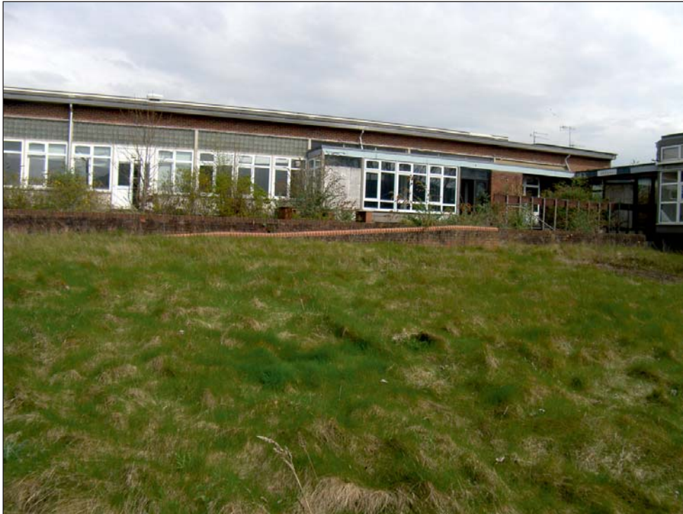
Plate 17: Building 17 Fitness centre south elevation
