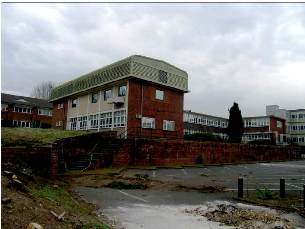
Plate 12: Building 16 Headquarters north extensions viewed from south-west
