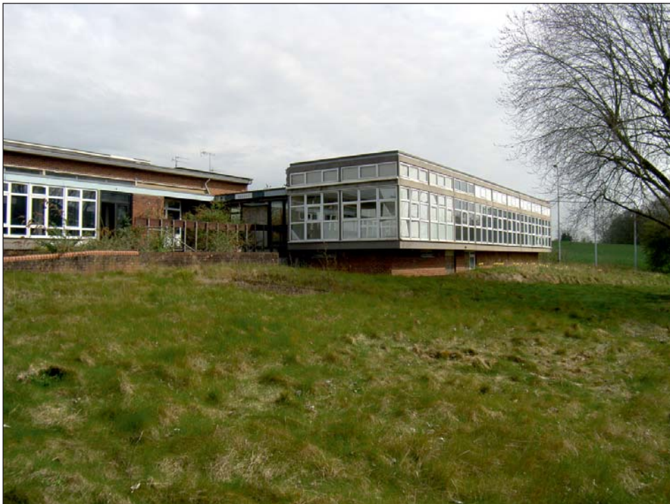
Plate 16: Building 17 Fitness centre viewed from south-west
