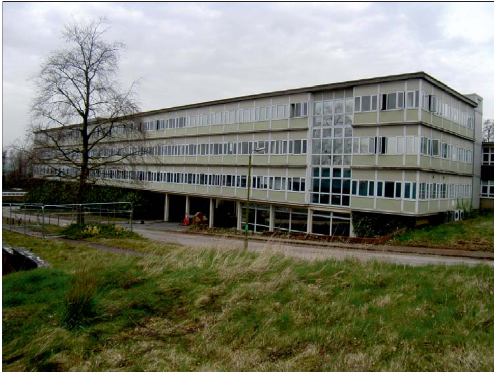
Plate 11: Building 16 Headquarters viewed from east
