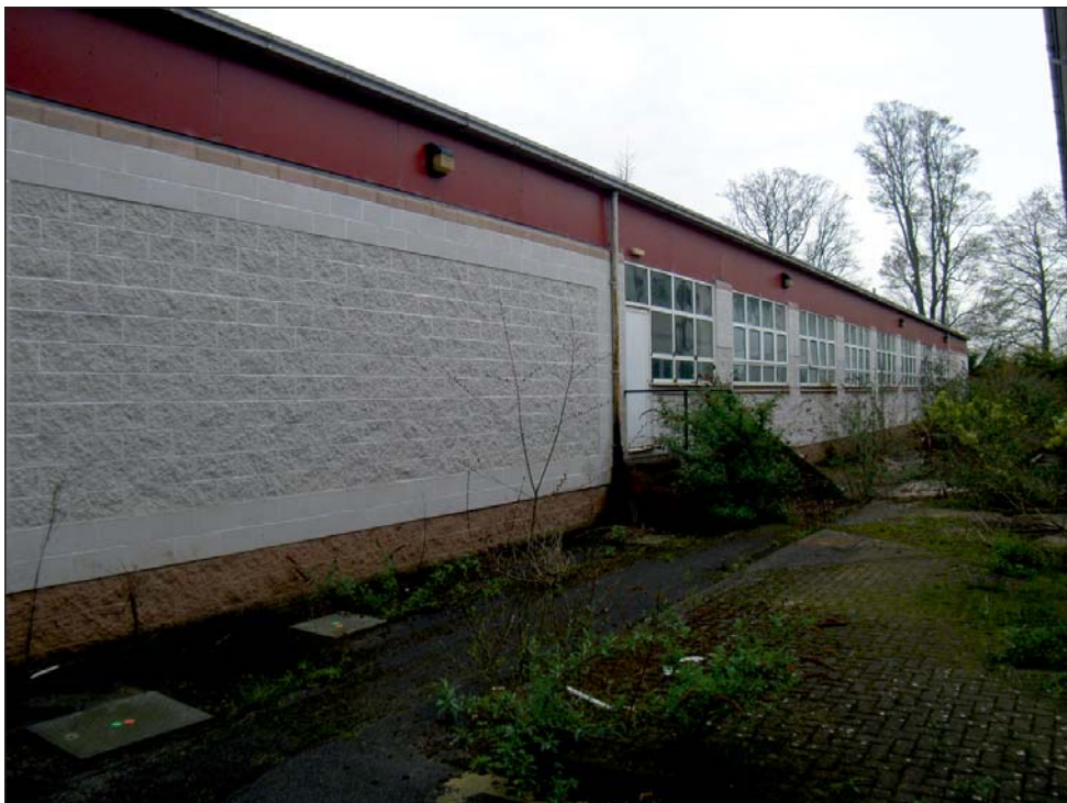
Plate 14: Building 16 Headquarters south extension viewed from east
