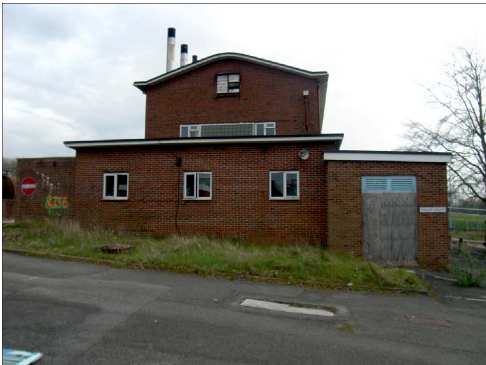
Plate 8: Building 10 Boiler house viewed from west
