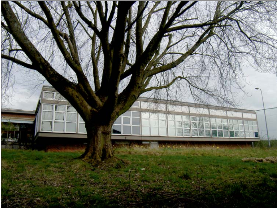
Plate 1: Building 7 Sergeants Mess viewed from south-east
