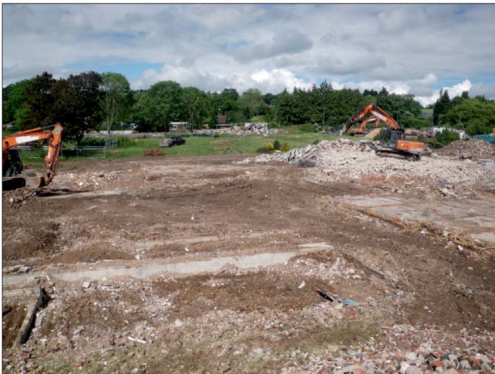
Plate 24: View to west showing demolition of southernmost building and associated surfaces
