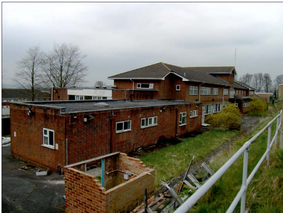
Plate 4: Building 7 Sergeants Mess viewed from east
