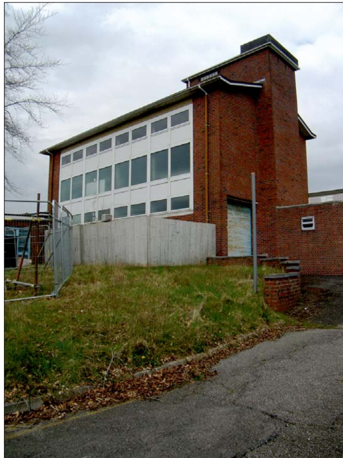
Plate 6: Building 10 Boiler house viewed from south
