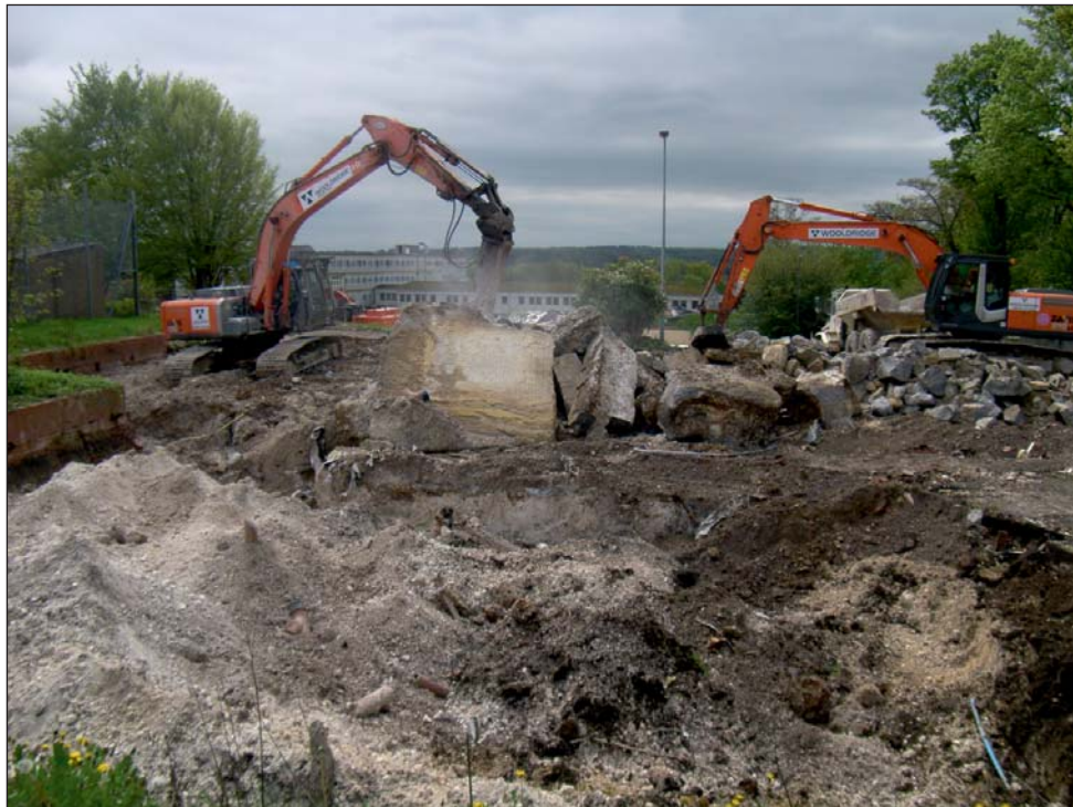
Plate 20: Deep excavation of substantial foundations of building 73
