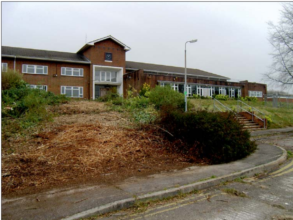
Plate 2: Building 7 Sergeants Mess viewed form south-west
