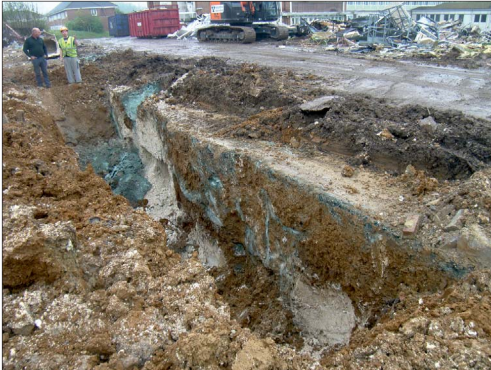
Plate 21: Deep excavation following removal of substantial foundation of building 56
