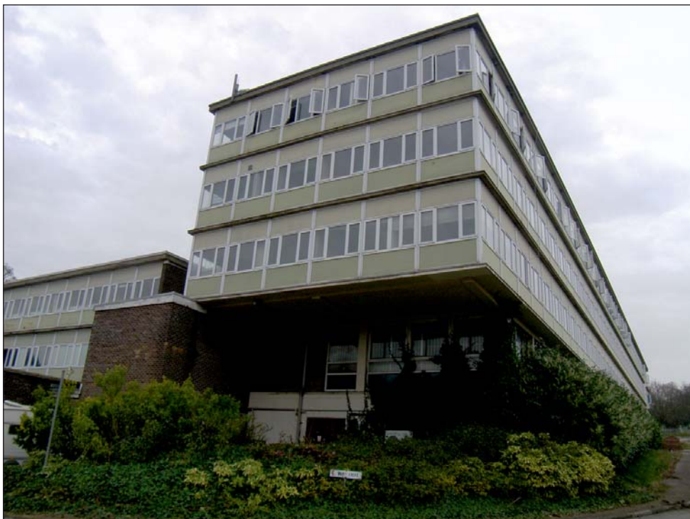
Plate 10: Building 16 Headquarters viewed from south
