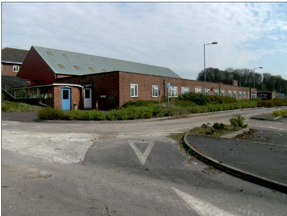
Plate 18: Building 27 Arnham block
