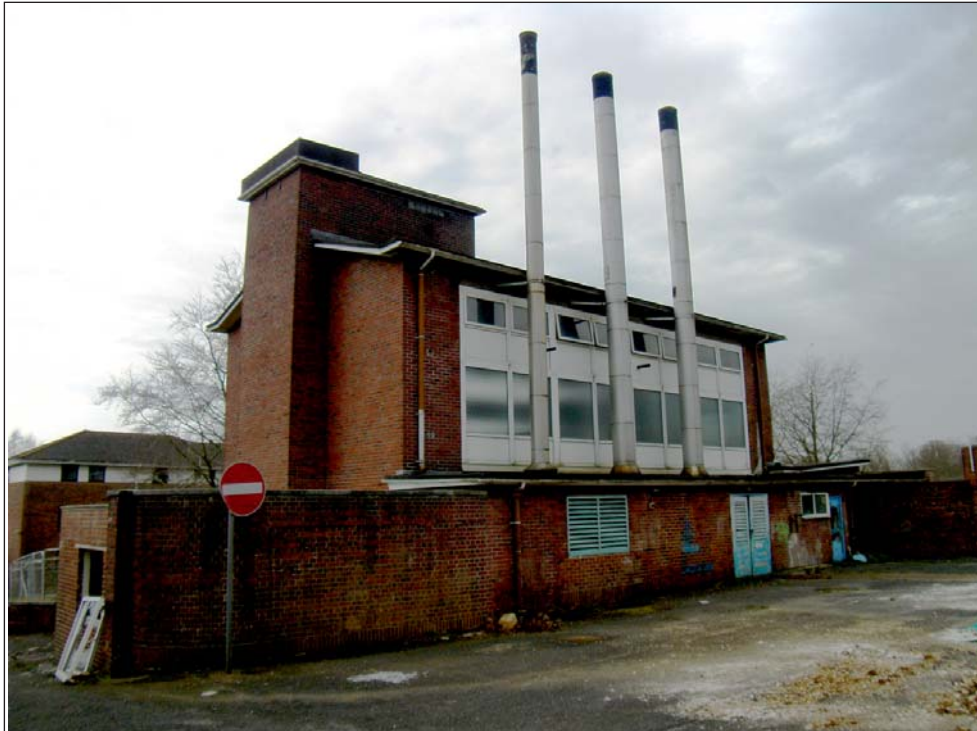
Plate 7: Building 10 Boiler house viewed from east
