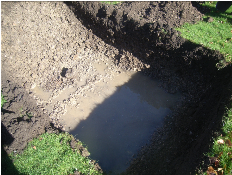
Plate 2: Machine excavation of Trench 2A taken from the south west
