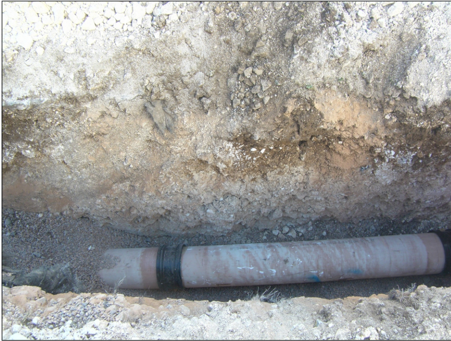
Plate 1: South-west facing section of the main Larkhill WWTW compound. Scale is 1 m
