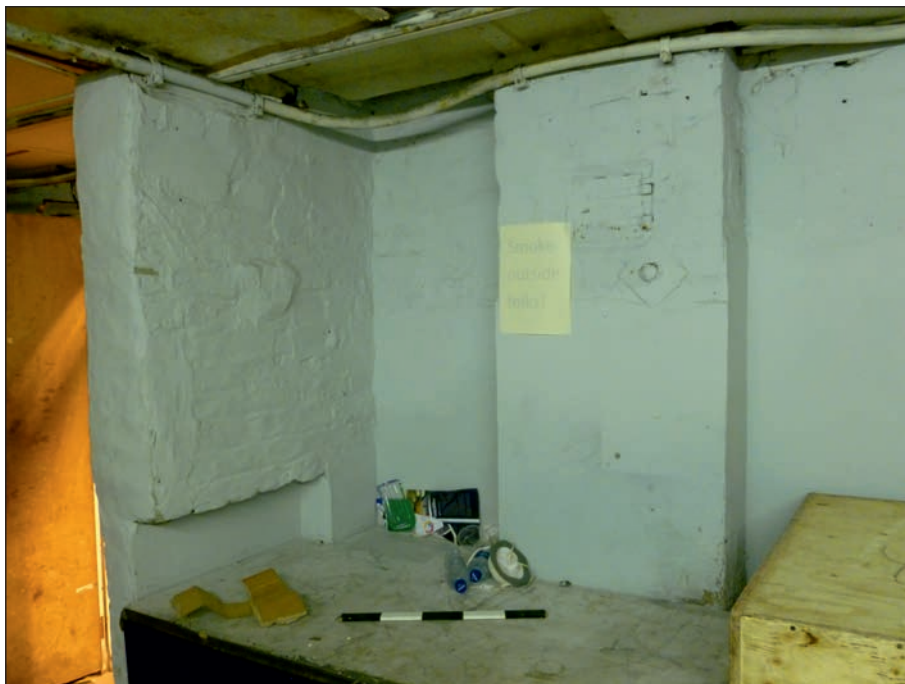
Plate 62: View of flue and truncated partition wall in Room 4G2
