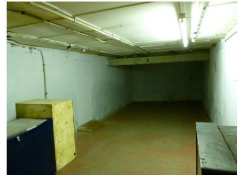
Plate 10 Room 4G2, looking west
