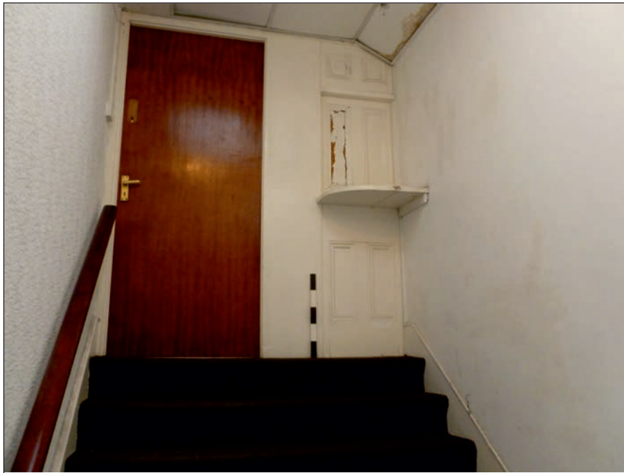
Plate 53: Detail of enquires hatch in Room 2G1 / 2F1
