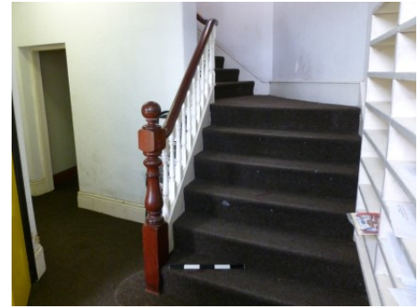
Plate 1 Room 2G1, looking west
