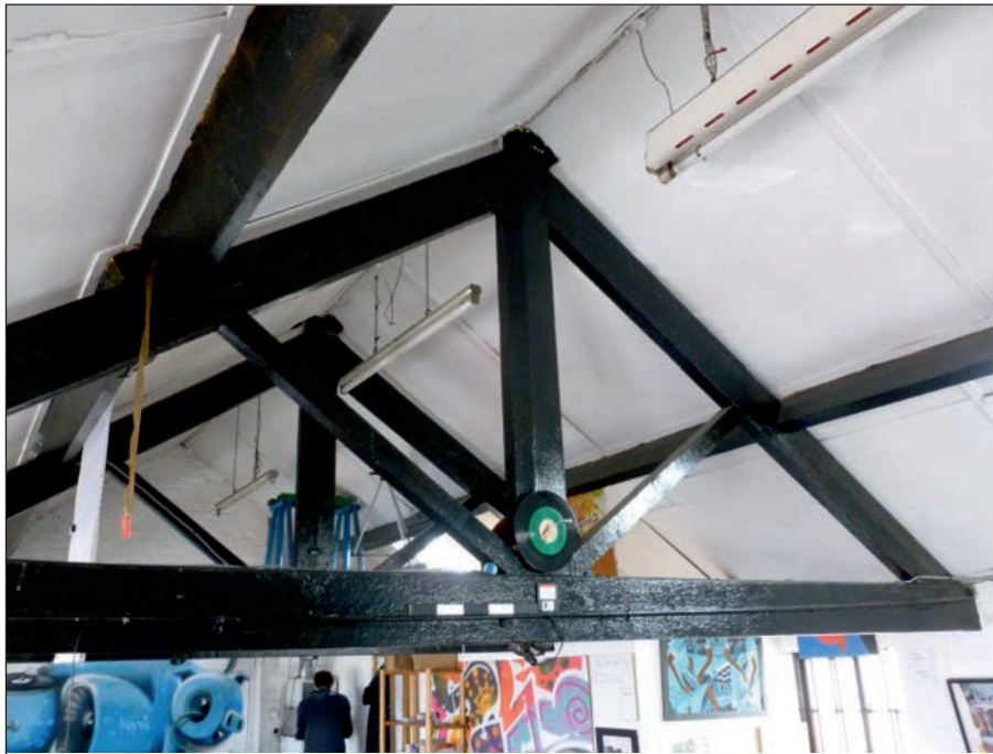
Plate 51: Detail of truss in Room 3S1
