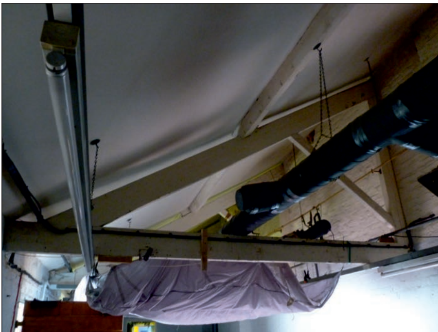
Plate 52: Detail of western truss in Room 4F2
