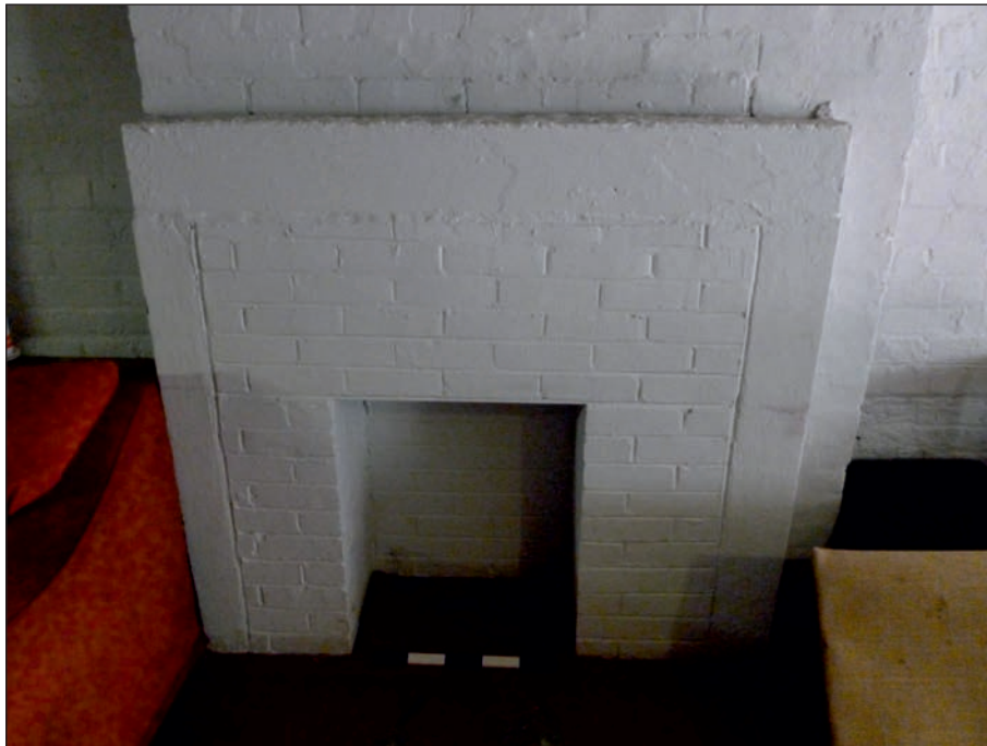
Plate 61: Detail of fireplace in Room 7F6
