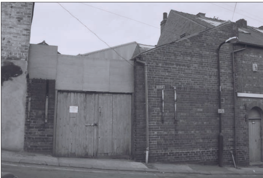
Plate 42: General view of east elevation of Building 10
