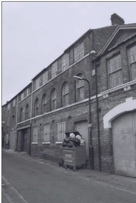
Plate 34: General view of east elevation of Building 3
