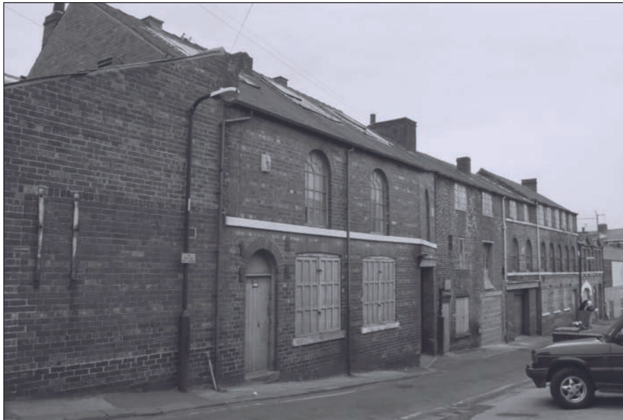
Plate 41: General view of east elevation of Building 9
