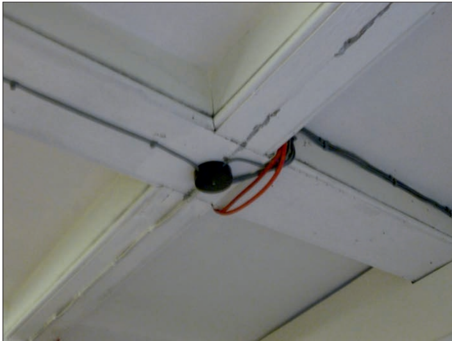
Plate 65: Detail of beaded joist in Room 7F1
