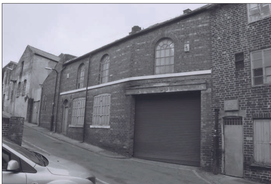
Plate 40: General view of east elevation of Building 9
