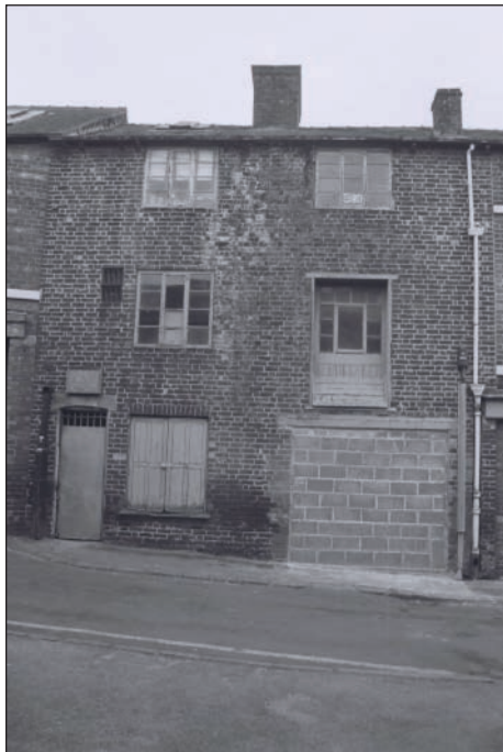
Plate 38: General view of east elevation of Building 7
