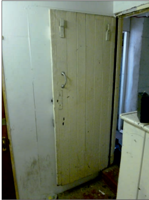
Plate 57: Battened door in Room 7G5
