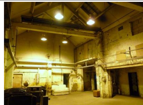
Plate 27 Room 8G1, looking north
