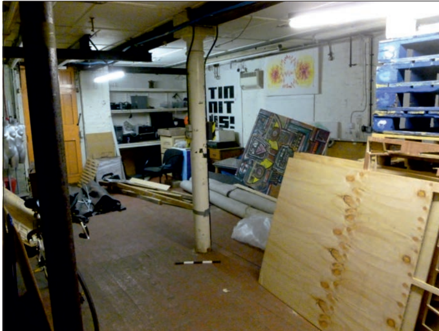
Plate 49: General view of Room 3G1, showing column and floor
