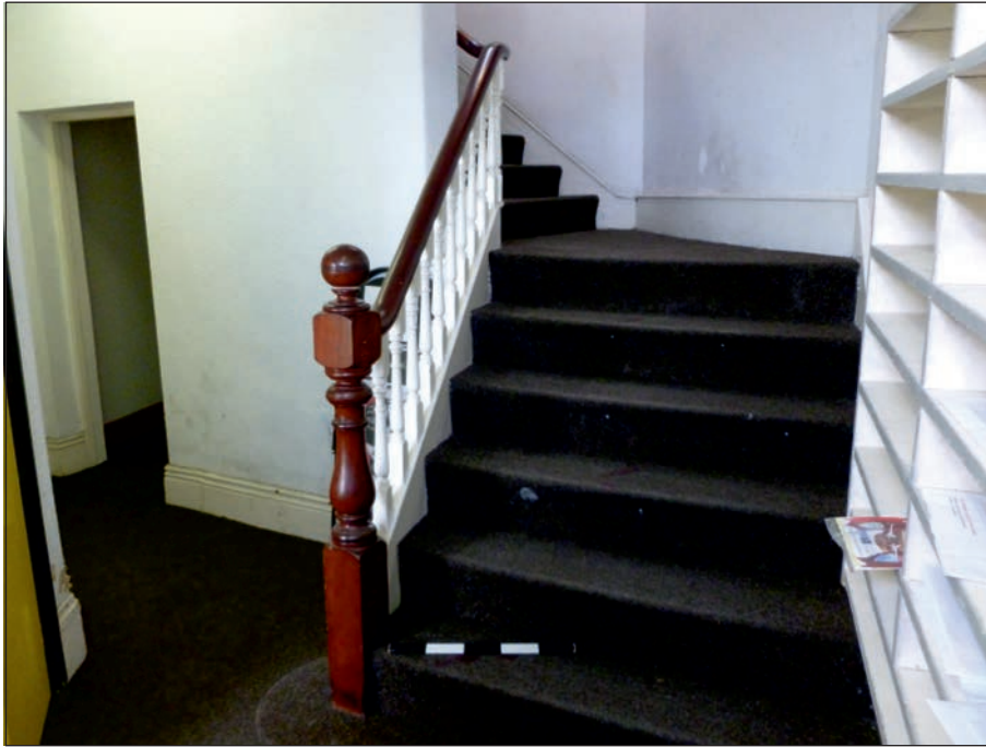
Plate 47: Detail of stairs and banister in Room 2G1
