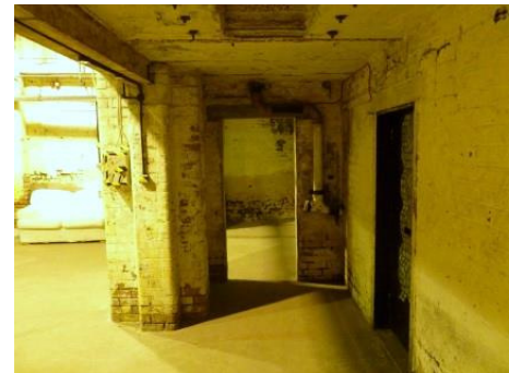
Plate 29 Room 8G3, looking north
