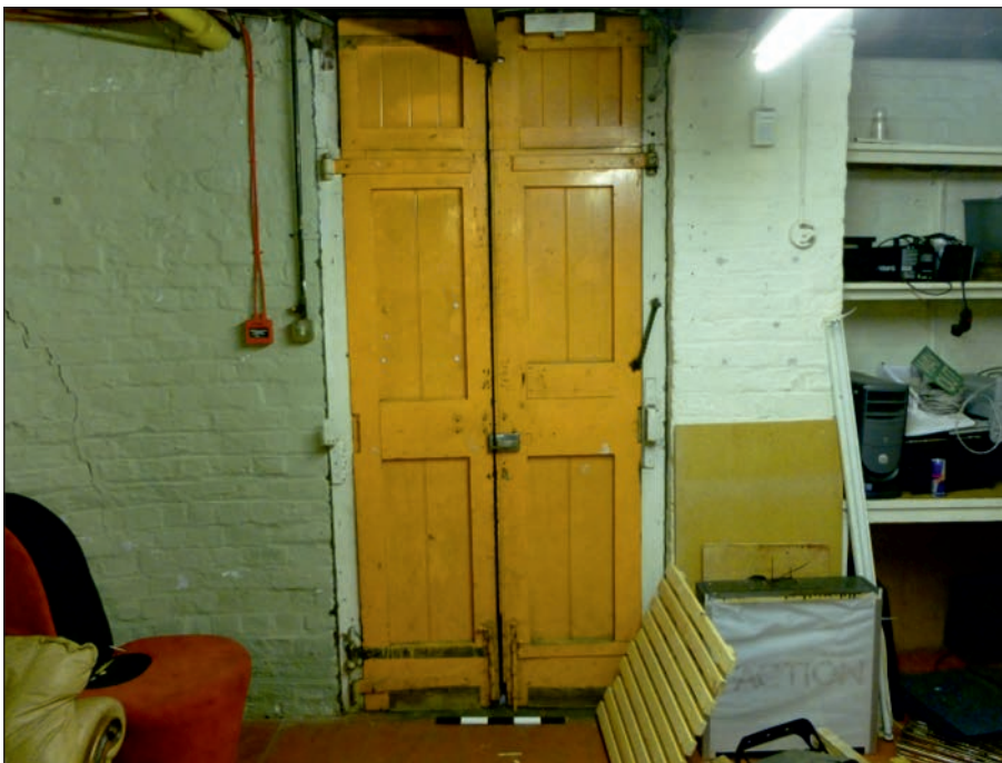
Plate 54: Panelled taking in door in north wall of 3G1
