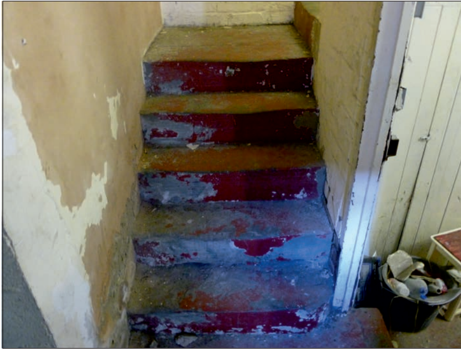
Plate 45: Detail of staircase in south of Room 7G5
