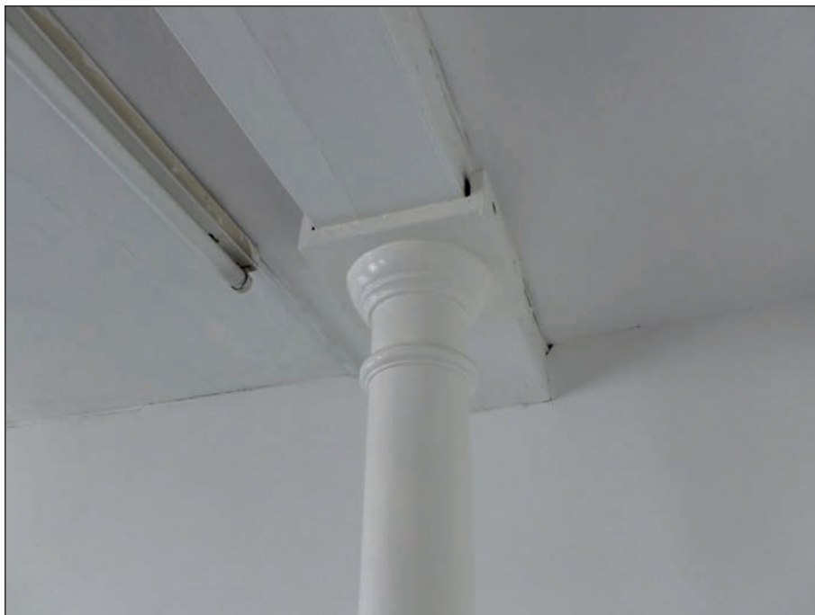
Plate 50: Detail of cast iron column in Room 3F
