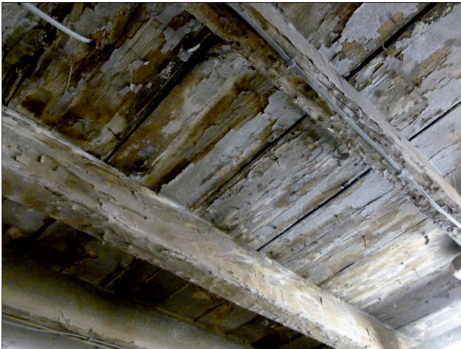
Plate 48: Detail of floor joists and boards in ceiling of Room 7G5
