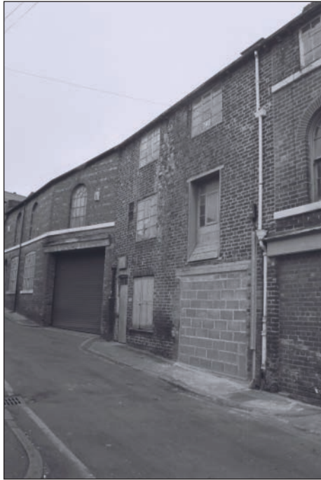
Plate 37: General view of east elevation of Building 7
