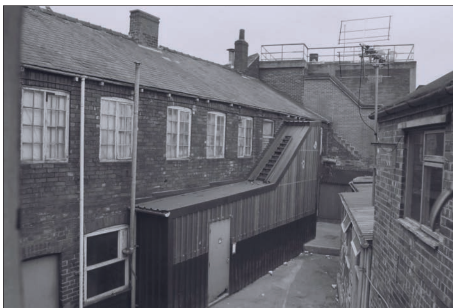
Plate 36: General view of north elevation of Building 4
