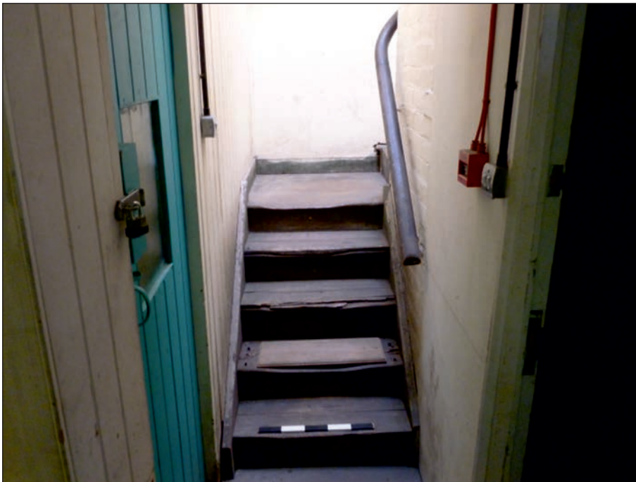
Plate 46: Detail of staircase in south of Room 7F4
