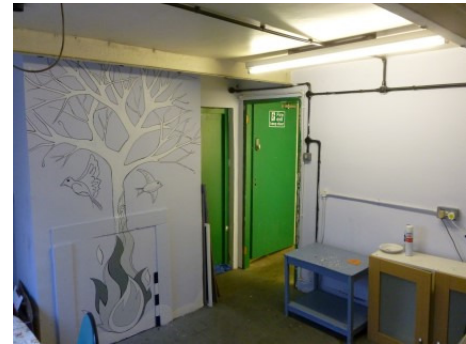
Plate 22 Room 7F6, looking northeast
