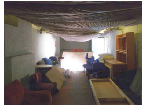
Plate 11 Room 4F1, looking west
