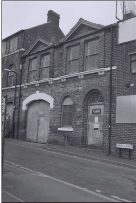
Plate 33: General view of east elevation of Building 2
