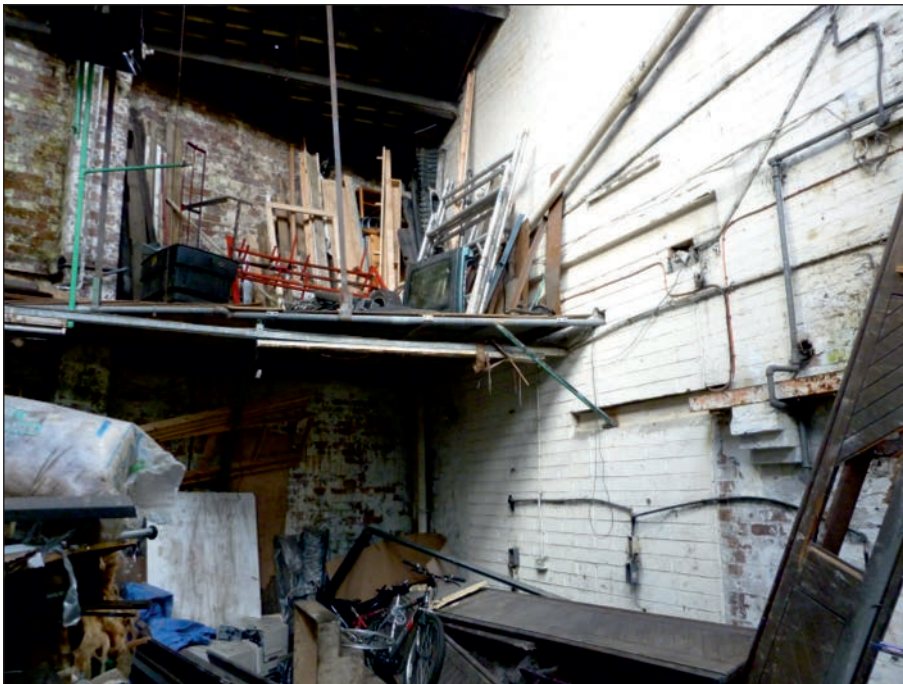
Plate 44: View of NW corner and blocked door in Room 9G1-2
