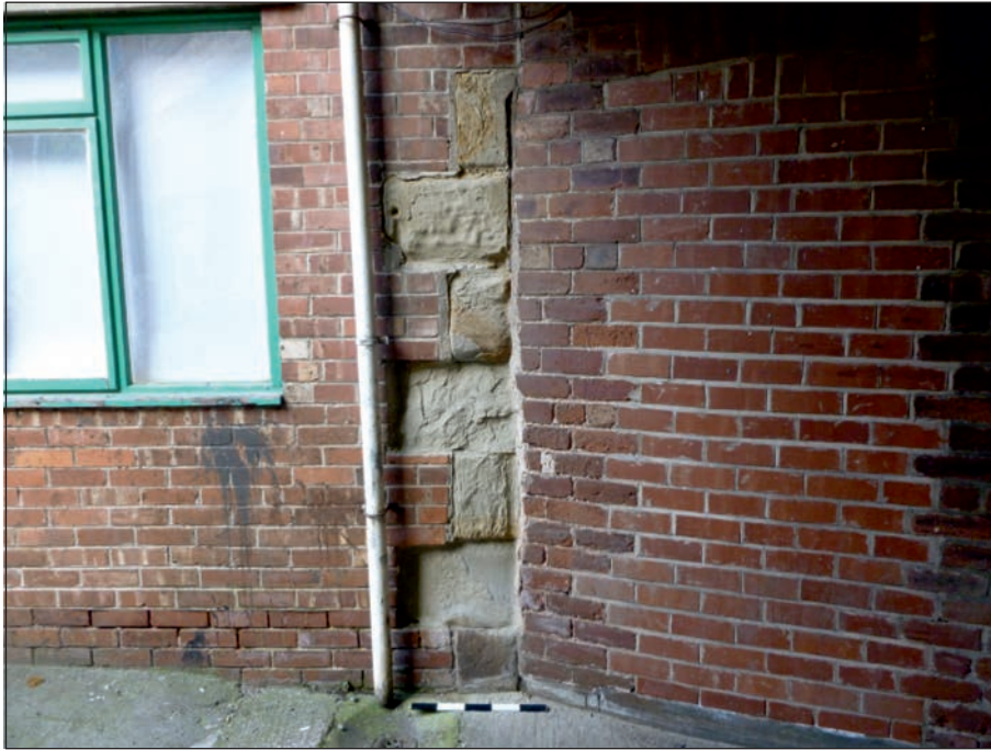
Plate 43: Detail of stone quoins to Building 5
