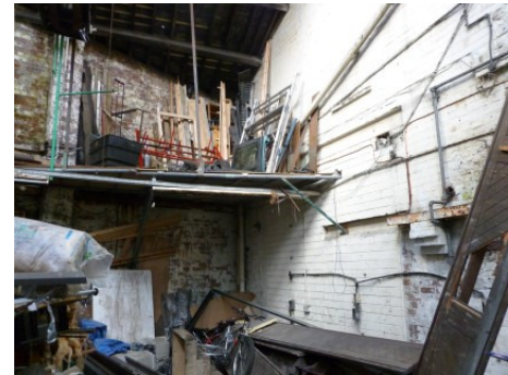
Plate 31 Room 9G1, looking west
