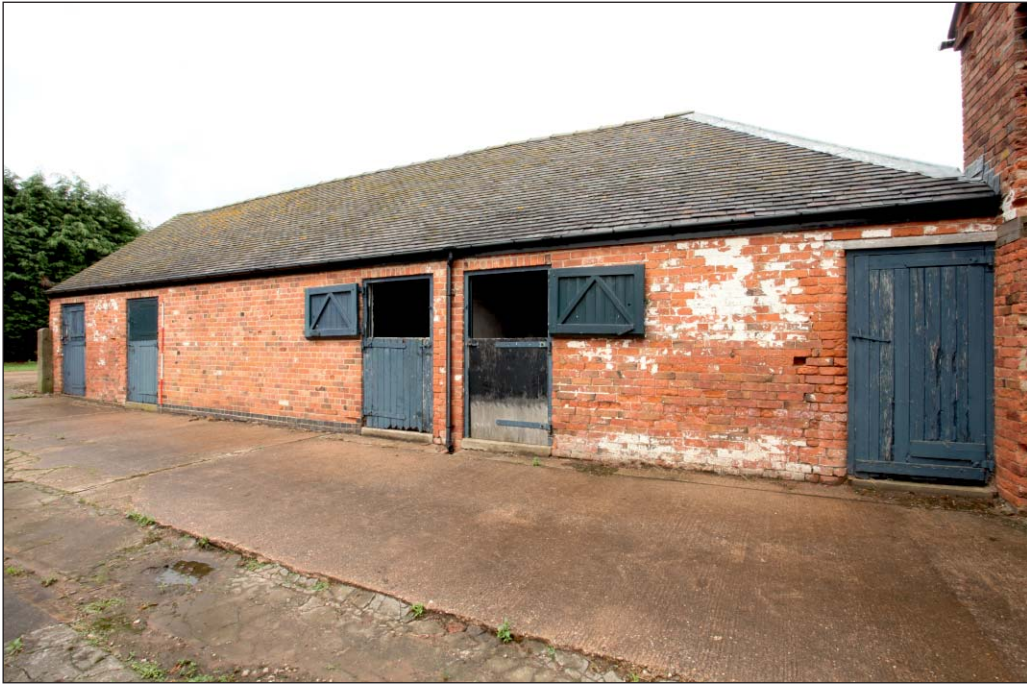
Plate 69: Building 6 viewed from the north-east
