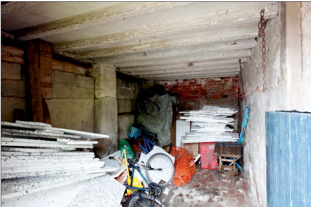
Plate 46: View of G13, Building 2, from the south-west
