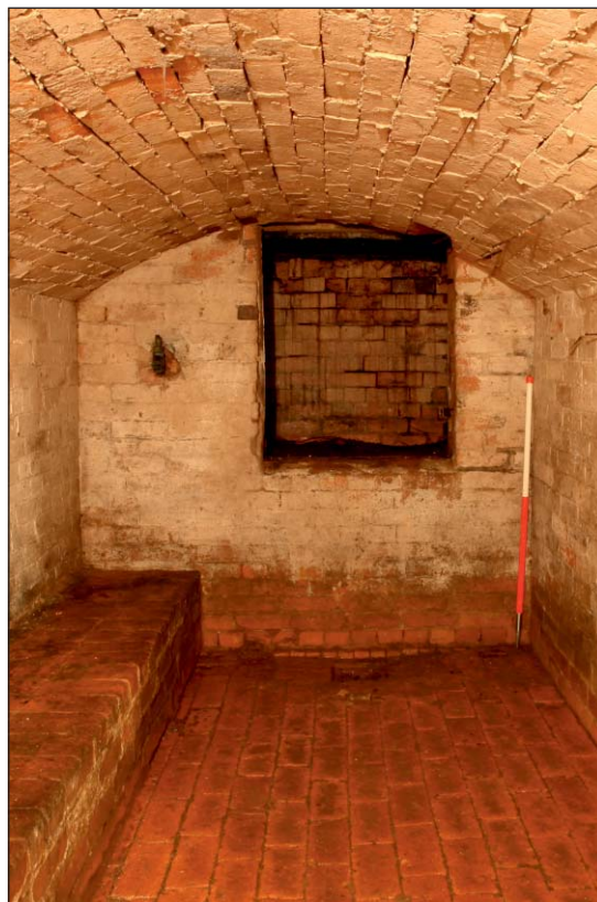
Plate 8: View of the lightwell, drain and tap at the north end of chamber B02, basement of Building 1
