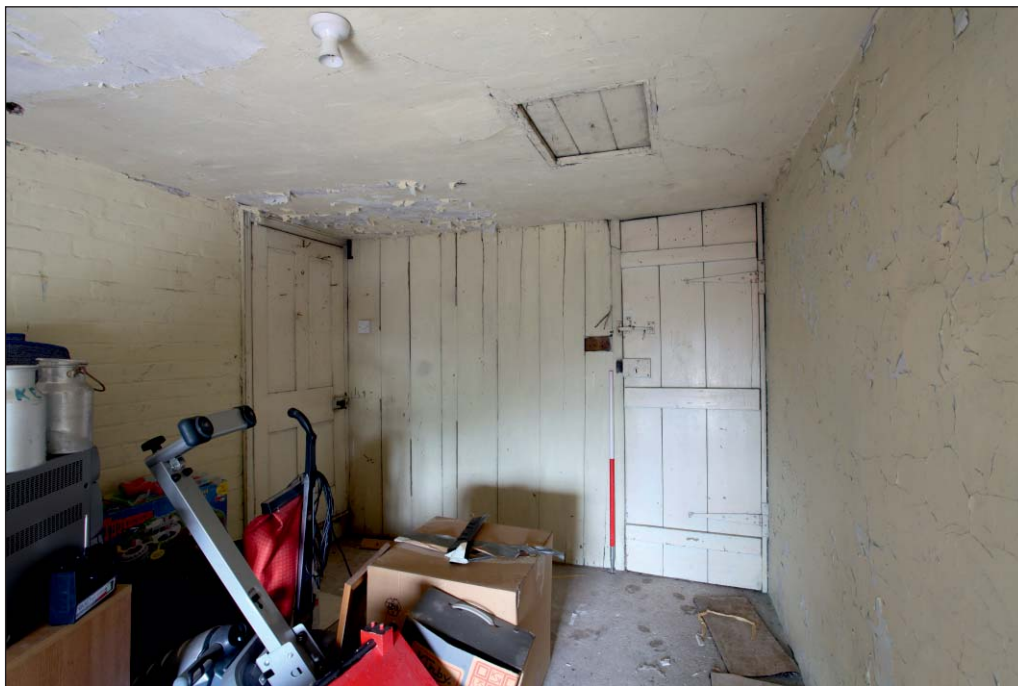
Plate 32: General view of the west wing store room F06, Building 1
