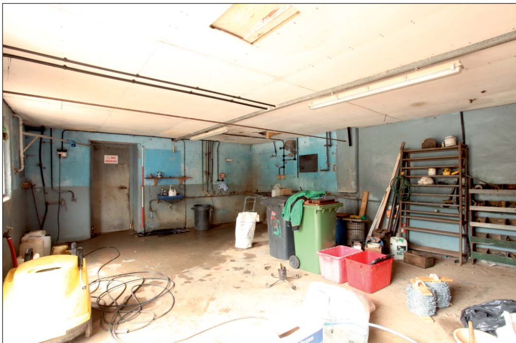
Plate 54: View of G23, Building 3, from the south-east
