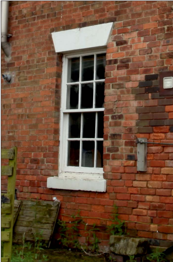
Plate 5: View of the remaining sash window to room G06, Building 1
