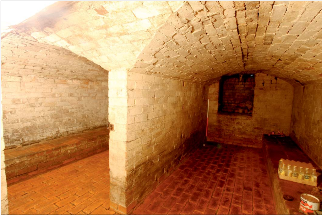
Plate 7: View of vaulted chambers B01 and B02, basement of Building 1
