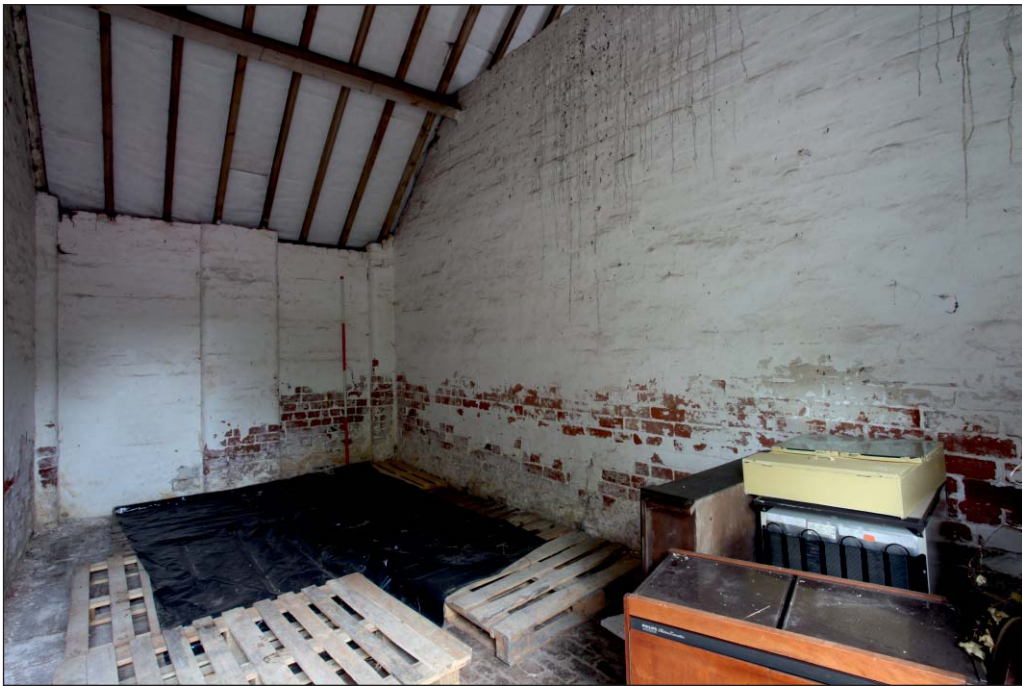
Plate 76: View of G19, Building 6, from the south-east
