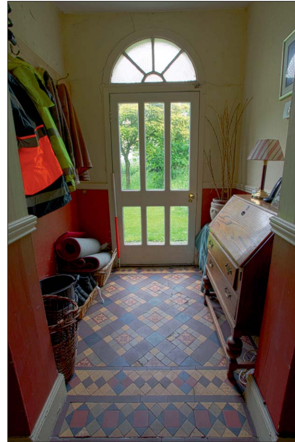
Plate 10: View of porch (G30), Building 1, showing the fanlight door and mosaic floor tiles
