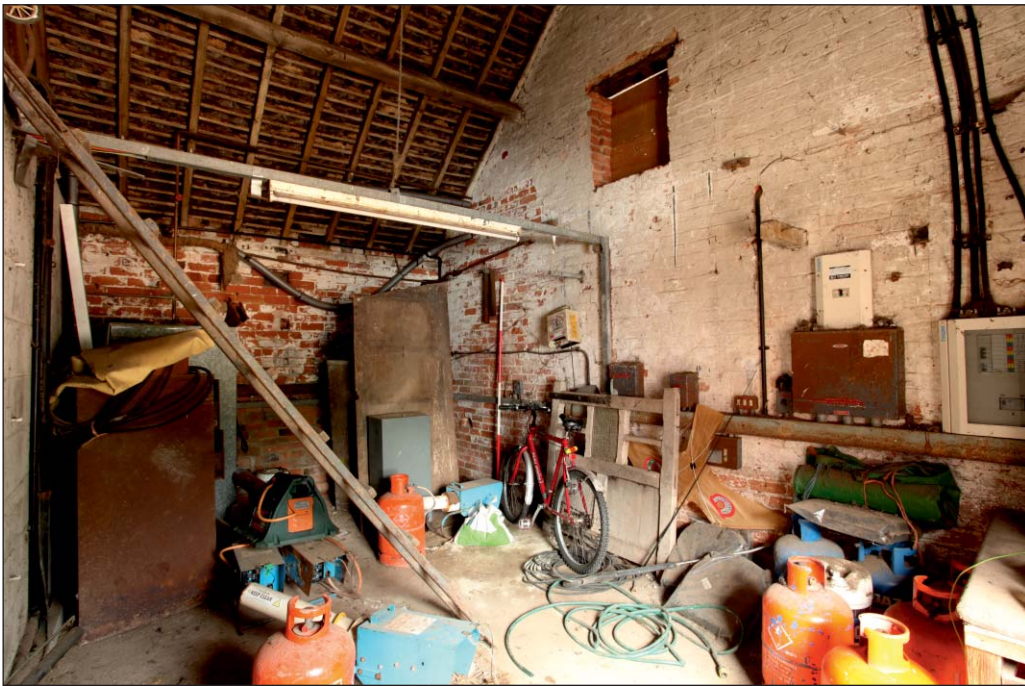
Plate 52: View of room G24, Building 3, from the south-west
