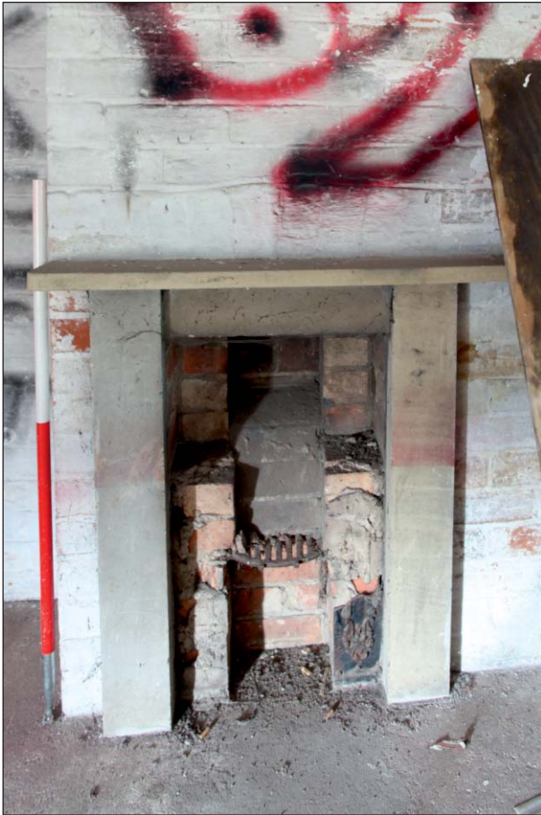
Plate 35: Detail of fireplace, F07, west wing of Building 1
