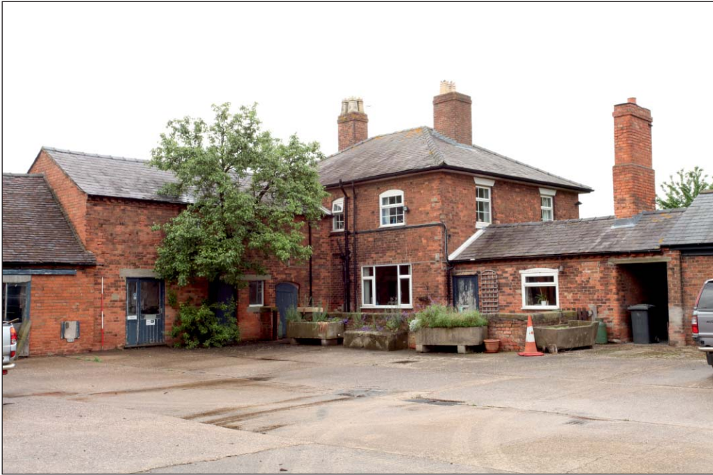
Plate 1: Building 1 farmhouse viewed from the southwest
