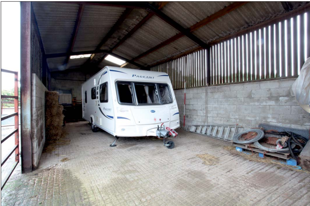
Plate 60: General view of G21, Building 4, viewed from the north-west
