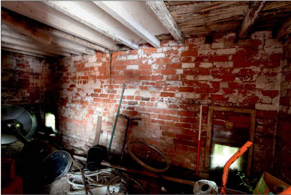
Plate 49: View of G15, Building 2 showing the hatches in the south wall
