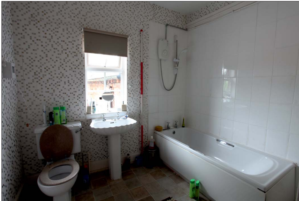
Plate 31: General view of bathroom F05, Building 1
