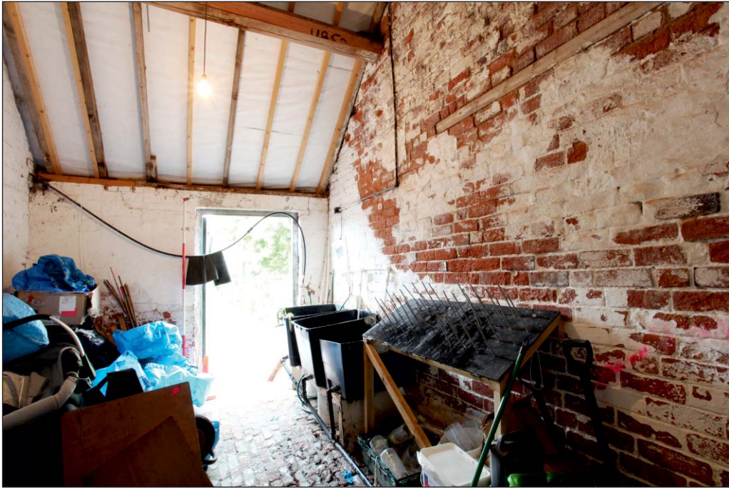
Plate 77: View of G20, Building 6, from the north-west
