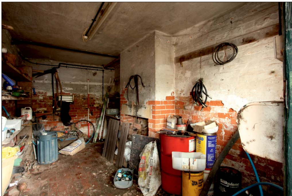
Plate 24: View of G26 in the west wing of Building 1
