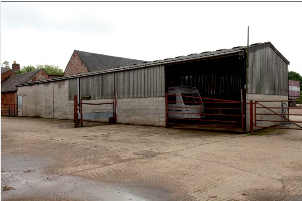
Plate 56: Building 4 viewed from the north-west
