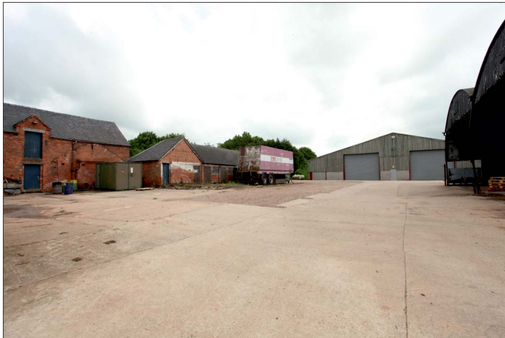
Plate 84: Vehicle shed and granary viewed in relation to Buildings 5 and 6 (left)
