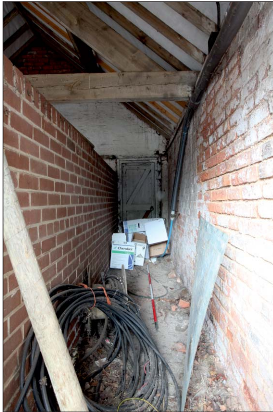
Plate 73: View of G16, Building 6, from the east
