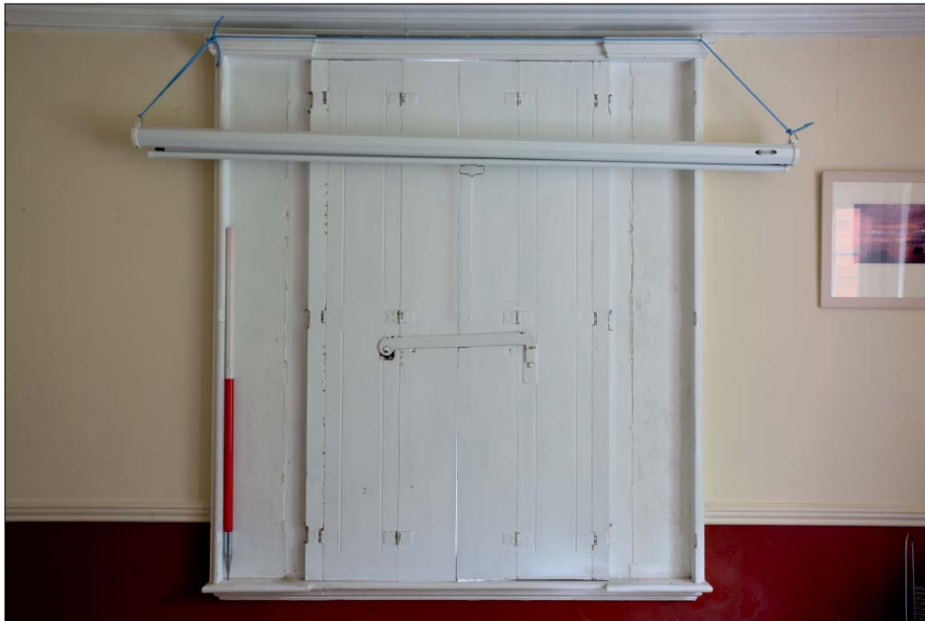
Plate 15: Detail of shuttered window in room G02, Building 1
