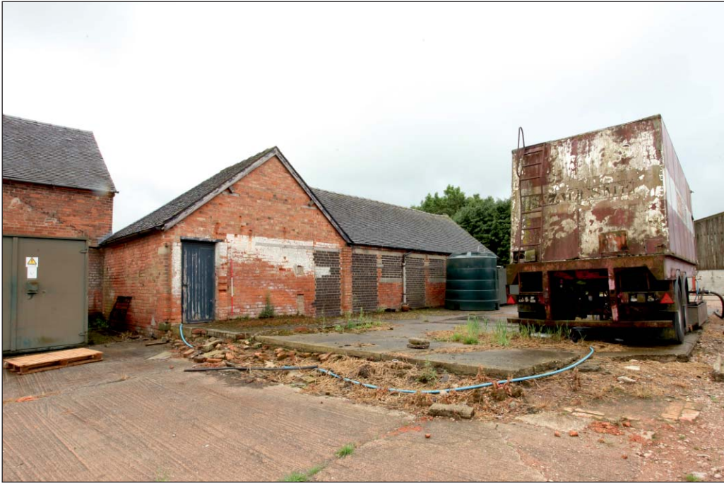
Plate 71: Building 6 viewed from the north-west
