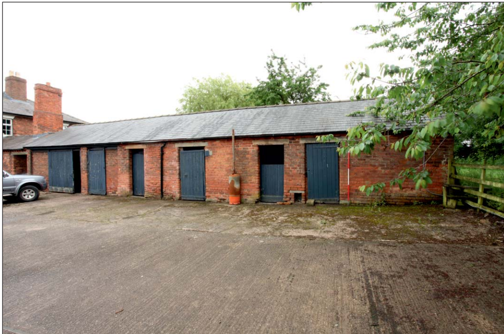
Plate 38: View of the west elevation of Building 2, viewed from the south-west
