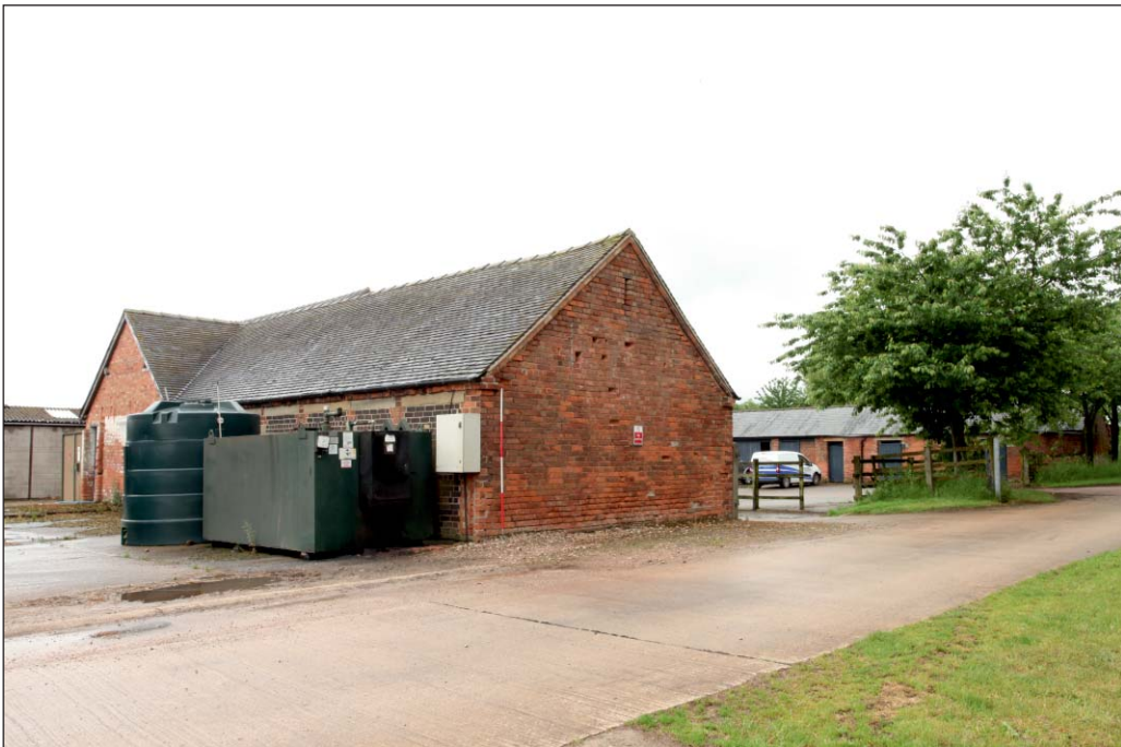
Plate 70: Building 6 viewed from the south-west
