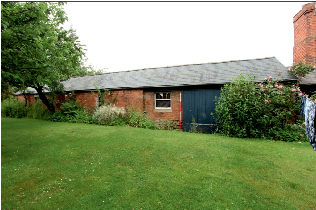
Plate 40: View of Building 2, east elevation, from the north-west
