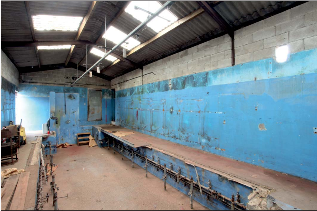
Plate 59: View of G22 milking parlour, Building 4, from the north-west
