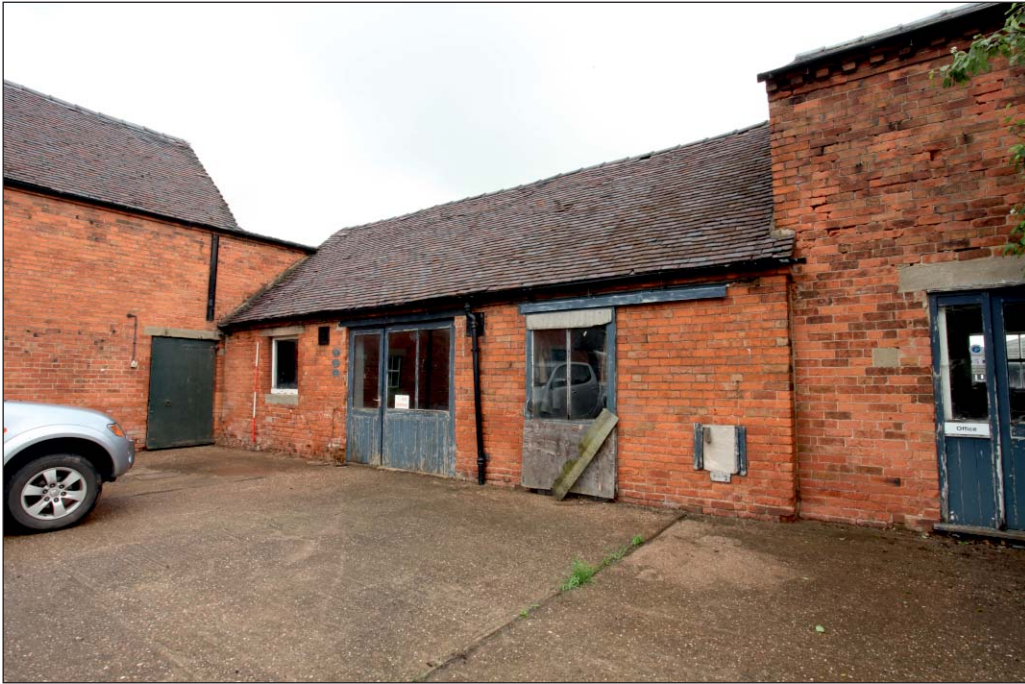
Plate 51: Building 3 viewed from the south-east
