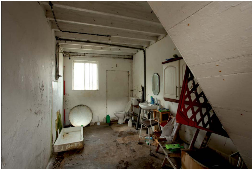
Plate 23: View of G27 in the west wing of Building 1
