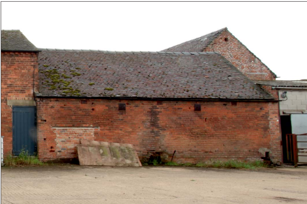
Plate 50: Building 3 viewed from the north
