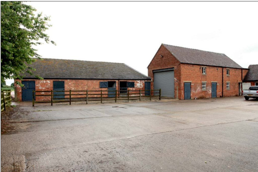
Plate 68: Building 5 and 6 (right to left) viewed from the south-east
