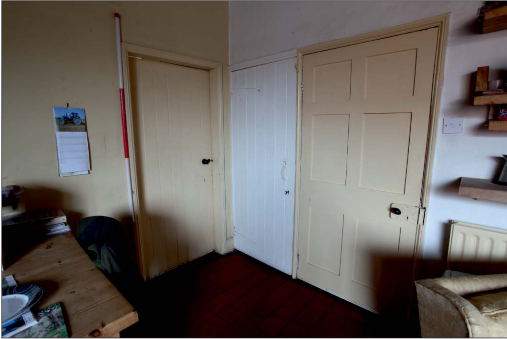
Plate 19: Detail view of the doors in the north-east corner of kitchen G05, Building 1, to illustrate the variety of door types and lock fittings in the building
