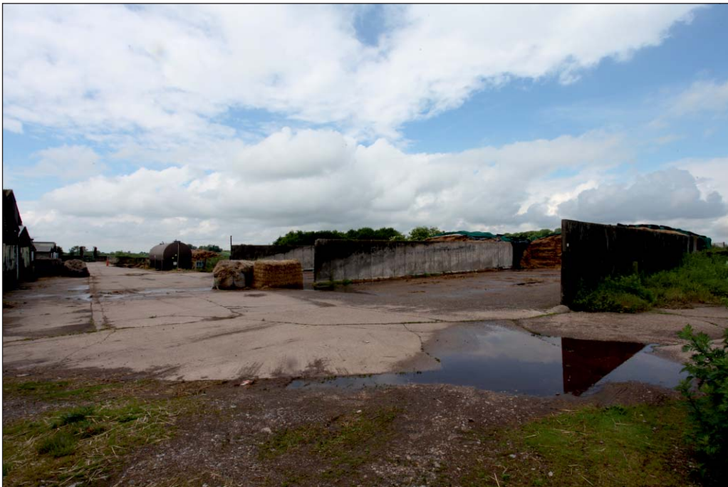
Plate 86: Slurry beds to the north of the farm buildings
