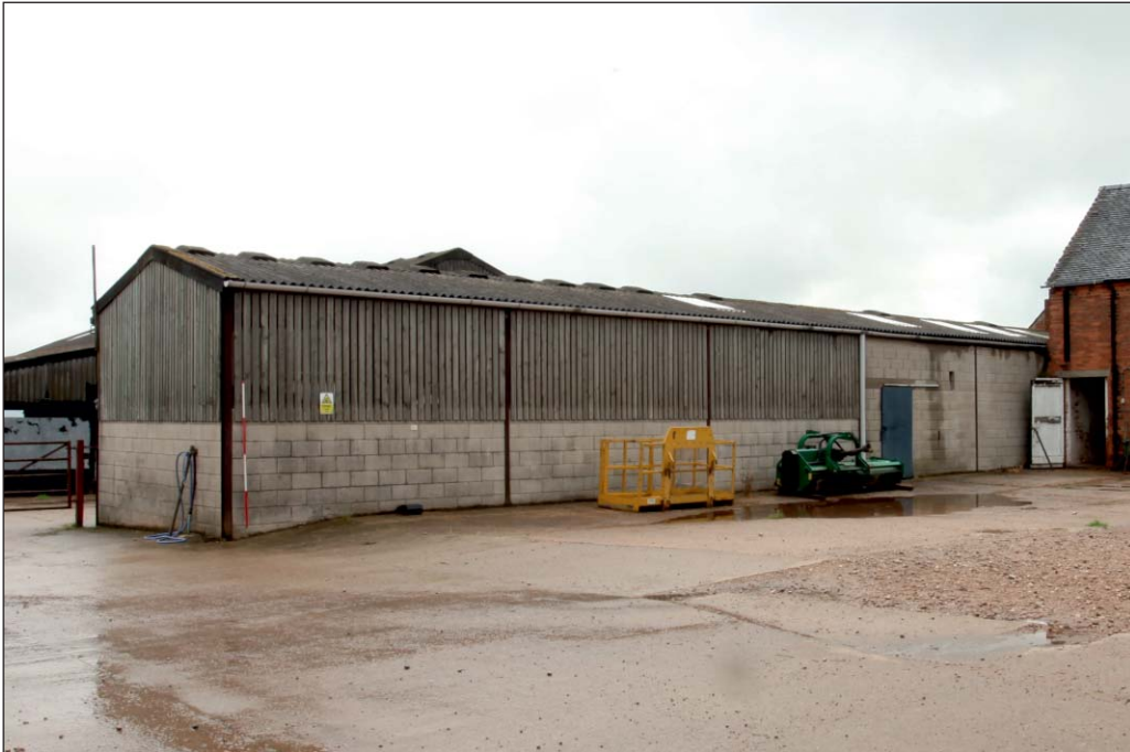
Plate 57: Building 4 viewed from the south-west
