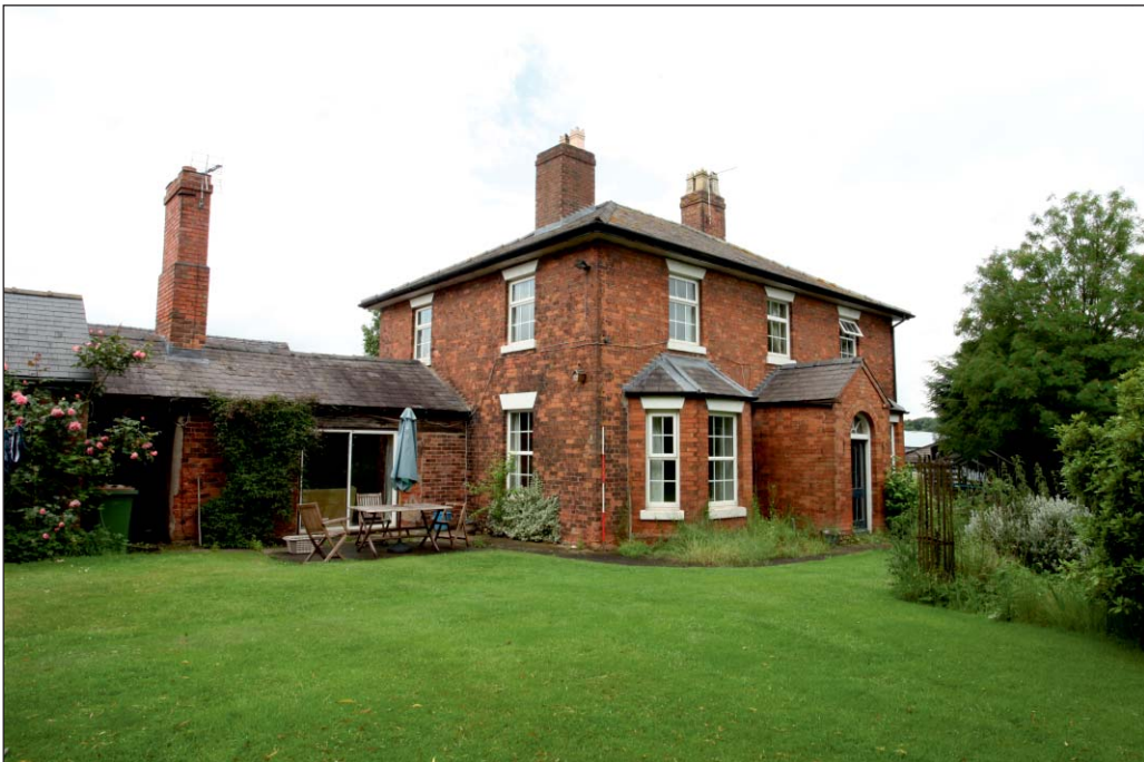
Plate 2: Building 1 viewed from the southeast
