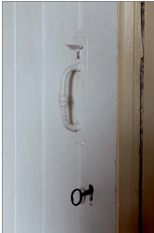
Plate 20: Detail view of basement door handle in G05, Building 1
