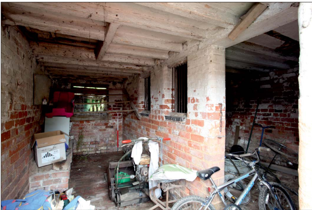
Plate 48: View of G14 (left) and G15 (right), Building 2
