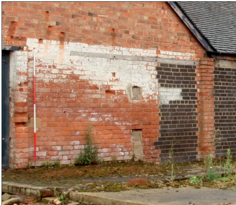
Plate 72: Detail of the long timber lintel and remnant concrete block wall on the west elevation of Building 6
