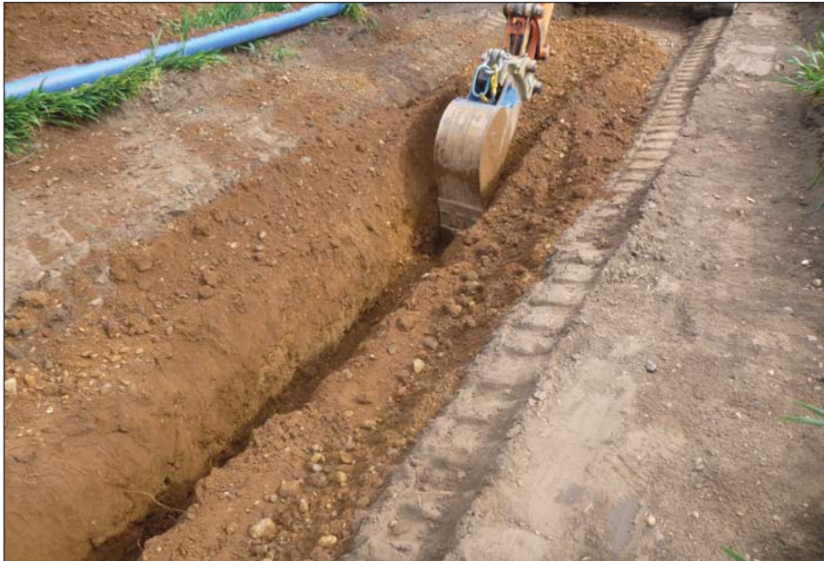
Plate 4: Working shot of pipe installation, view from the south-west
