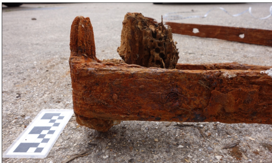
Plate 8: MAG_6384 Wooden and metal debris
