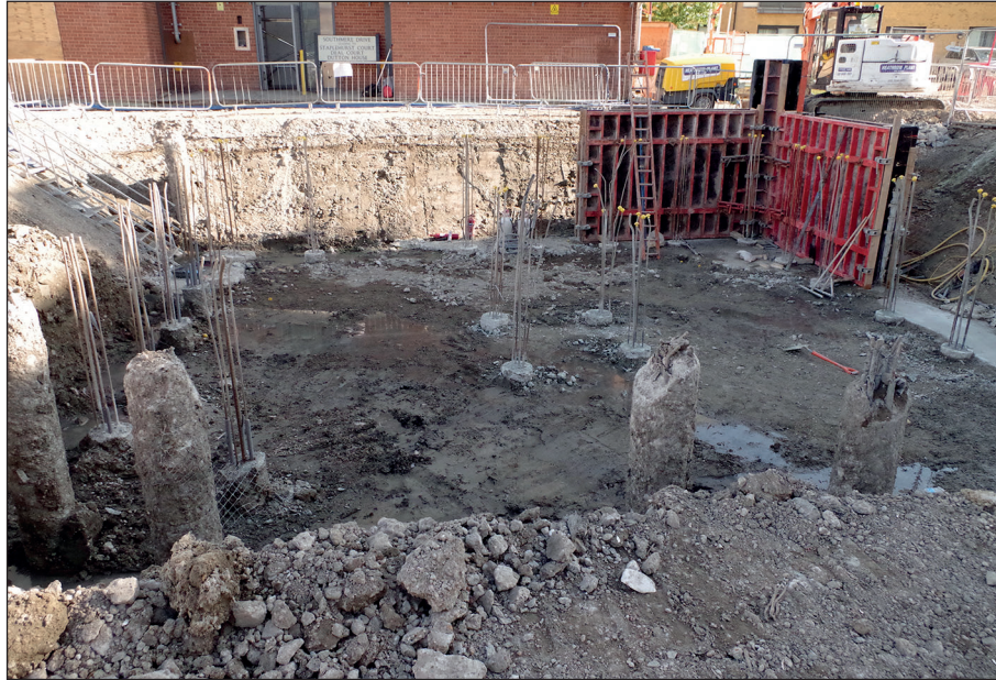
Plate 1: Overview of Area 1, taken from the south.
