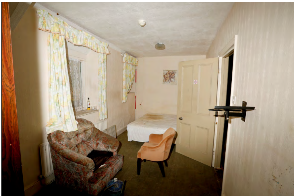
Plate 40: Bedroom F09 constructed on top of Kitchen corridor
