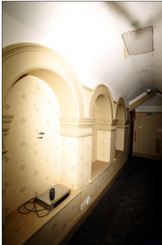
Plate 39: Late 19th century blocked arches in first floor landing
