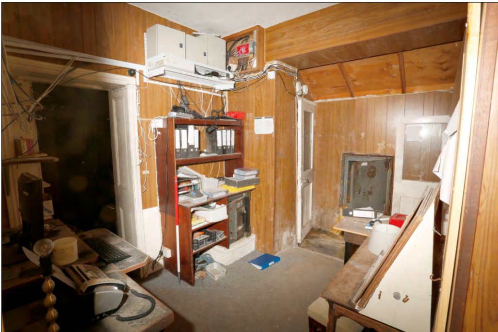
Plate 22: Ground floor office G04
