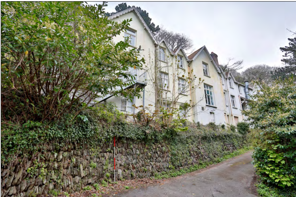
Plate 10: South-west elevation viewed from the west
