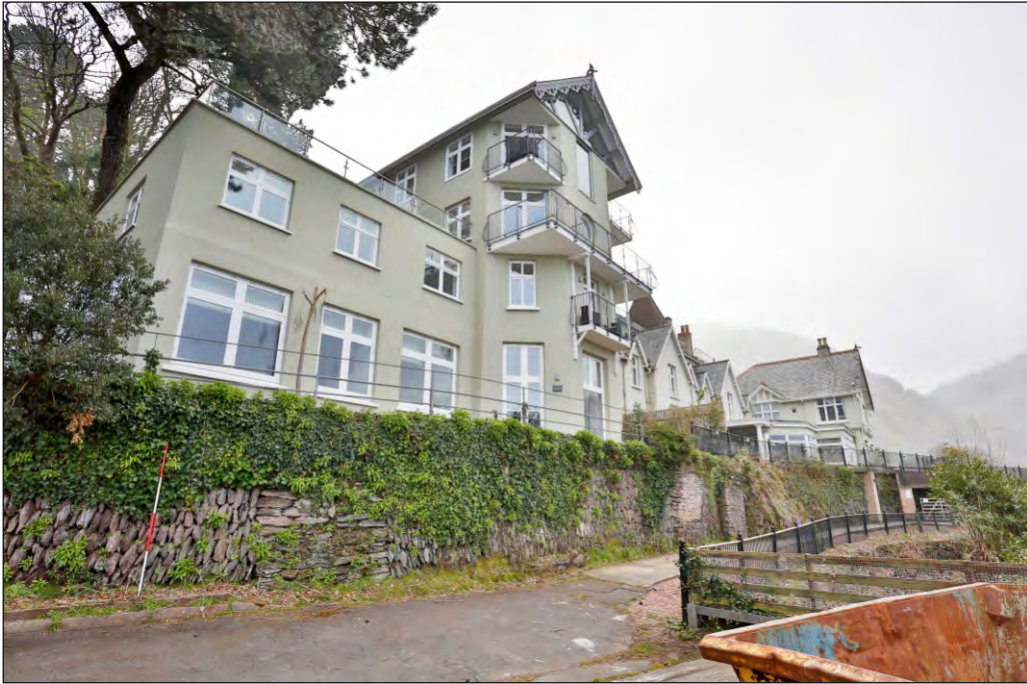
Plate 9: North-west elevation showing refurbished north-east tower
