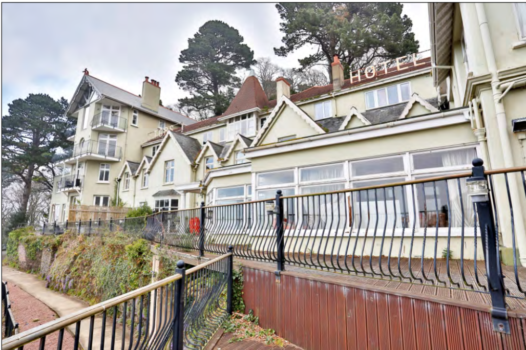
Plate 8: North-west elevation showing multiple phases of build viewed from the south-west
