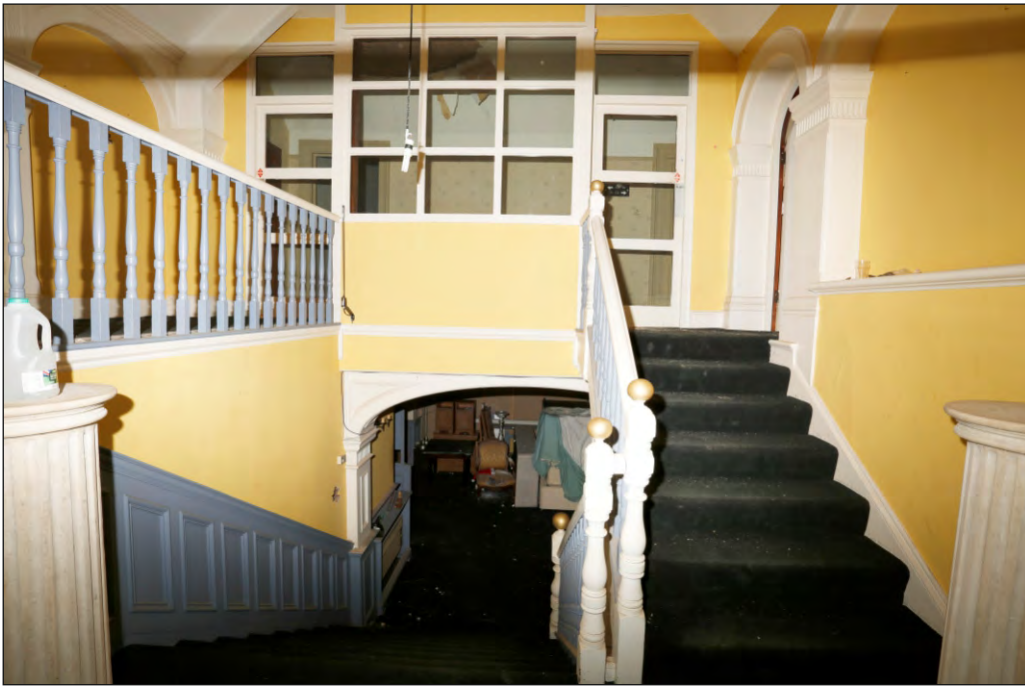
Plate 35: Main staircase F01
