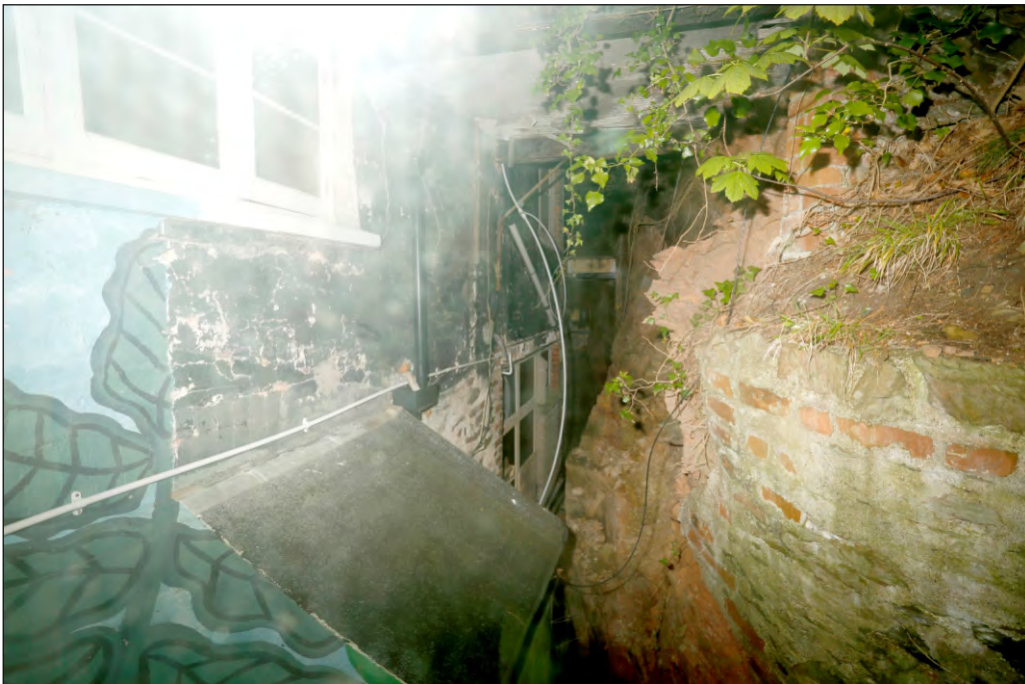
Plate 12: Rear of north-west range close up against rock face
