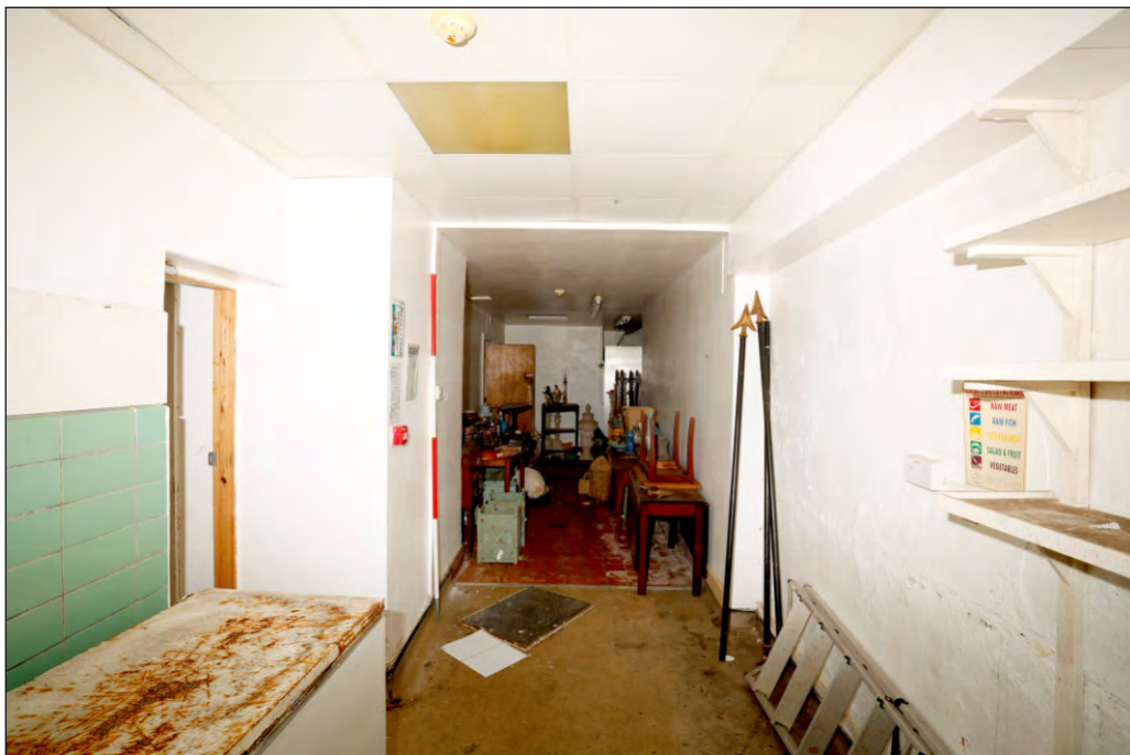
Plate 30: South-west wing enclosed kitchen corridor
