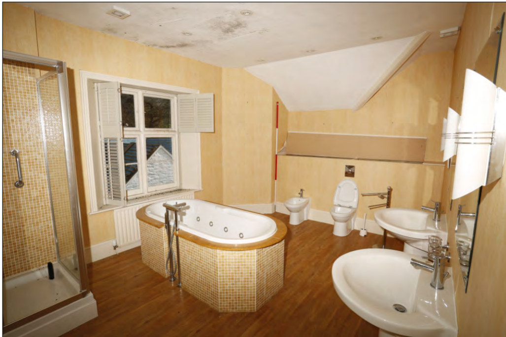
Plate 47: Second floor bathroom S09
