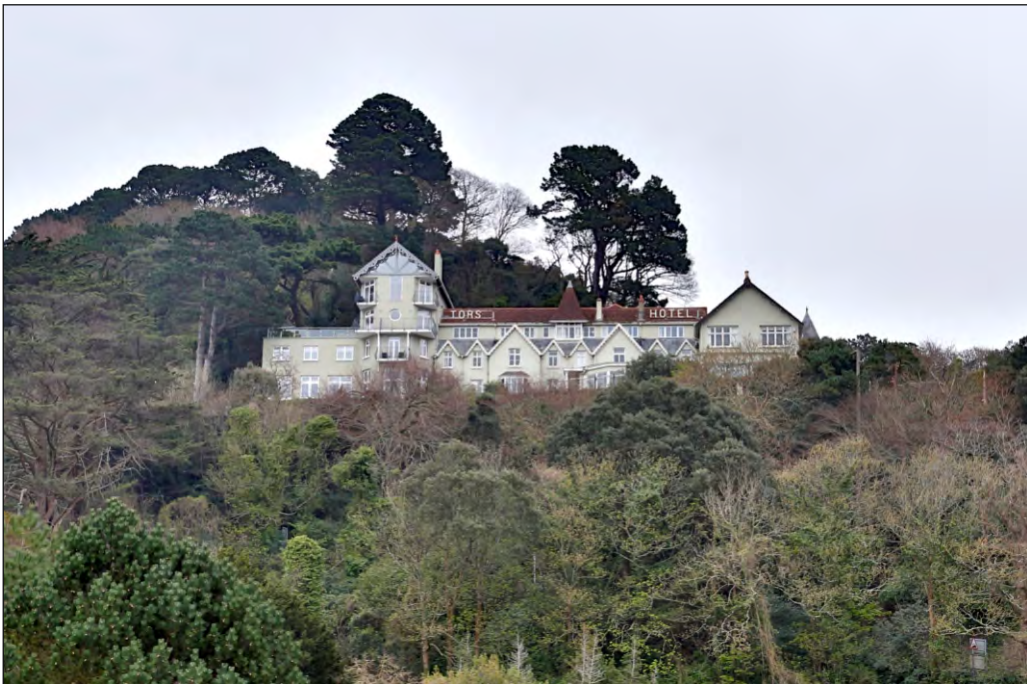
Plate 2: Low level view of north-west elevation from the west
