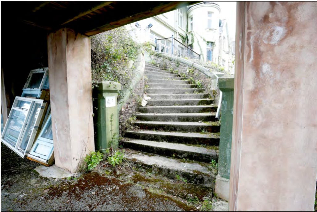
Plate 5: Main access steps and piers
