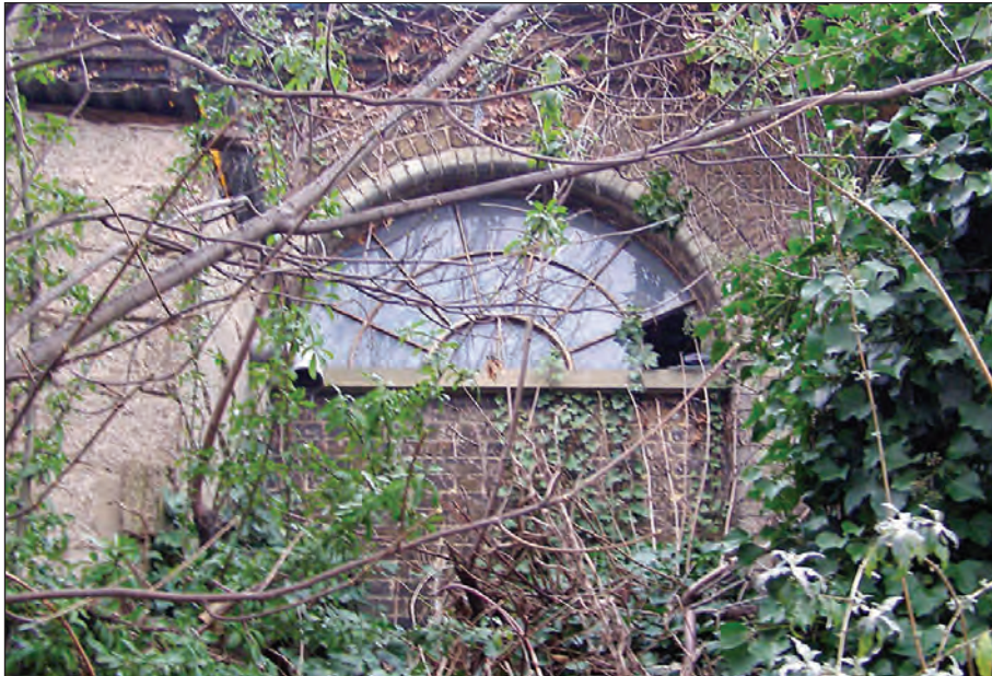
Plate 10: Example of the semi-circular cast iron windows (external), facing north
