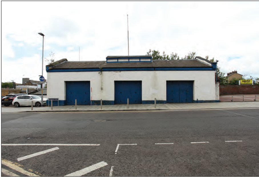
Plate 3: View of the north elevation, facing south
