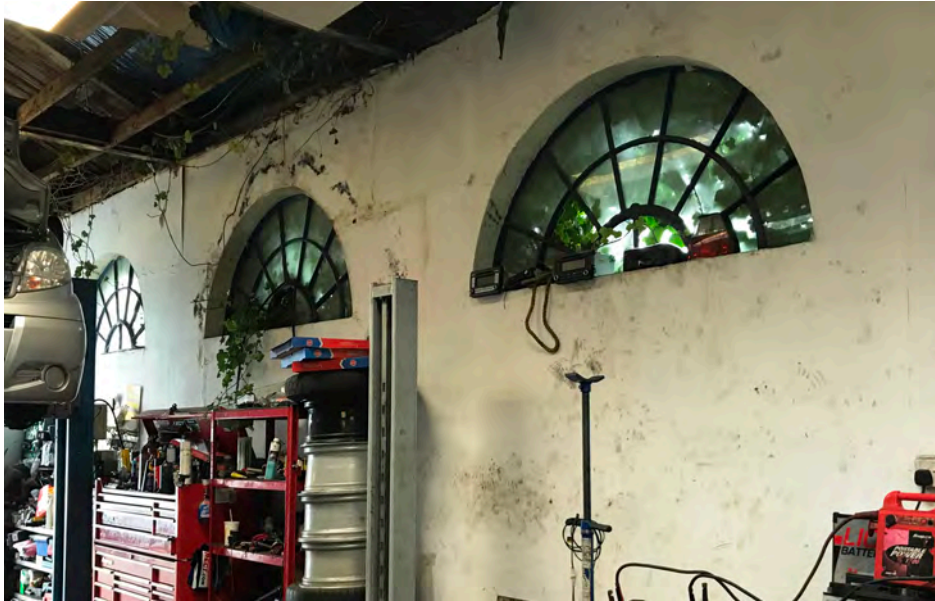
Plate 7: Semi-circular cast iron windows on the south wall facing southeast
