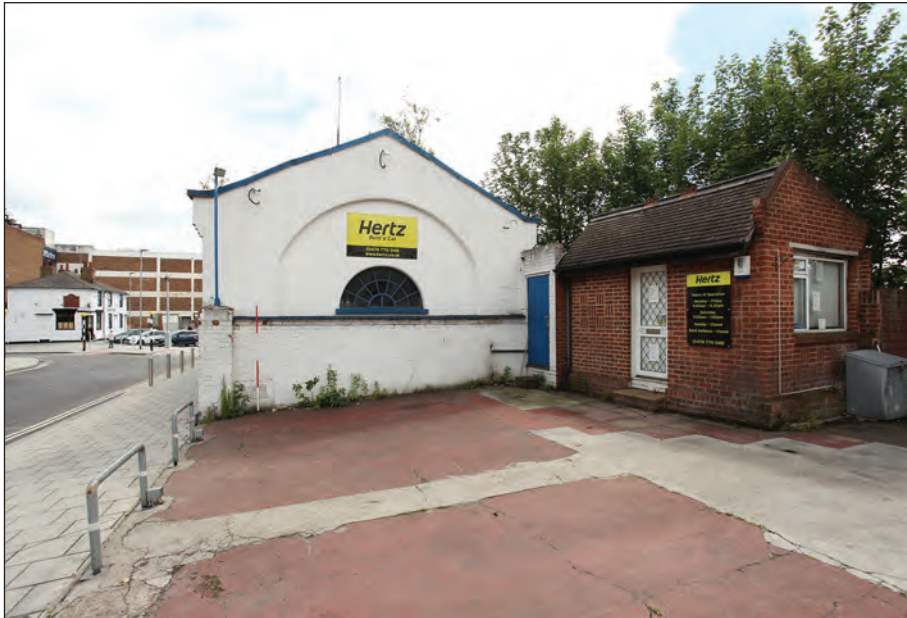
Plate 4: View of the rear elevation, facing southeast
