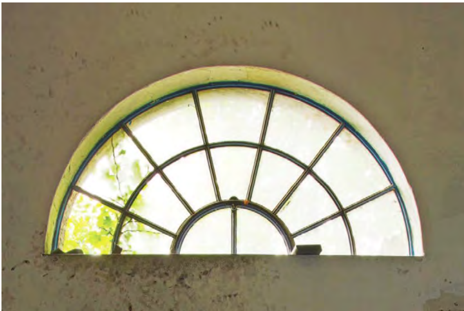
Plate 8: Example of a semi-circular cast iron windows facing south
