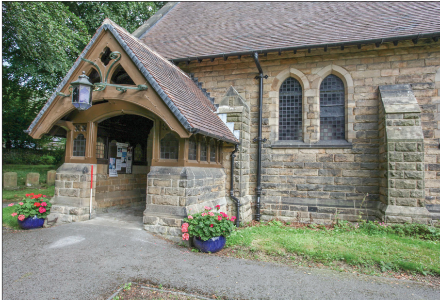
Plate 4: General view of the South Porch, viewed from the south-east
