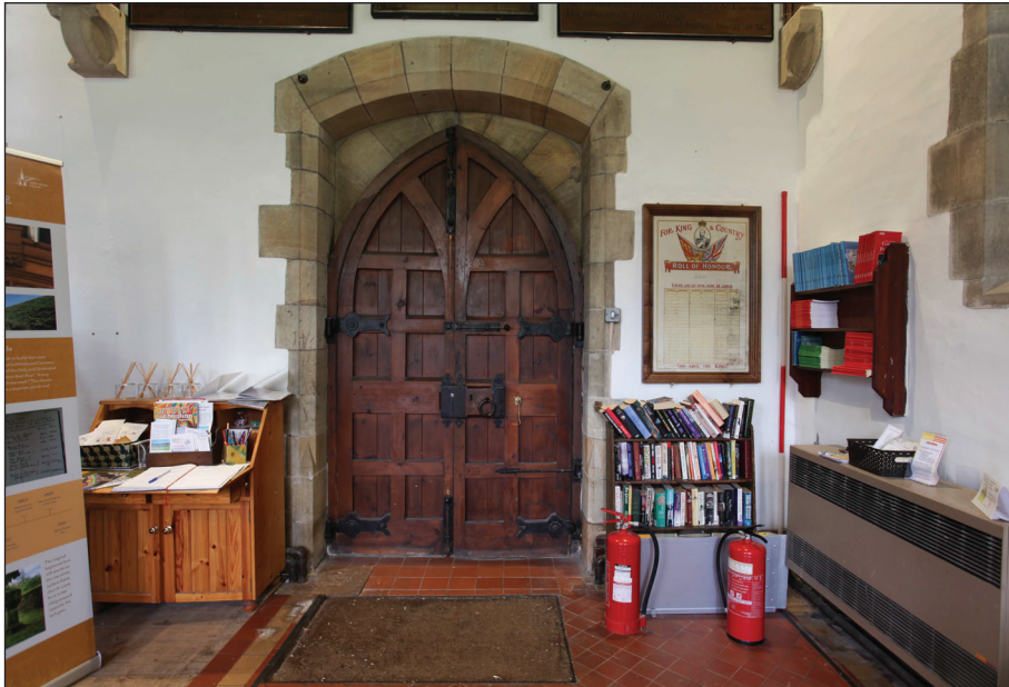
Plate 14: Western end of the south wall adjacent to the doorway to the South Porch
