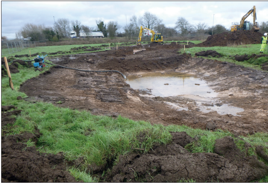
Plate 5: Overview of working area, view from the south-west
