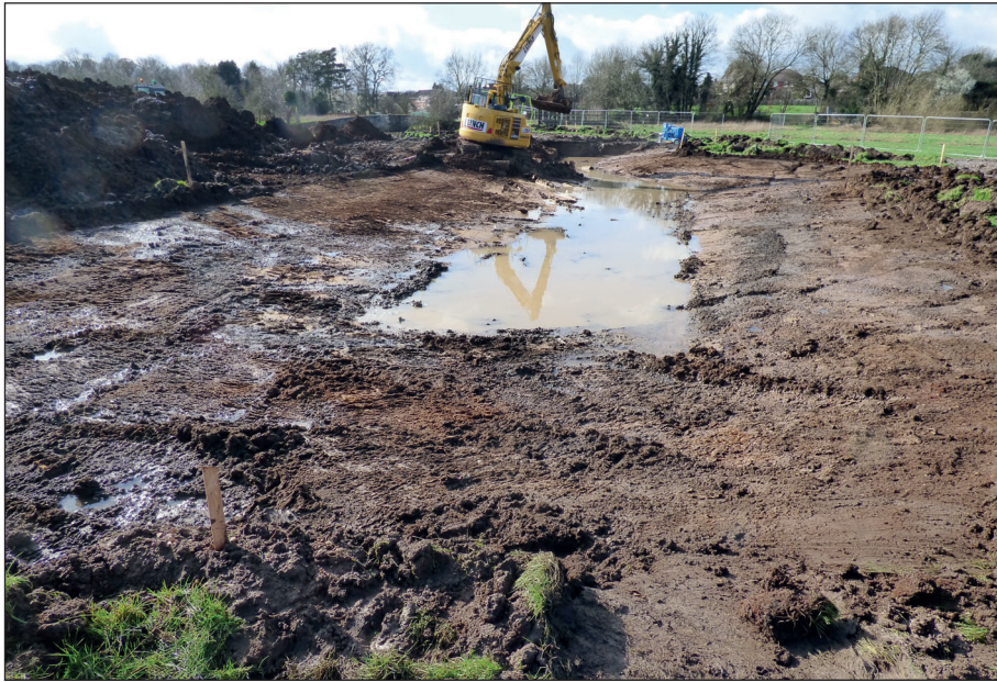
Plate 7: Overview of working area, view from the north
