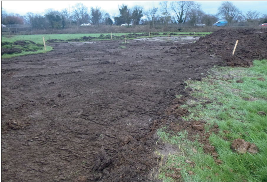
Plate 1: Overview of area topsoil stripped, view from the south
