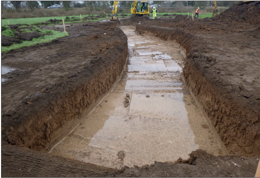
Plate 3: Trench in middle of the site, view from the south-west
