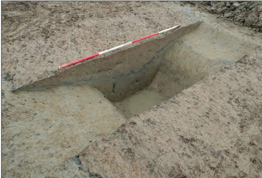
Plate 12: North-west facing section through ditch 35, viewed from the north. Scale: 2 m
