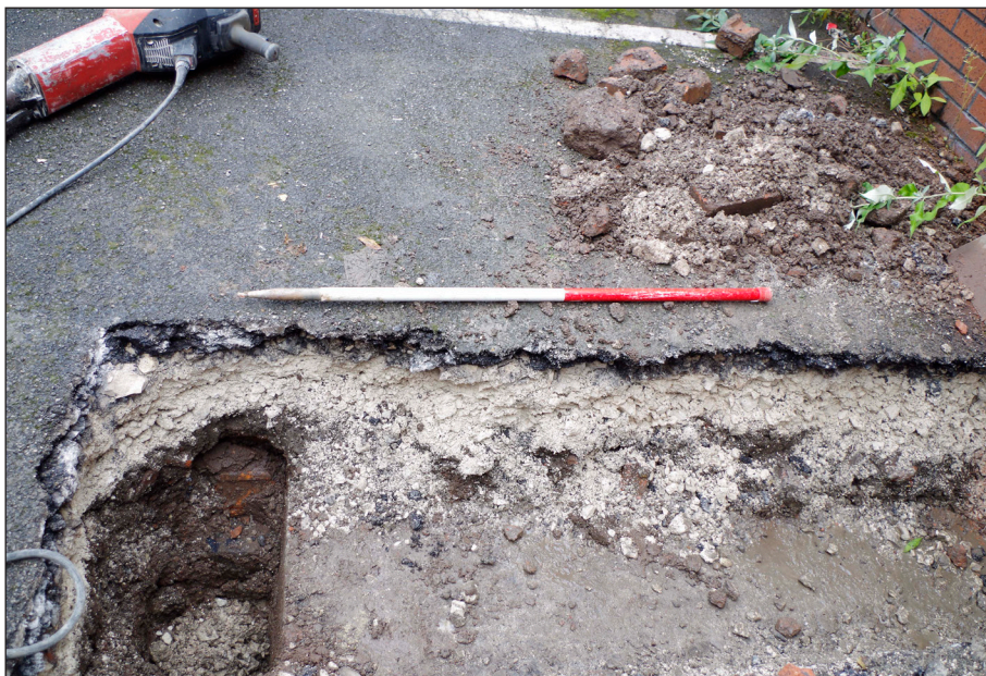
Plate 24: FP 13, section view from the west
