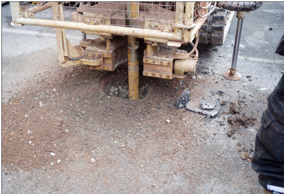
Plate 29: BH 16, layer at around 3.0 m
