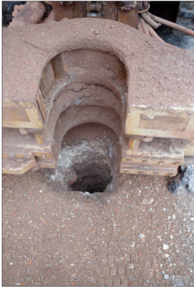
Plate 27: BH 16, Rotary drilling rig
