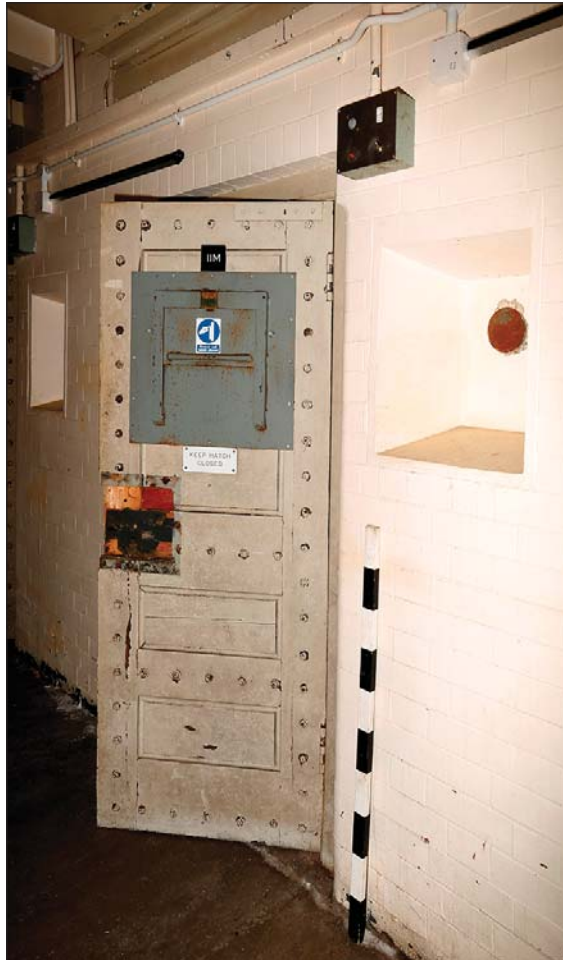
Plate 48: Detention lower ground floor: Eastern Cell Block - a typical cell door (11M)
