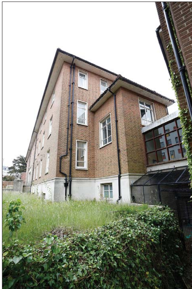
Plate 6: Stair tower at the north-west end of the Police Station and glazed link to the Annexe
