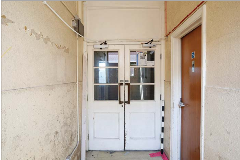
Plate 25: Main range ground floor: double doors to rear entrance lobby (G25)
