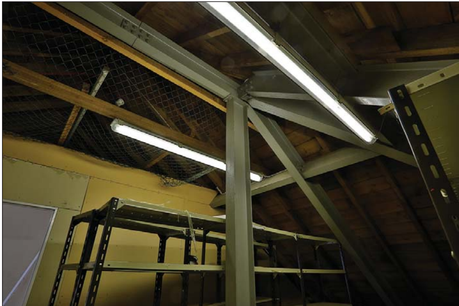
Plate 35: Main range third floor: Steel frame roof structure (T03)
