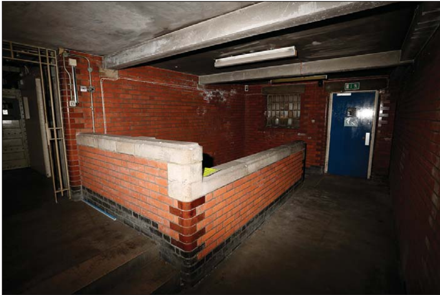
Plate 54: Ground floor: Link stairwell between the Eastern Cell Block and the County Court
