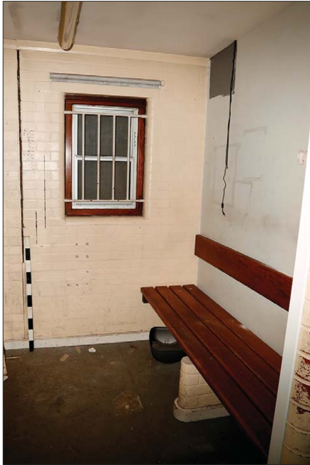
Plate 40: Custody ground floor: reception area (G01) - north corner
