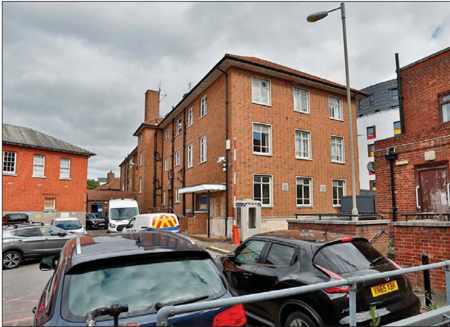
Plate 7: Police Station side (south-east) and rear (south-west) elevations
