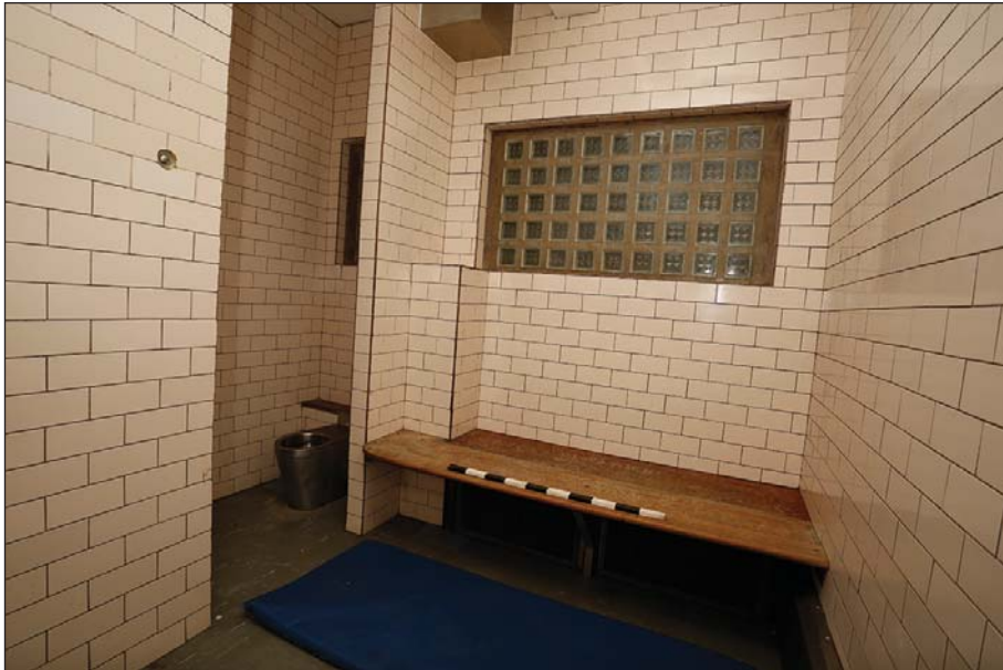
Plate 65: Detention lower ground floor: Western Cell Block - a typical cell (D2)
