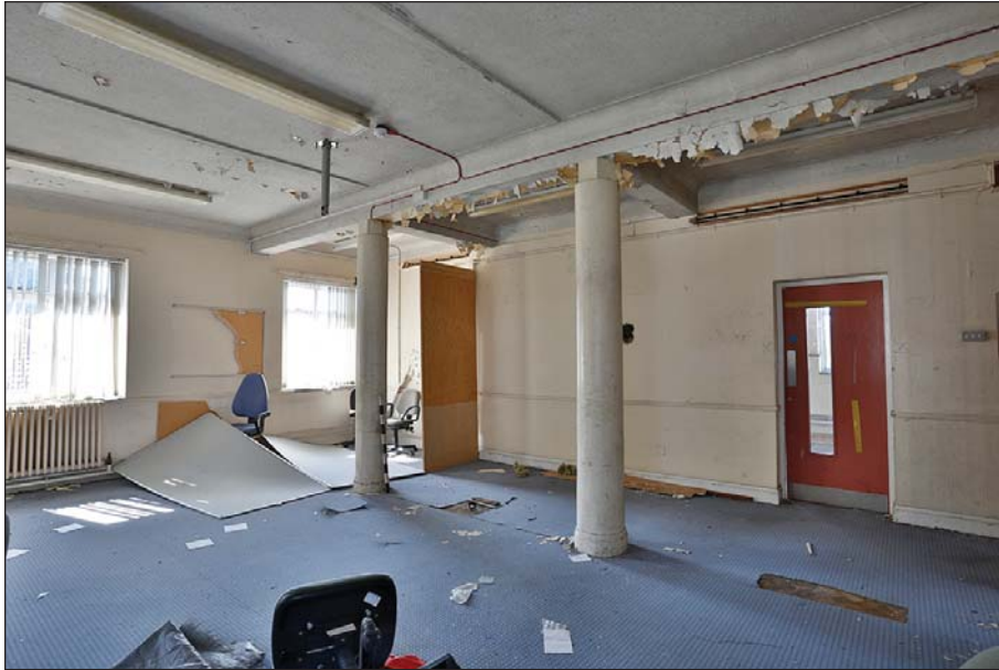
Plate 28: Main range second floor: communal room, likely the officers' mess (S11)
