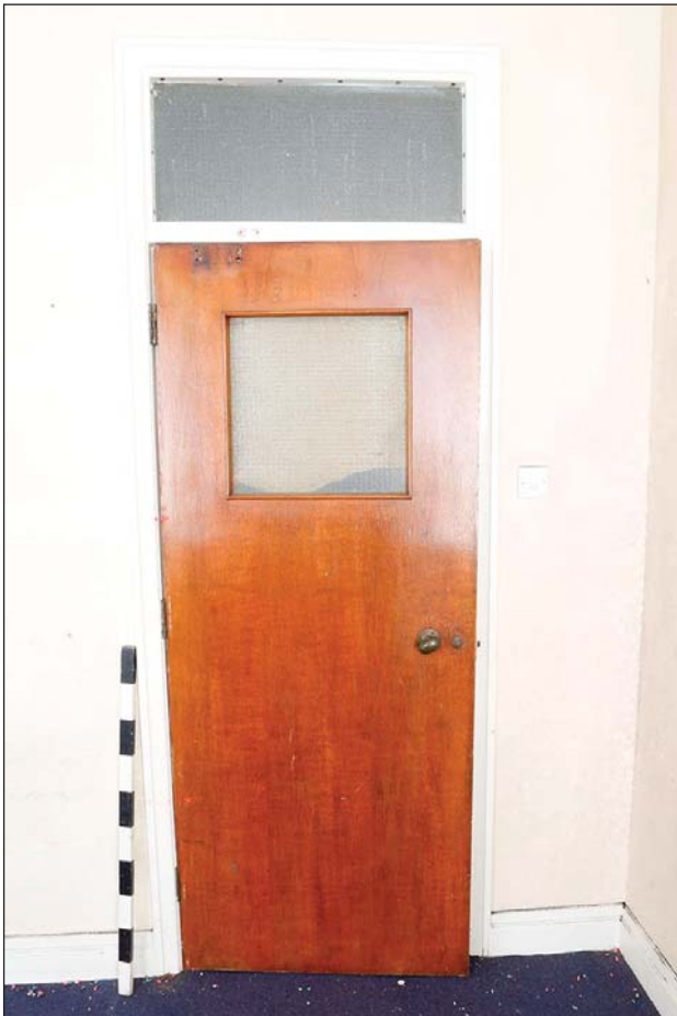
Plate 26: Main range first floor: typical example of an original office door with brass fittings (F17)
