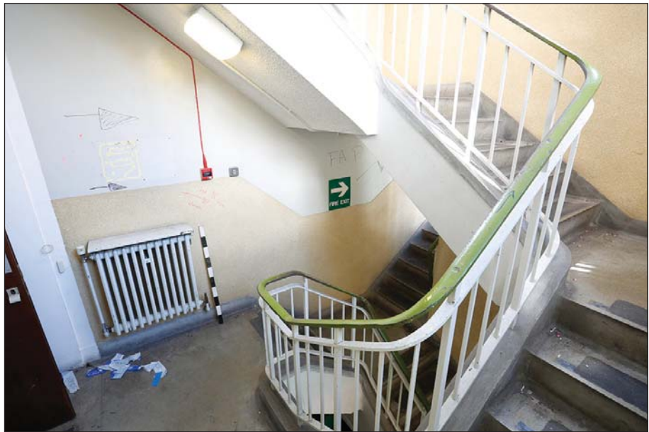
Plate 18: Main range ground floor: north-west stairwell (G15)
