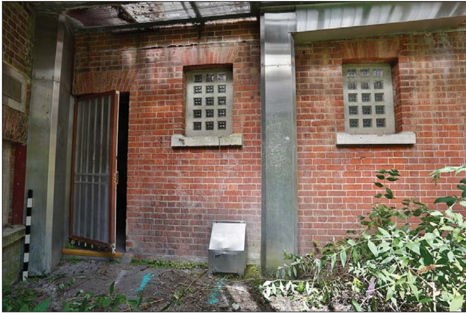
Plate 56: Exercise yard - north-east wall
