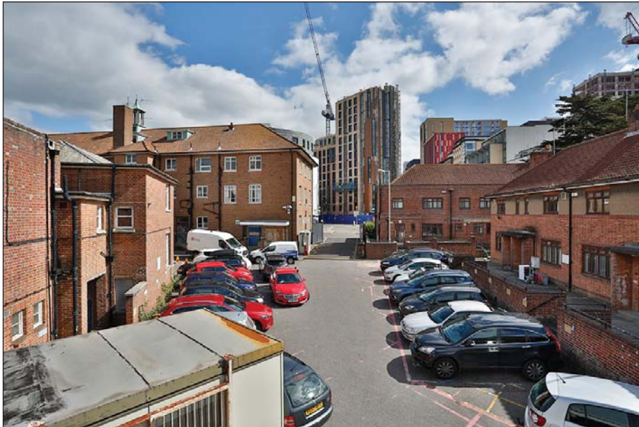
Plate 4: View from the multi-storey car park within the Site. It shows the open car park surrounded by the law courts and police station (left) and 2, 4, 6 Madeira Road and 1-4 Madeira Court buildings (right)
