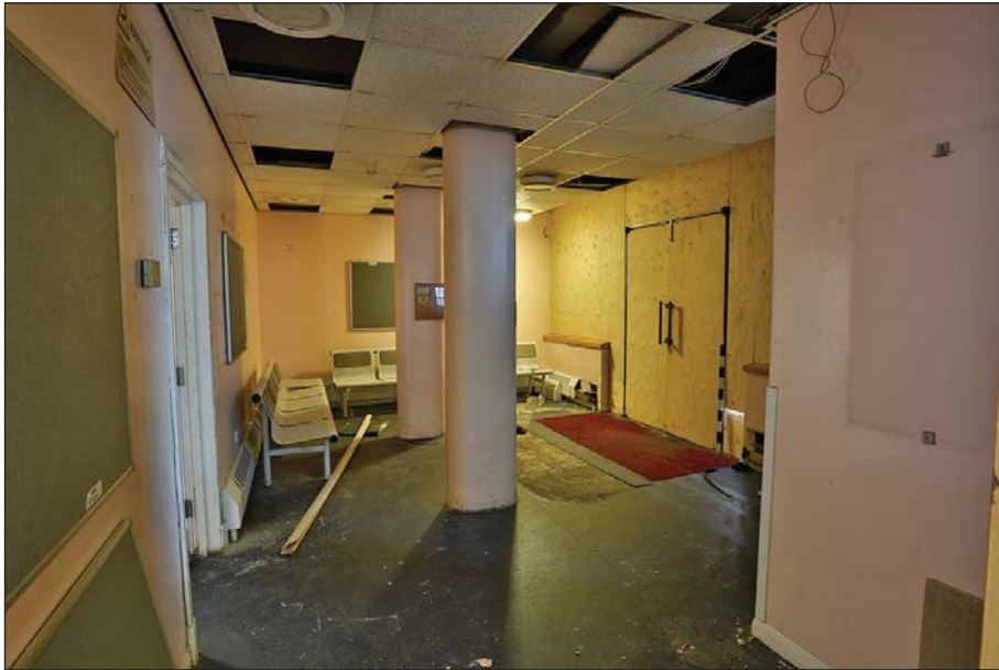
Plate 14: Main range ground floor: entrance foyer for enquiries (G32) - north-west end
