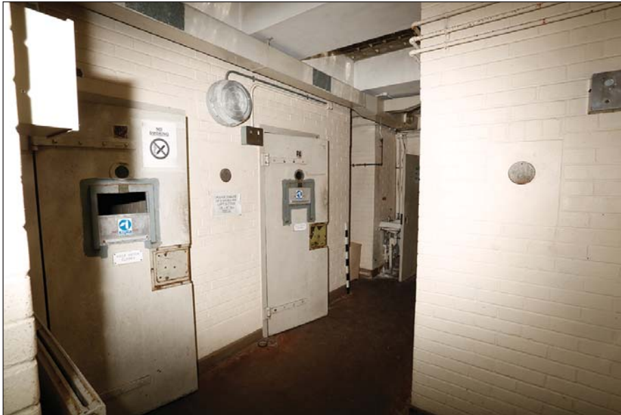
Plate 63: Detention ground floor: Western Cell Block - circulation area (G12)
