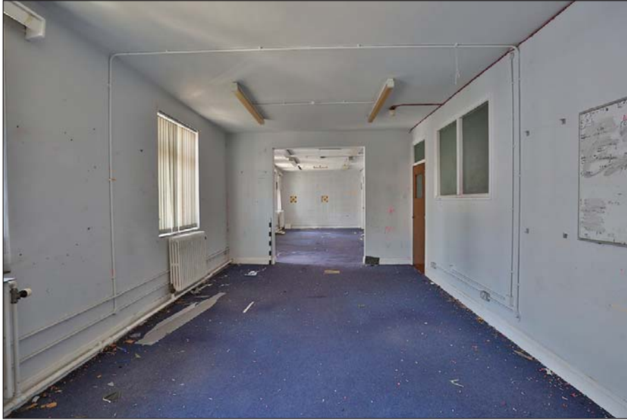
Plate 24: Main range second floor: offices S07 and S08 joined together by cutting through a partition wall
