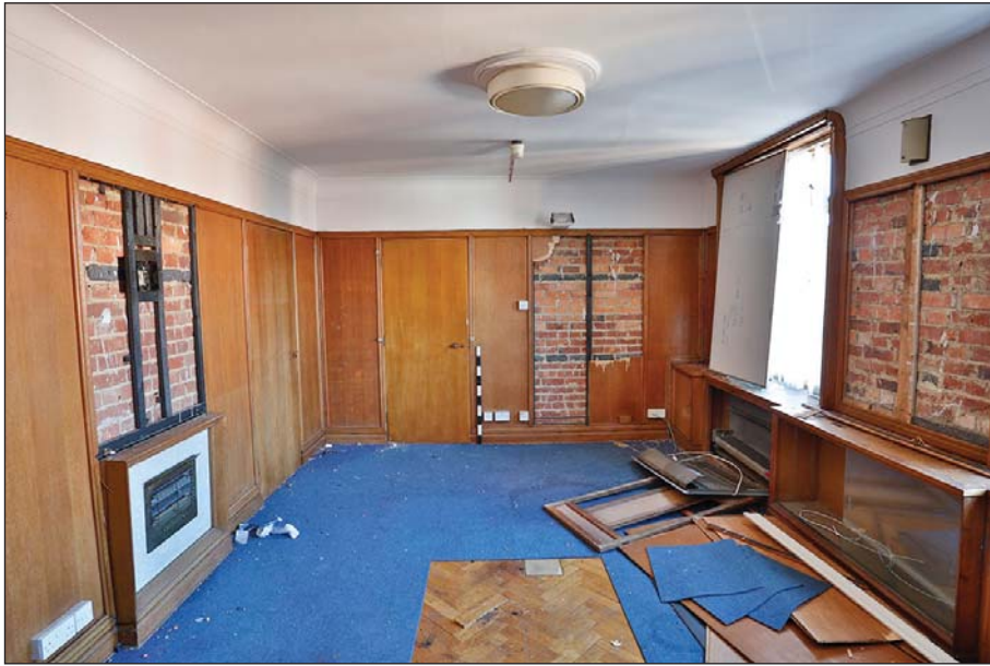
Plate 22: Main range first floor: Chief Constable's office (F24)
