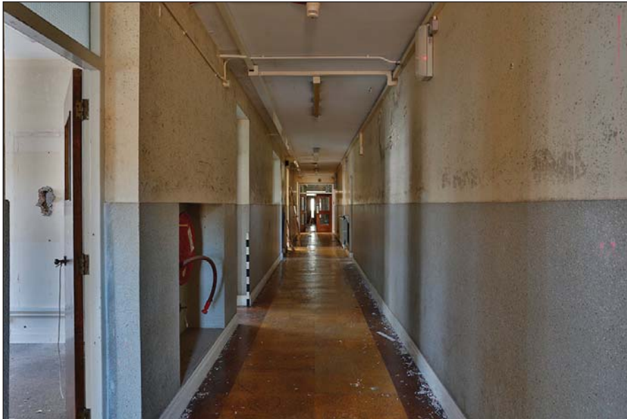
Plate 23: Main range second floor: main corridor (S03)
