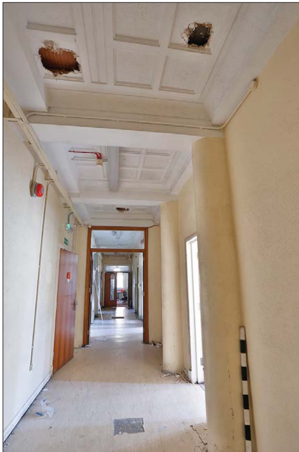
Plate 16: Main range ground floor: main corridor (G14), note the coffered ceiling
