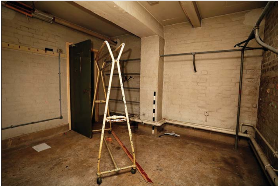
Plate 37: Main range lower ground floor: drying room (LG18)
