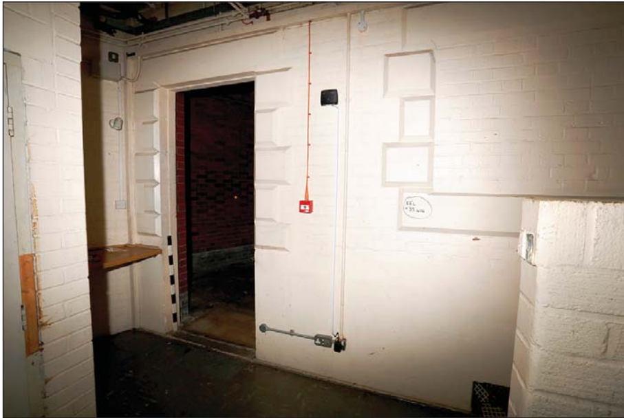
Plate 46: Detention lower ground floor: Rusticated door opening and blocked window in the previously external wall
