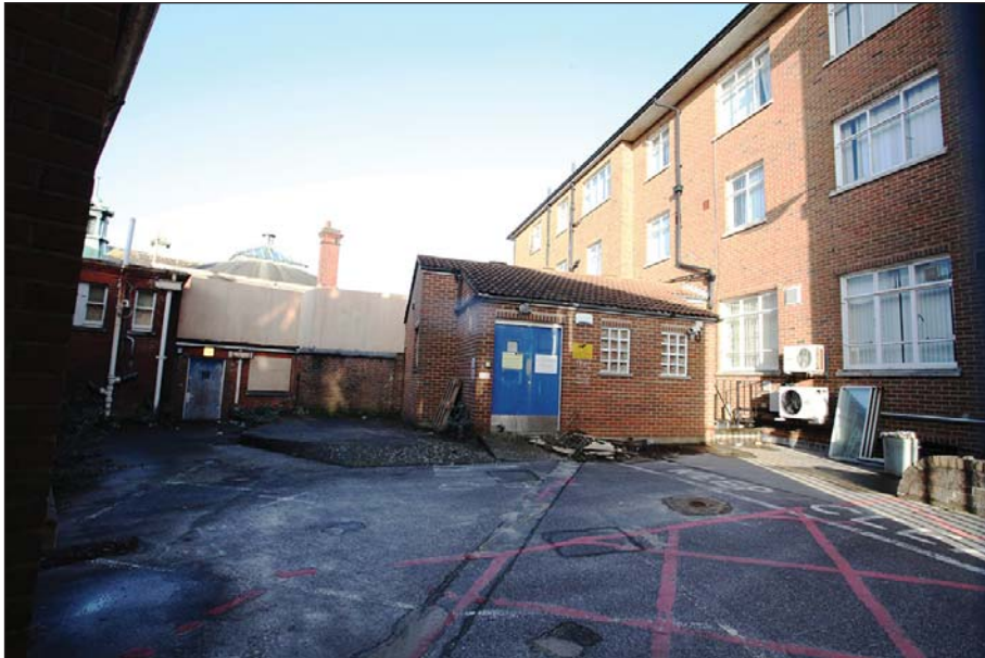
Plate 8: Rear west corner of the Police Station. The custody block is in the centre, with the exercise yard and cell blocks hidden behind it. The domed roof of Court 1 is visible in the background
