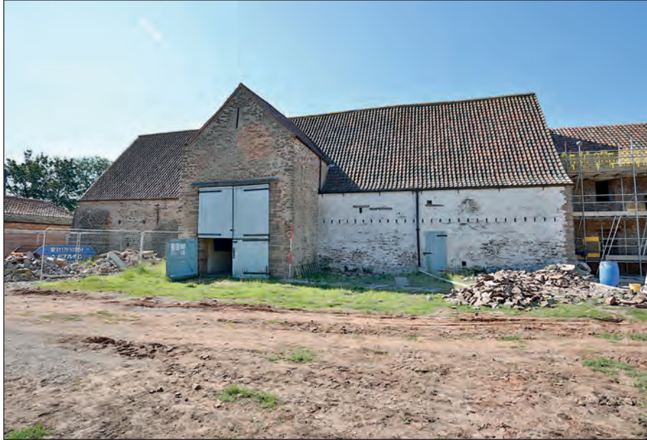
Plate 2: Main Barn viewed from north
