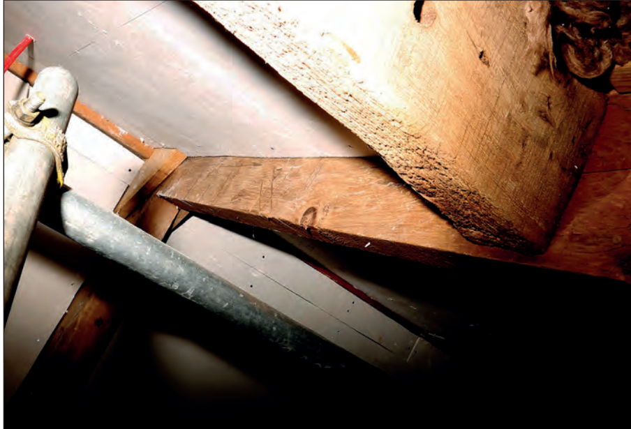
Plate 18: West Barn detail of race knife marks to principal rafter
