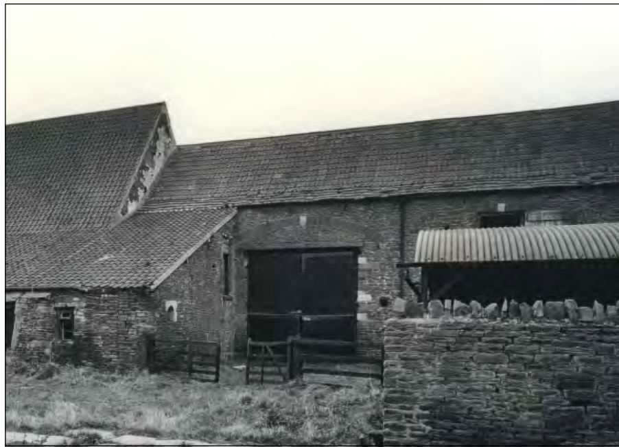
Plate 22: Undated photograph showing West Barn north elevation
