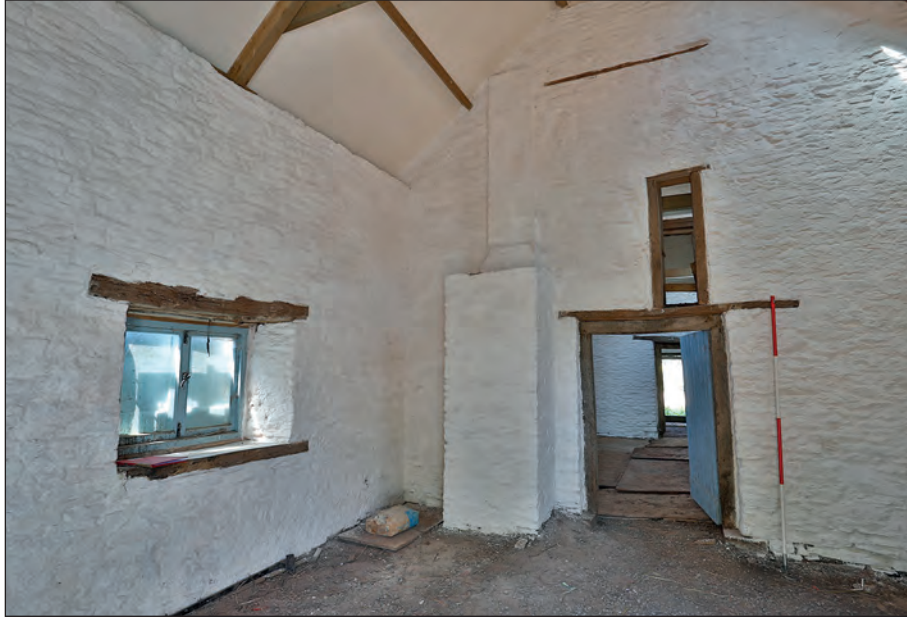
Plate 8: South Range east room interior
