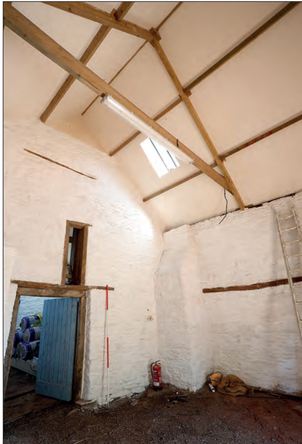
Plate 9: South Range east room roof
