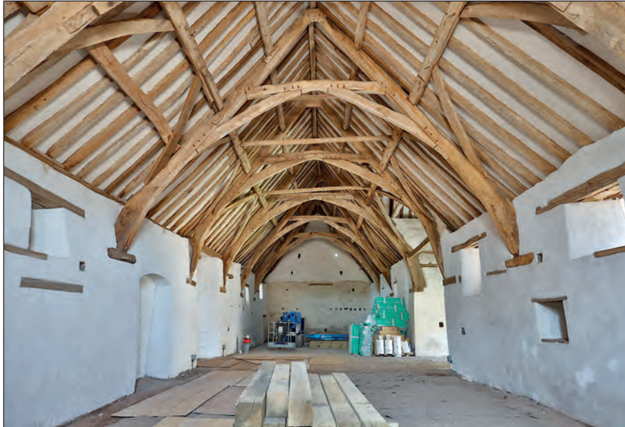
Plate 3: Main Barn interior viewed from east
