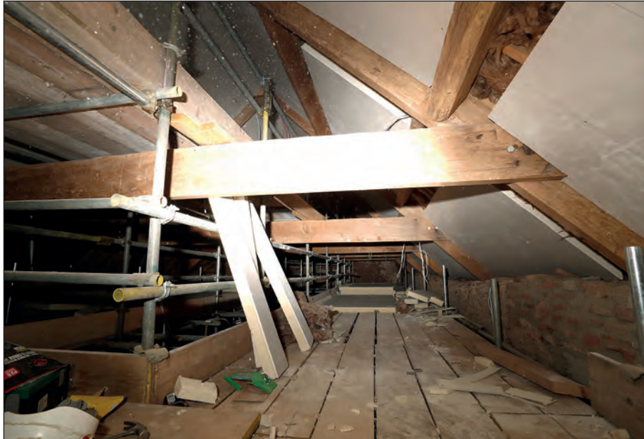
Plate 17: West Barn view of roof trusses
