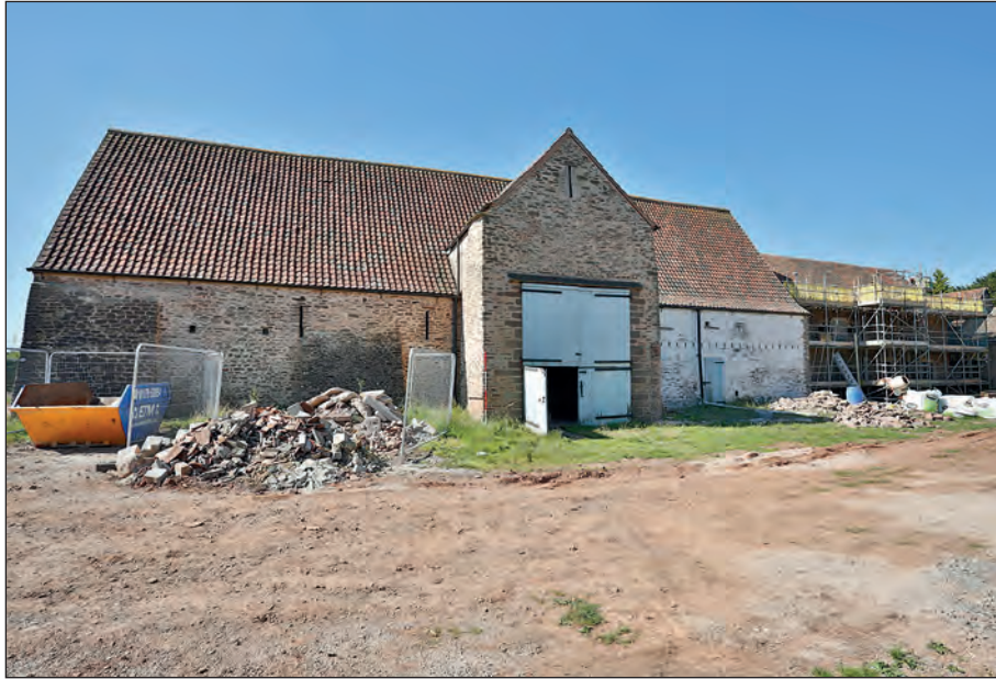
Plate 1: Main Barn viewed from north-east
