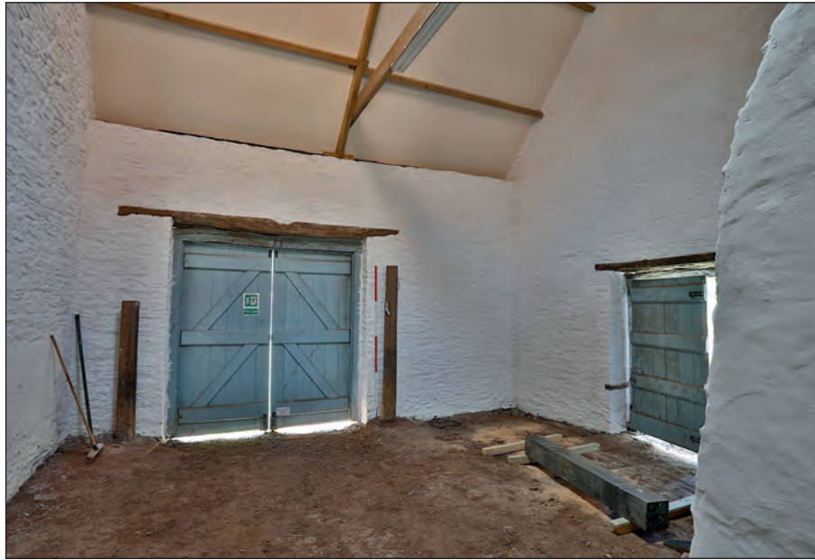
Plate 11: South Range west room interior
