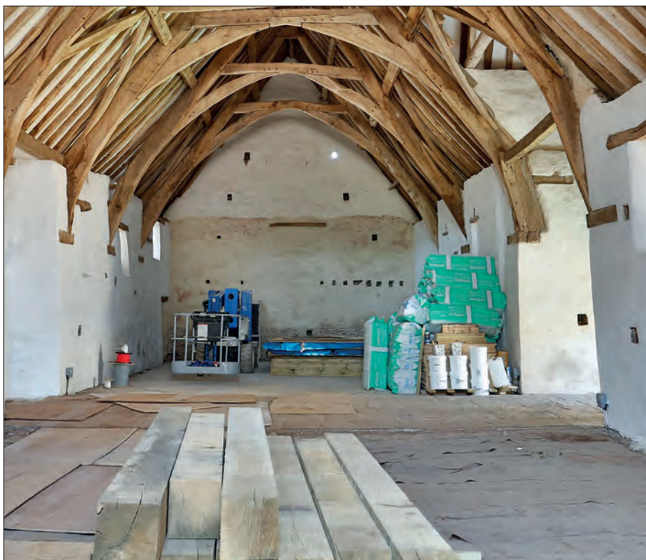
Plate 5: Main Barn interior centre and west end
