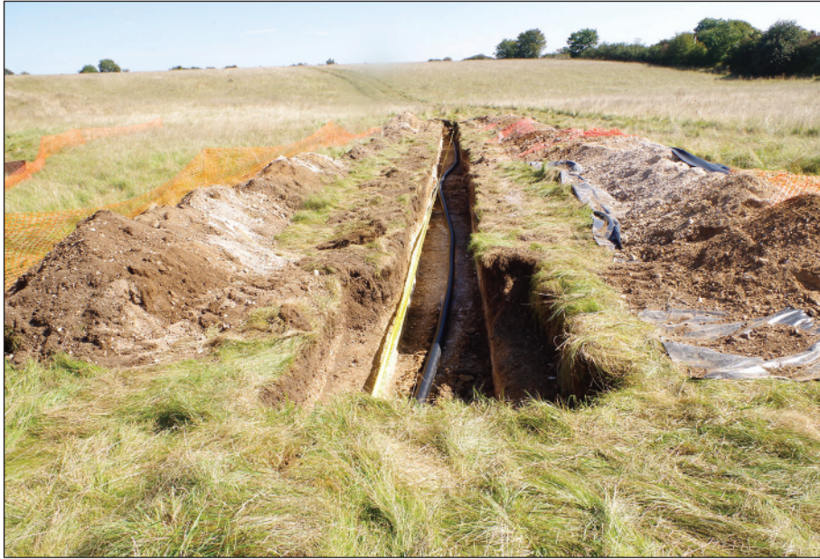
Plate 5: Trench 5 showing Roman Road, GRP 511, during excavation taken from the south-east
