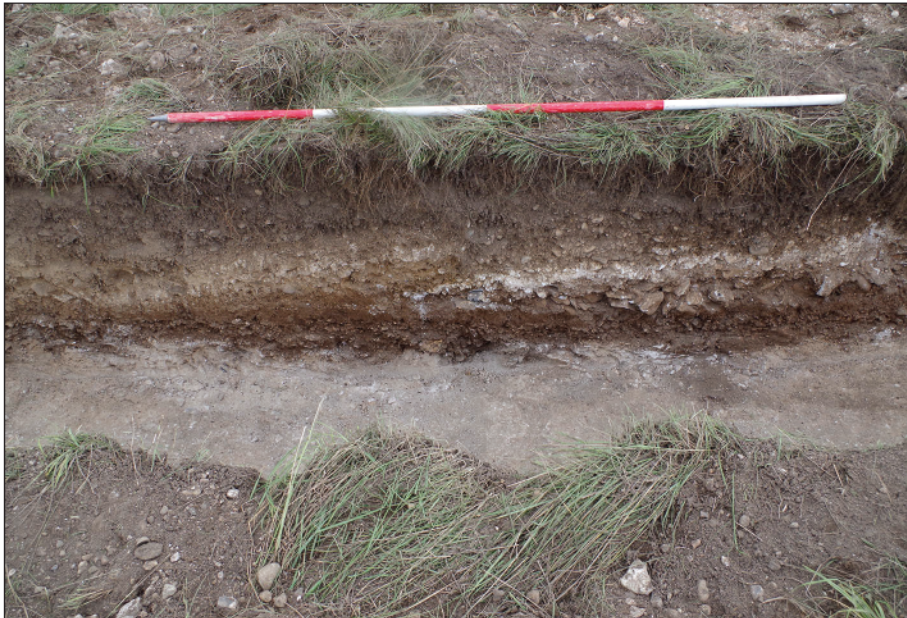
Plate 16: Section through Roman Road GRP 511, taken from the north, showing slumping. Scale is 2 m
