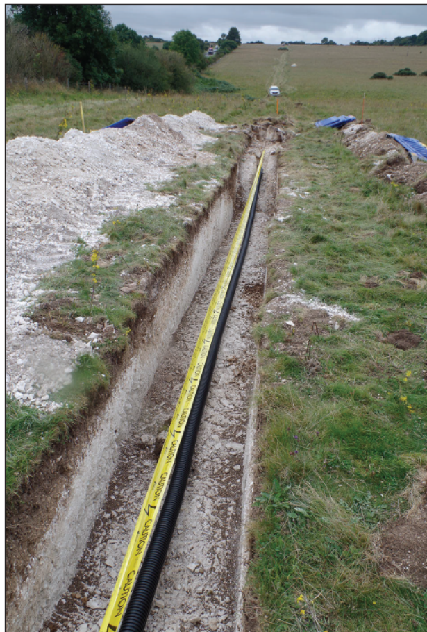
Plate 2: Trench 2 showing Grim's Ditch, 208, during excavation
