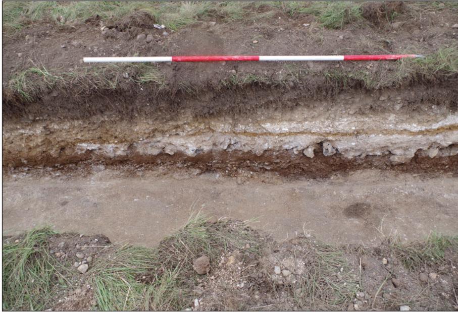
Plate 13: Section through Roman Road GRP 511, taken from the south. Scale is 2 m
