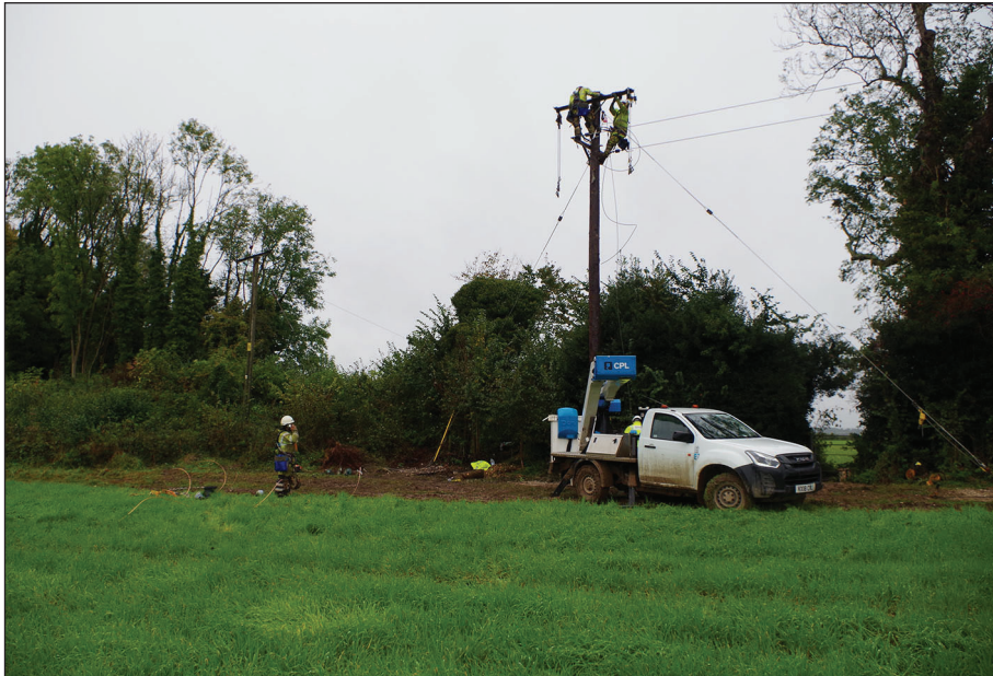
Plate 2: View of the site from the north-east during the works
