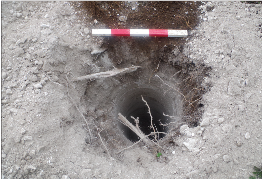
Plate 5: View of BH2, borehole for stay (1 x 0.50 m scale)
