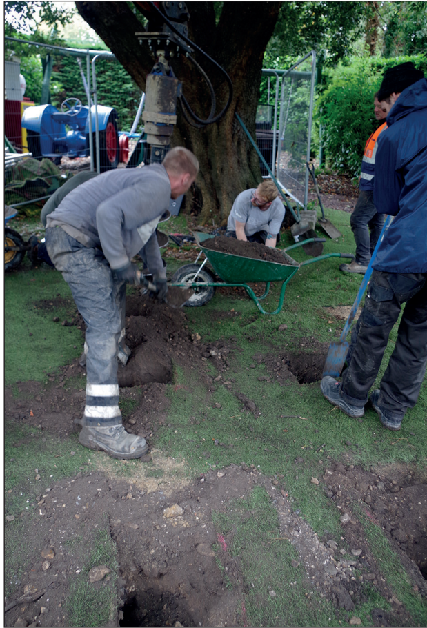
Plate 5: Working shot of hand excavation of pits.
