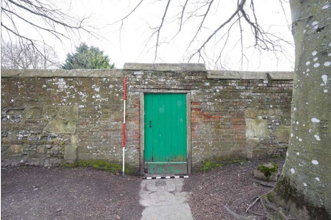
Plate 3: Doorway viewed from the west
