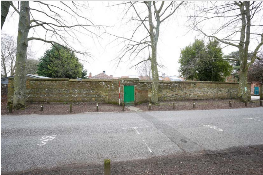
Plate 2: Wall viewed from the west
