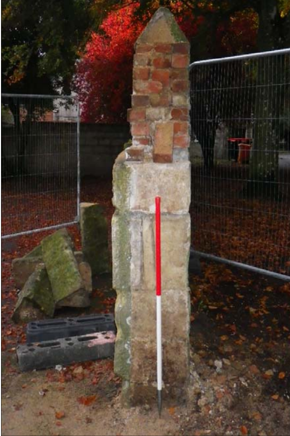
Plate 7: Detail of end of south section of wall following removal of blocking, viewed from the north
