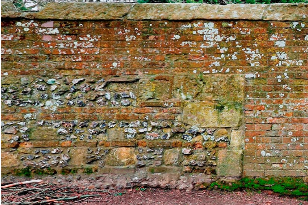
Plate 5: Detail of lacing courses on the west side of the wall to the north of the new emergency access
