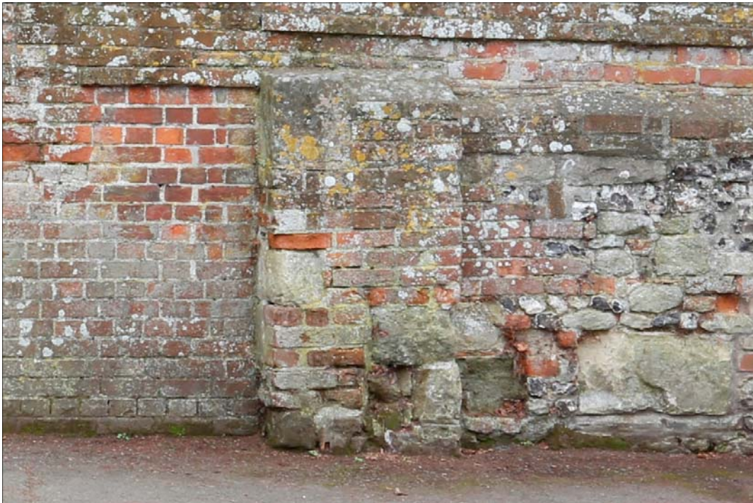
Plate 6: Detail of stone and brick buttress to the north of the doorway viewed from the east
