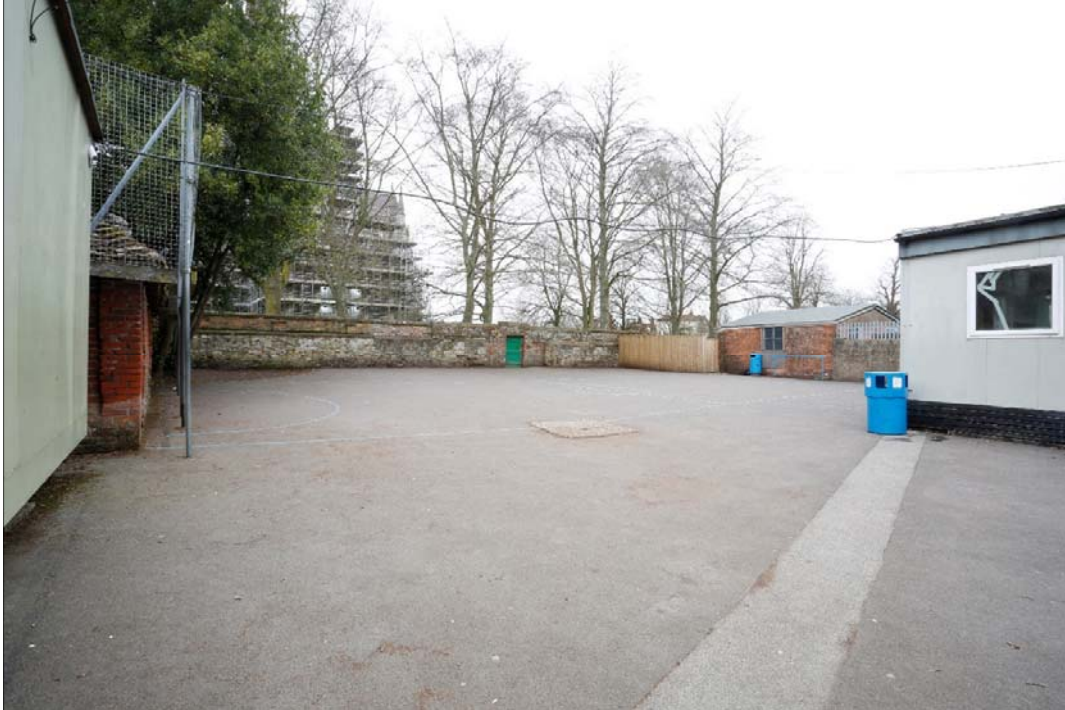
Plate 1: Wall viewed from the south-east across the school playground
