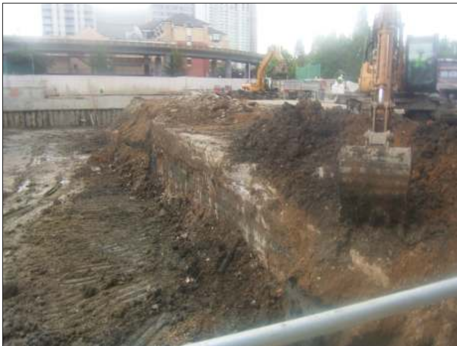
Plate 4: Working shot of walls from northeast
