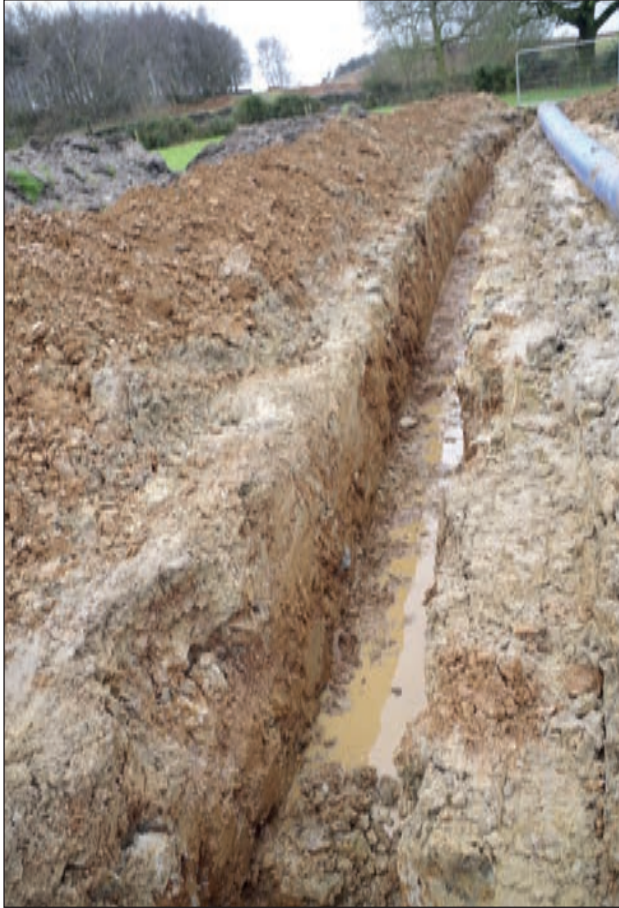
Plate 11: Open cut trenching, area 4 (1 m scale)
