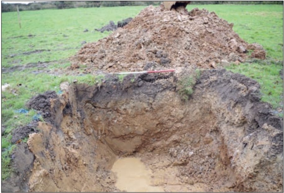
Plate 9: Drilling egress pit 2, north-facing section (1 m scale)
