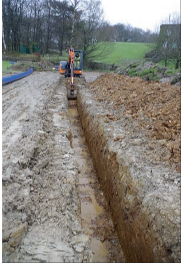
Plate 12: Open cut trenching, area 4, eastern end of scheme (1 m scale)
