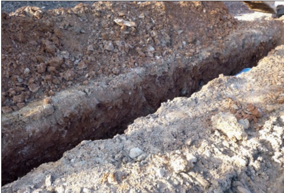
Plate 14: Open cut trenching, area 3
