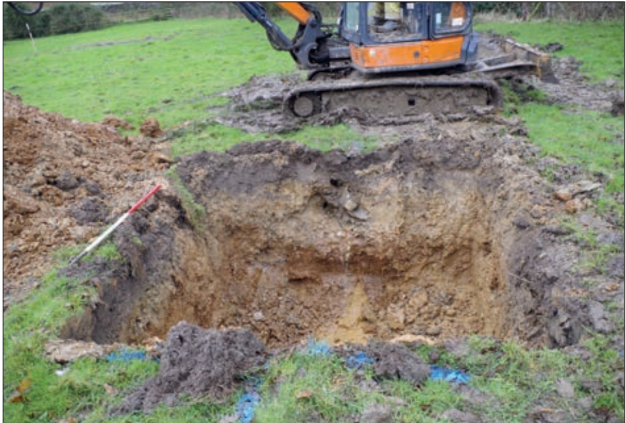
Plate 10: Drilling egress pit 2, plan view ( 1 m scale)
