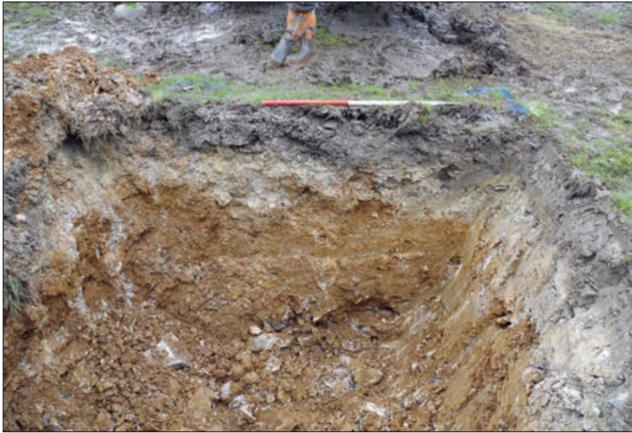
Plate 7: Drilling access pit 1, east-facing section (1 m scale)
