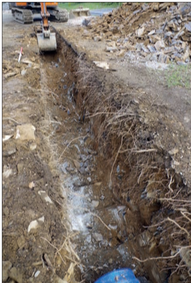
Plate 6: Open cut trenching, area 2-car park section (1 m scale)
