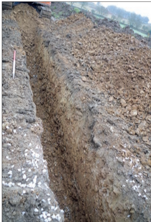
Plate 4: Open cut trenching, area 2-western end of scheme (1 m scale)
