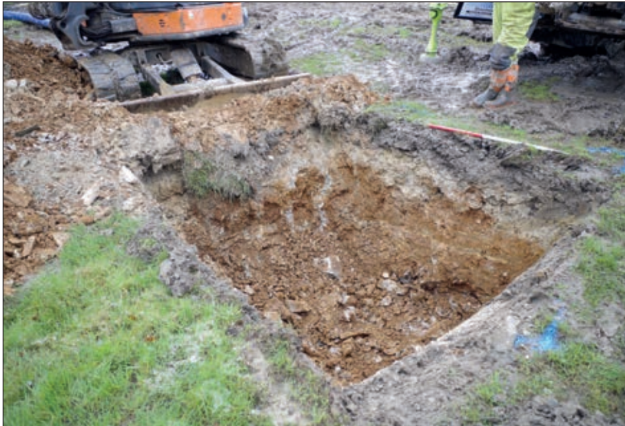
Plate 8: Drilling access pit 1, oblique plan view (1 m scale)
